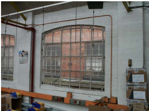
Plate 21: Factory extension: reused window from main factory building
