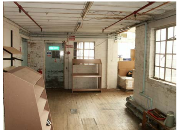
Plate 22: Utility block, first floor, looking north
