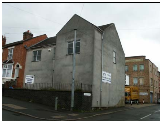
Plate 17: 41 Kettering Road, from west
