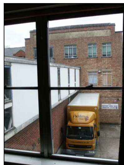
Plate 18: Office extension and bridge, from west
