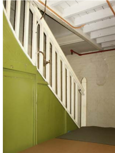
Plate 14: Main factory, central stairs
