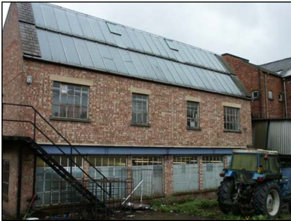
Plate 19: Factory extension, from north-east
