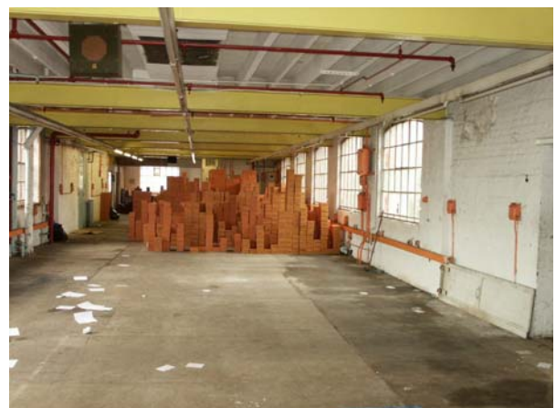
Plate 12: Main factory interior: first floor, rear wing
