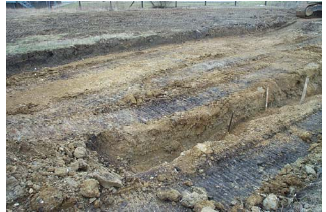
Plate 2: Area stripped of contaminated soil
