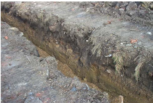
Plate 3: General view of the drainage trench
