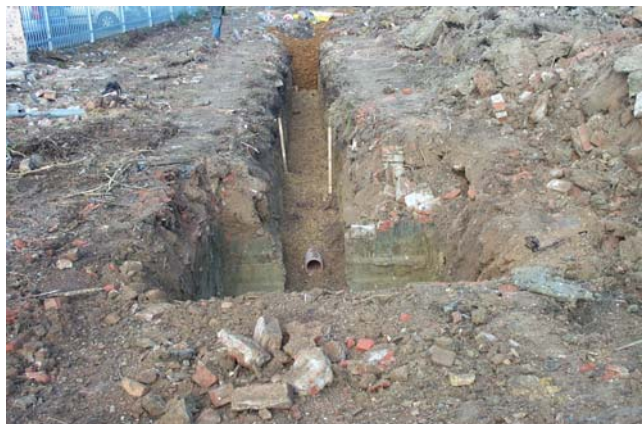
Plate 4: General view of the drainage trench
