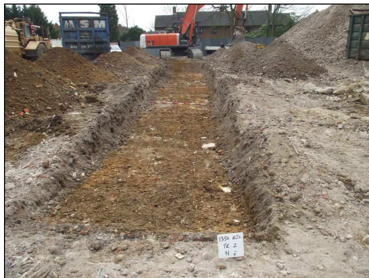
Plate 3: General view of Trench 2 looking south
