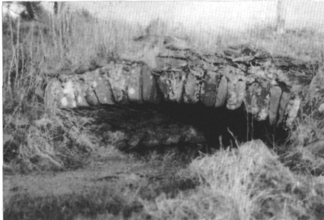
Fig 28. Bridge over Barmore Cut at entrance to Ardscaipsie Farm (NS 050 583). (see p 67)
