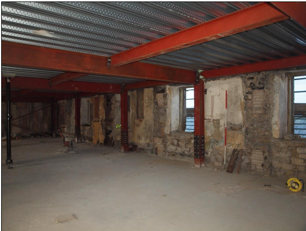
Plate 53: First floor following floor insertion with blocked openings, possibly flues, in wall scars to north wall
