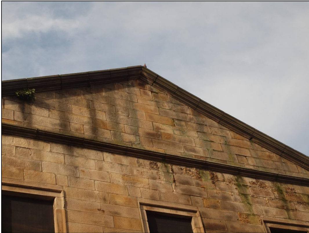
Plate 15: Apex of gable showing moulded coping
