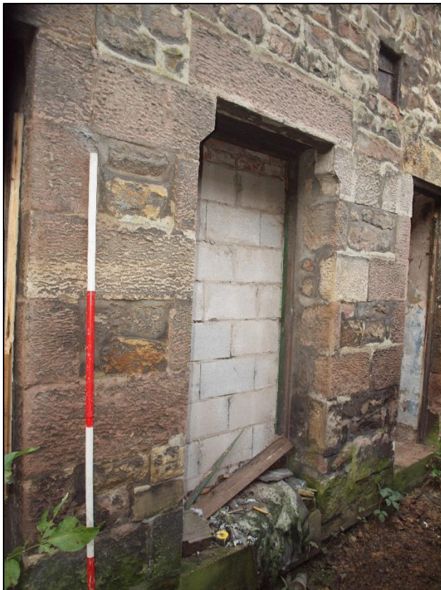
Plate 20: Blocked 'Caernarfon' doorway with corbelled lintel and blocked ventilation hole above
