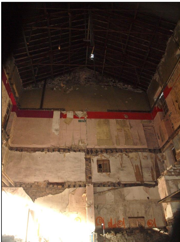
Plate 40: West wall showing first floor window and second floor doorway
