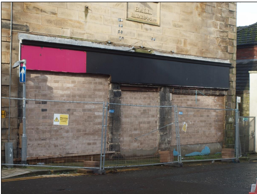
Plate 12: Ground floor blocked openings with scar of portico over central doorway
