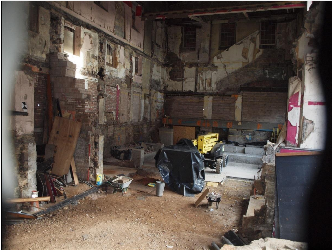
Plate 33: General shot of interior showing wall stubs (former party walls) extending from basement to first floor level
