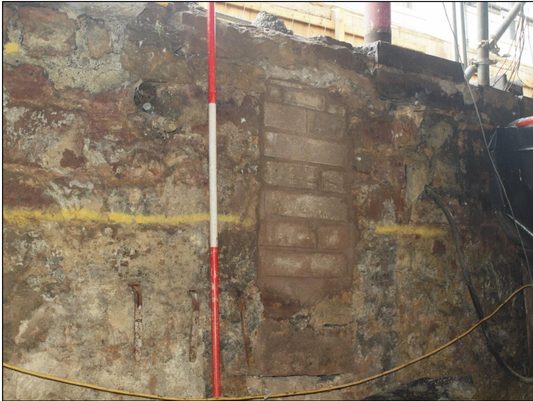
Plate 48: Blocked cellar opening to south wall
