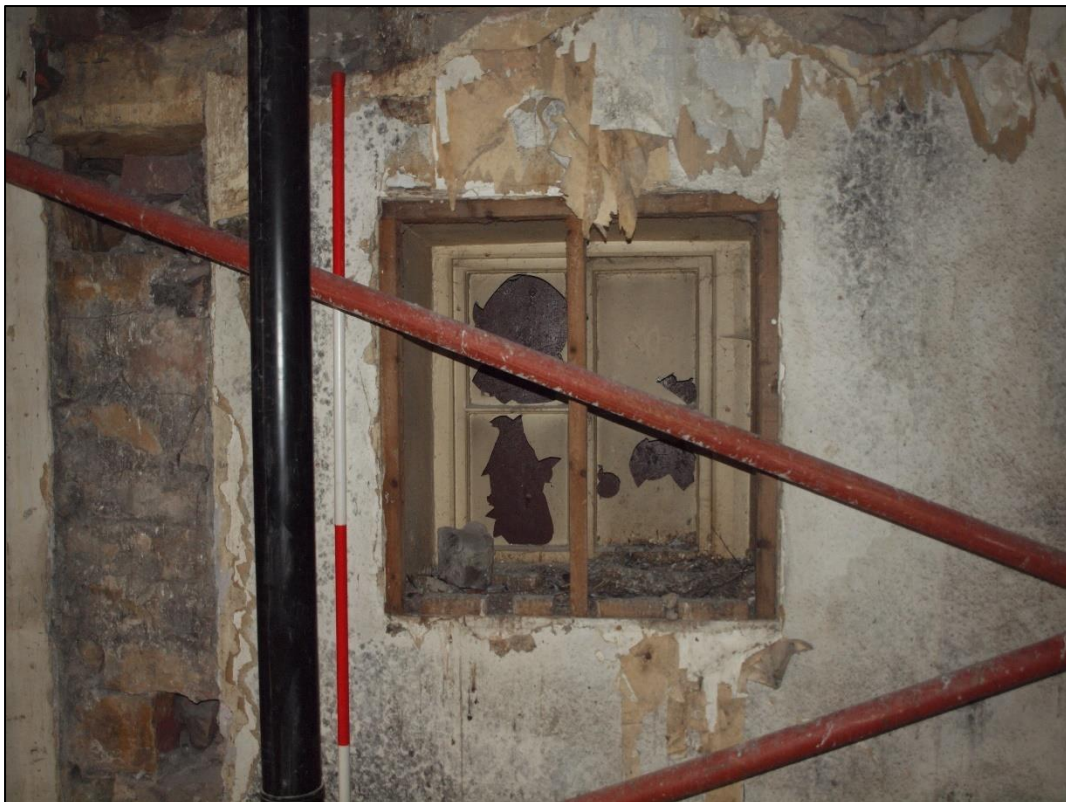
Plate 59: Window to west wall with wall scar to the left
