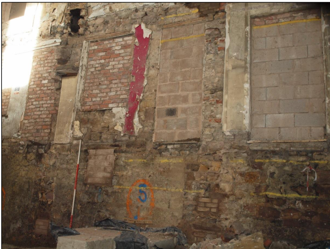
Plate 45: Blocked ground floor openings to eastern end of north wall and blocked cellar light
