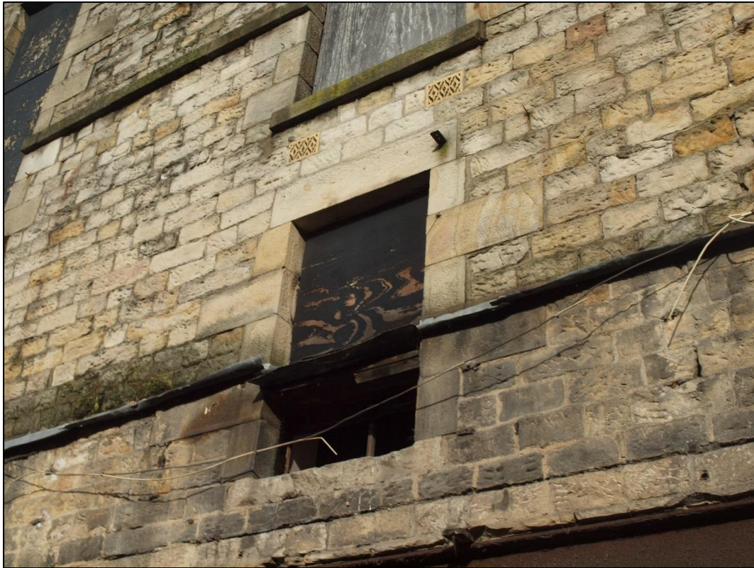
Plate 9: First floor window to west side without blocking showing even and consistent yellow colour of stonework and metal vents
