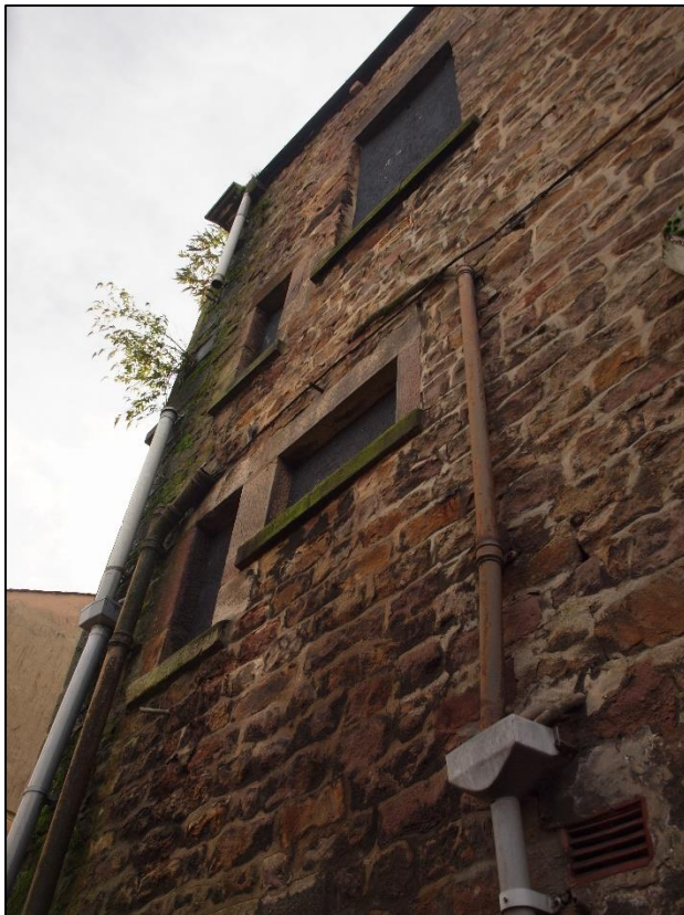
Plate 18: First and second floor windows at eastern end with large square sandstone jambs and inserted modern vent above ground floor doorway
