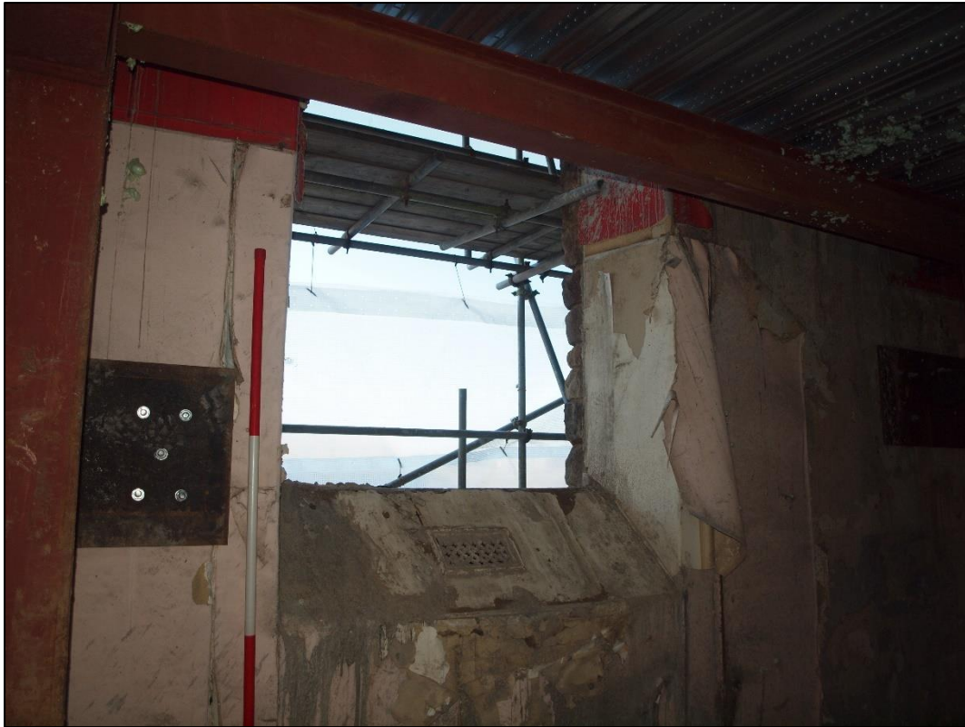
Plate 62: Northern window showing cast iron ventilation grill
