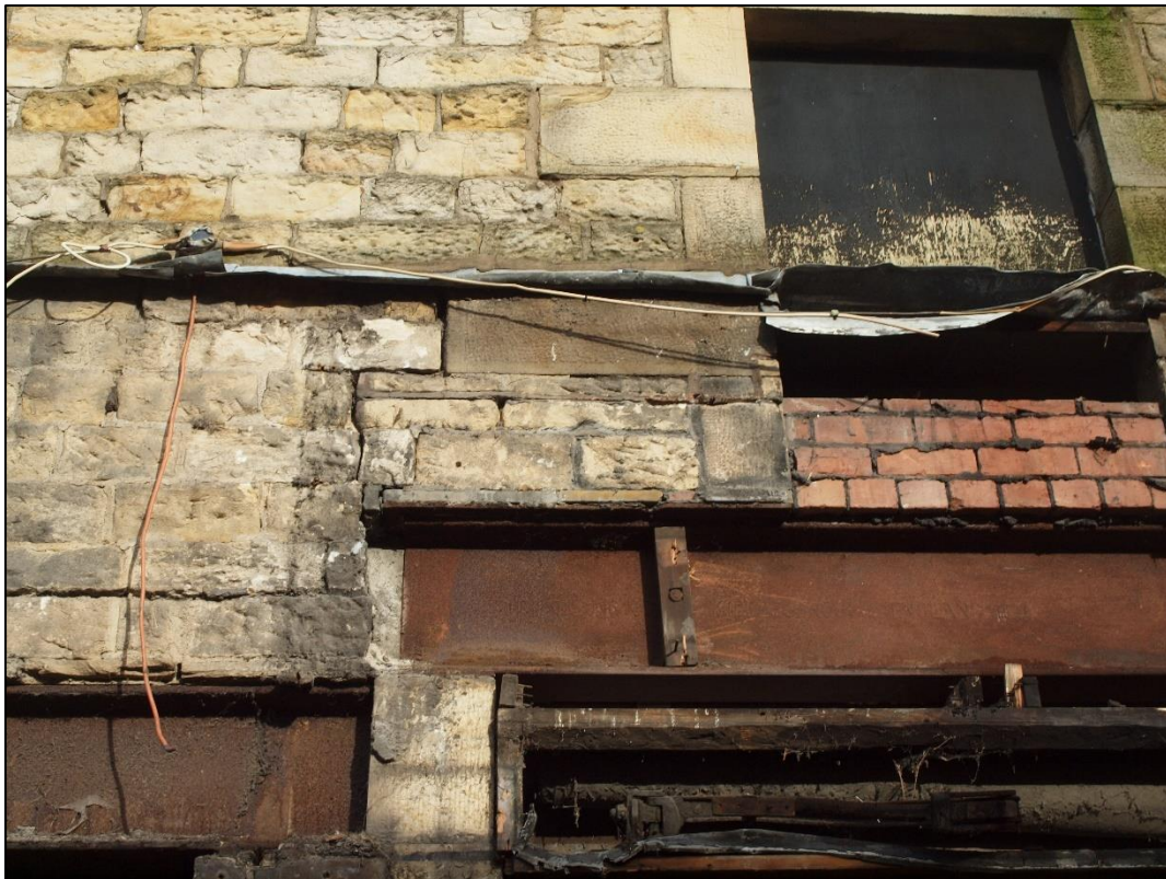
Plate 6: RSJ lintels of openings to centre of south face
