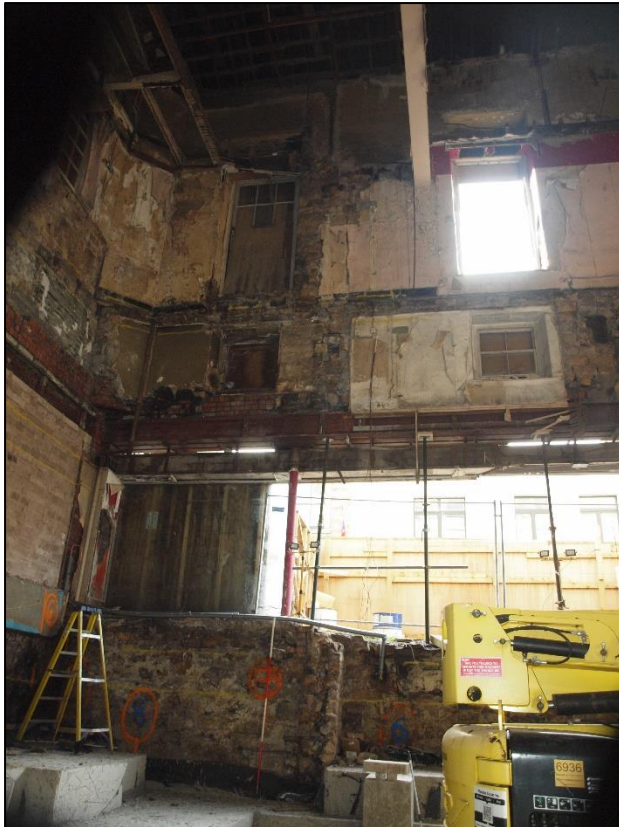
Plate 46: Eastern end of south elevation with chamfered corner chimney and scantling framework
