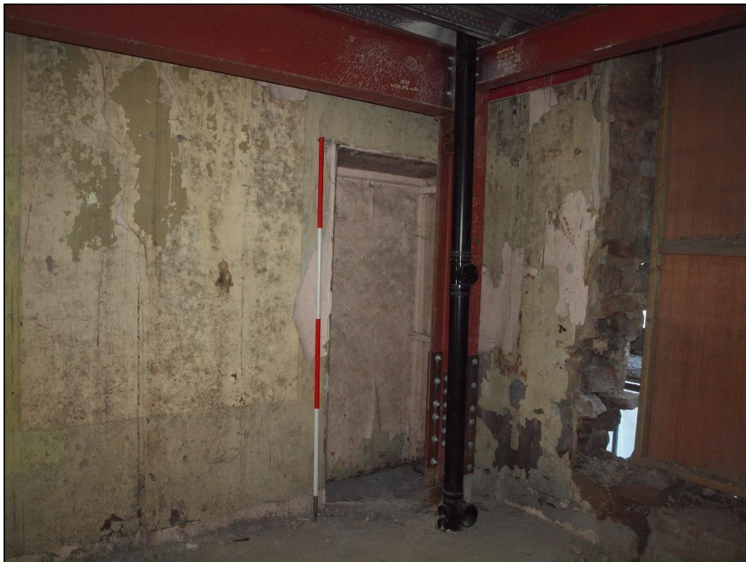
Plate 61: Blocked doorway at northern end of west wall
