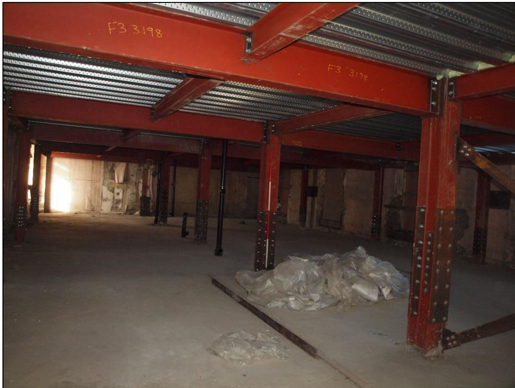
Plate 60: Second floor following floor insertion
