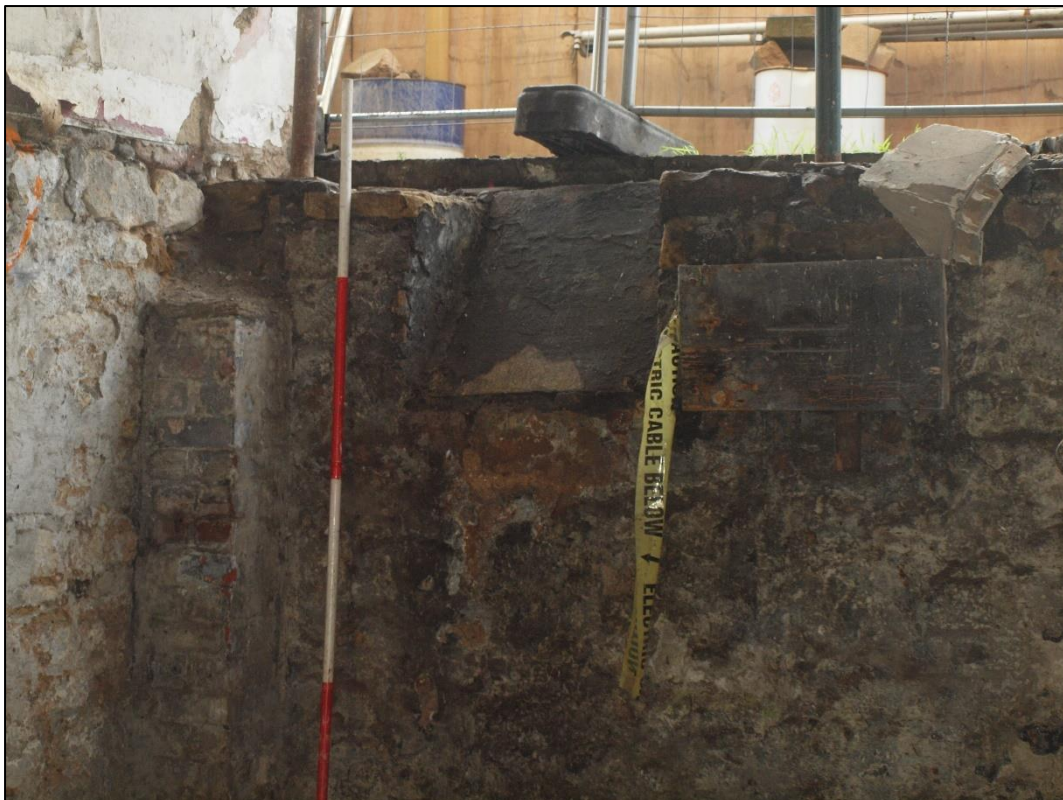
Plate 49: Chamfered opening of cellar light
