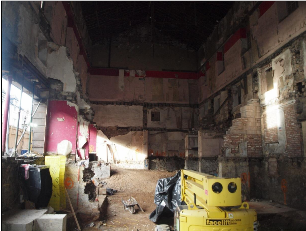
Plate 37: General shot looking west showing scar of former spine wall
