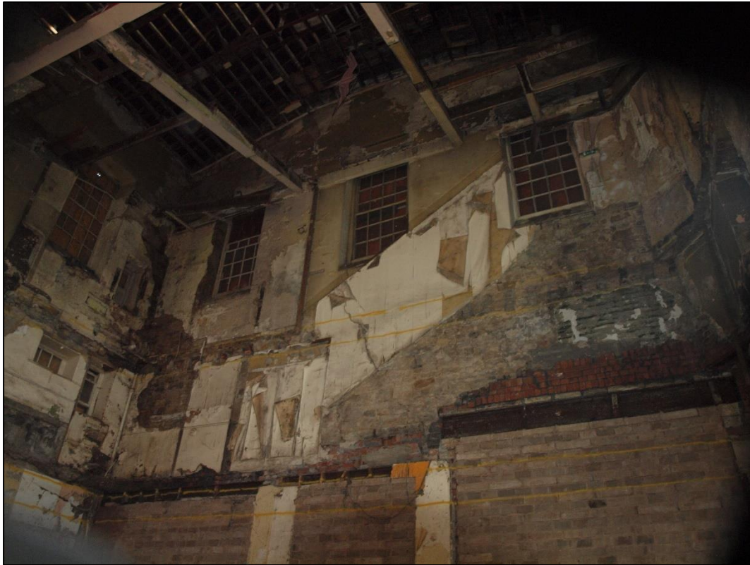
Plate 39: Ghost of staircase cutting across second floor windows to east wall and scantling timber of former gallery
