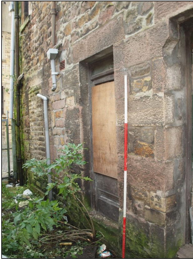
Plate 19: Doorway blocked internally with timber door remaining
