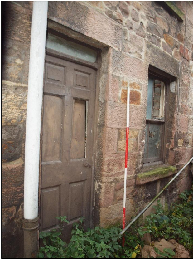
Plate 23: Timber 6-panel door with horizontal fanlight; 2 over 2 sash window adjacent with blocked cellar light below
