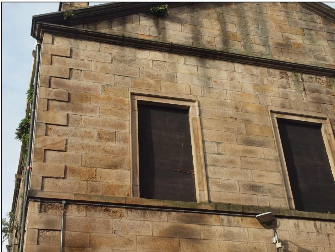
Plate 14: Second floor windows with moulded string course above to represent base of portico; wraps around end of wall.
