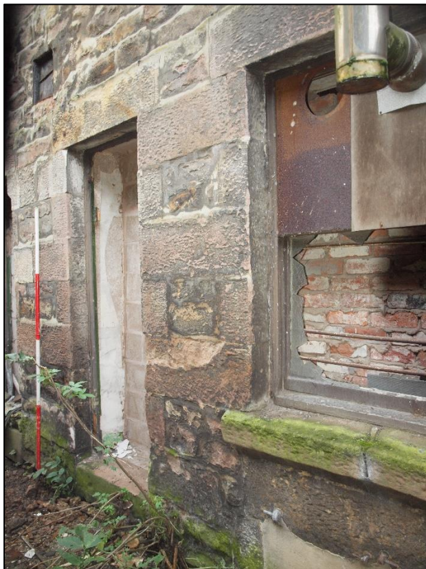
Plate 22: Doorway with adjacent window and blocked cellar light below
