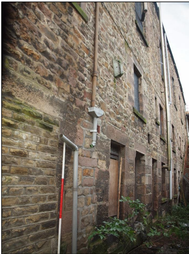
Plate 16: North elevation with coursed squared rubble walling and stone colour variable from yellow to buff to pink.
