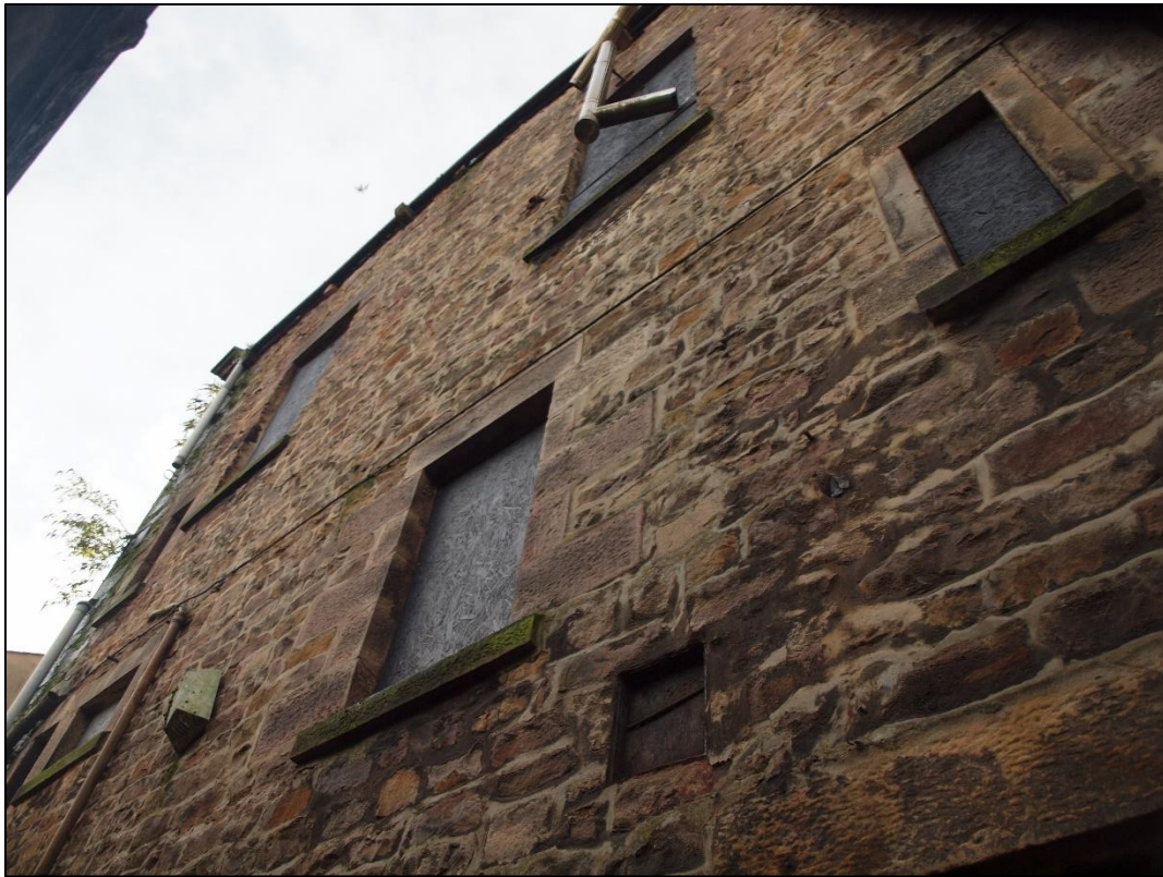
Plate 21: First and second floor windows showing difference in first floor window jambs
