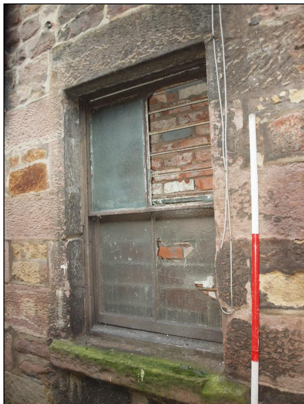
Plate 28: Sash window blocked internally
