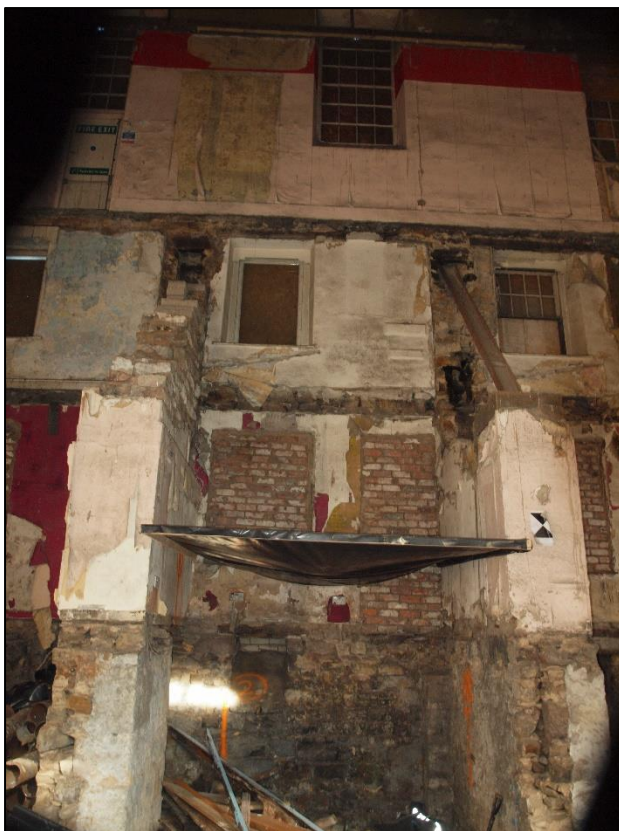
Plate 43: Blocked ground floor openings and first floor windows to north wall with blocked cellar light below
