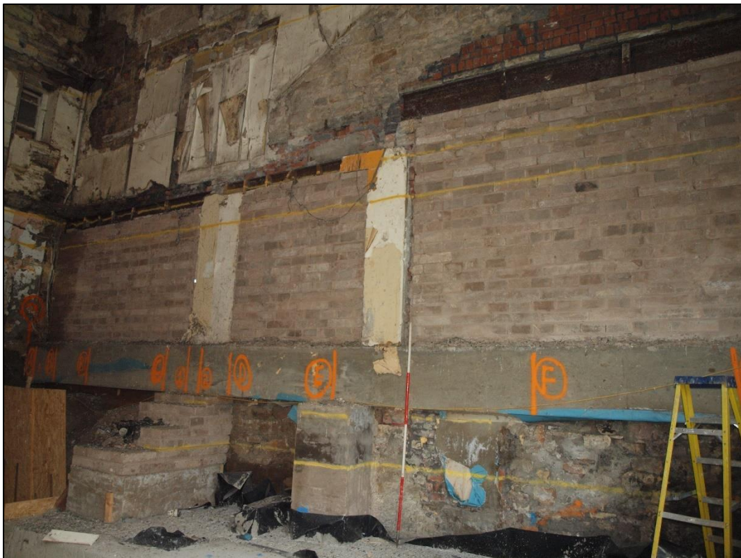
Plate 38: Modern locked openings to east gable
