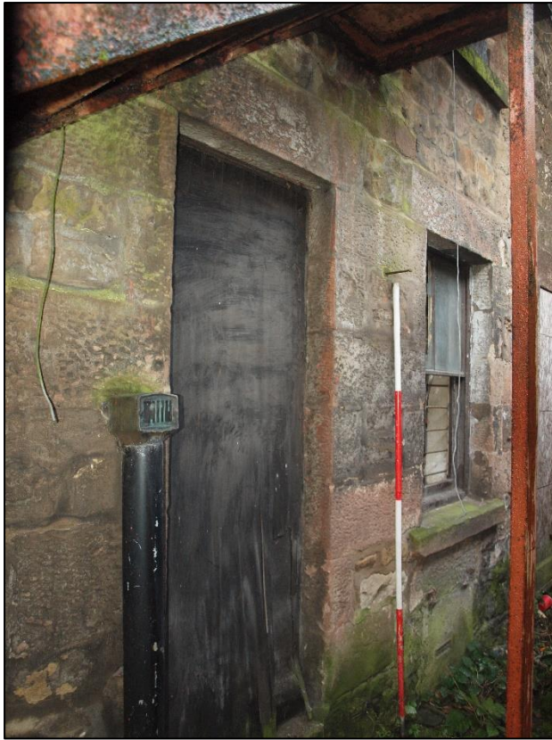
Plate 29: Blocked doorway and window with blocked cellar light below
