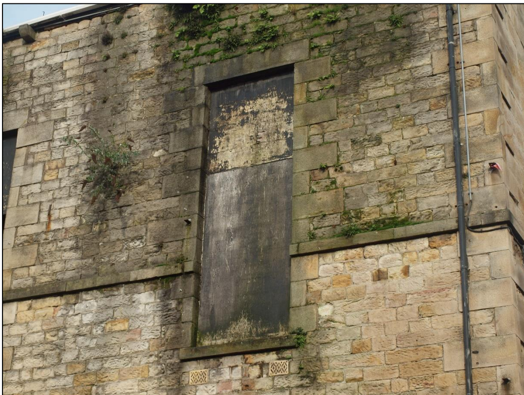
Plate 10: Second floor window detail at east end of south face, extending through string course. Metal vents below and gutter cut through string course
