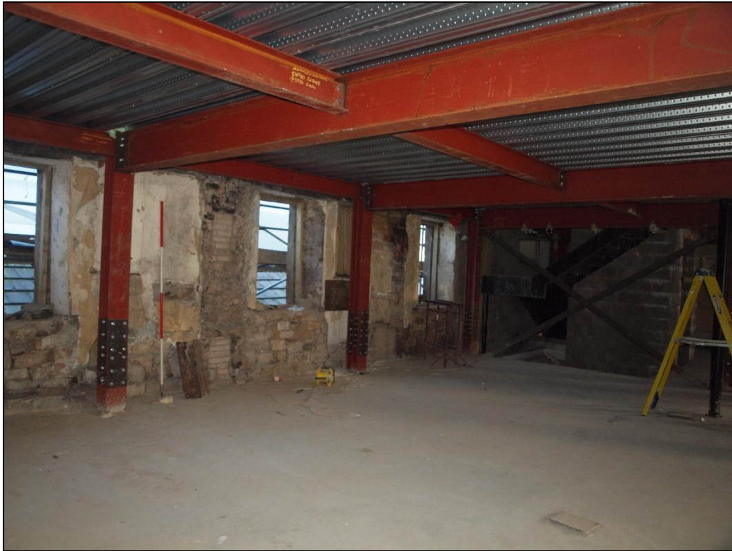
Plate 54: North wall of first floor following floor insertion
