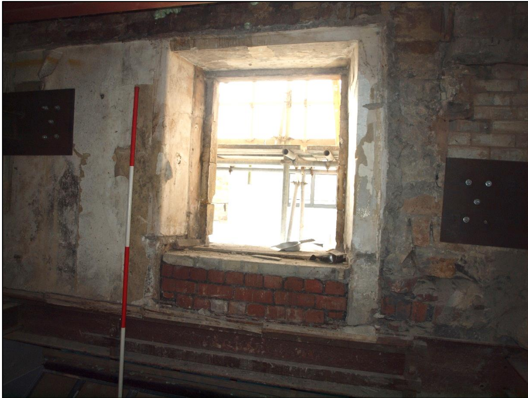
Plate 56: Window to south wall with partial blocking
