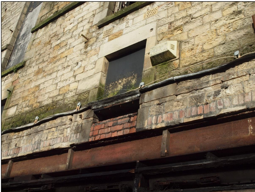
Plate 8: First floor window with partial blocking and metal vents above
