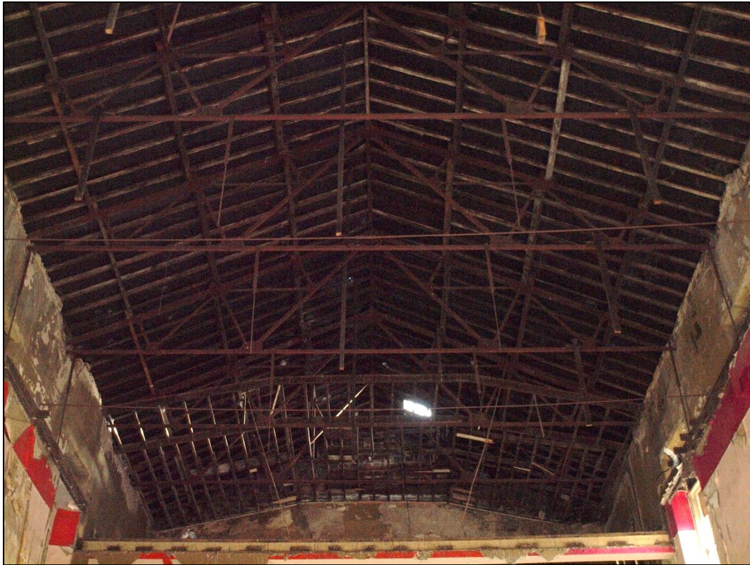
Plate 41: Roof detail showing trusses and arched ceiling remains
