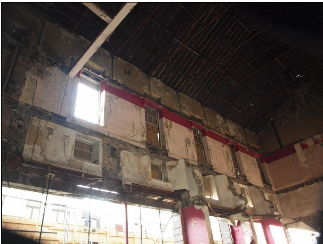
Plate 47: First and second floor windows to south elevation with metal fittings for second floor suspended ceiling cutting the top of the windows
