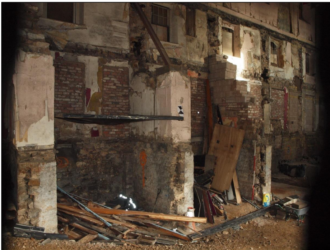
Plate 34: Stub walls and blocked openings to north wall
