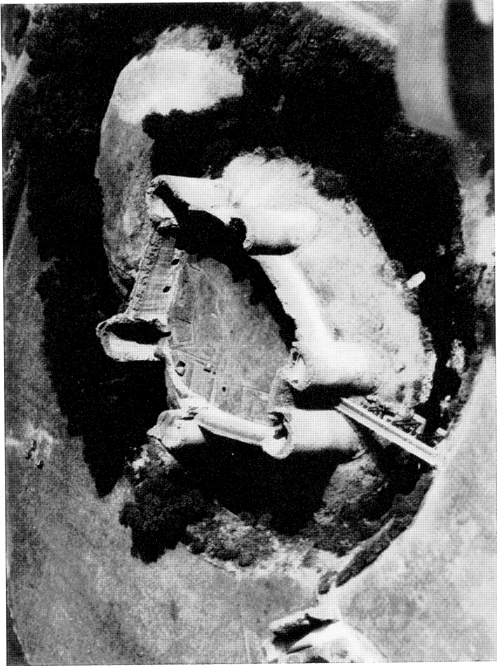
WHITE CASTLE, MONMOUTHSHIRE Aerial view of inner ward from NW. showing, on far side, foundation of square keep underlying later stretch of curtain wall. (p. 171)
