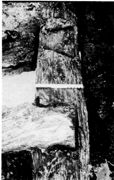
B. Detail of dovetail joints at the S. end of the wheel-pit. Scale 30 cm
