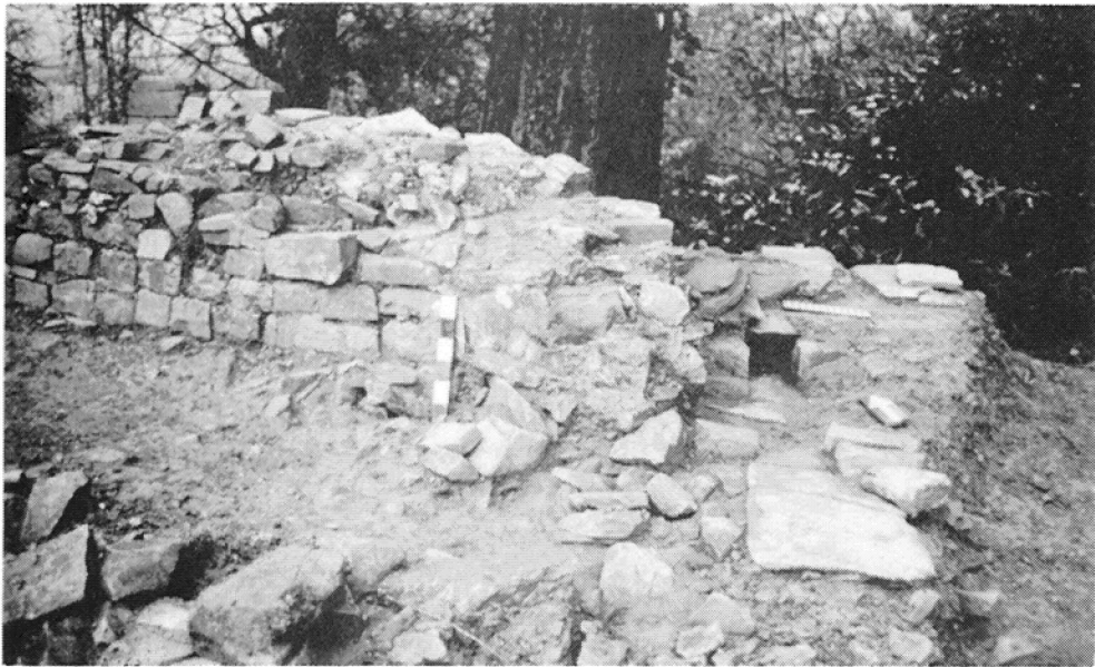
B. NE wall of Period VI hall, Building H, pierced by a drain RUMNEY CASTLE
