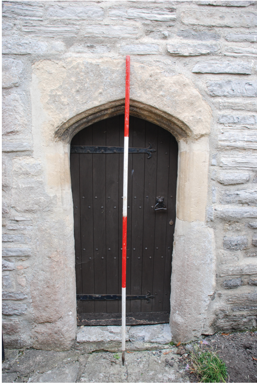
Plate 3 The south doorway, looking north.
