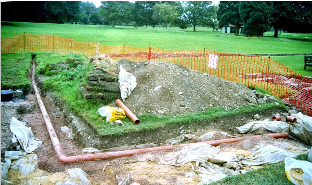
Photograph 39. The new plastic pipe installed. The archaeological layers are protected with plastic sheets and cushioned with sand. The new pipe is bedded on, and covered by, sand and gravel.
