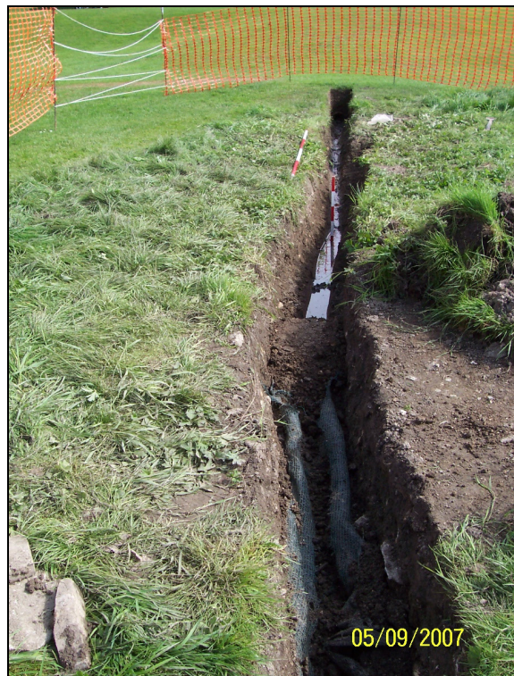
Photograph 35. Clay pipe drain trench looking E. The pipes have been removed and a small dam holds the water back from the trench.
