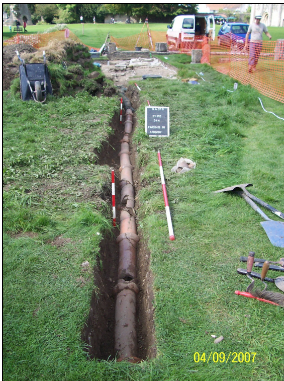
Photograph 34. Clay pipe drain looking W. Showing breaks and holes in the pipes.
