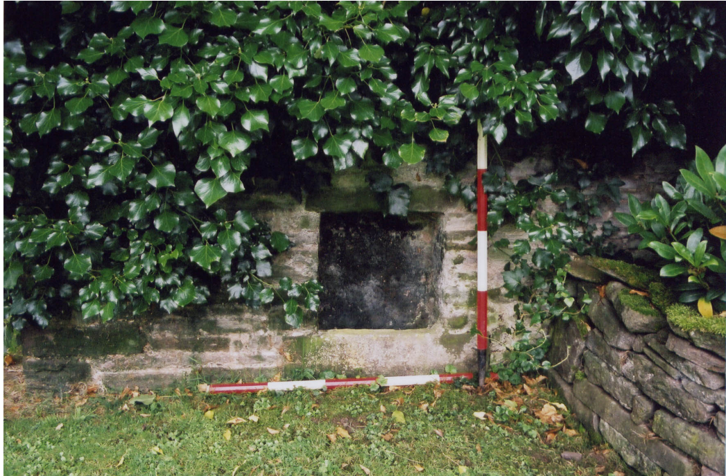
Plate 8: Stone opening for feeding chute, as seen from the garden
