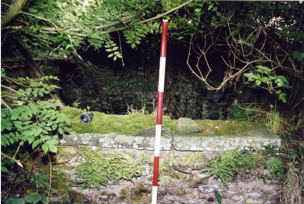
Plate 2: Coping stones on wall of southern stone pig pen
