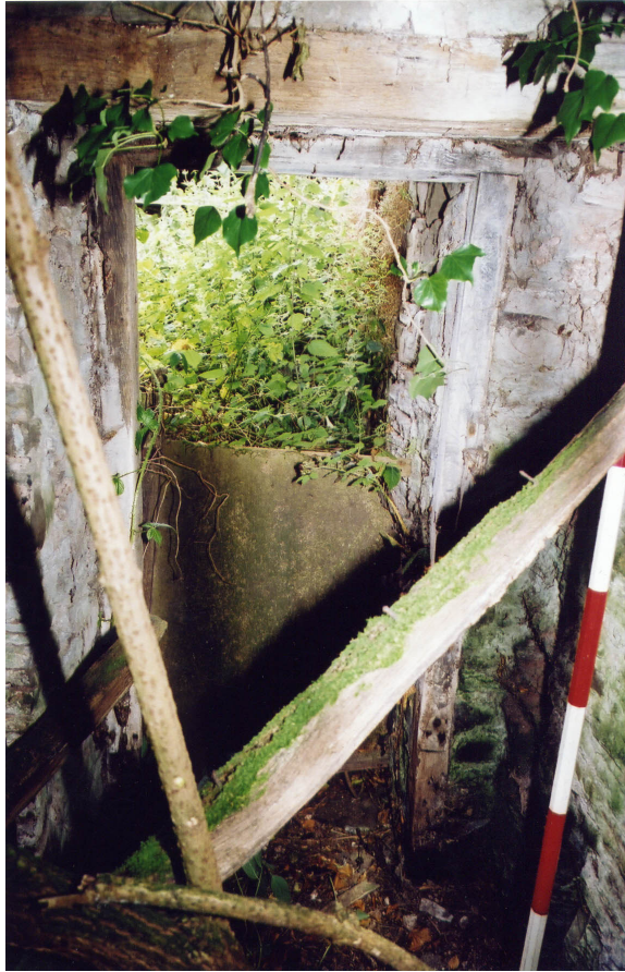
Plate 3: Timber-frame doorway into the old pig pens
