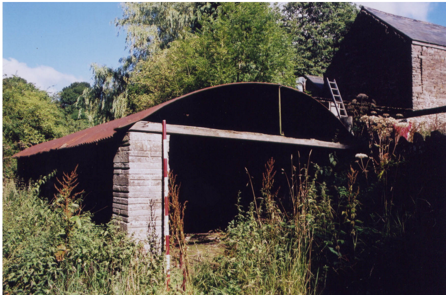
Plate 6: Modern pig pen with curved tin sheeting roof
