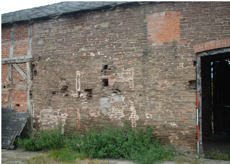
Figure 12: Photograph showing the change in brickwork where the roofs of both the timber-framed barn (1) and the stone barn have been raised
