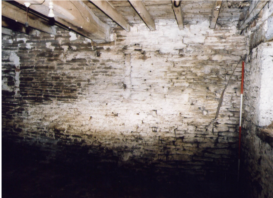
Figure 13: Whitewash and plaster present in the lower level of barn (2)
