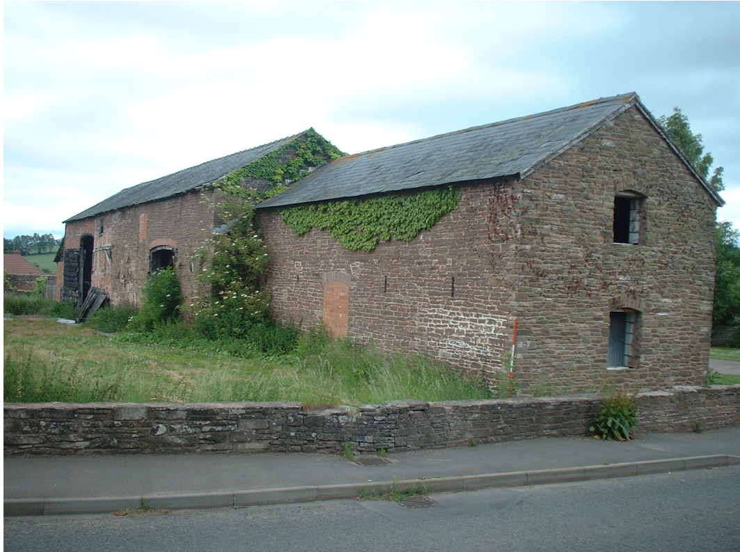
Figure 15: View of the barns from the opposite direction, with later stone building (3) in the foreground
