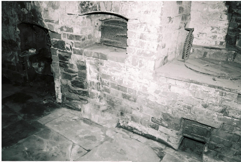
Plate 7: The baking oven and copper wash pot on the north side of the stack
