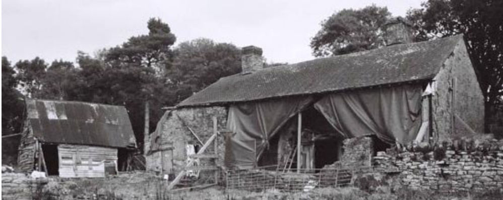
Plate 3: The west elevation of the house while under reconstruction
