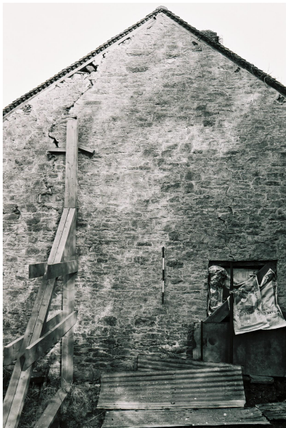
Plate 1: The south gable wall with wooden support.
