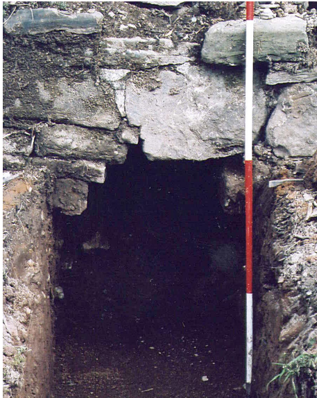
Plate 12: Example of pits dug for the underpinning of the walls
