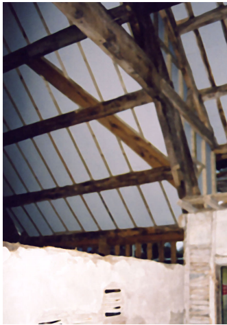
Plate 14: Passing wind brace in the restored roof at Pound farm
