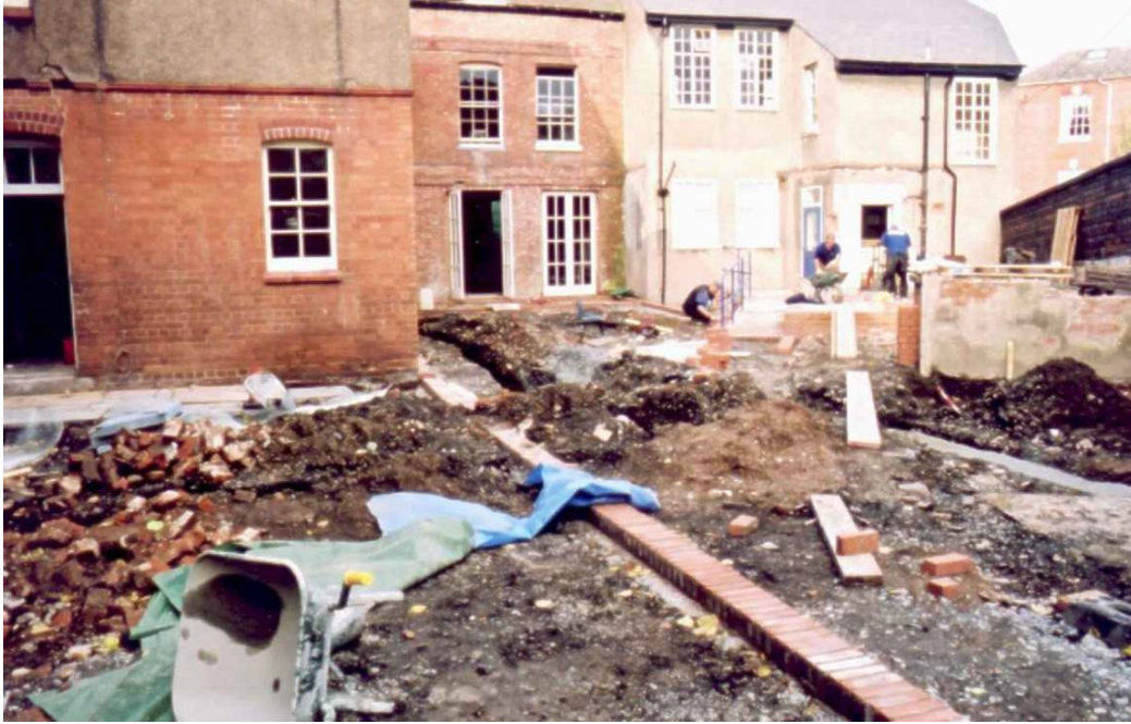
Plate 1: General view of Choir House yard during construction work
