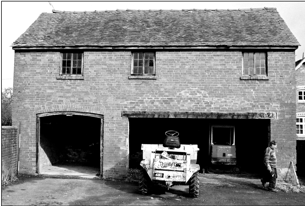
Plate 1: The southern elevation of the building
