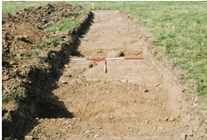
Plate 2: Service pipe in trench 4
