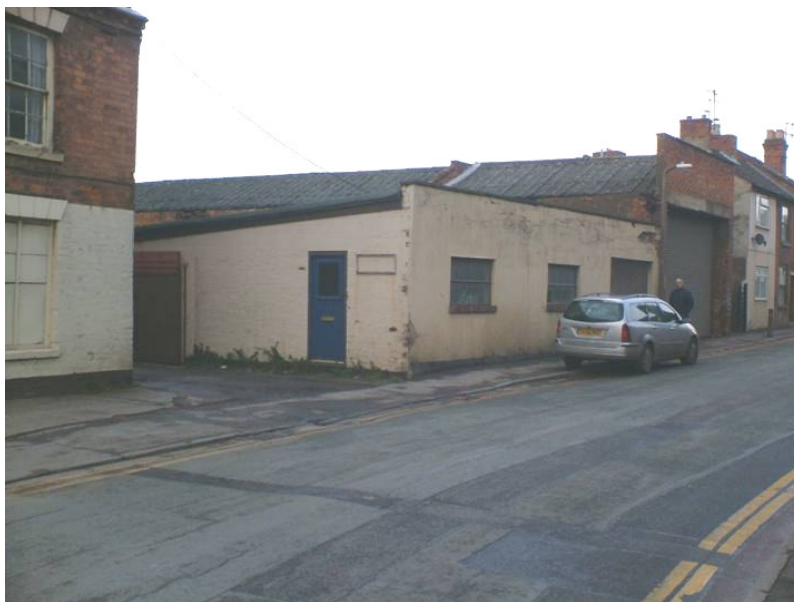
Plate 13: The front elevation of building E
