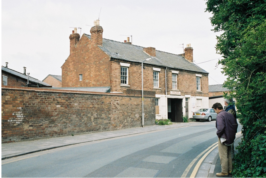
Plate 1: Numbers 48 to 52 from the southeast. Number 48 lies to the left. Note the ginnel between Numbers 50 and 52.
