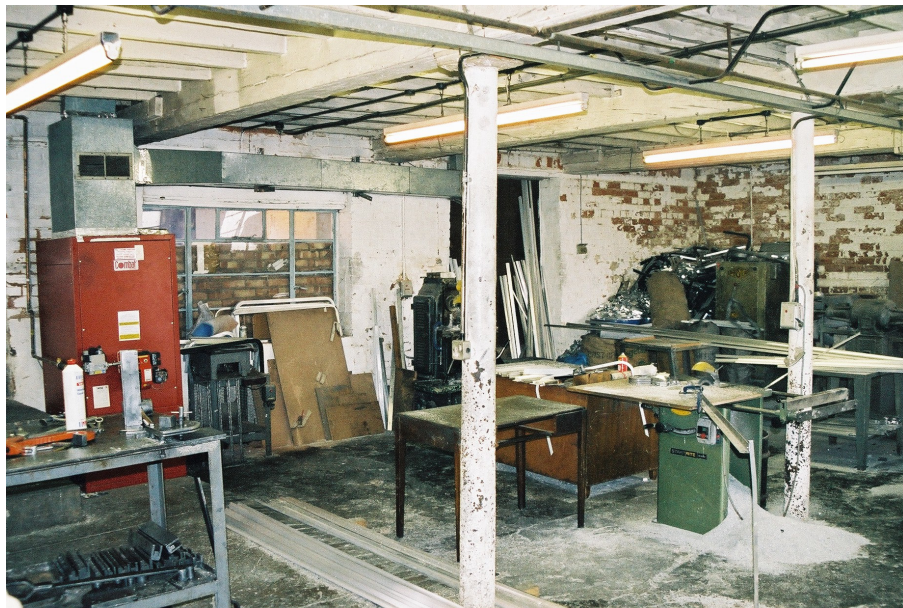
Plate 9: The ground floor of Building B showing cast-iron pillars
