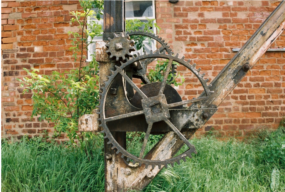
Plate 7: The fixed-jib crane of around 1815
