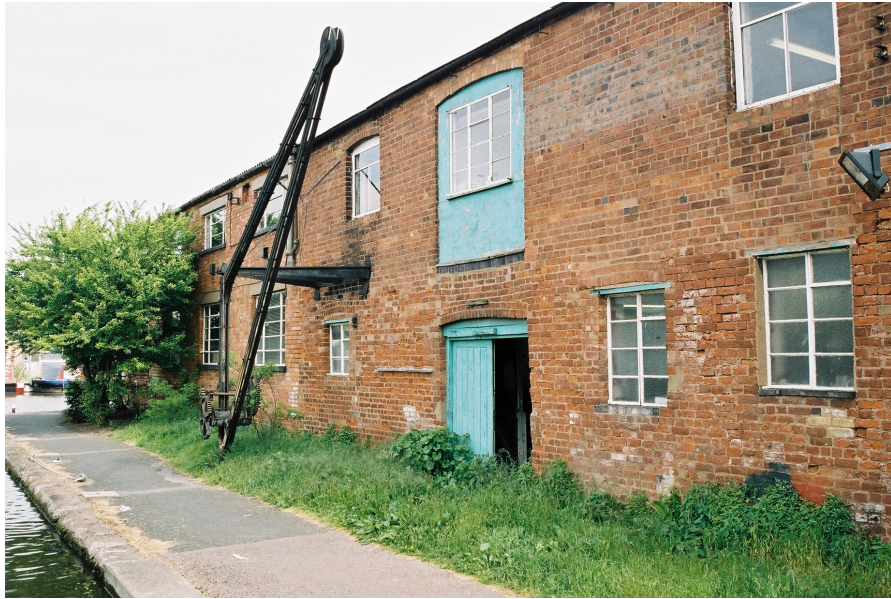
Plate 8: The canal front of Building B
