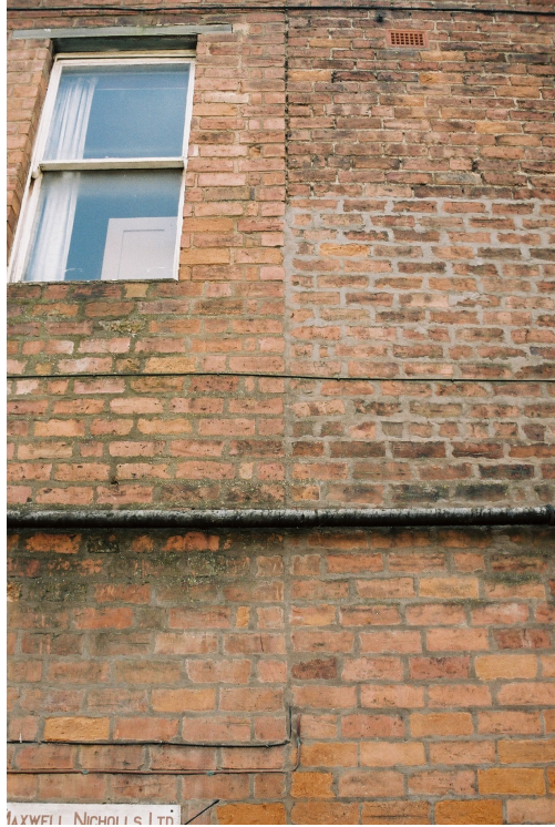
Plate 4: Building break between Number 52 and the annex (on the right)
