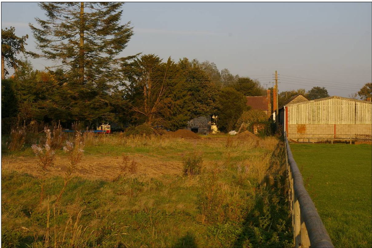
Figure 6 : Photograph of the site with trench 1 and 2 open, looking West, from the back of the plot towards Oakwood.
