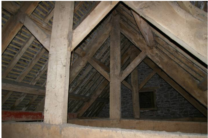
Plate 87 – SMR No: 55694 – the roof supported by king post trusses with angles struts (55694)
