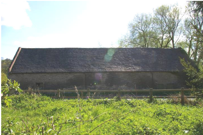
Plate 86 – SMR No: 55694 – the north elevation; the large blocked entranceway can be seen in the middle (55694)
