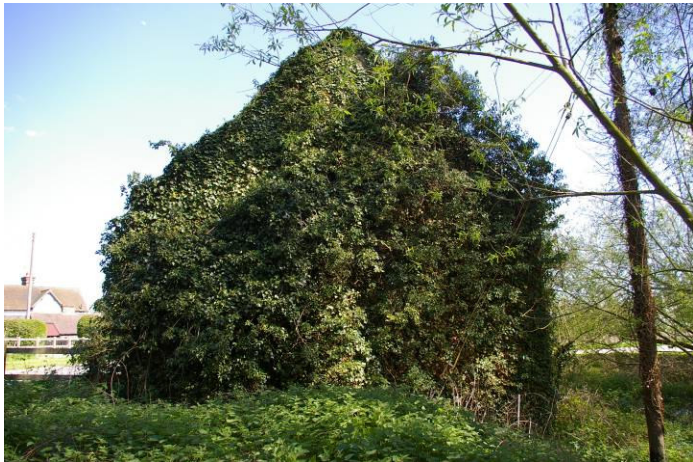
Plate 85 – SMR No: 55694 – the west elevation showing the vegetation that is causing damage to barn (55694)
