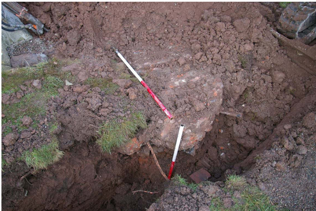
figure 23: brick soakaway with concrete capping, looking south-west
