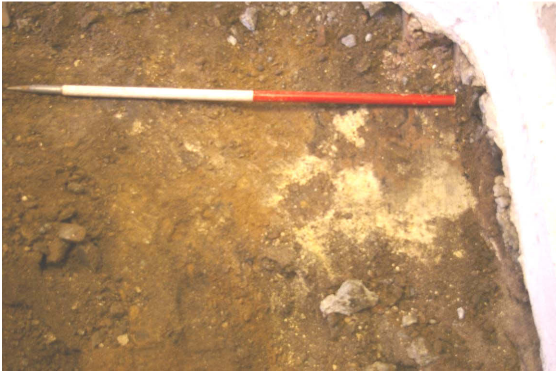
figure 13: area of mortar flooring (3) in the north-west of the church tower, looking west
