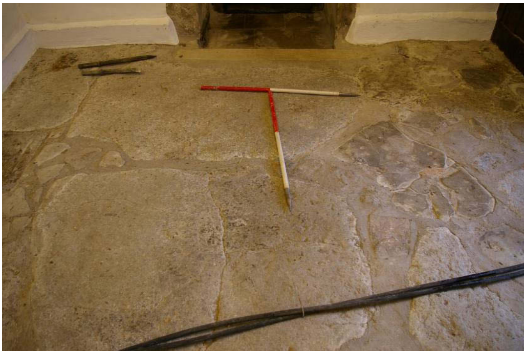
figure 7: concrete floor of church tower laid in 1990 before work began
