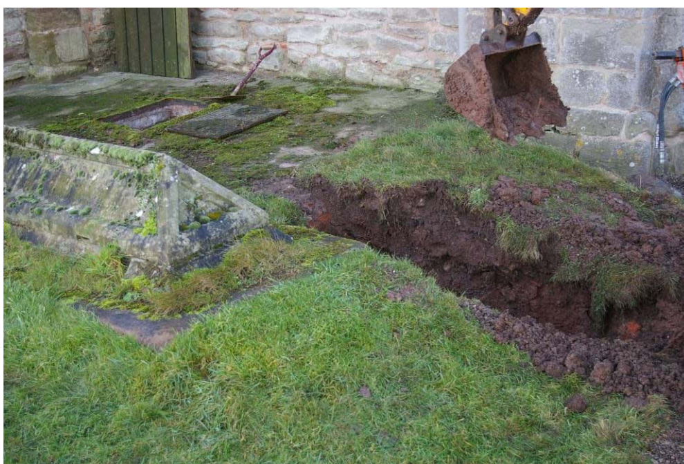
figure 22: excavation of the trenches from the basement to the footpath
