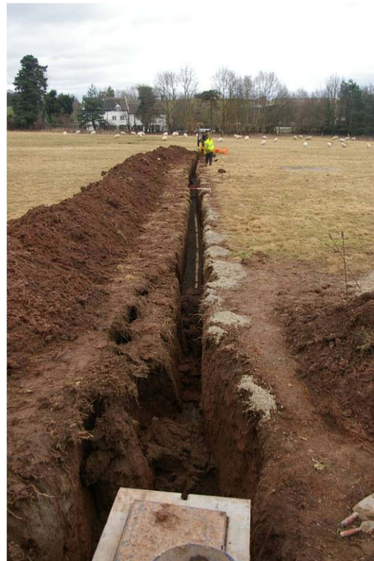
figures 32 and 33: excavation of trench in field north of graveyard in progress; full length from concrete manhole to connecting mains manhole
