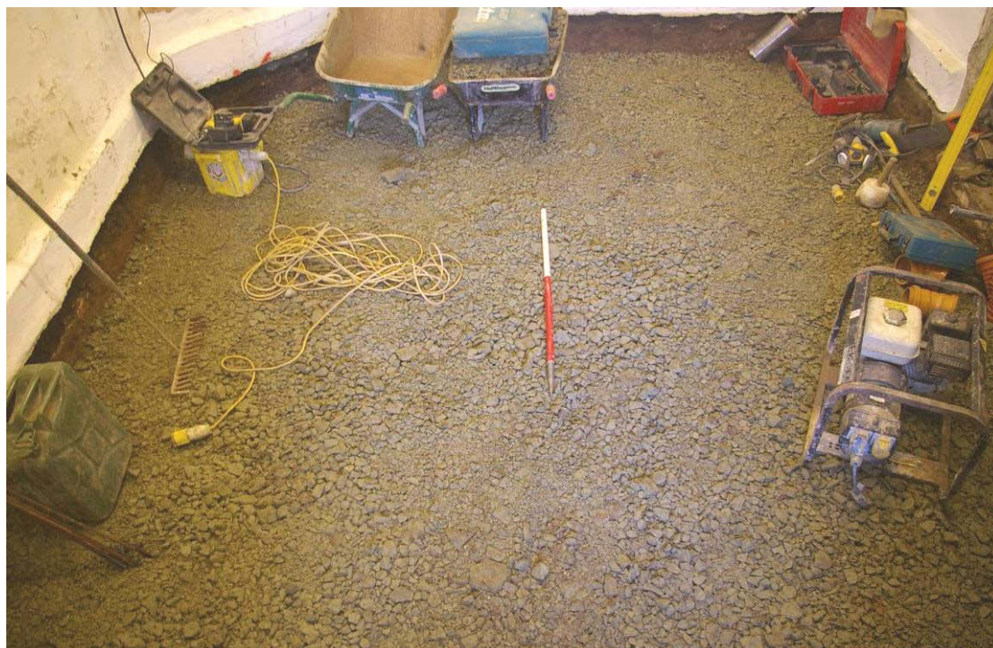
figure 17: tower floor re-levelled before concreting
