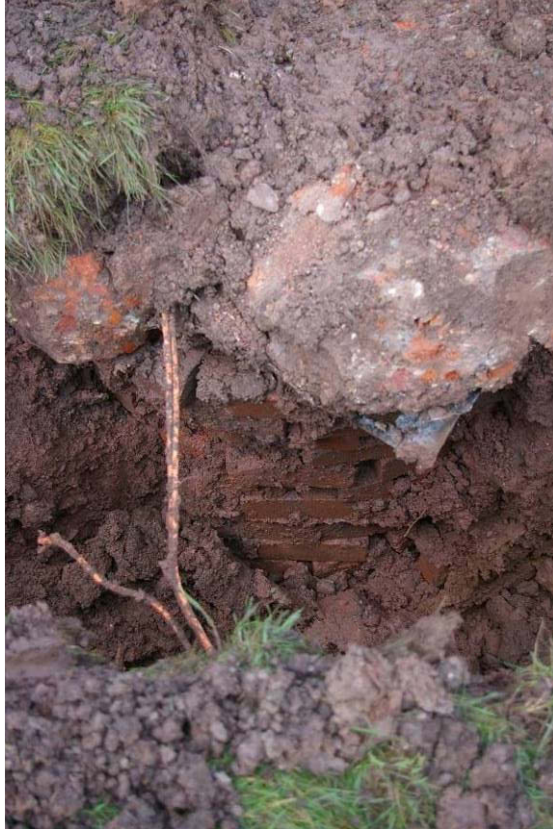
figures 25 and 26: modern brick built soakaway, looking south from above, with and without scale
