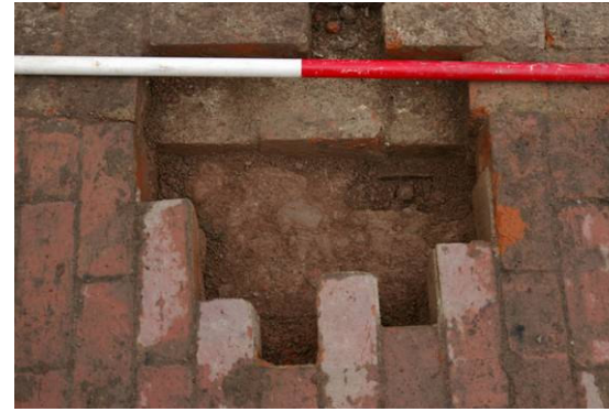
Plate 3: Concrete below the stable floor
