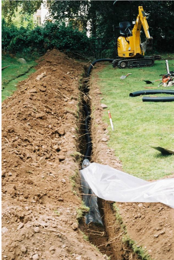
Plate 5: Trench heading south from the church
