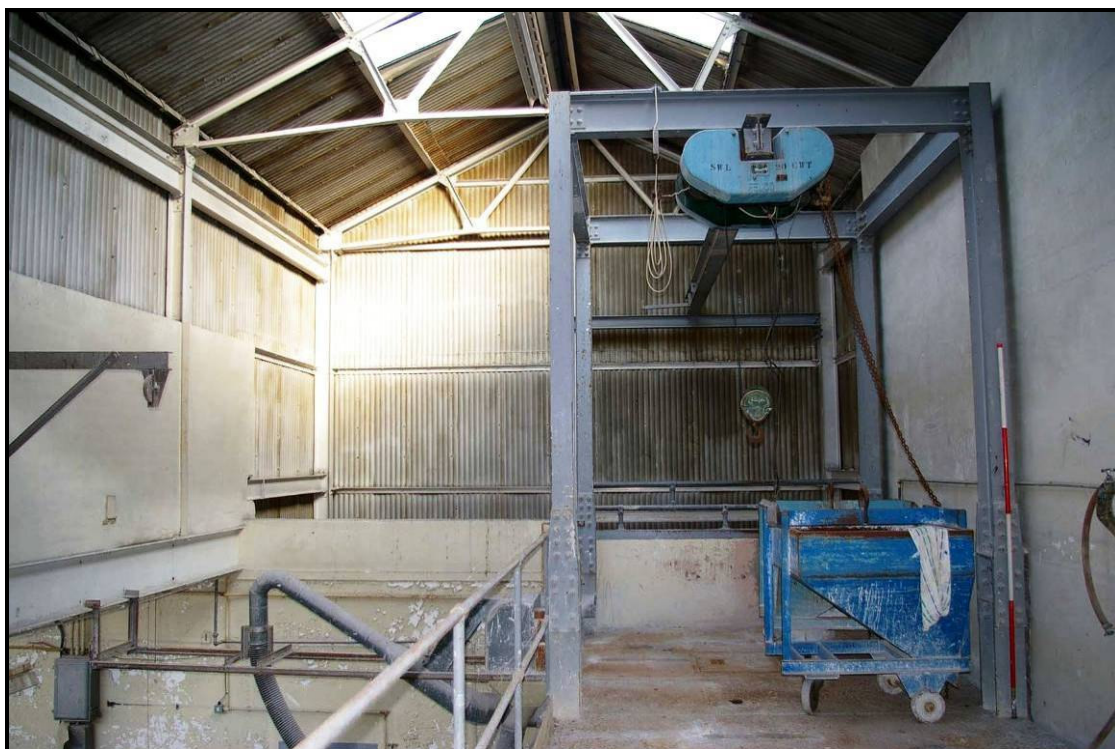
Figure 46: Inside the mezzanine floor of the cross-tower, looking north
