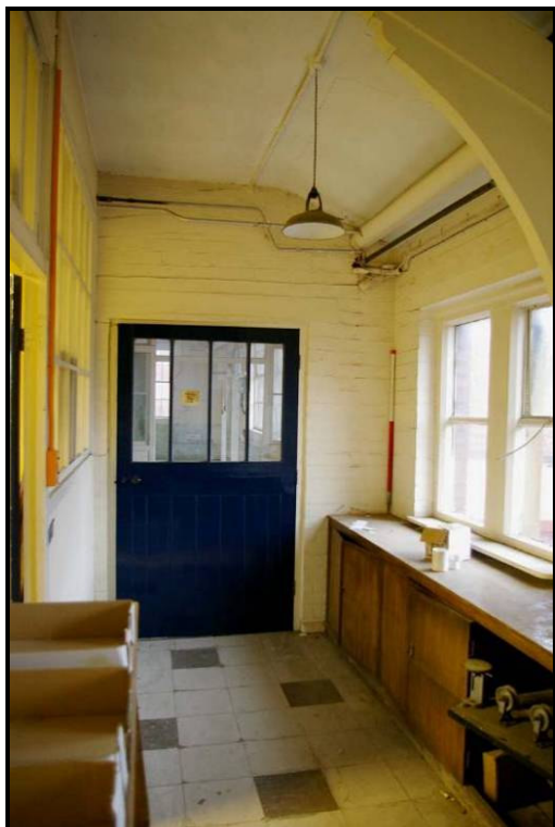
Figure 75: Southern corridor, looking east
