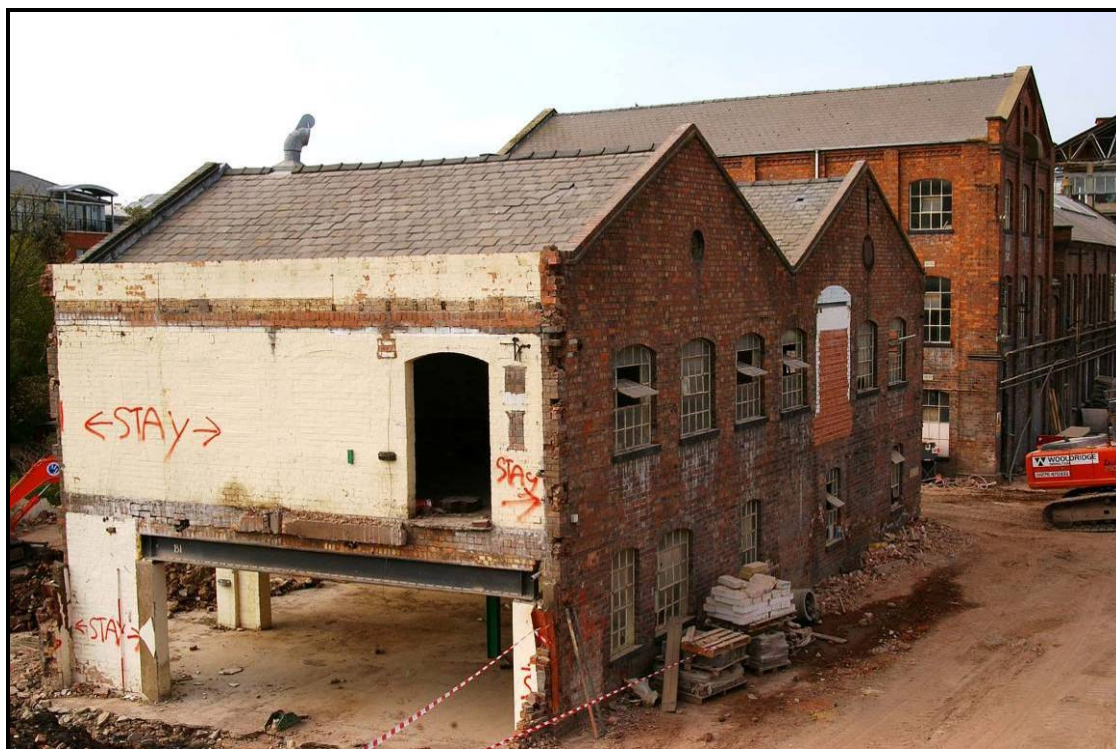
Figure 98: North elevation of Building H after demolition of adjacent buildings
