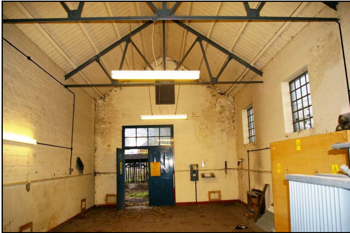
Figure 85: Inside Building B, looking north
