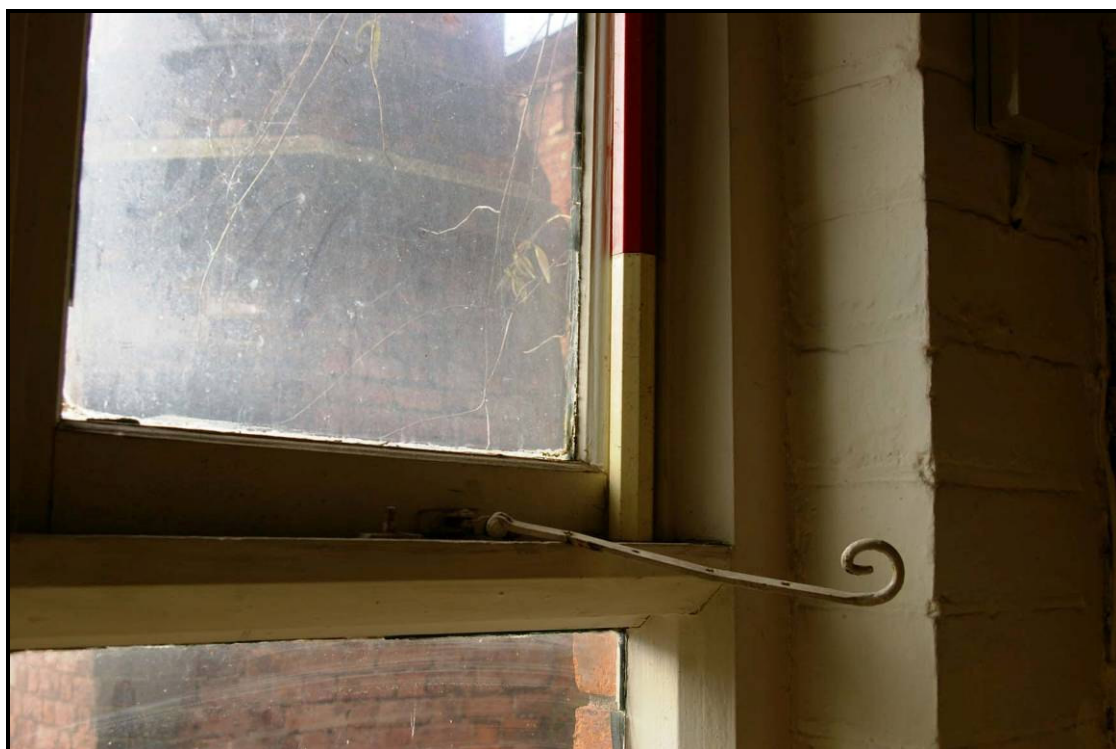
Figure 72: Detail of wrought-iron window stay with rat tail handle
