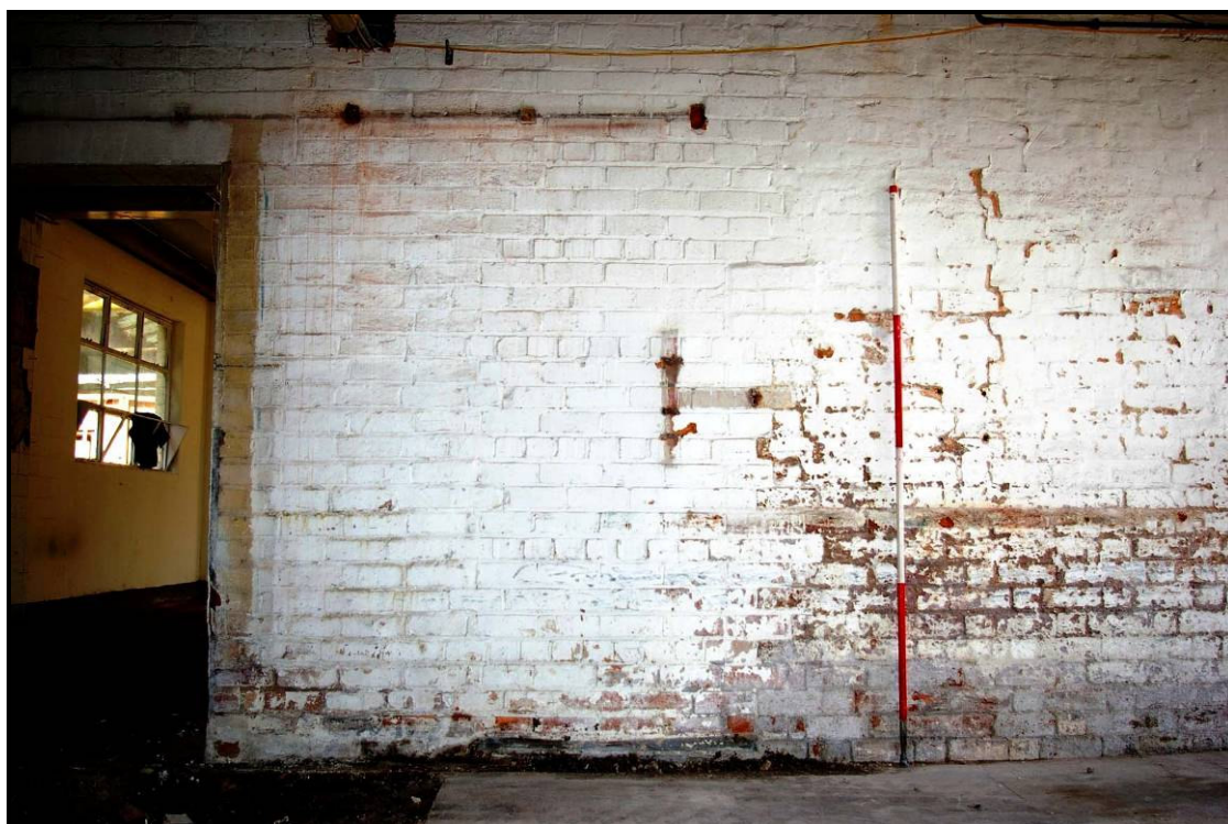
Figure 32: The passageway with a blocked doorway in the centre of the west wall
