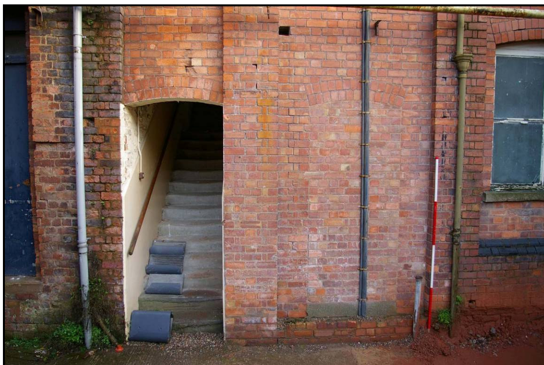
Figure 58: Staircase and blocked doorway on the south elevation of Building B
