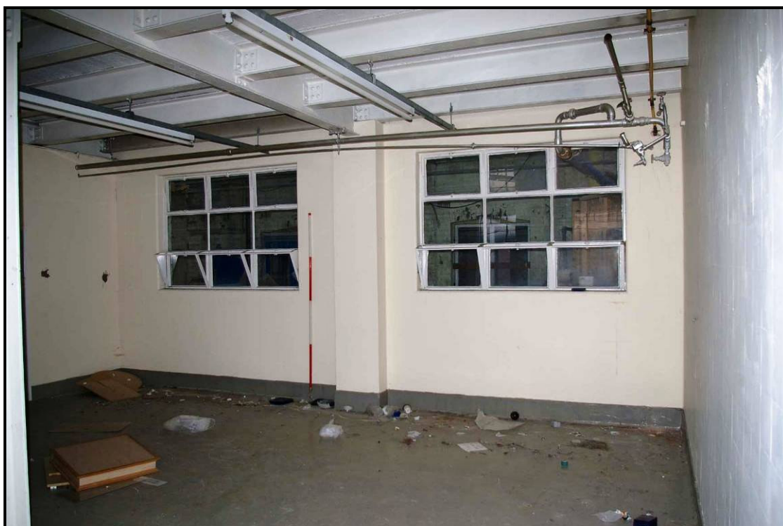
Figure 35: Western workshop, looking south
