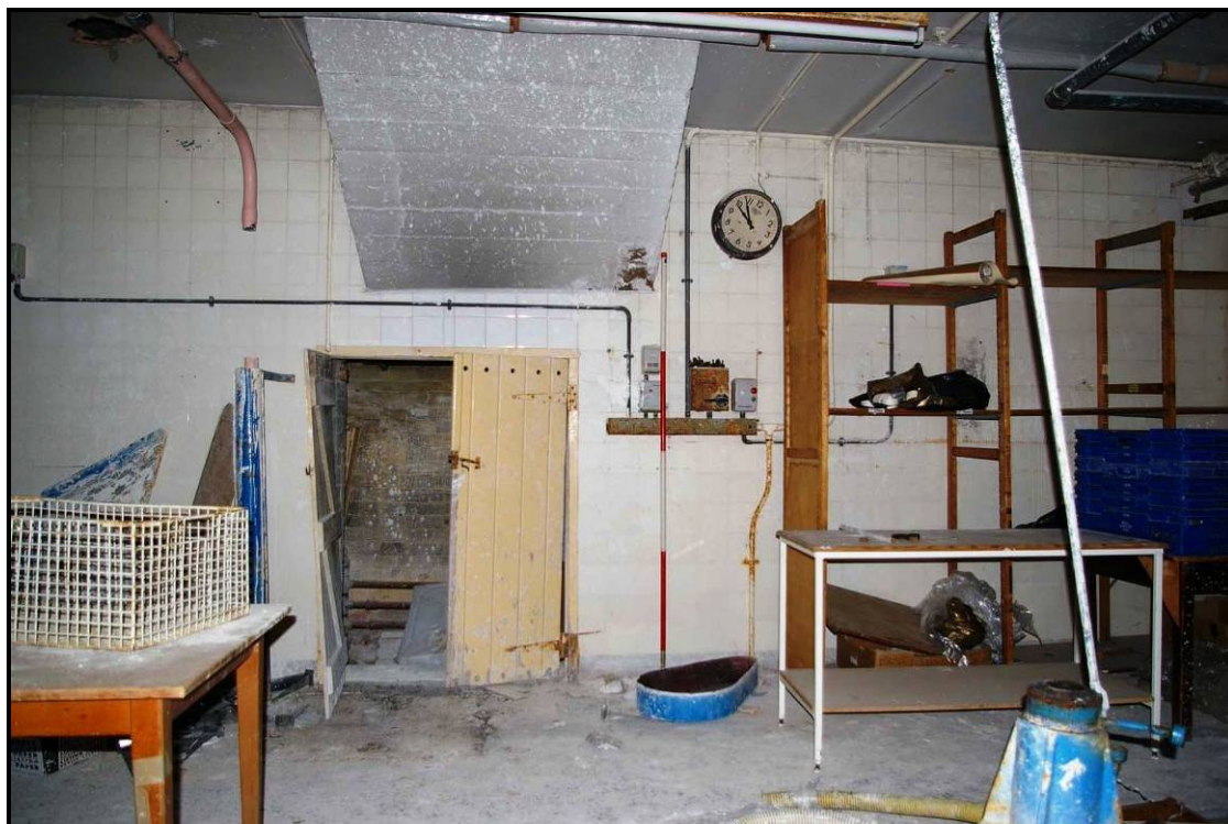
Figure 23: Eastern workshop with concrete stairwell over doorway, looking east
