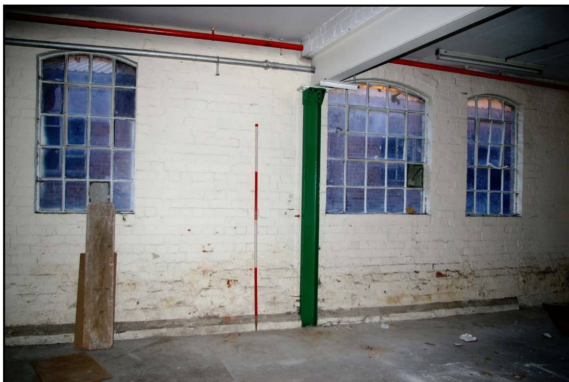
Figure 100: Windows on the west wall of Building H
