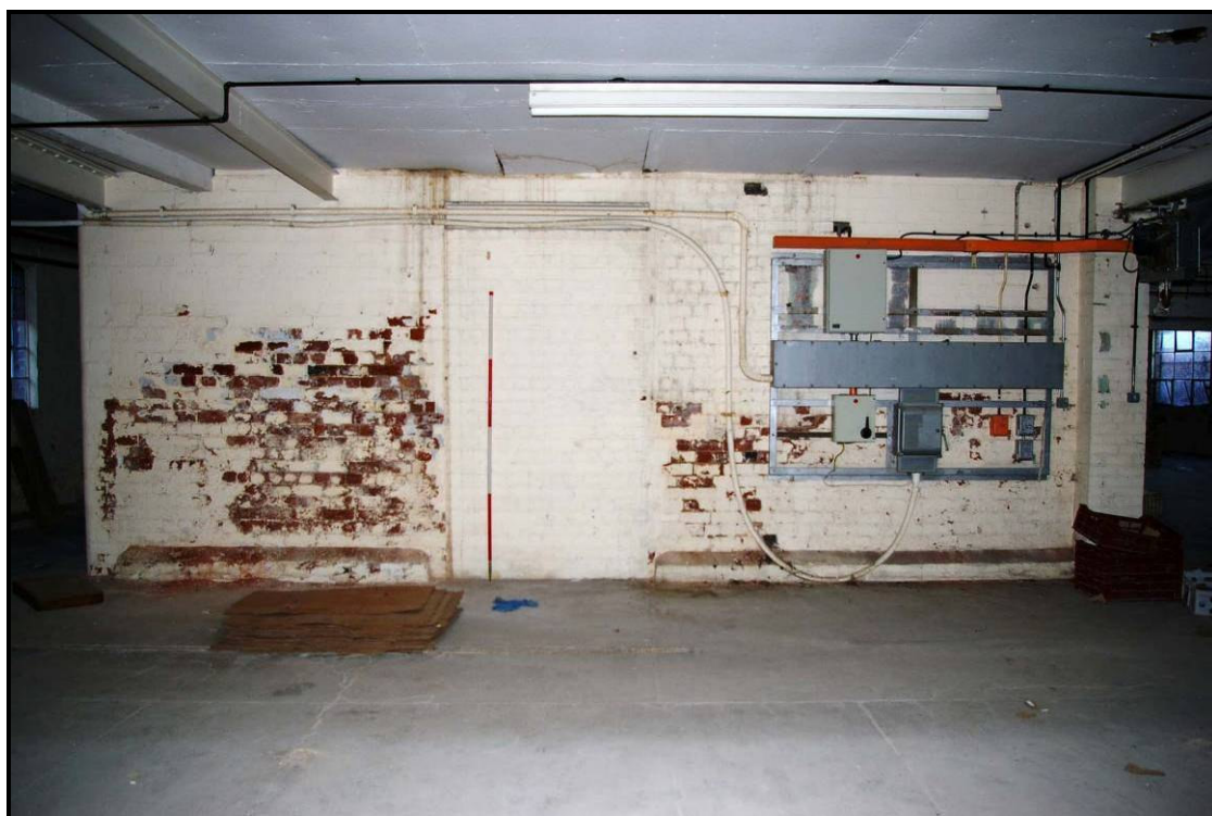
Figure 99: Partition wall on the ground floor with blocked doorway, looking south
