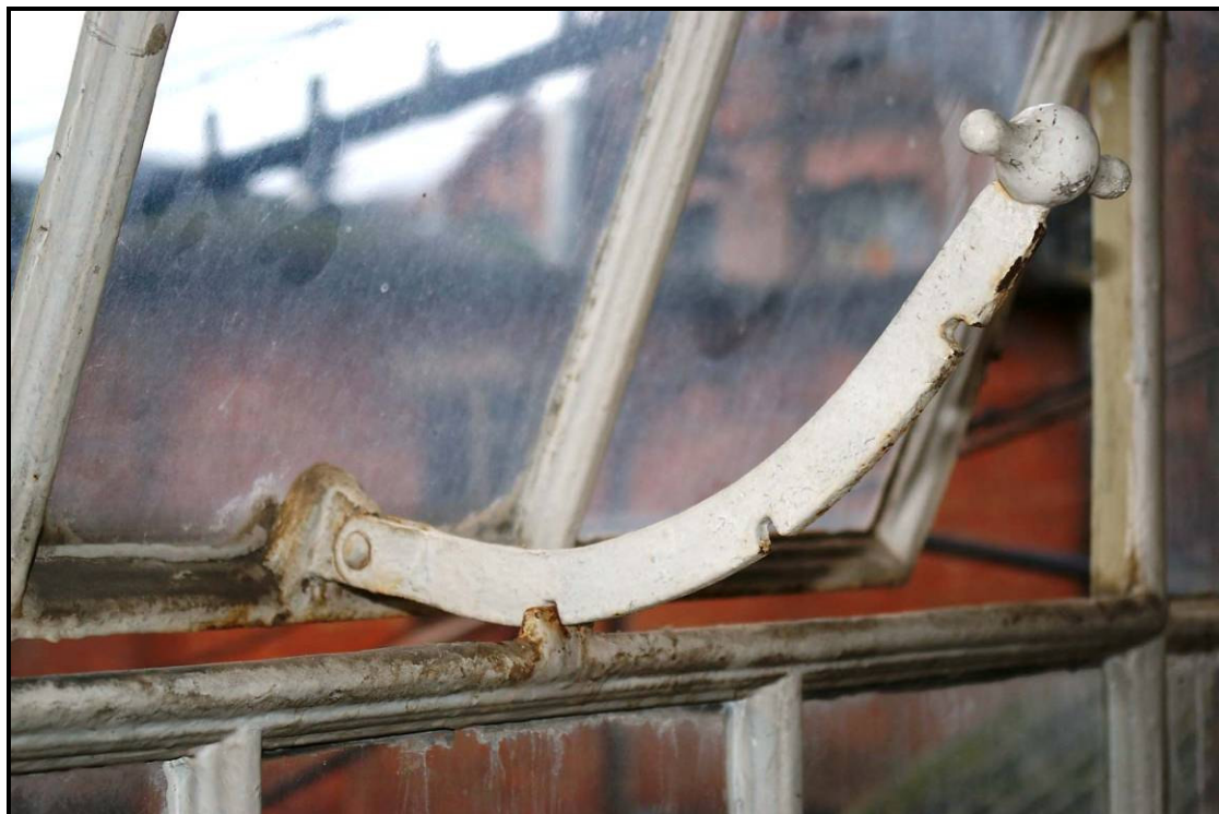
Figure 113: Handle of window opening with pivotal central hinges
