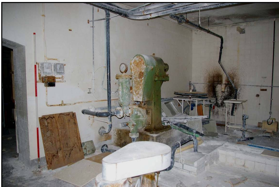
Figure 25: Eastern workshop with machinery, looking north-west
