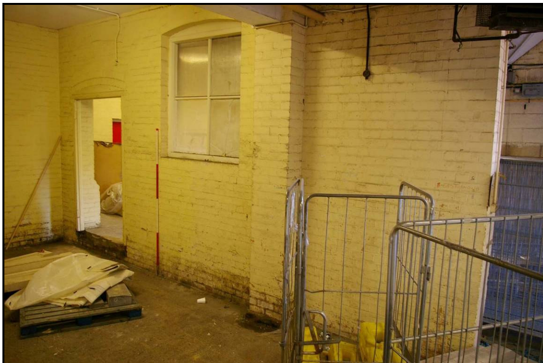
Figure 68: Northern end of the ground floor, looking north-west
