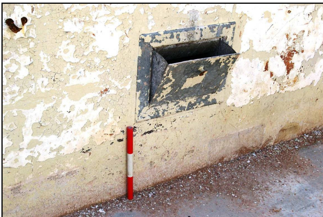
Figure 53: Example of vent with hopper opening on the first floor
