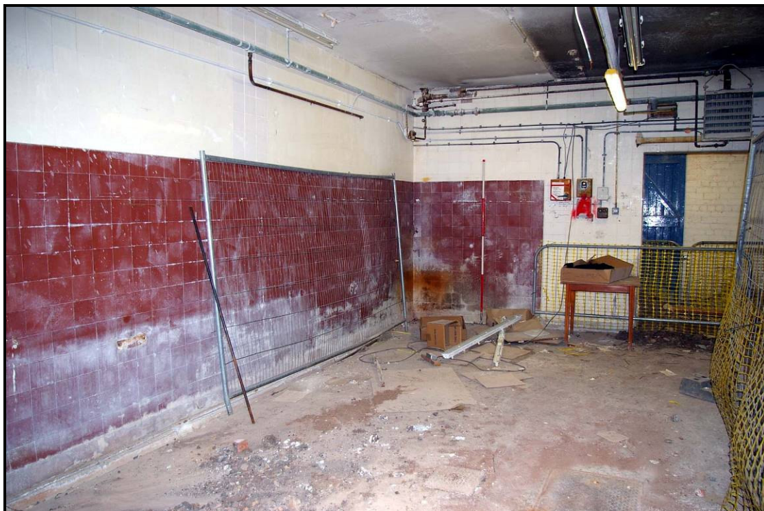
Figure 29: The central workshop, looking west
