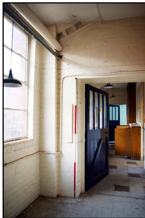
Figure 74: The corridor from Building C1
