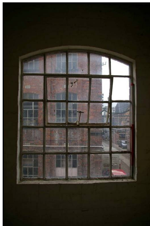
Figure 112: Cast-iron window
