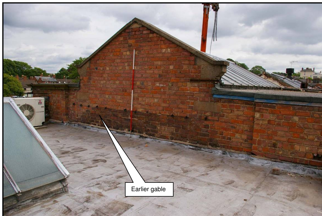
Figure 22: West elevation of Building A
