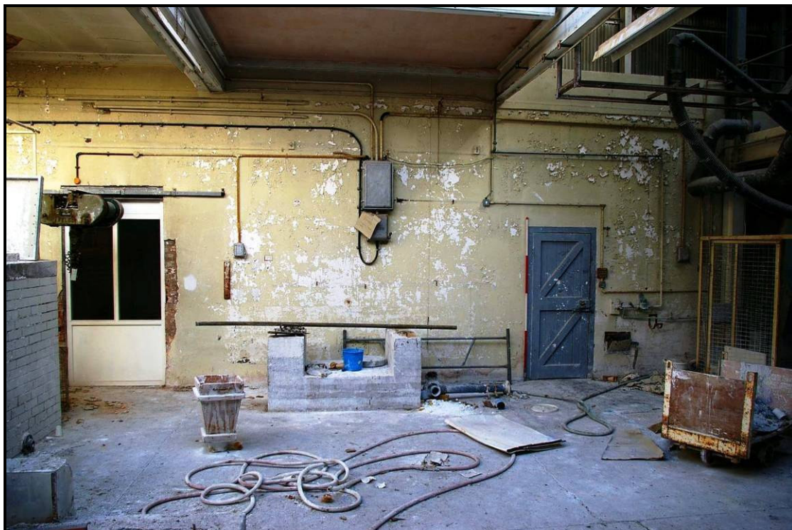
Figure 47: The western workshop of the first floor, looking north
