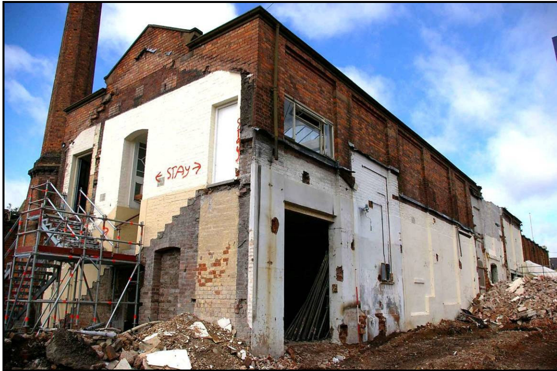
Figure 7: North and east elevations of Building A
