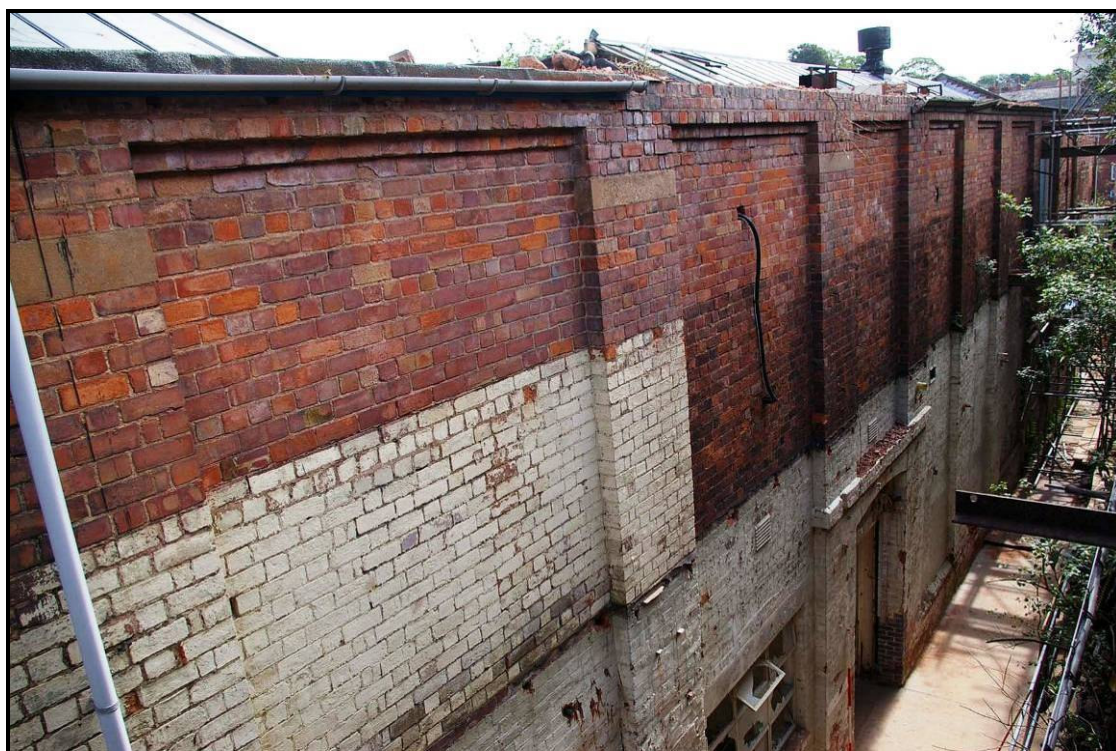
Figure 14: South elevation after demolition of the cross-tower
