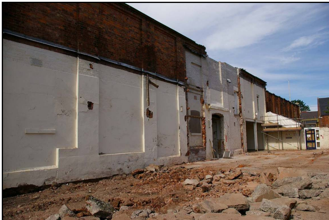
Figure 5: North elevation after demolition of the lean-to extensions
