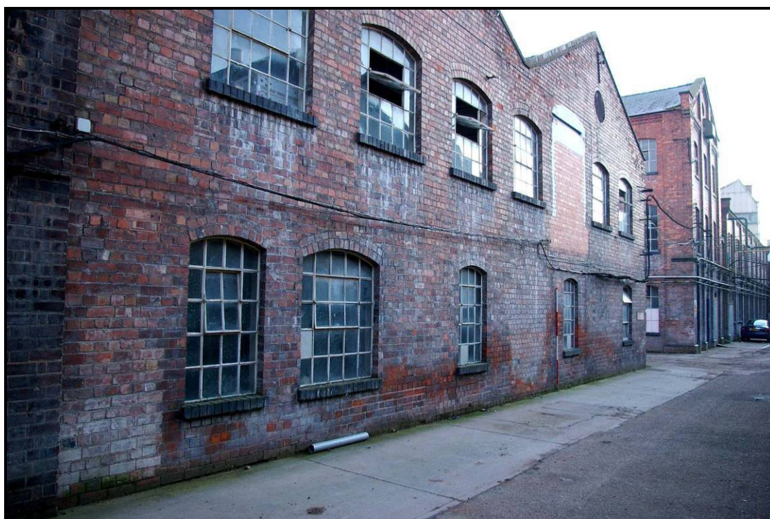
Figure 88: West elevation of Building H
