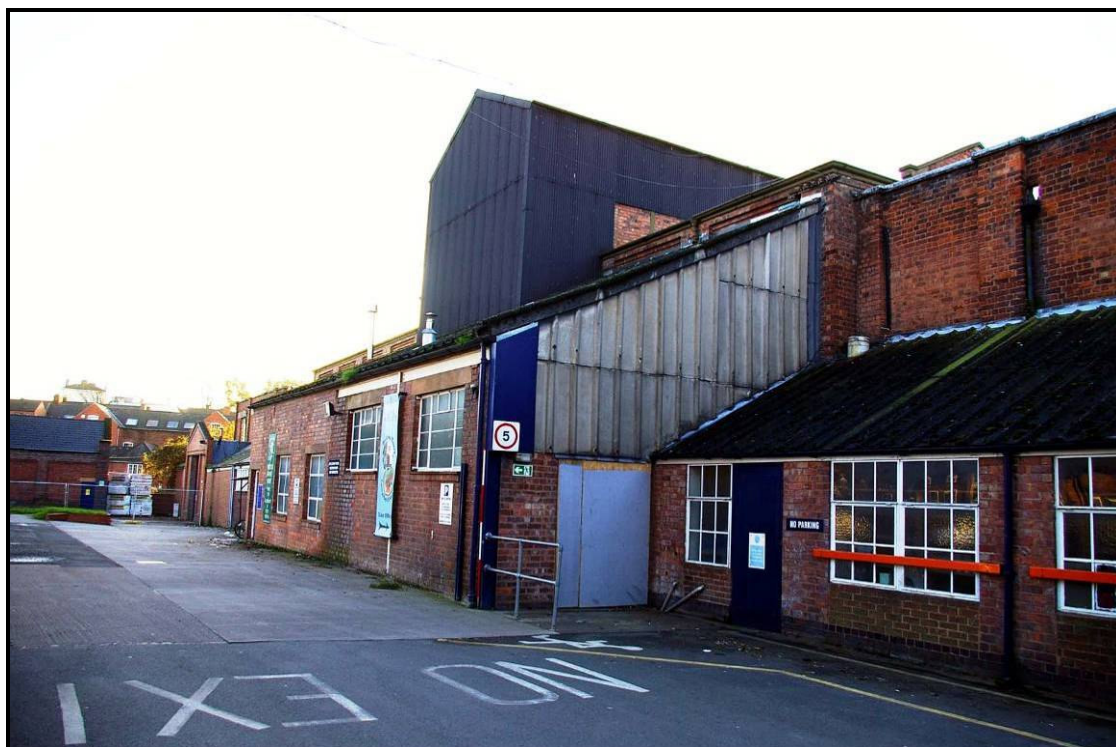
Figure 4: North elevation with lean-to extensions and cross-tower over the roof
