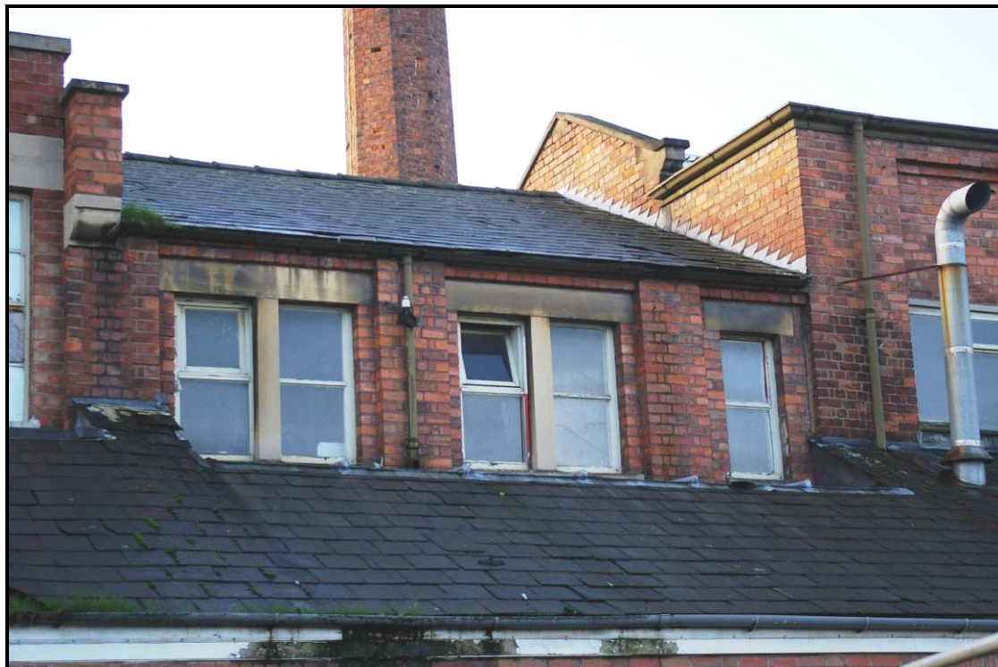
Figure 61: First floor of the north elevation
