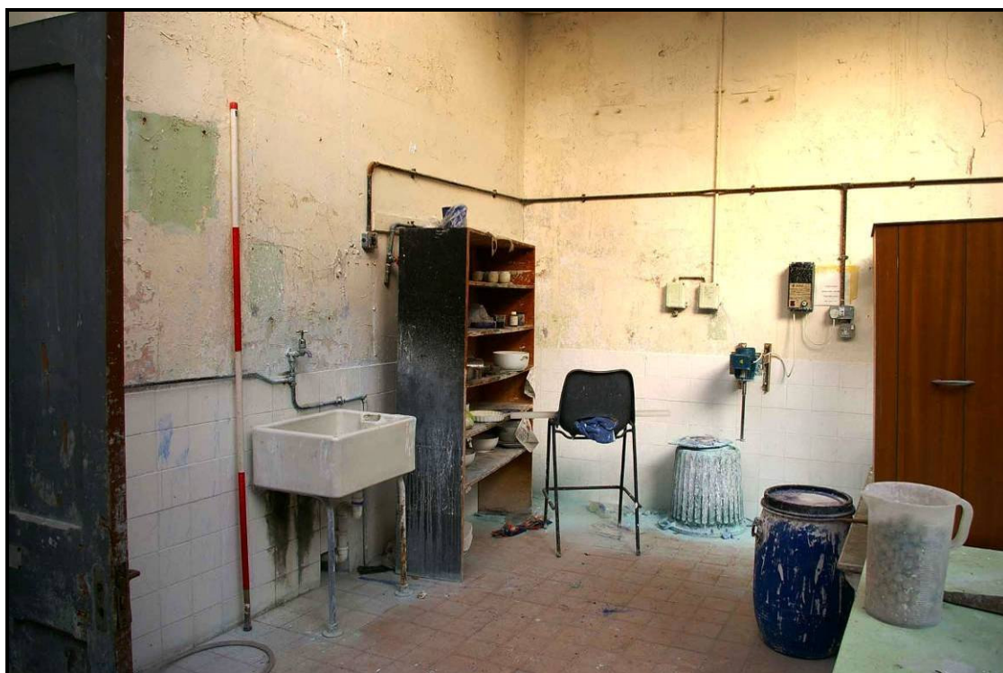
Figure 44: West end of the laboratory, looking north
