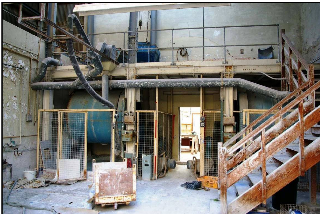
Figure 45: Staircase to the mezzanine floor of the cross-tower, looking east
