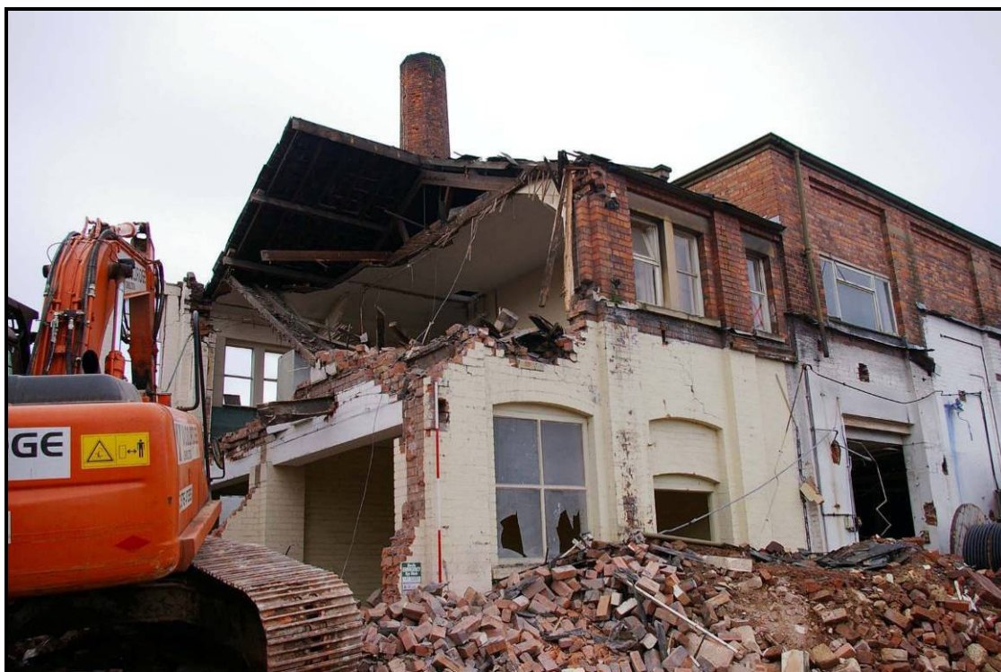
Figure 63: North elevation during demolition
