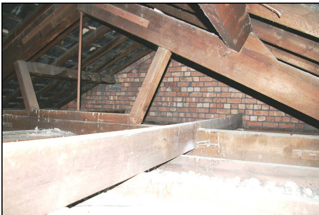
Figure 77: Roof truss of Building B
