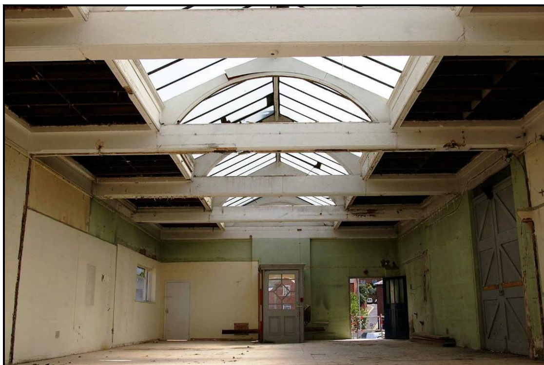
Figure 50: The first floor after interior clearance, looking east
