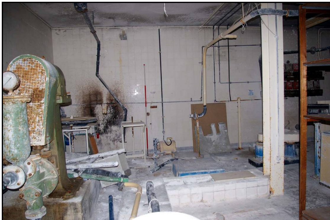
Figure 26: Eastern workshop, looking north
