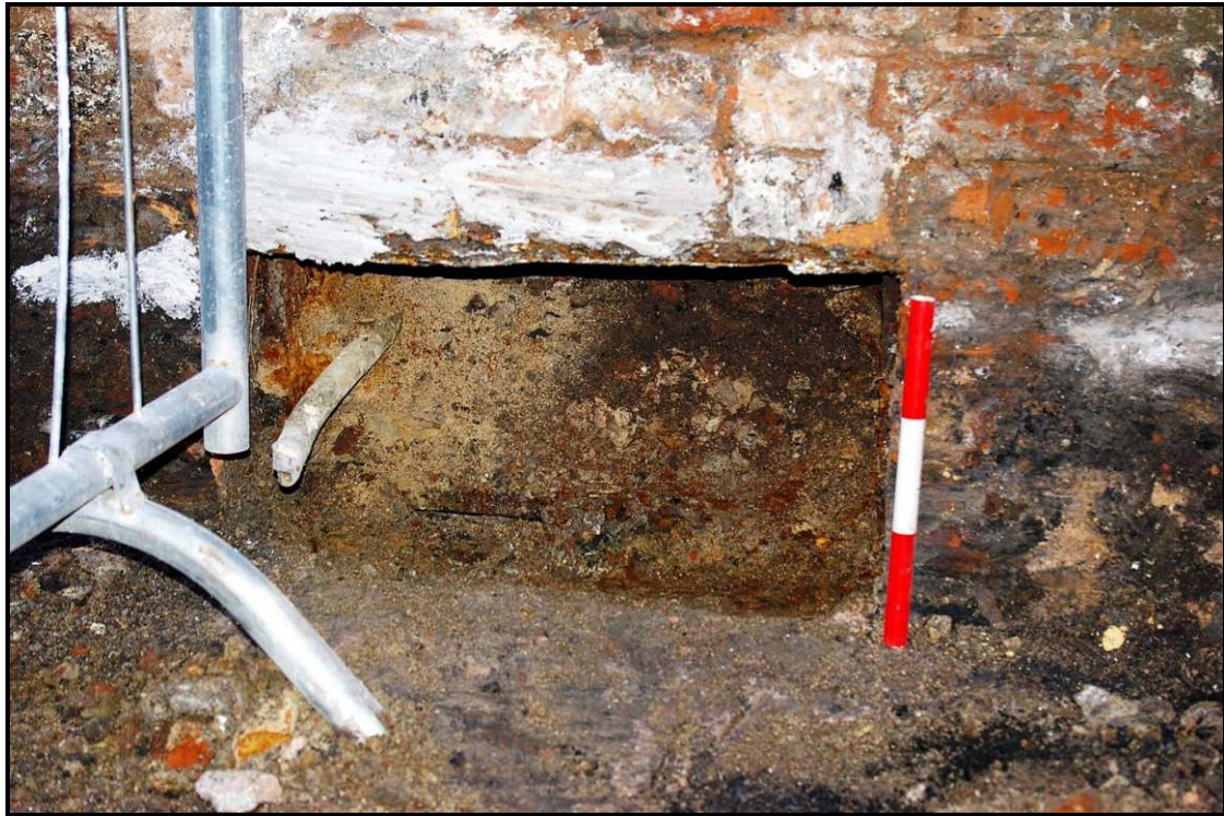
Figure 17: Cast-iron frame of former horizontal drive shaft
