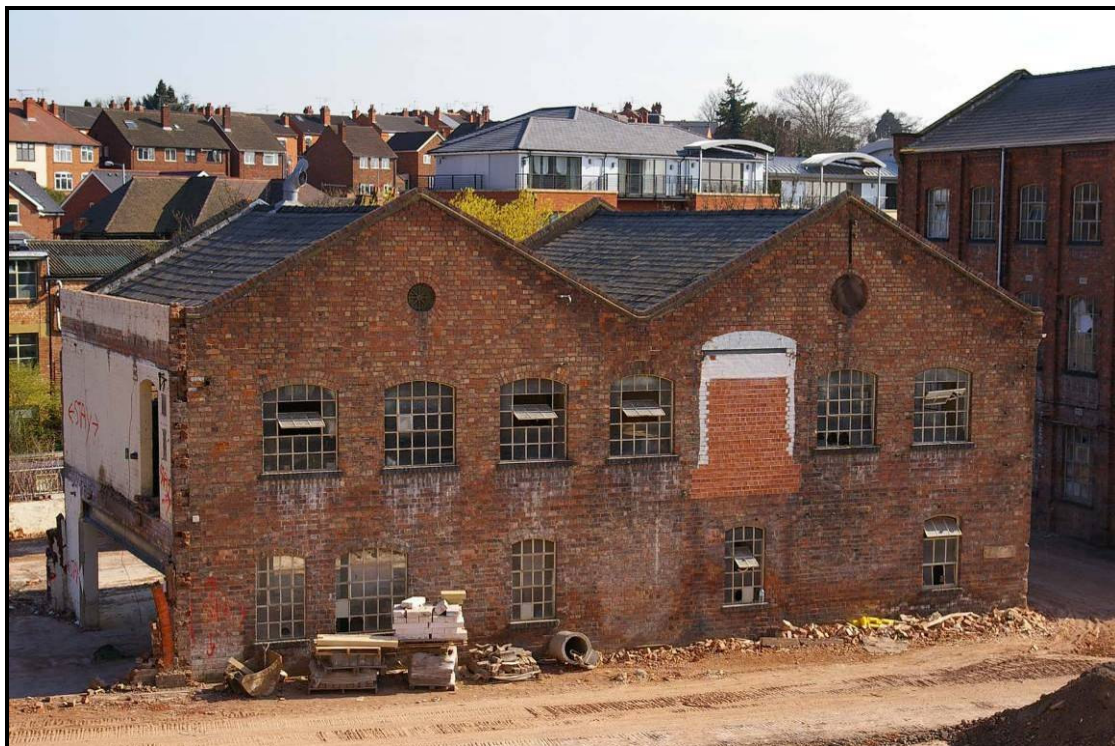
Figure 89: West elevation of Building H after demolition of adjacent buildings
