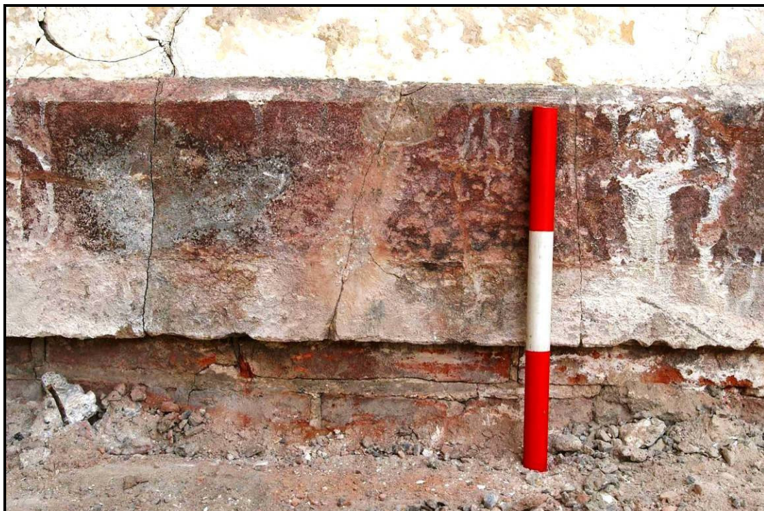
Figure 52: Detail of plinth revealed after the dismantling of the raised platform
