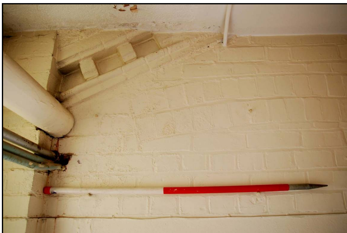
Figure 64: Moulded dentilled brickwork on the first floor of the east elevation
