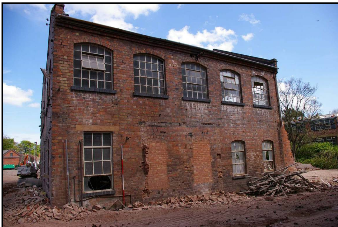
Figure 95: South elevation of Building H
