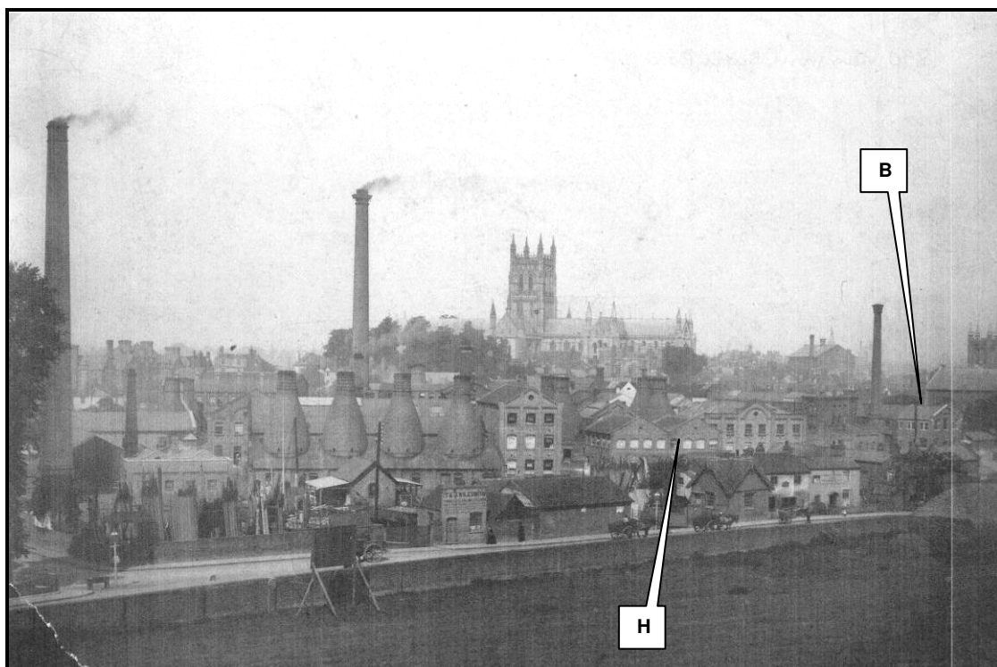
Figure 124: A view of the Works in around 1890 (WPM)
