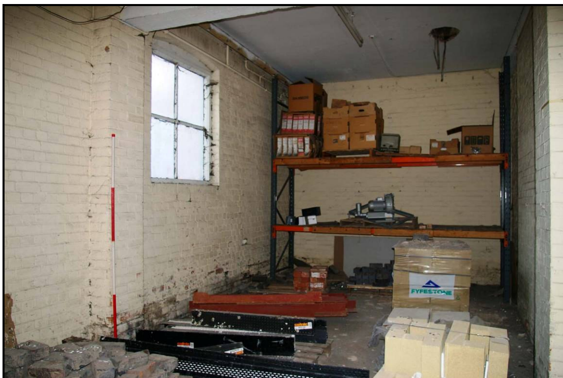
Figure 69: Southern end of the ground floor, looking west
