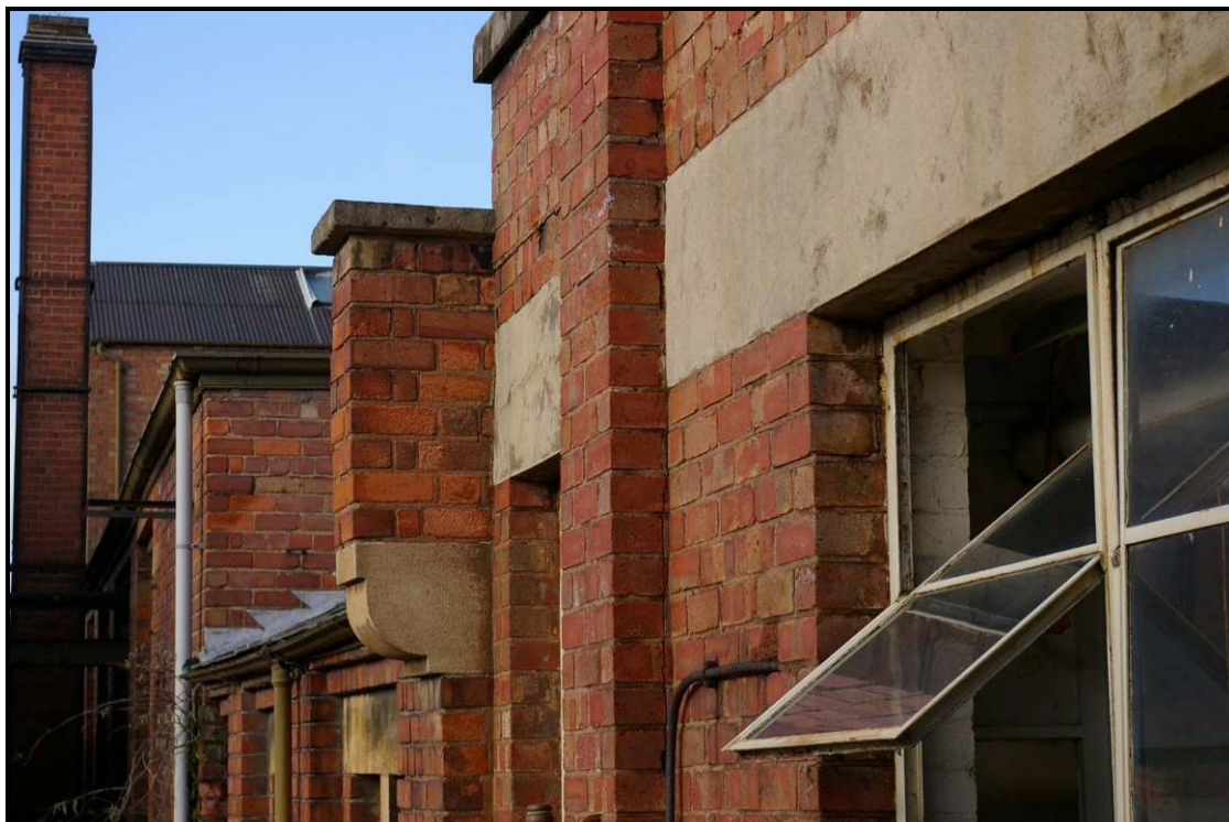
Figure 65: Ovolo moulded kneeler stone of the east elevation
