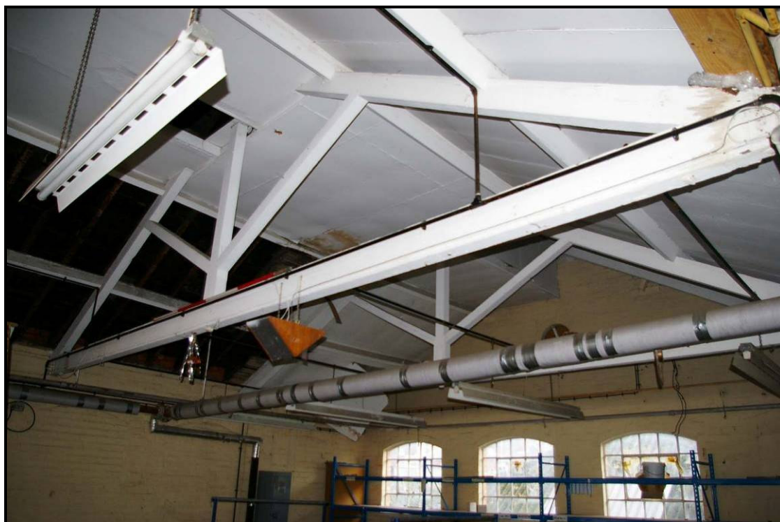
Figure 114: King post roof trusses of Building H
