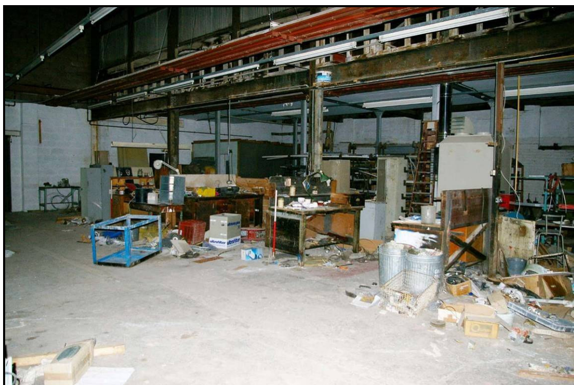
Figure 172: Original roof structure supported by RSJ I-beams and stanchions
