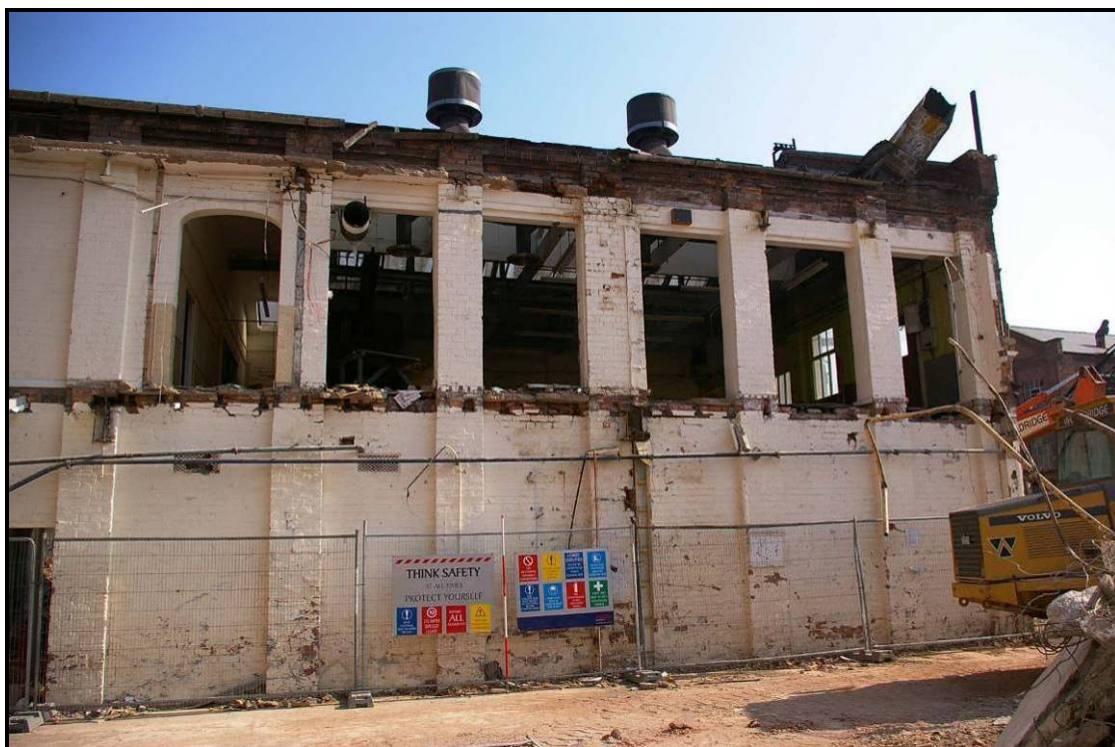
Figure 13: Central and eastern side of the south elevation of Building M
