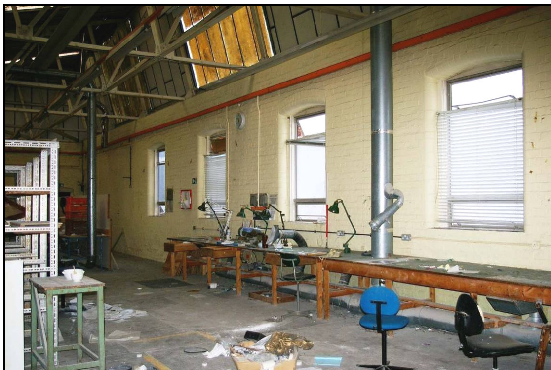
Figure 157: First floor of Building S, looking north-west
