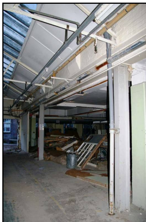
Figure 155: RSJ stanchions and I-beams
