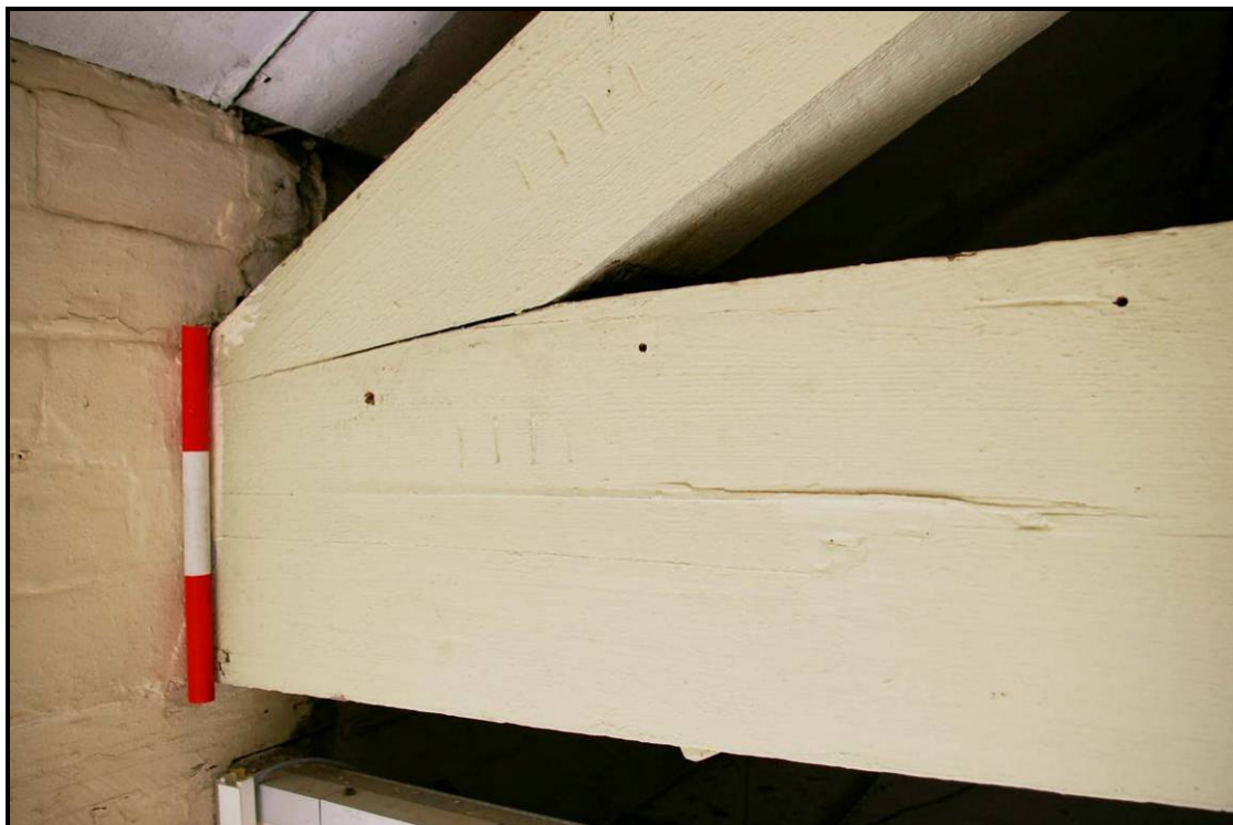
Figure 92: Carpenter's marks on tie beam and principal rafter
