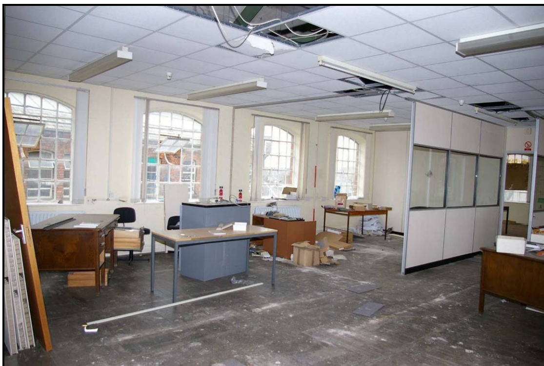
Figure 91: Second floor of Building Q with suspended ceiling under timber trusses
