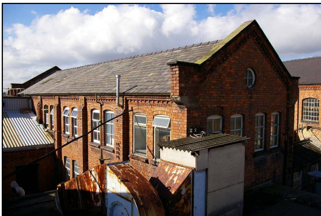
Figure 103: East elevation of Building R
