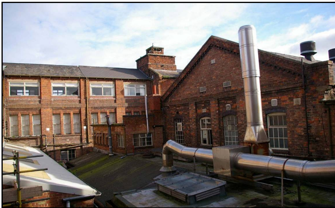
Figure 9: West elevation of Building M
