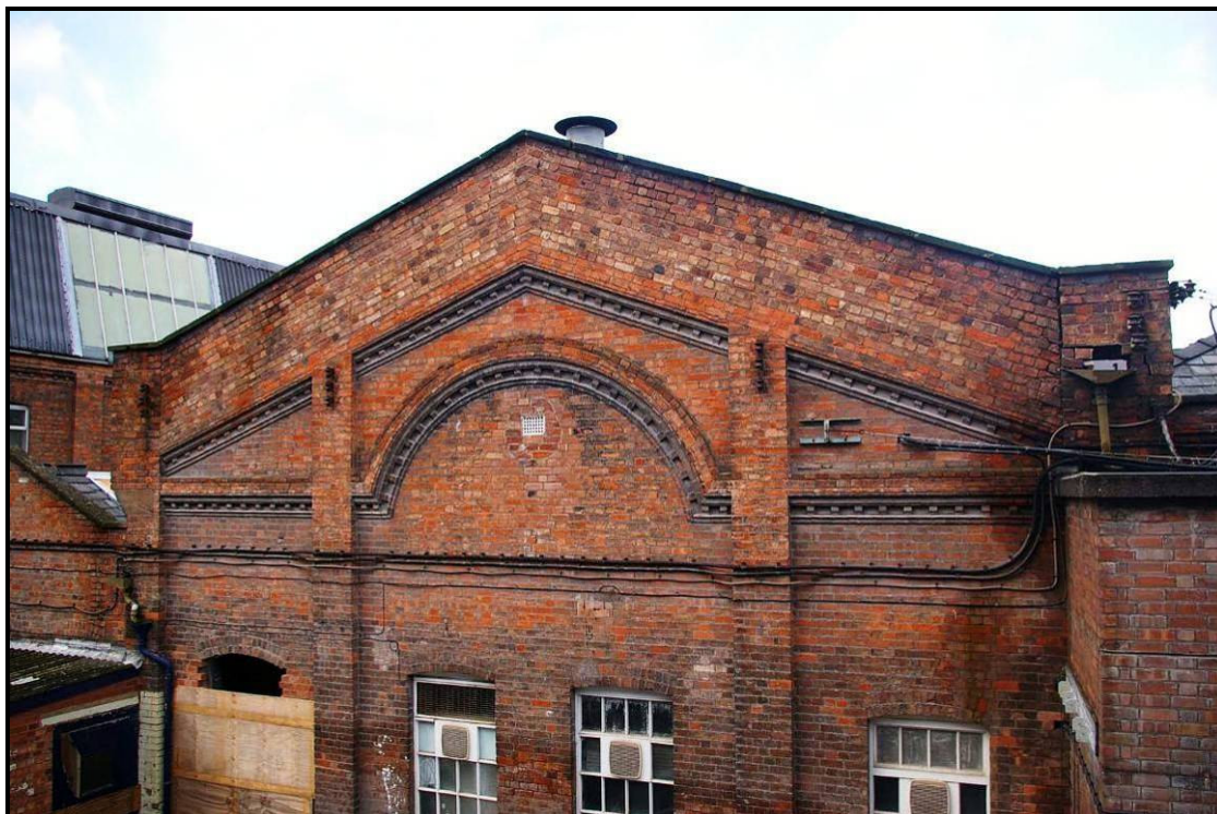
Figure 30: West elevation of Building N, viewed from Building K2
