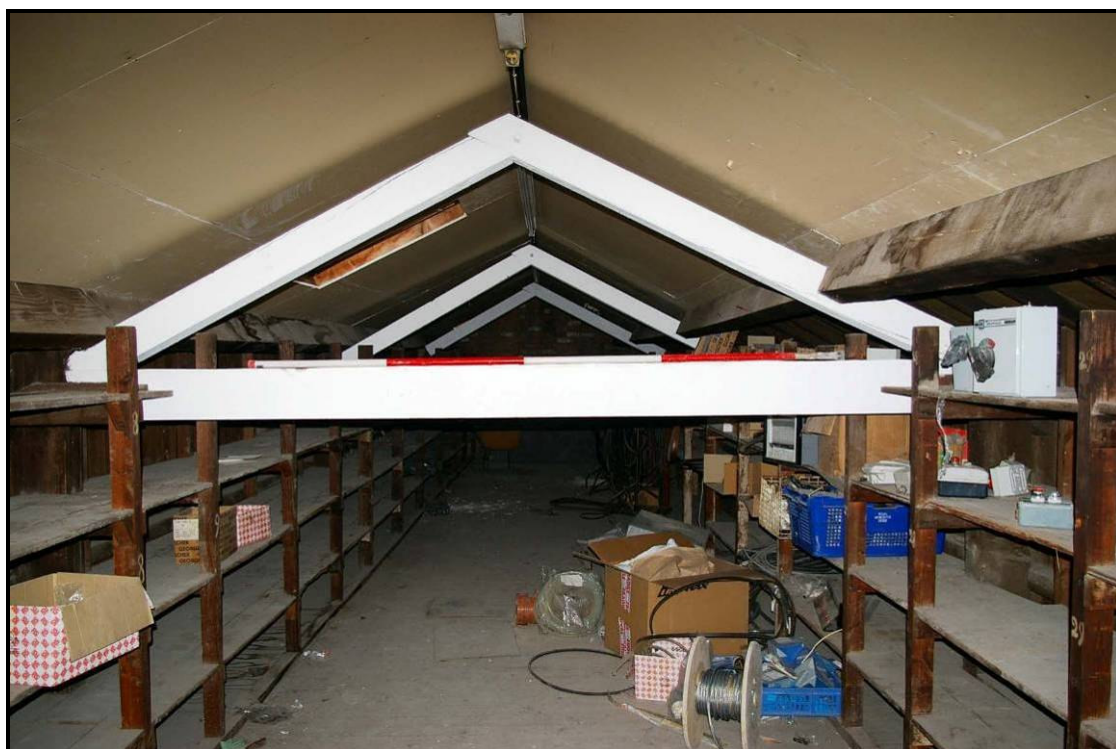
Figure 165: Loft inside the New Mould Shed
