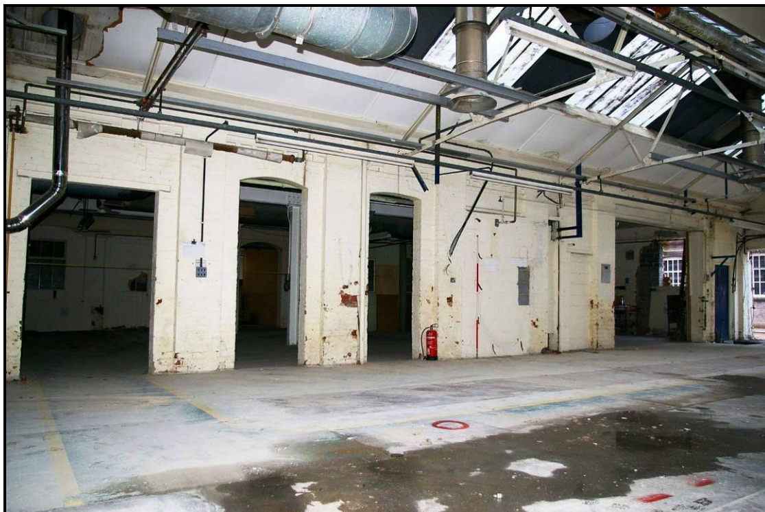
Figure 36: South elevation of Building N
