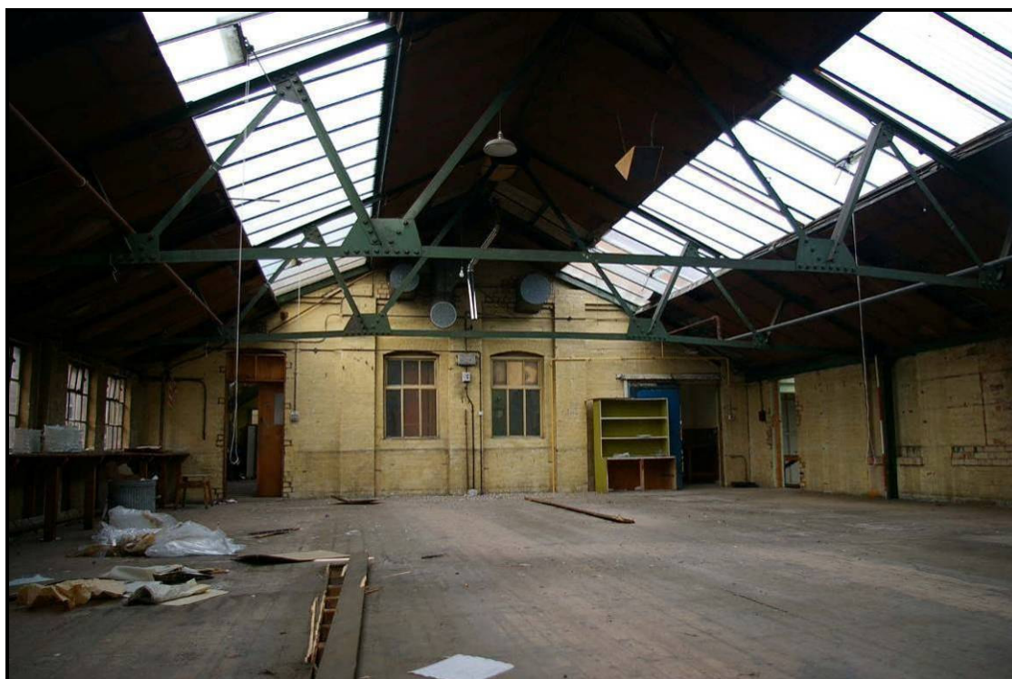
Figure 3: East elevation of Building M, from Building N
