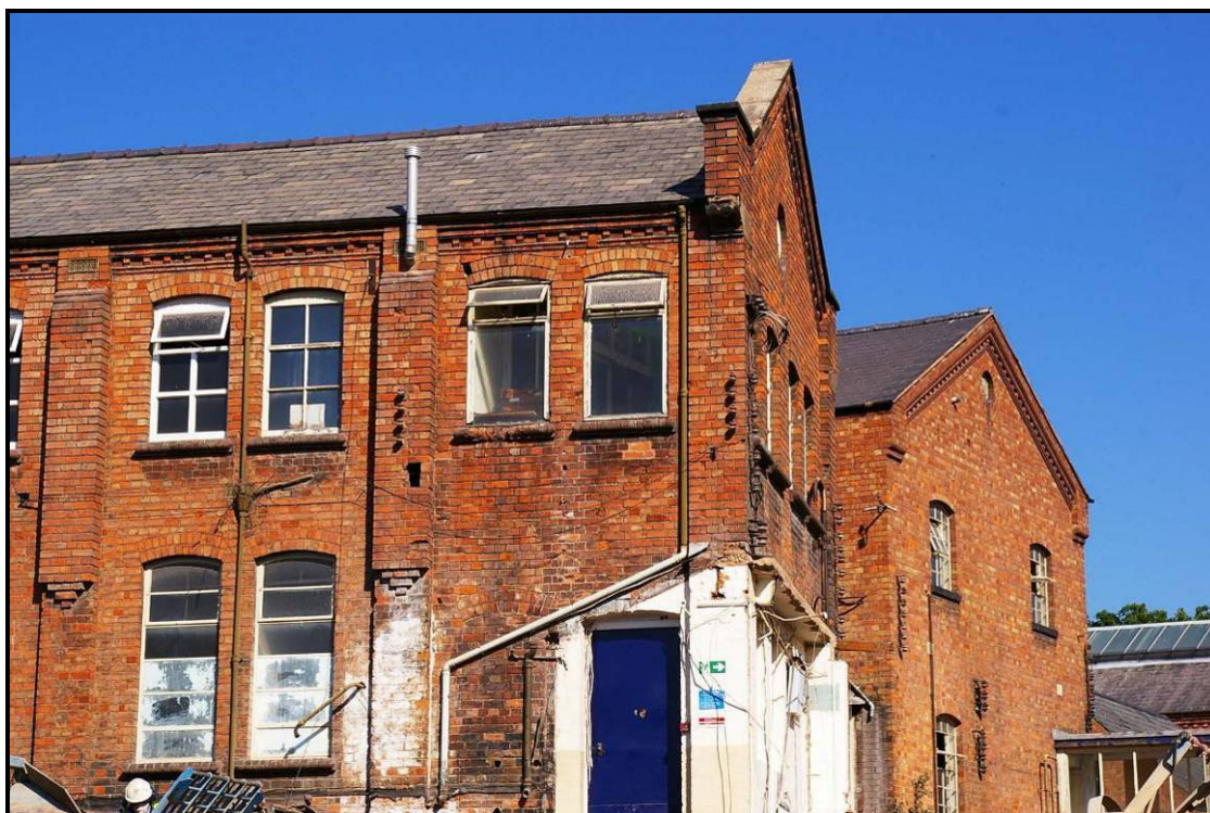
Figure 108: Northern end of the east elevation of Building R
