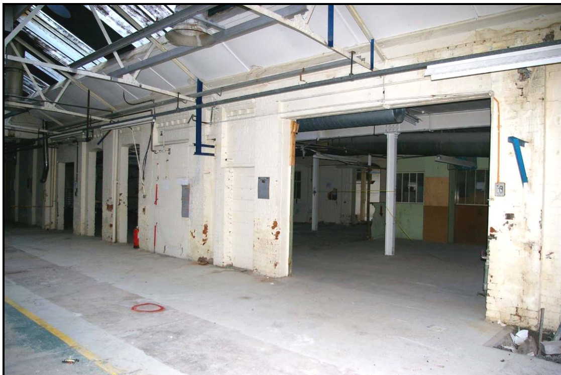
Figure 34: South elevation of Building N, looking south-west
