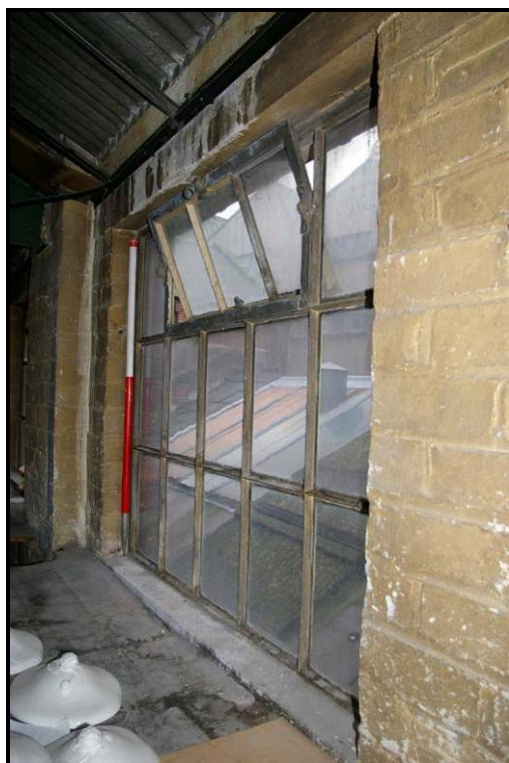
Figure 54: Detail of window
