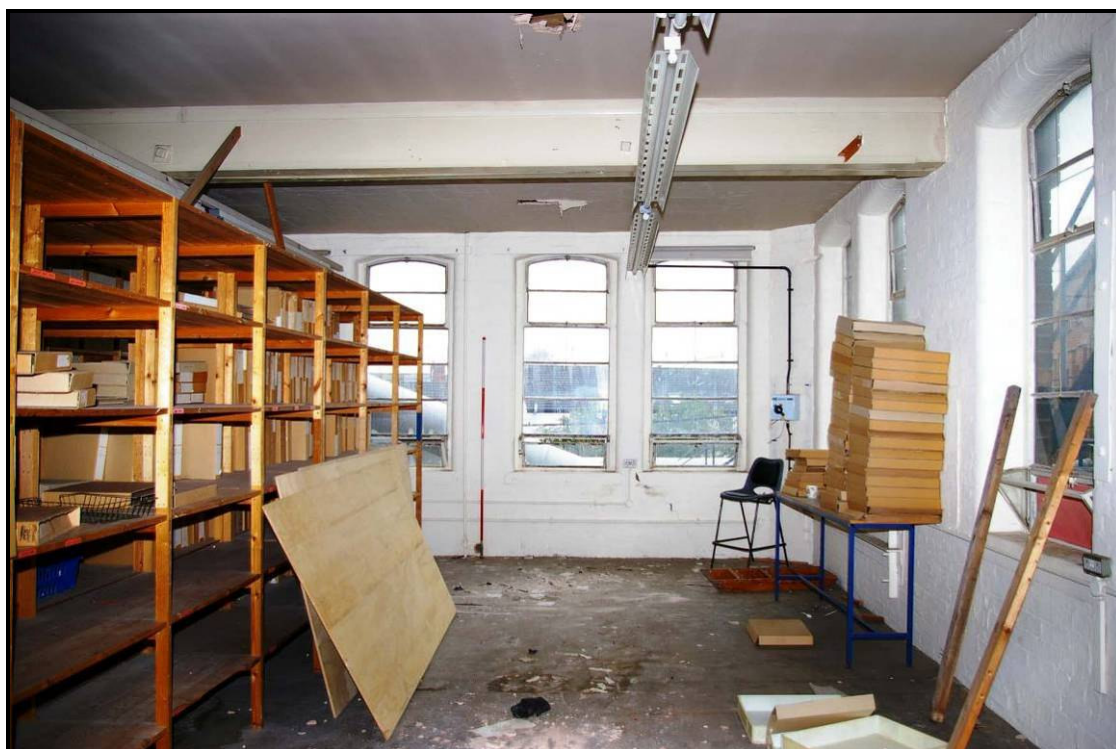
Figure 126: South-west corner of the first floor of Building R
