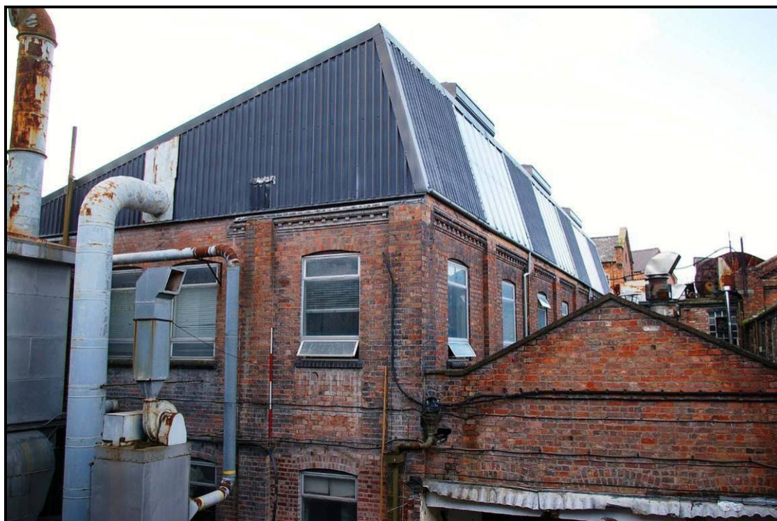
Figure 141: East elevation of Building S
