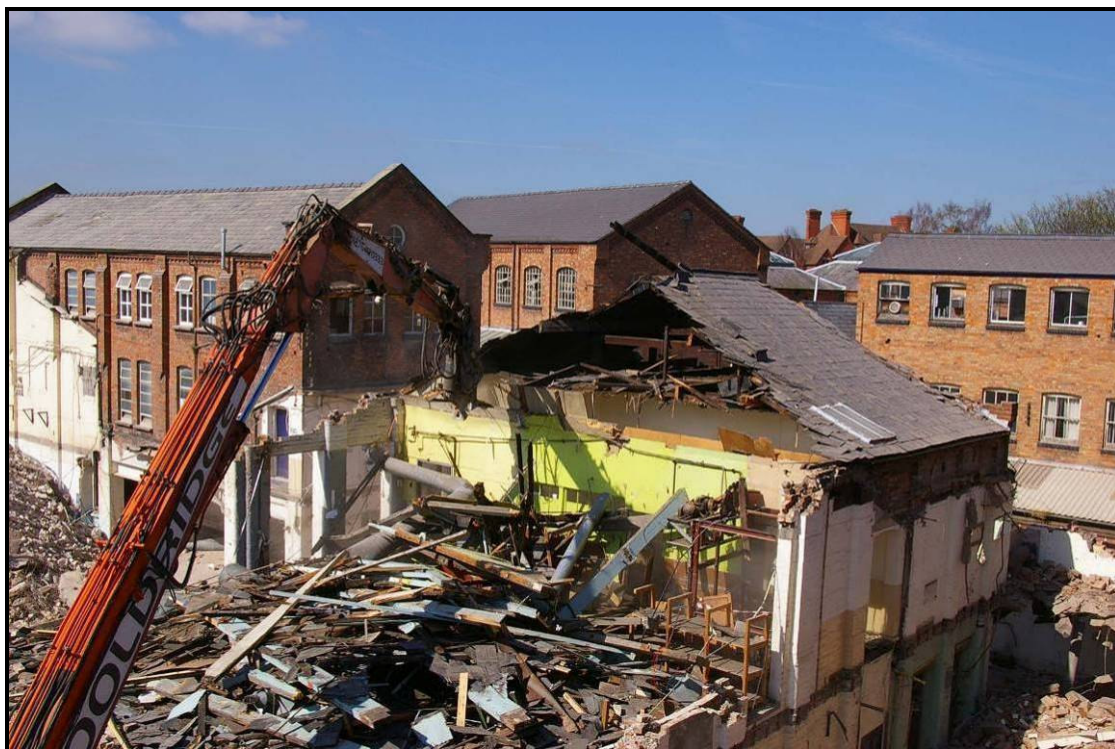
Figure 26: Building M under demolition, looking south-west
