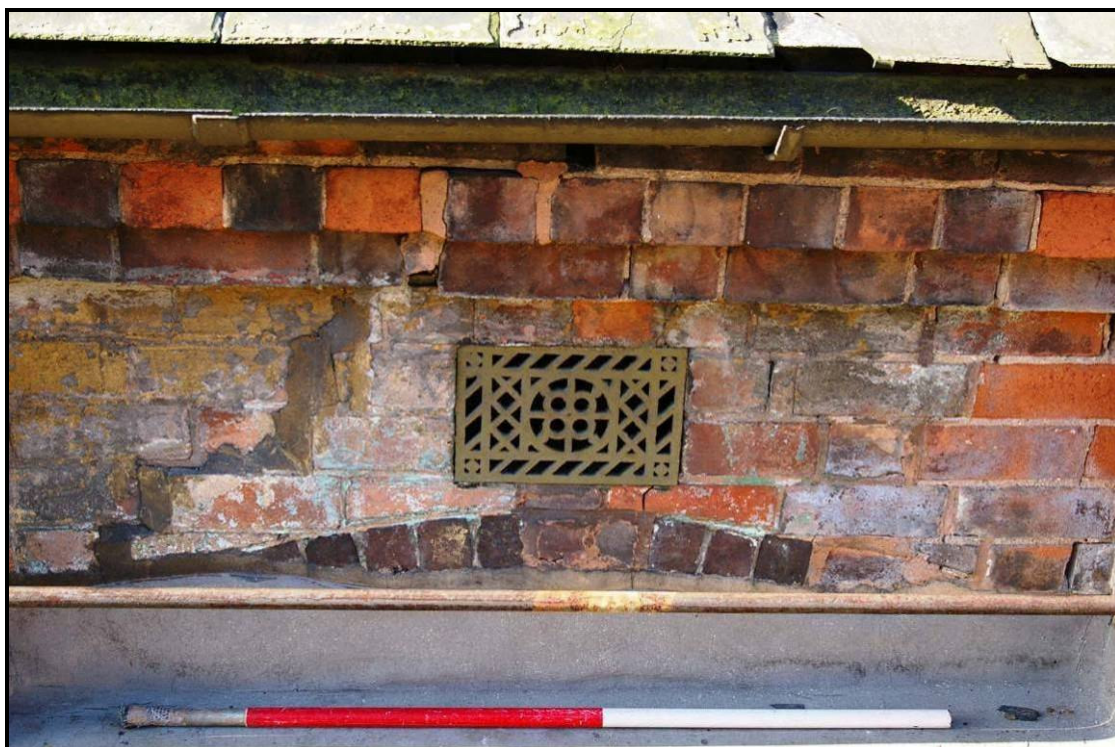
Figure 16: Detail of cast-iron vent on the north elevation of Building M
