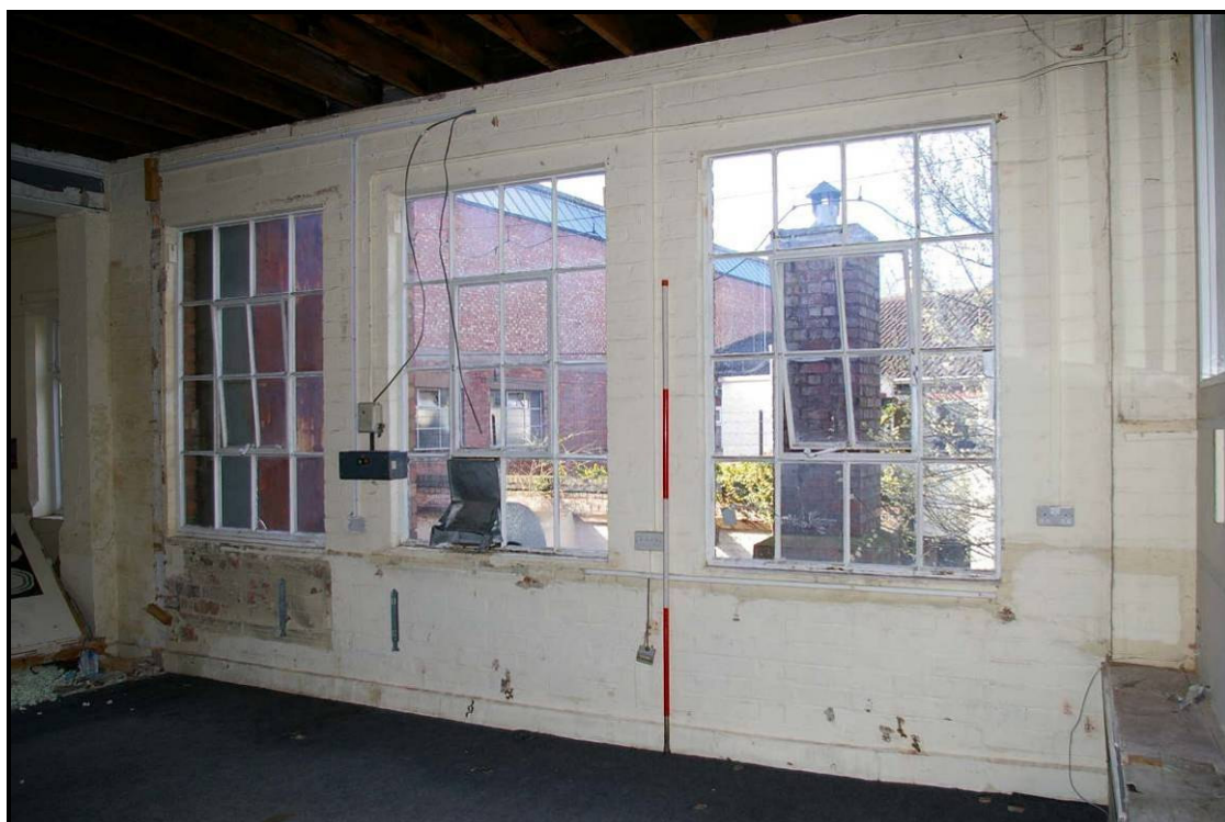
Figure 83: Windows of the southern bridge of Building Q, looking south
