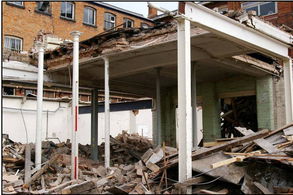
Figure 22: Detail of jack-arched ceiling during demolition
