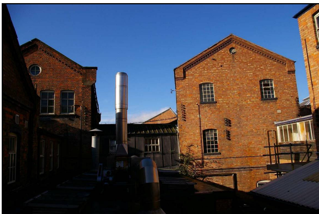
Figure 65: General view of the north elevation of Building Q
