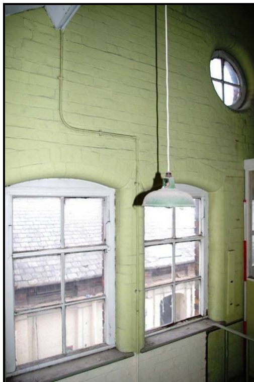
Figure 128: Northern gable wall
