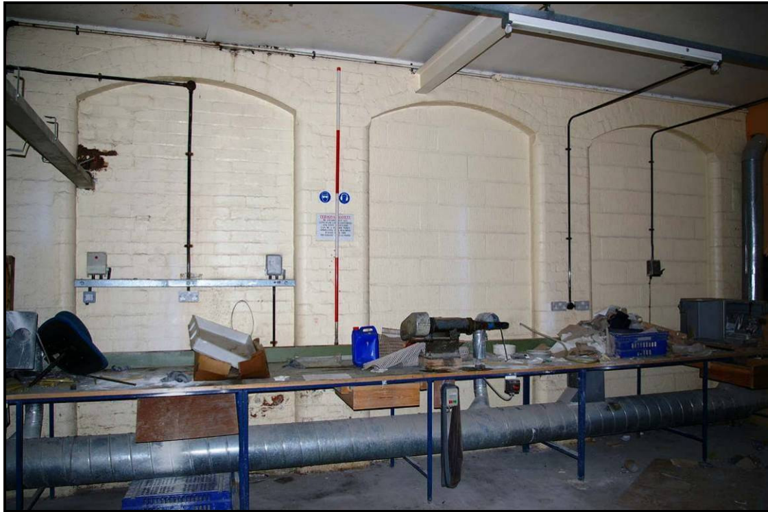
Figure 40: Ground floor of the north elevation of Building N
