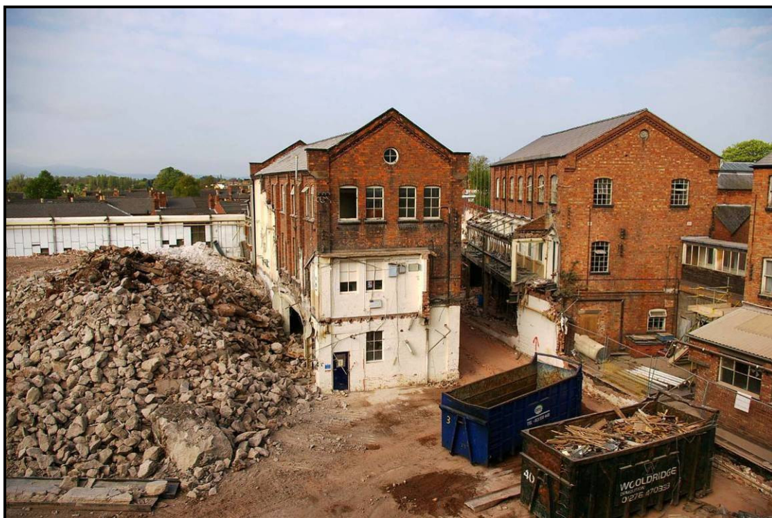
Figure 67: Buildings Q and R after demolition of surrounding buildings, looking south
