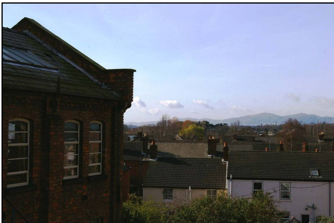
Figure 102: Southern gable end of Building R
