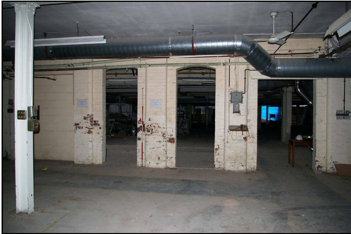
Figure 43: Ground floor of Building N, looking south
