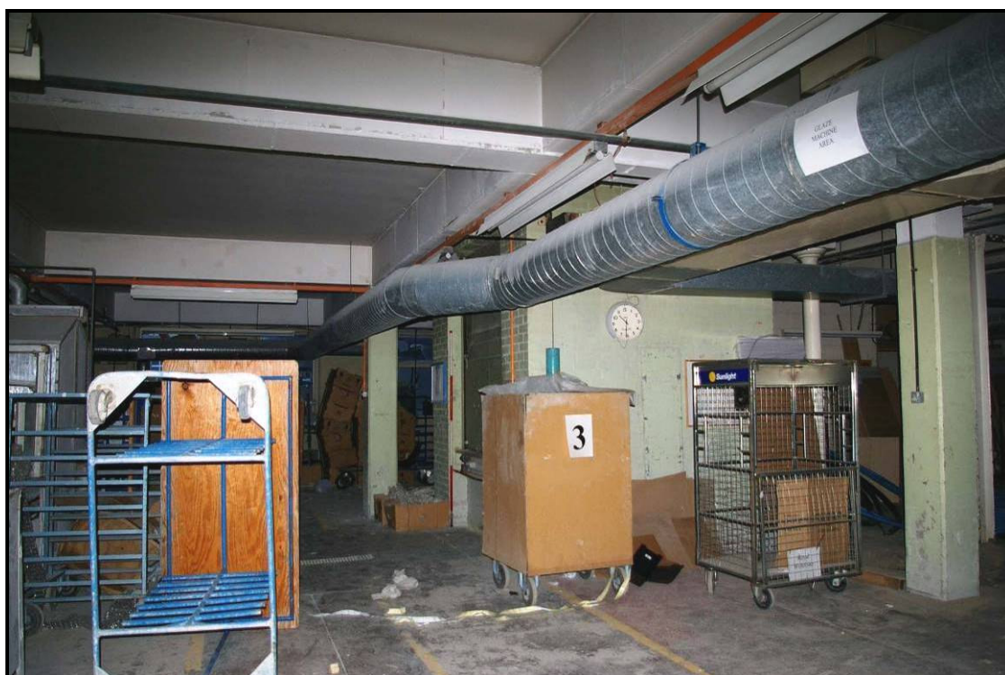
Figure 152: Ground floor of Building S, looking east
