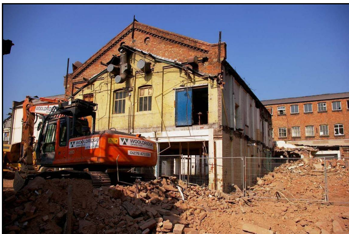
Figure 6: East elevation of Building M after demolition of surrounding buildings
