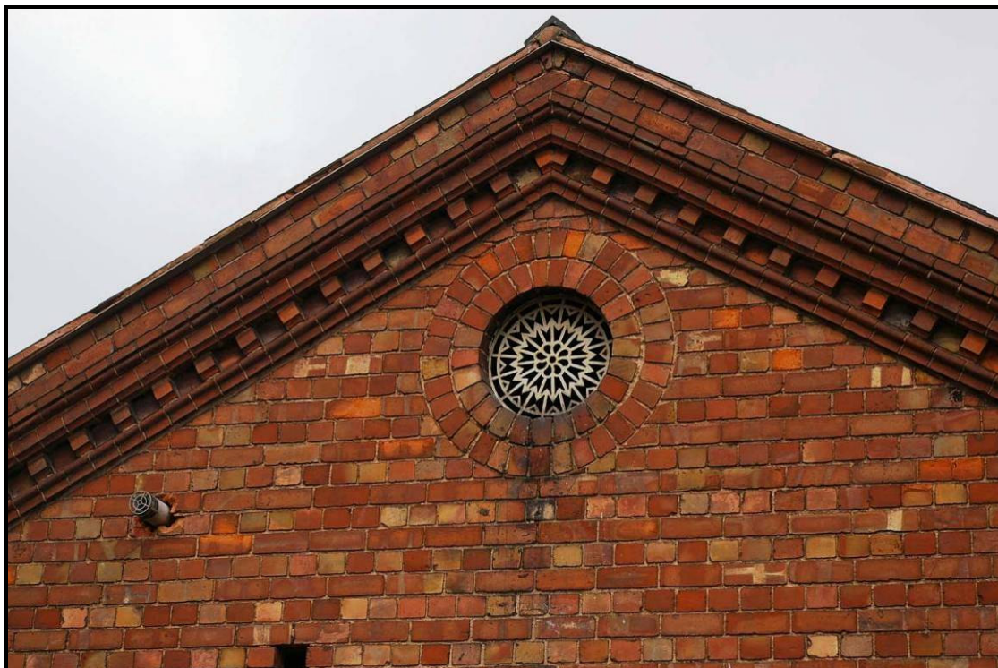
Figure 66: Detail of cast-iron vent on the northern gable of Building Q
