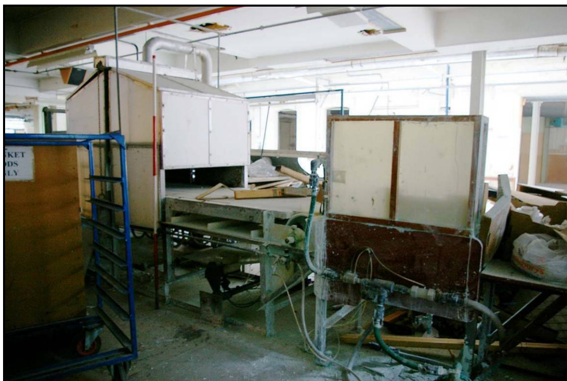
Figure 151: Ground floor of Building S, looking north towards Building N
