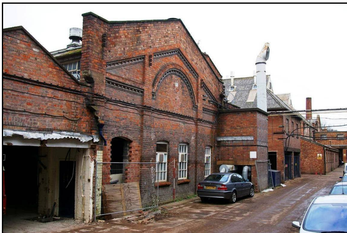
Figure 29: West elevation of Building N, looking north-west
