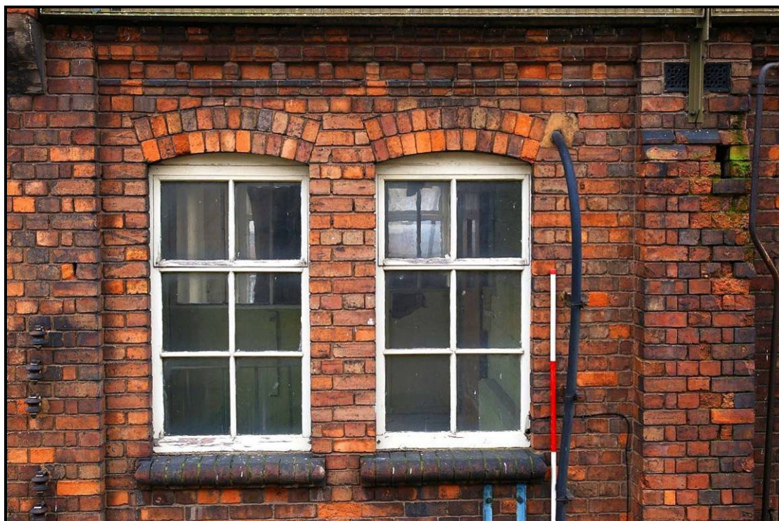
Figure 105: Detail of windows on the second floor of Building R
