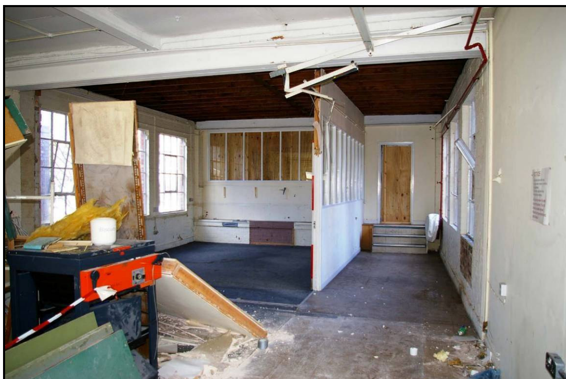
Figure 82: Southern bridge on the first floor of Building Q, looking west
