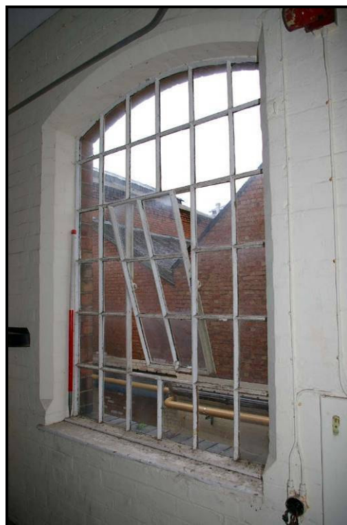
Figure 85: Window on the first floor
