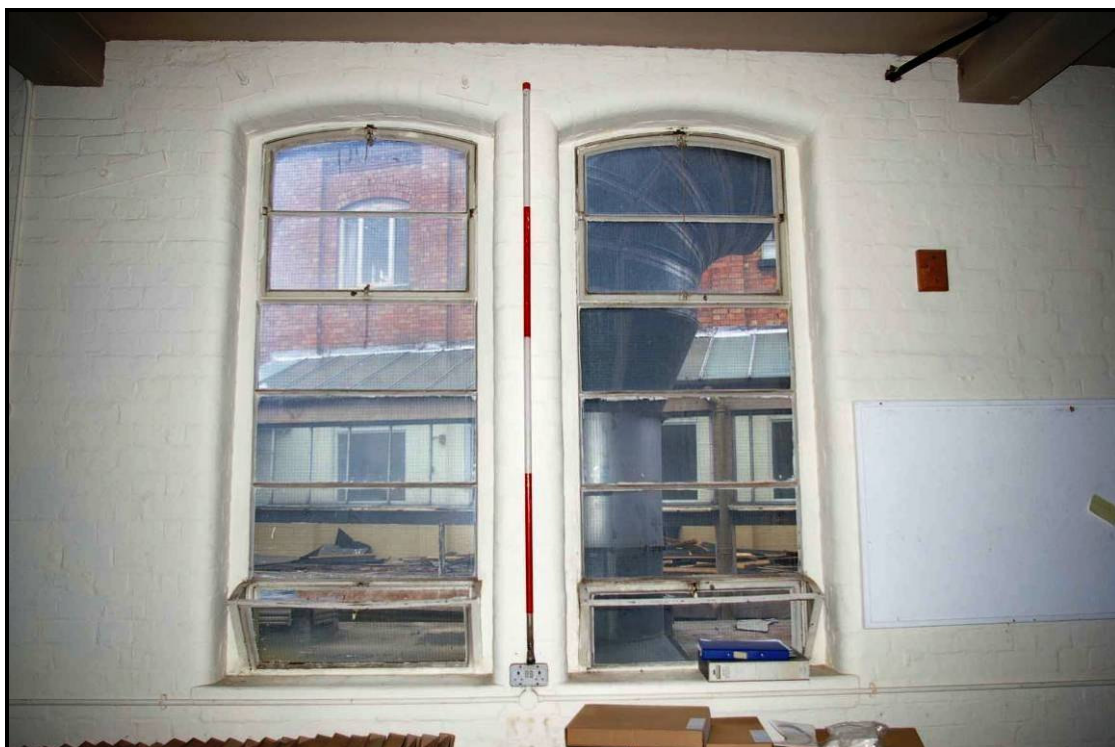
Figure 125: Detail of windows of the first floor of Building R, looking west
