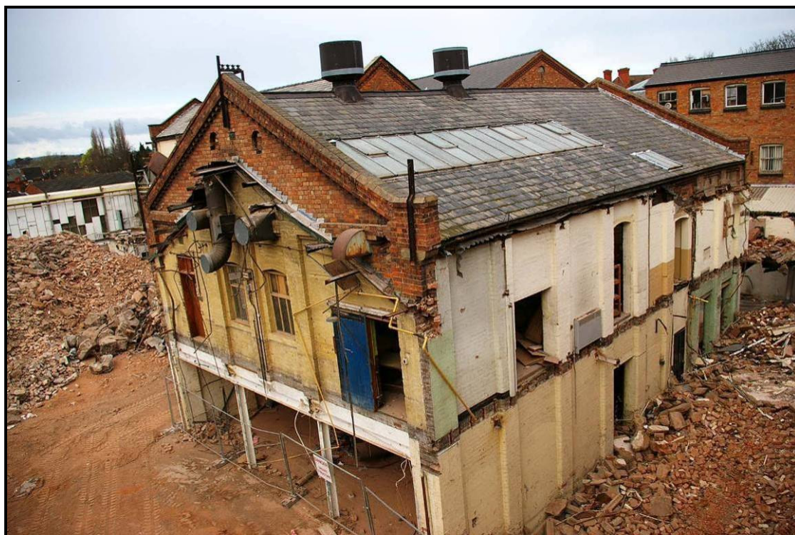
Figure 14: North and east elevations of Building M
