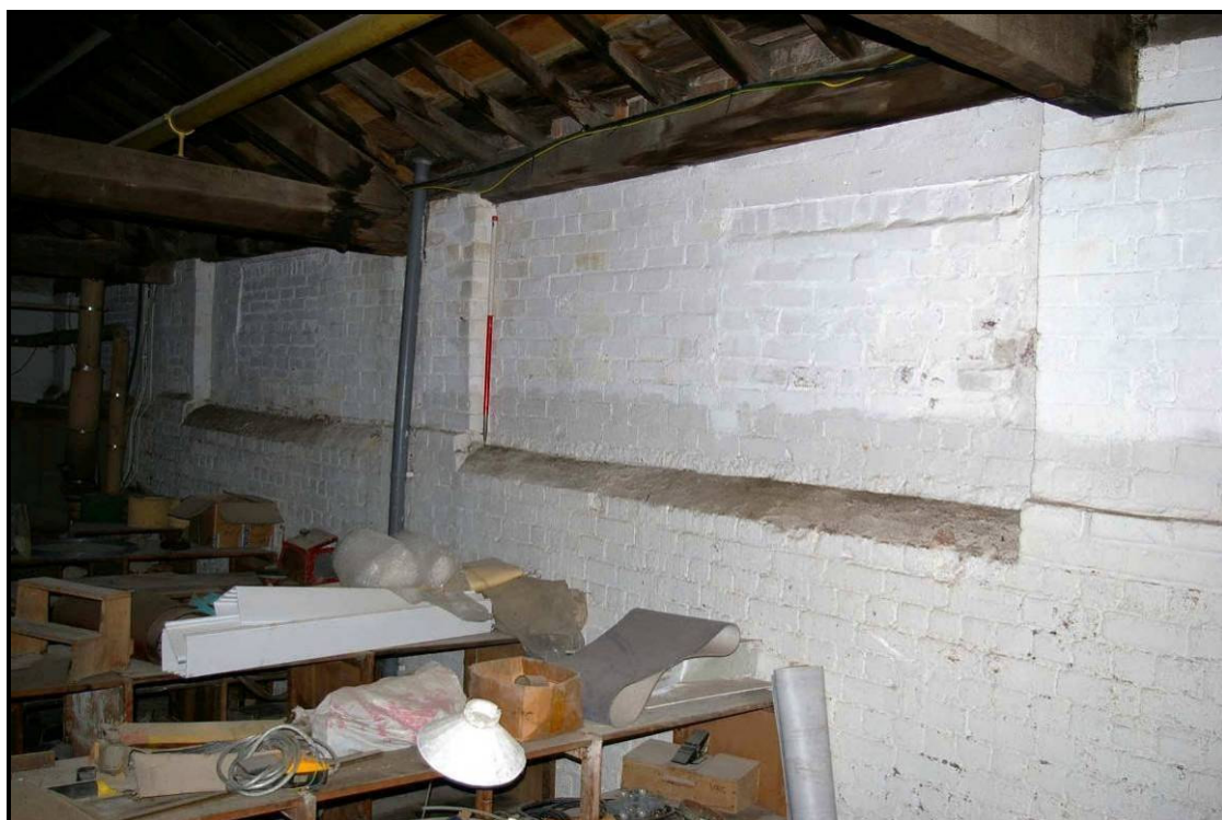
Figure 171: Boundary wall with blocked chutes, looking south-east
