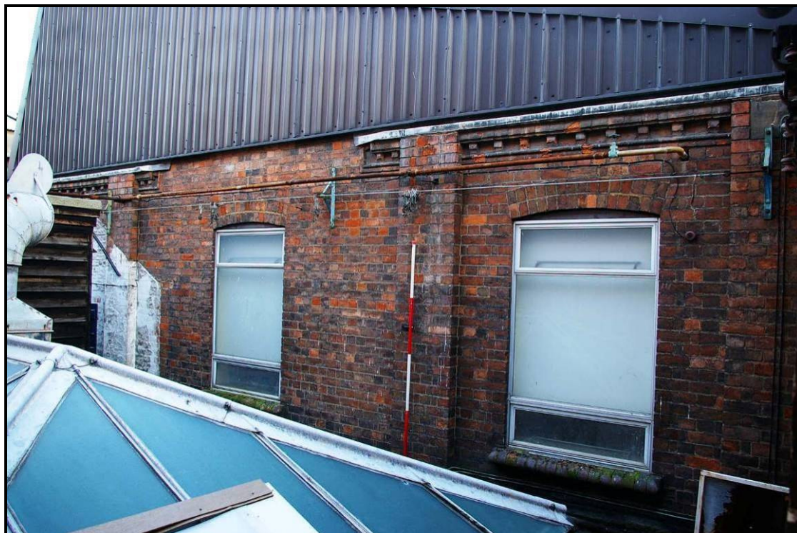
Figure 145: West elevation of Building S
