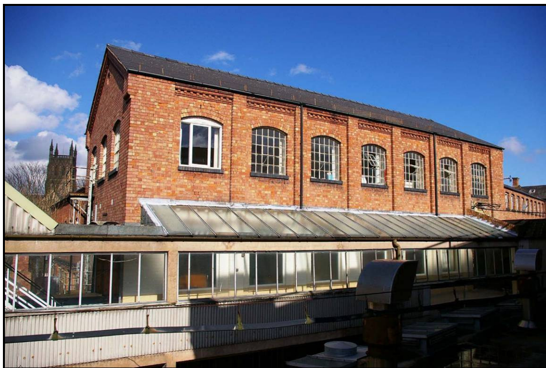
Figure 57: East elevation of Building Q
