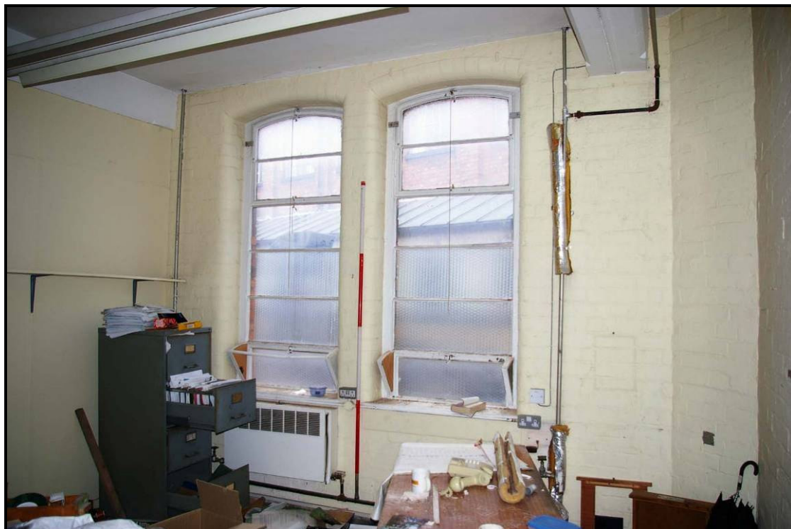
Figure 122: Office on the first floor of Building R, looking west
