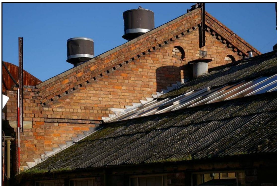
Figure 5: Detail of the eastern gable of Building M
