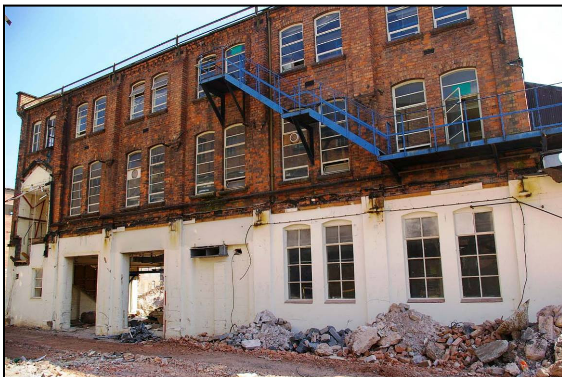
Figure 113: West elevation of Building R, after demolition of Building P
