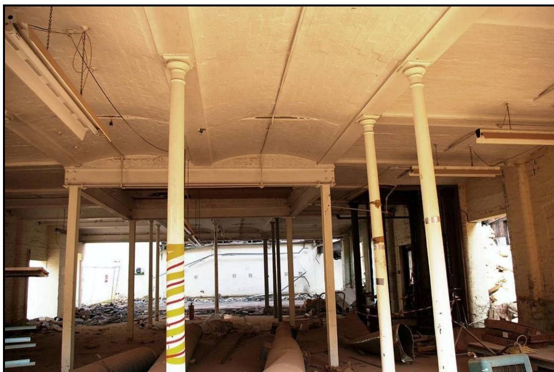
Figure 18: Ground floor of Building M, looking west
