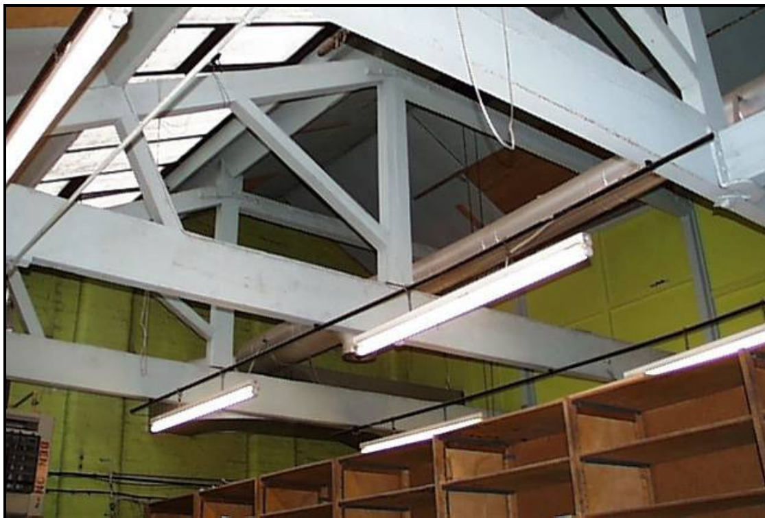
Figure 25: Queen-post trusses on the first floor of Building M, looking east
