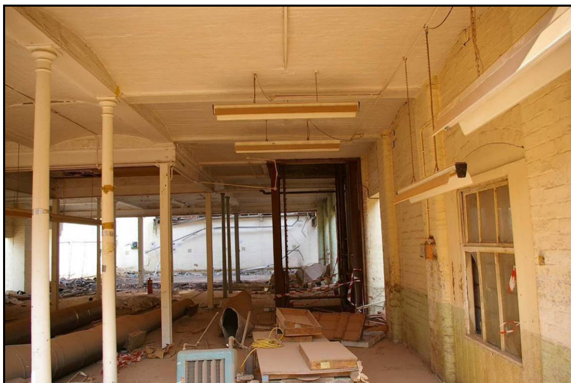
Figure 19: Northern bay on the ground floor of Building M, looking west
