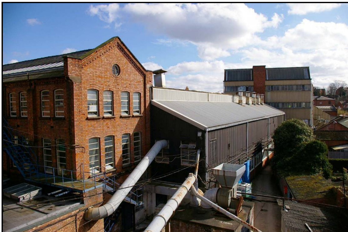
Figure 101: South elevation of Building R viewed from Building U
