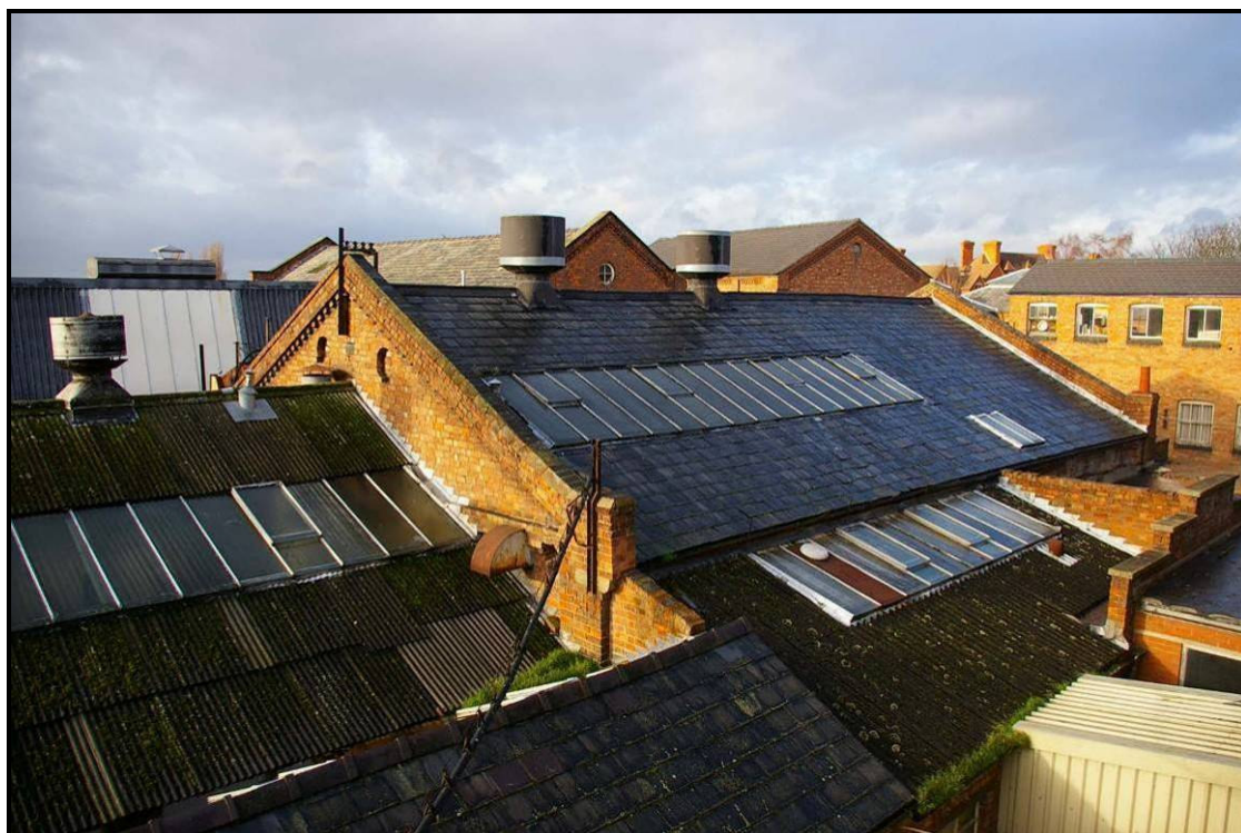
Figure 4: Eastern gable of Building M, from Building K1
