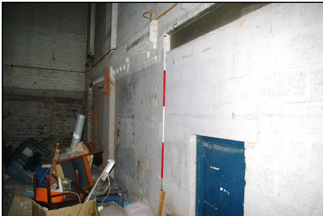
Figure 163: Detail of the dentilled cornice, looking south
