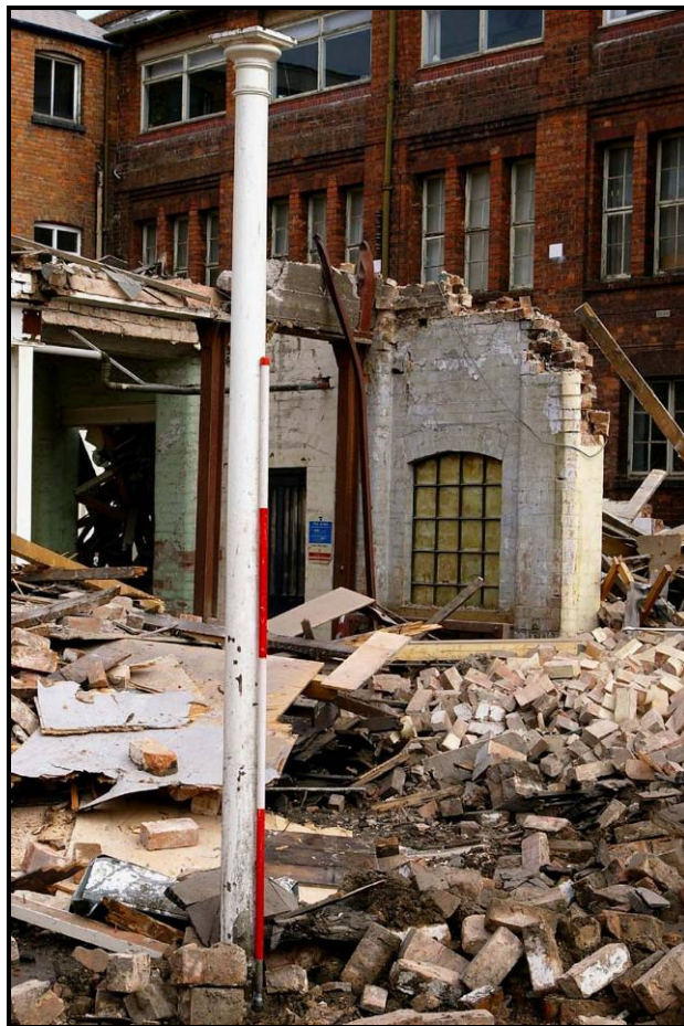
Figure 23: Detail of cast-iron column
