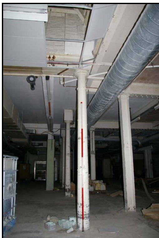
Figure 154: Row of cast-iron columns
