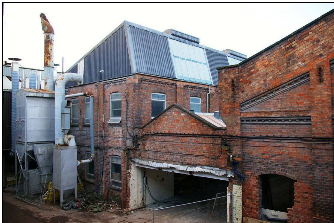
Figure 146: North and east elevations of Building S
