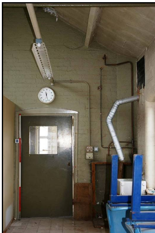
Figure 130: Partition wall of staircase
