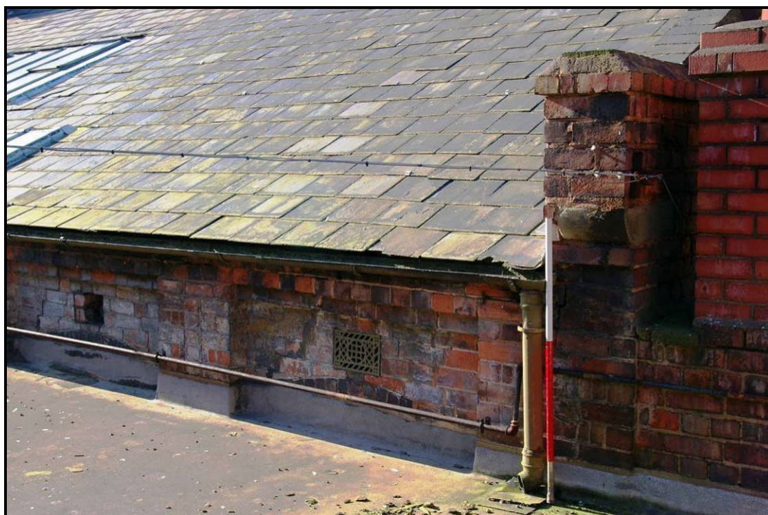
Figure 11: Detail of kneeler stone on the west elevation of Building M
