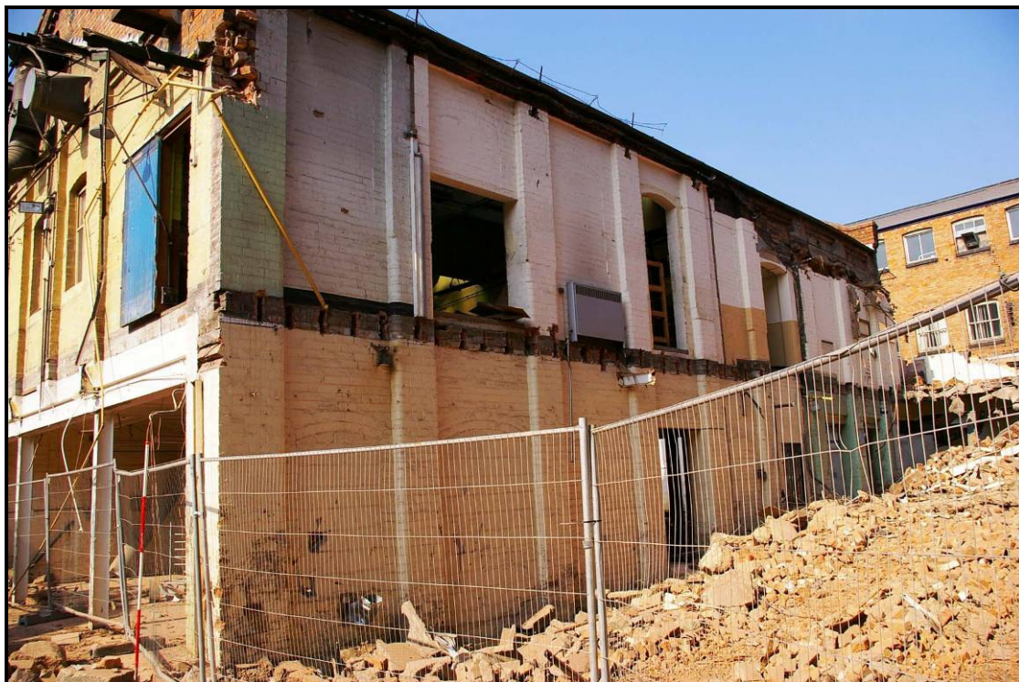
Figure 15: North elevation of Building M
