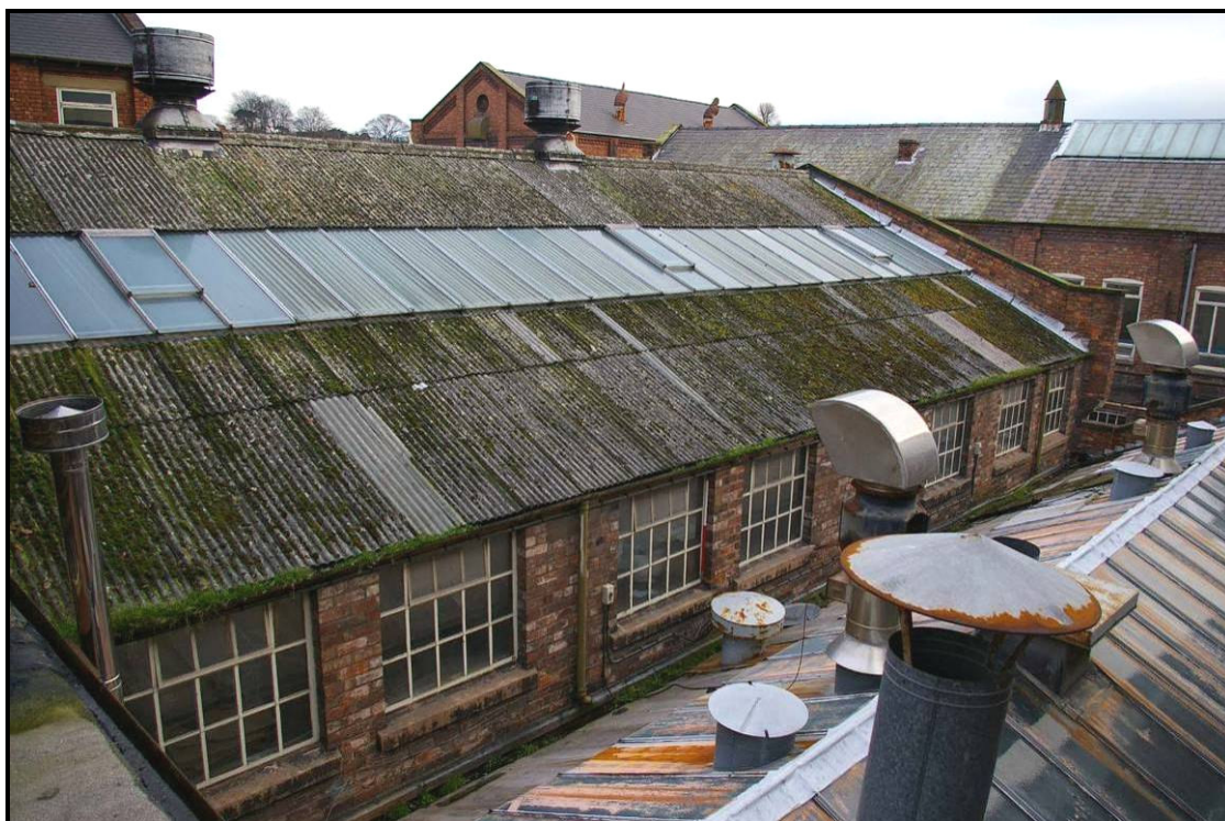
Figure 37: First floor of the south elevation of Building N
