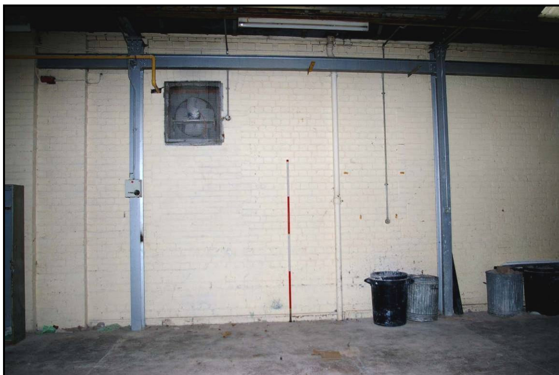
Figure 150: Blocked windows on the south elevation of Building S
