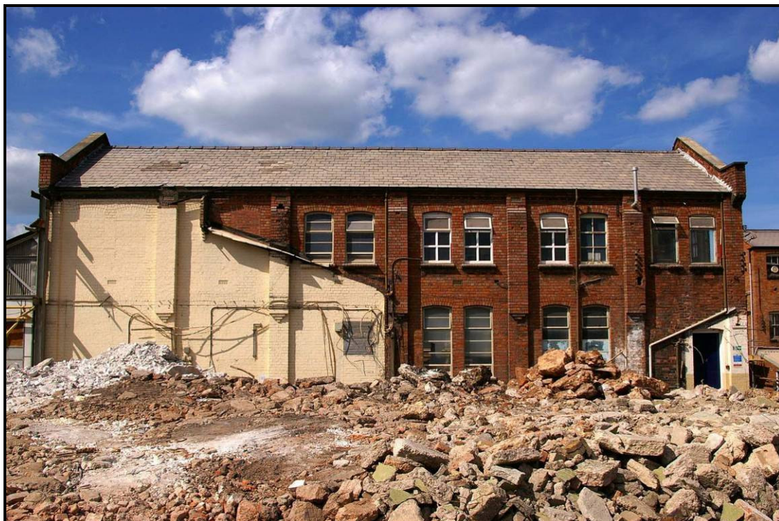
Figure 109: East elevation of Building R after demolition of adjacent buildings
