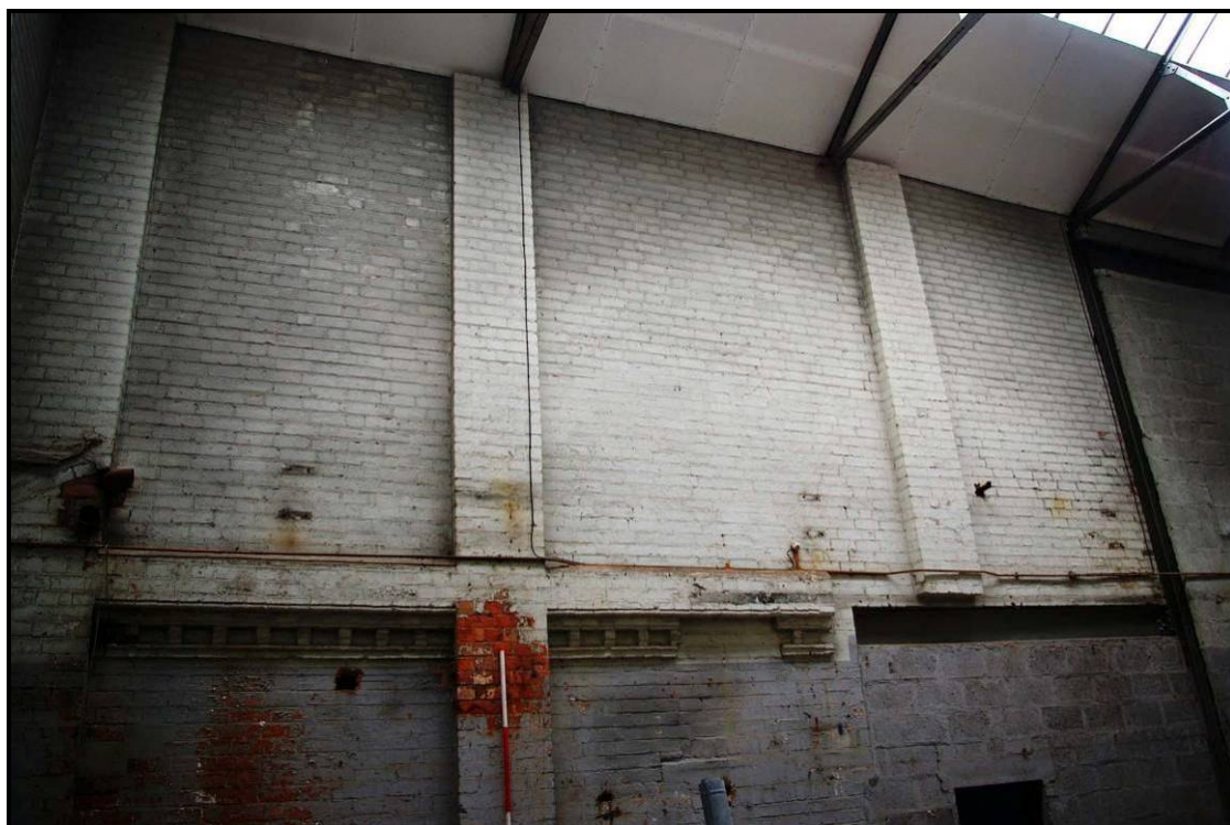
Figure 164: Ghost gable of the New Mould Shed
