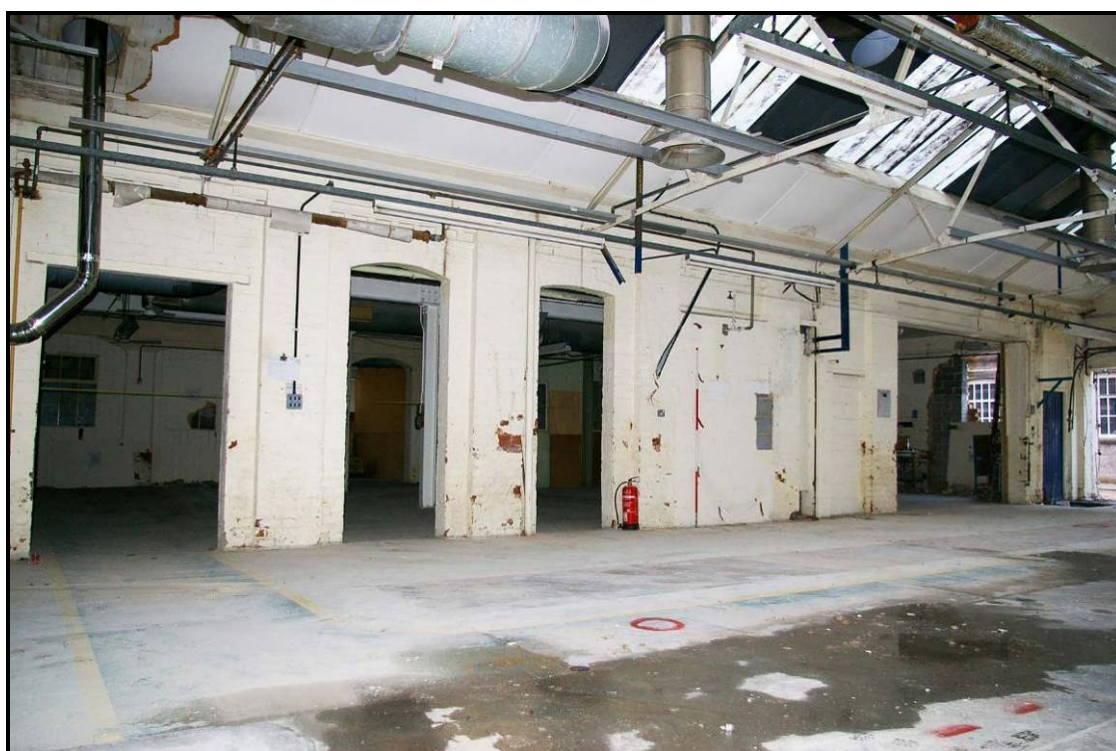
Figure 33: South elevation of Building N, looking north-east
