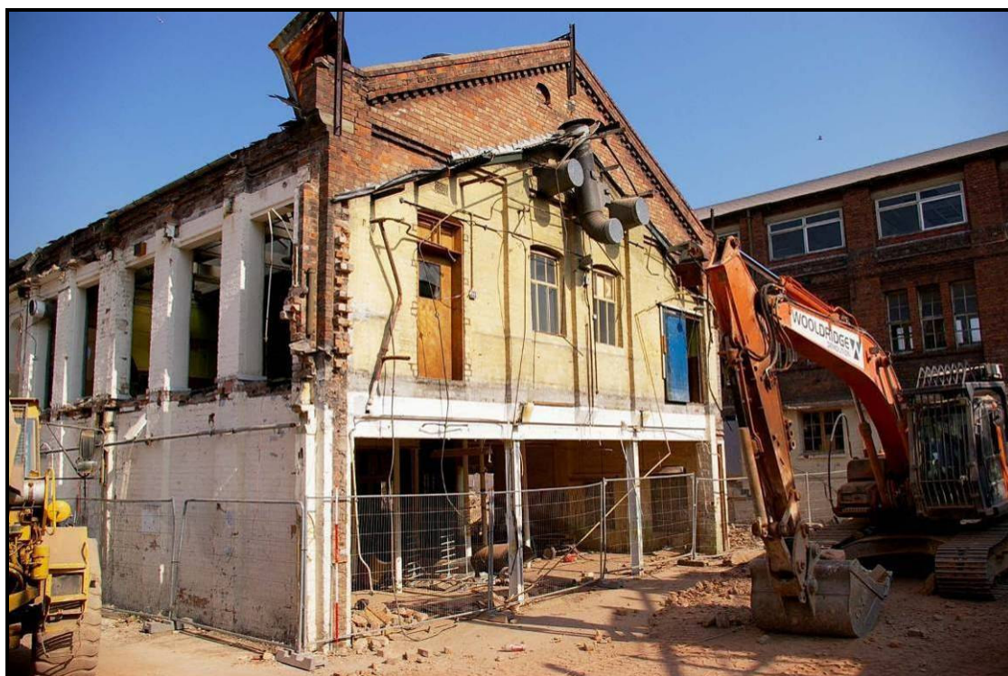
Figure 7: East and south elevations of Building M
