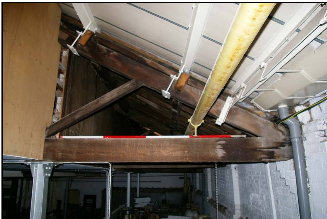
Figure 167: Southern end of original timber truss set on later brickwork
