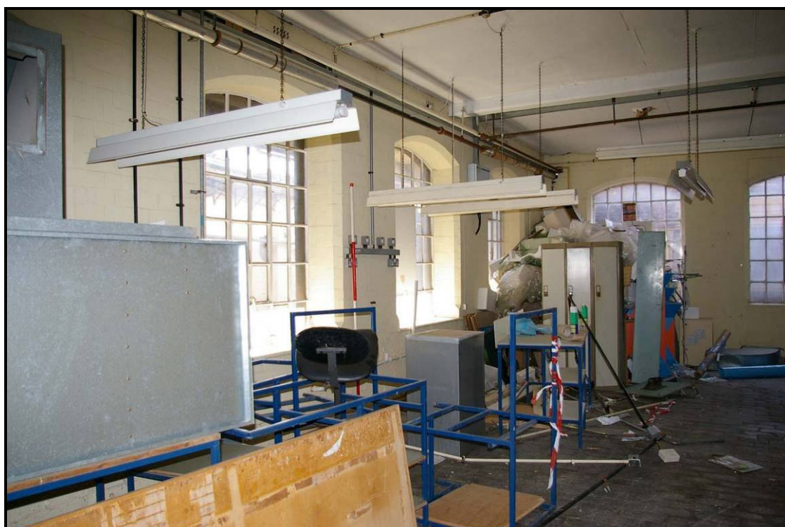
Figure 73: Ground floor of Building Q, looking south-east
