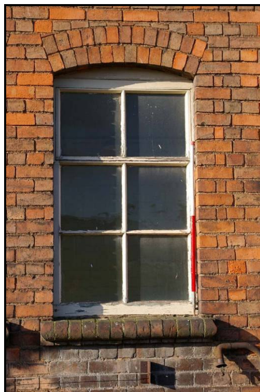
Figure 99: Window on the second floor
