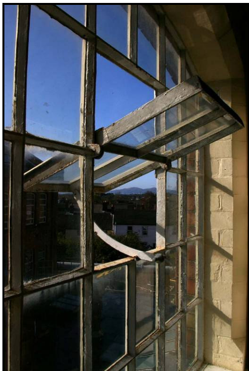
Figure 89: Detail of handle of window opening
