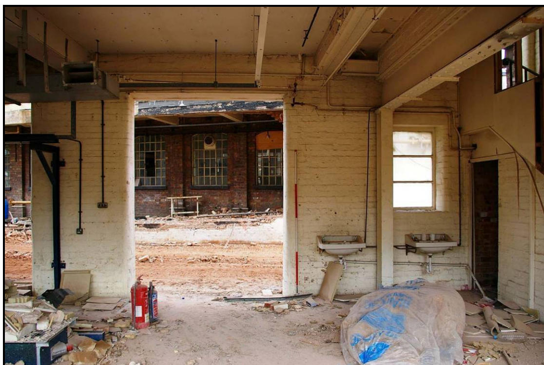
Figure 115: Ground floor of Building R showing opening to Building P
