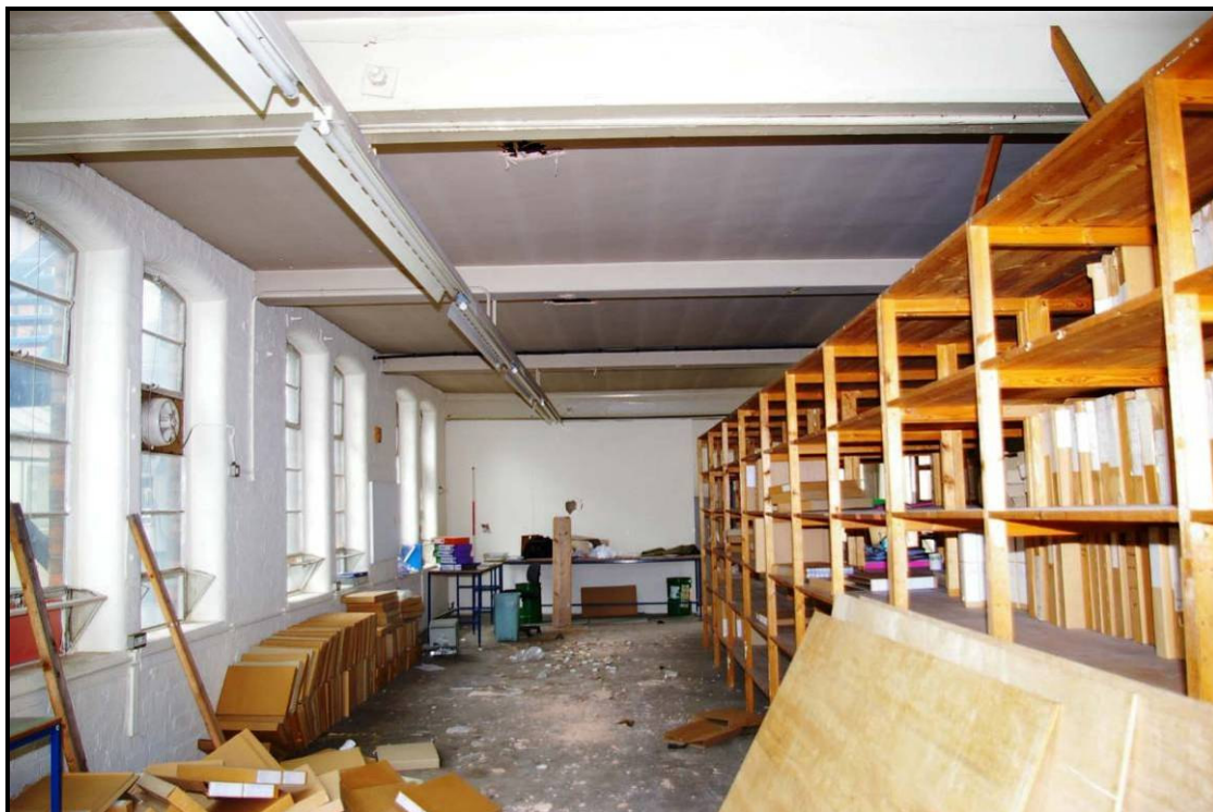
Figure 124: General view of the first floor of Building R, looking north
