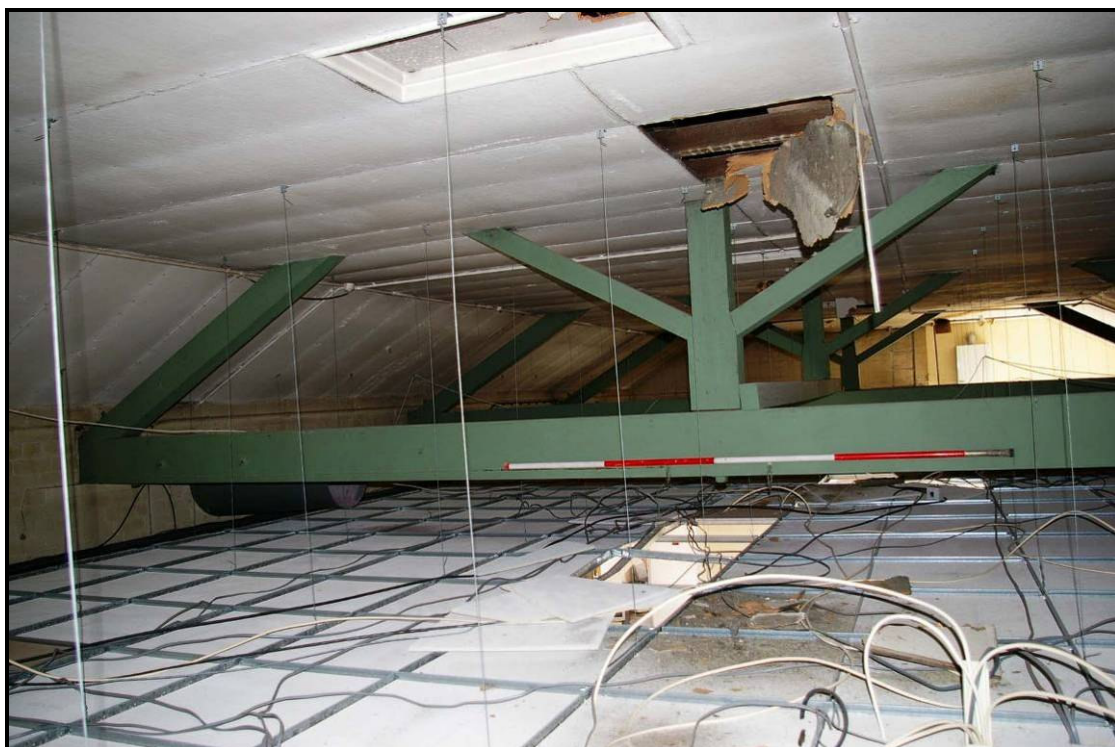
Figure 93: King-post trusses over the suspended ceiling
