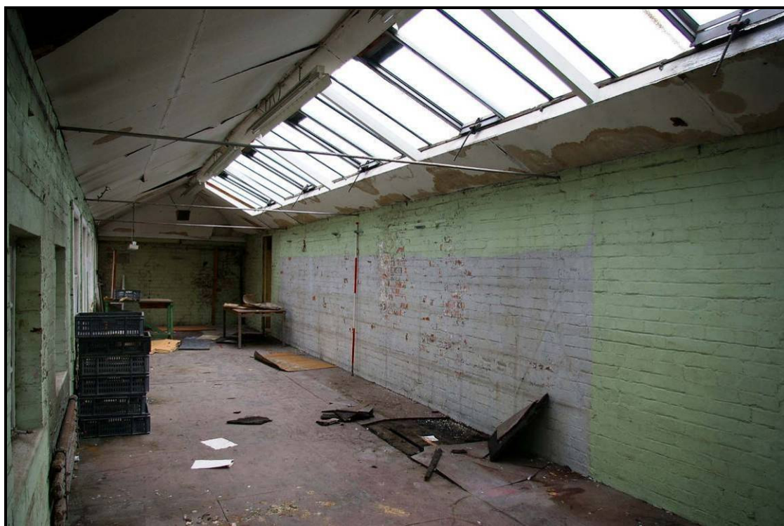
Figure 42: The first floor of the north elevation with internal blocked windows
