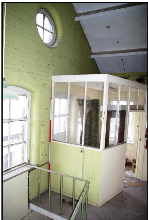
Figure 129: Landing of the second floor
