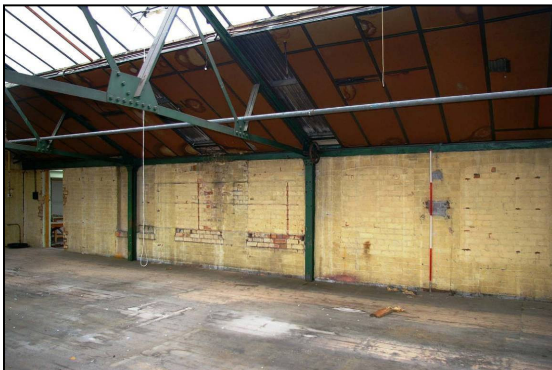
Figure 53: North wall of the first floor of Building N
