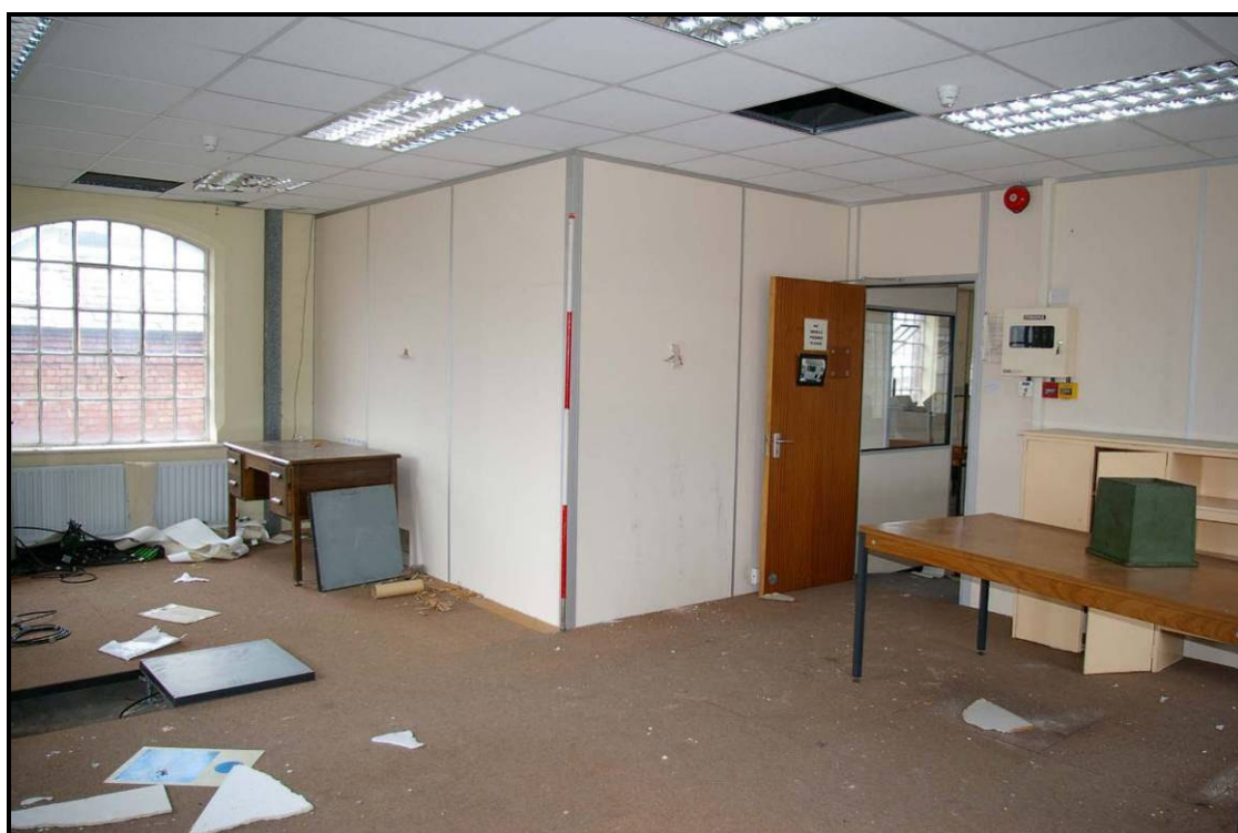
Figure 86: Southern office on the second floor of Building Q, looking north-west
