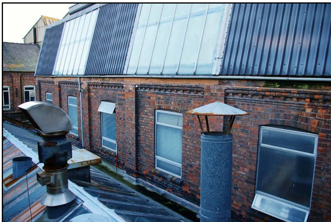
Figure 147: North elevation of Building S, looking south-east
