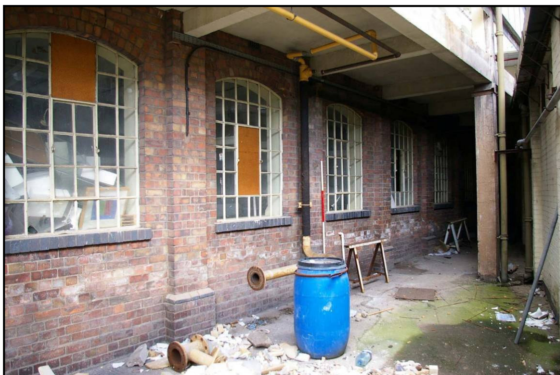
Figure 59: Ground floor of the east elevation of Building Q
