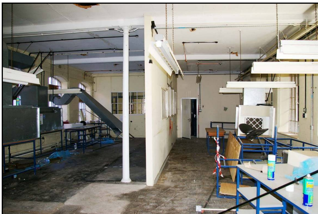
Figure 72: Ground floor of Building Q, looking north
