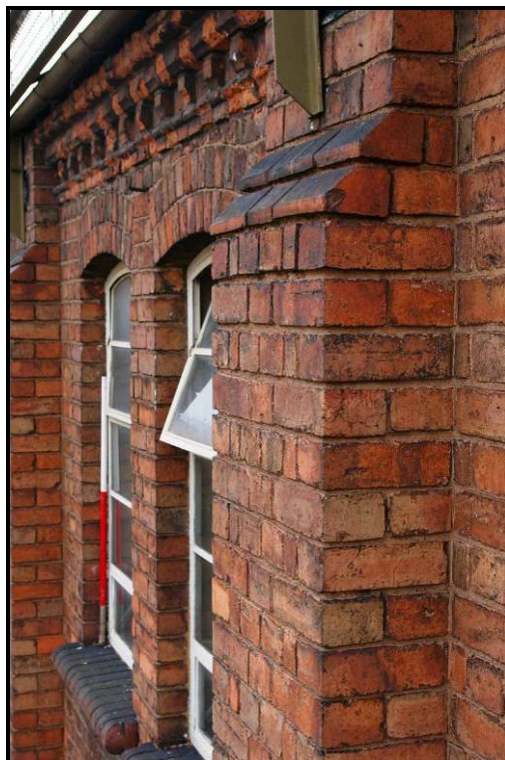
Figure 107: Detail of pilaster and cornice
