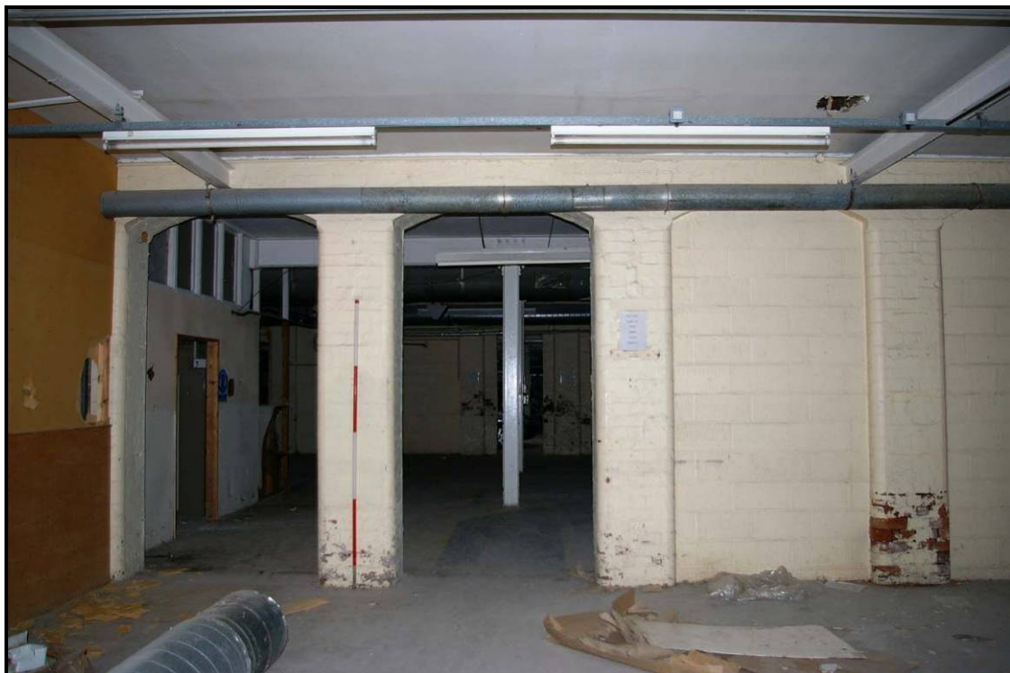
Figure 41: Western end of the north elevation of Building N
