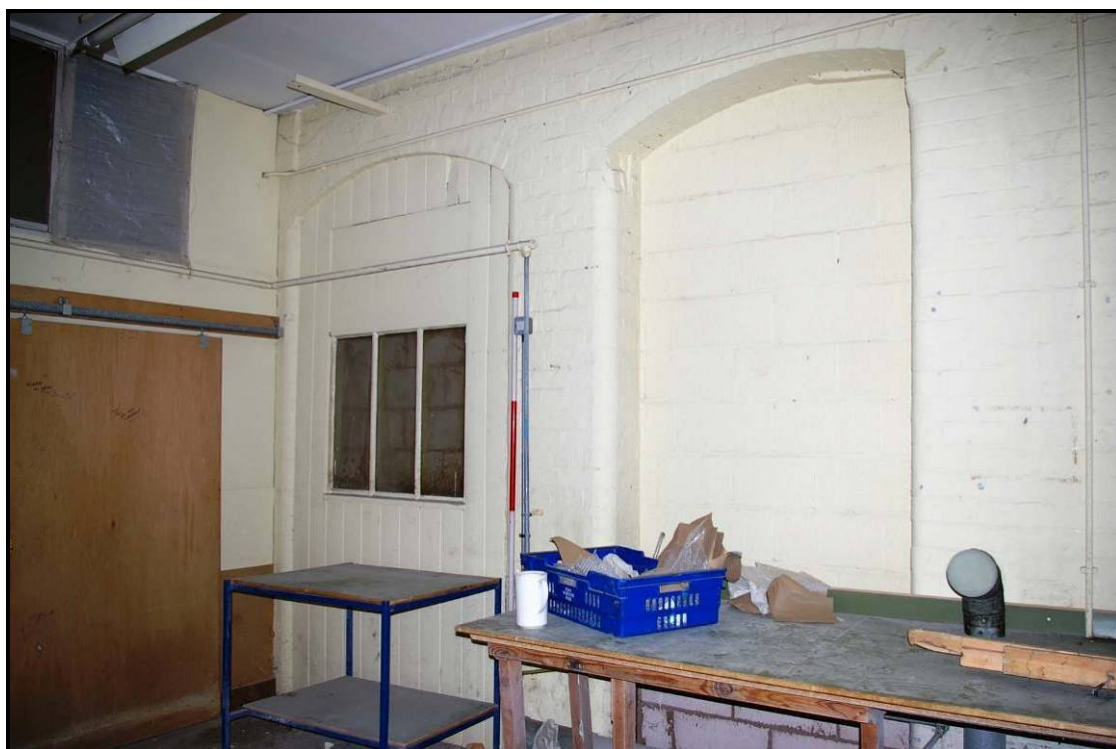
Figure 45: North wall of the ground floor of Building N
