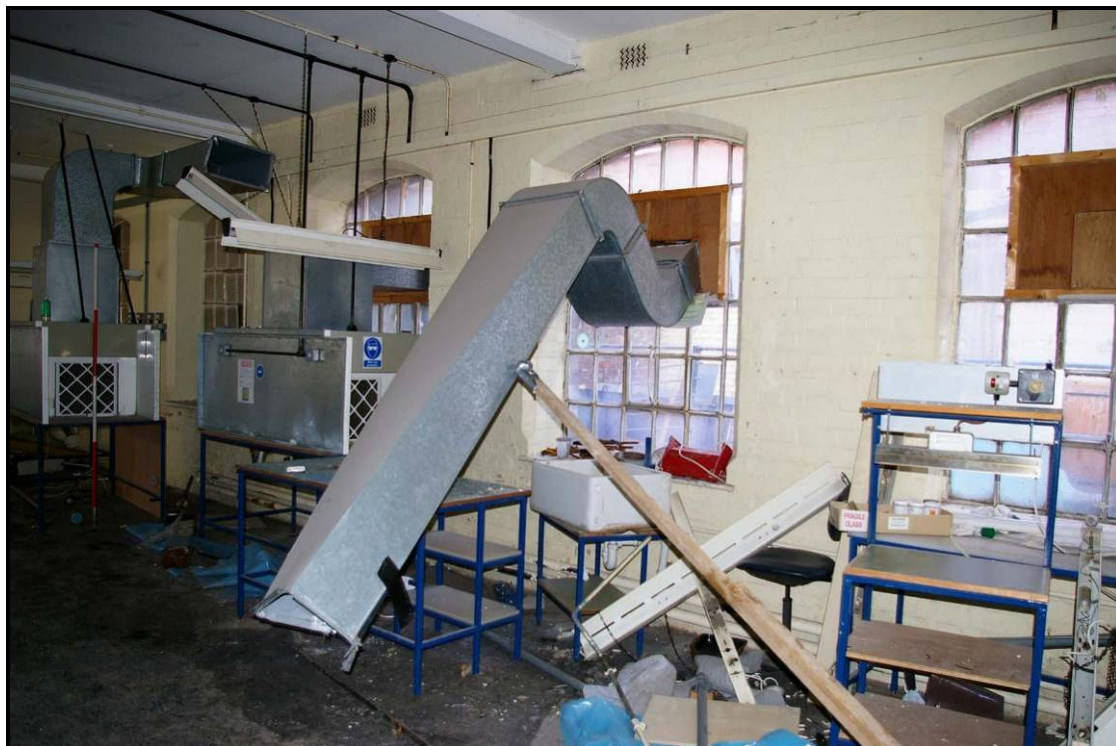
Figure 74: West wall of the ground floor of Building Q
