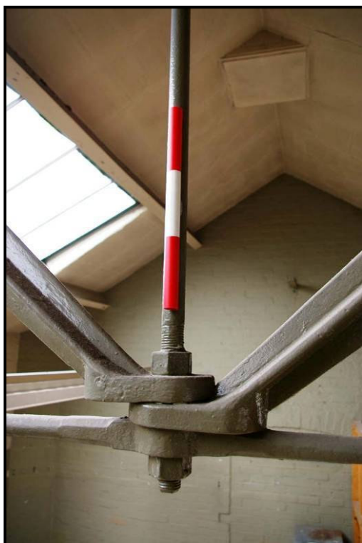
Figure 134: Detail of interlocking bolt
