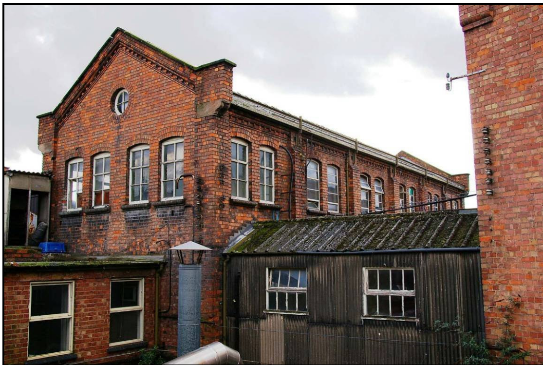
Figure 97: North and west elevations of Building R
