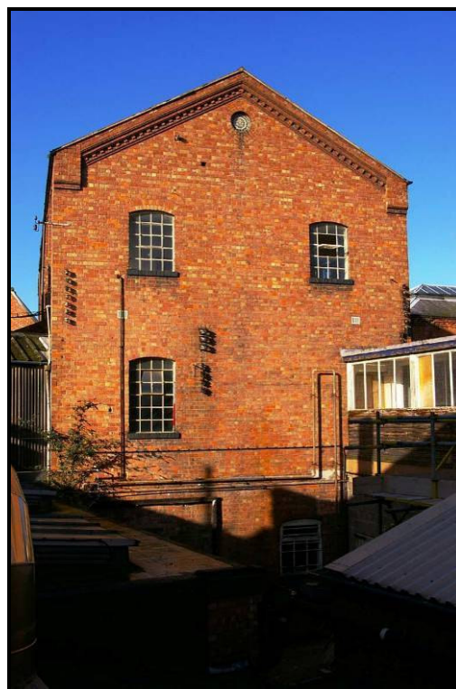
Figure 63: North elevation of Building Q
