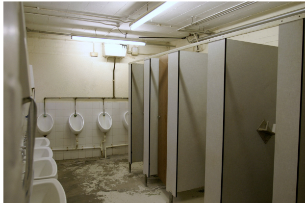
Figure 39: Building L. Part of the male lavatories.
