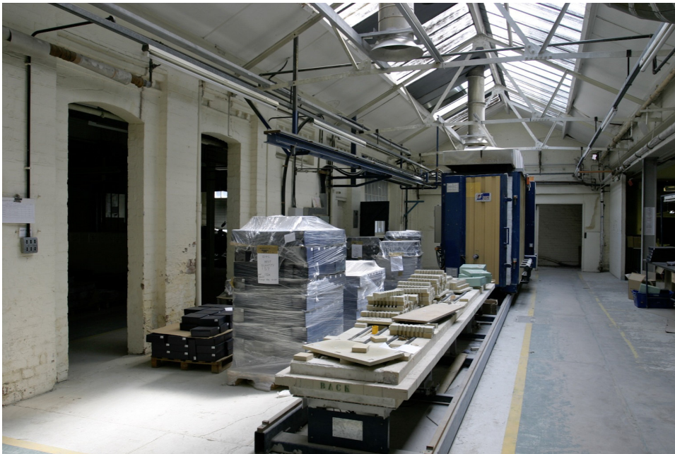
Figure 25: Interior of Building O, looking east. Building N is to the left (with dentil course) and Building S to the right (with corbelling). A tunnel kiln lies in the centre.
