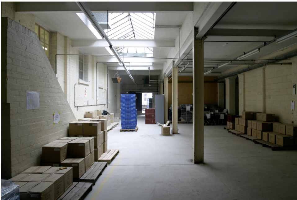
Figure 49: Building L, interior, looking east. The 1951 tunnel kiln lay to the right. To the left lies the wall to Building J and to the right the wall to Building N. The stairs on the left were originally external. Note the lantern light as shown in Figure 43 and underpinning for the extant wall above.
