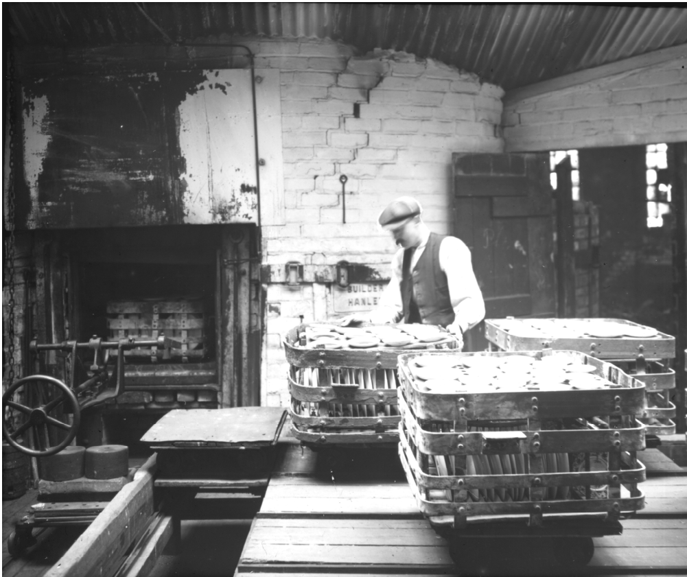
Figure 10: Enamelling kiln under a corrugated-iron roof as originally built for Building N (source: Worcester Porcelain Museum)
