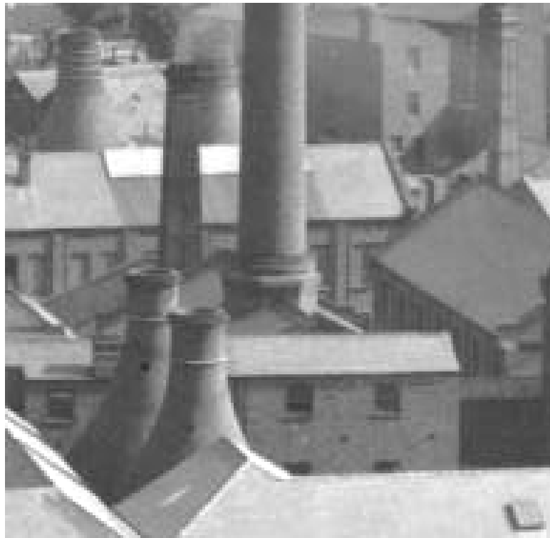
Figure 5: Buildings M and N viewed from the top of the Cathedral. The large round chimney belongs to M and the square chimney behind to N (detail from a photograph held by the Worcester Porcelain Museum).
