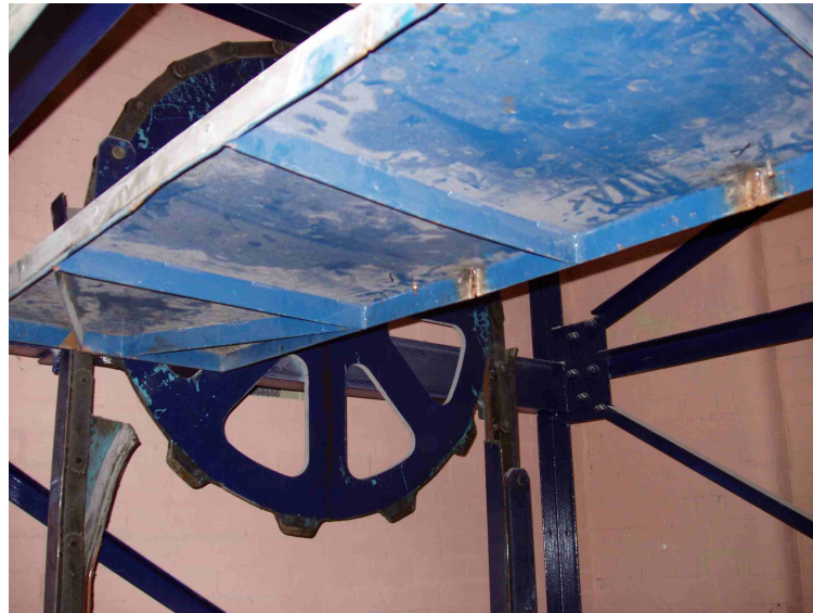
Figure 14: The wheel for the dumb waiter engaged in a chain to control the rate of ascent and descent
