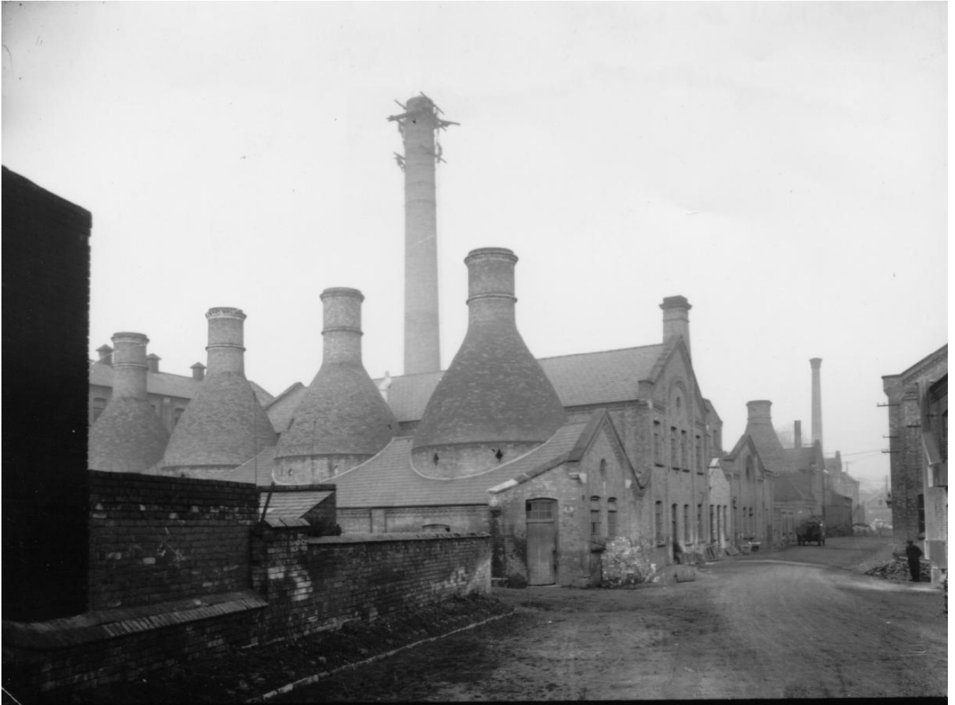
Figure 7: Prince's Drive from the south-east showing some of George Ford's fronts around 1923 when the chimney to M was repaired. The kilns belong to Building T with S beyond, followed by O and N. The chimney stacks to Buildings N (right, just behind the gable of S can just be seen (source: Worcester Porcelain Museum).
