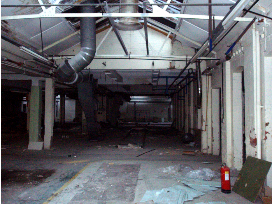
Figure 24: Building O looking west into Building P showing the ceiling from M as extended around 1941
