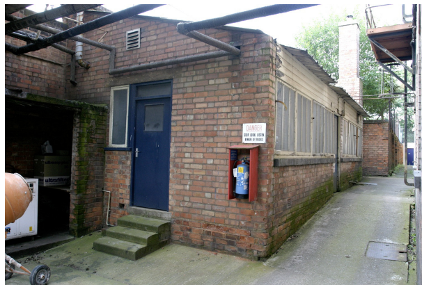
Figure 10: The Acid Shop from the east
