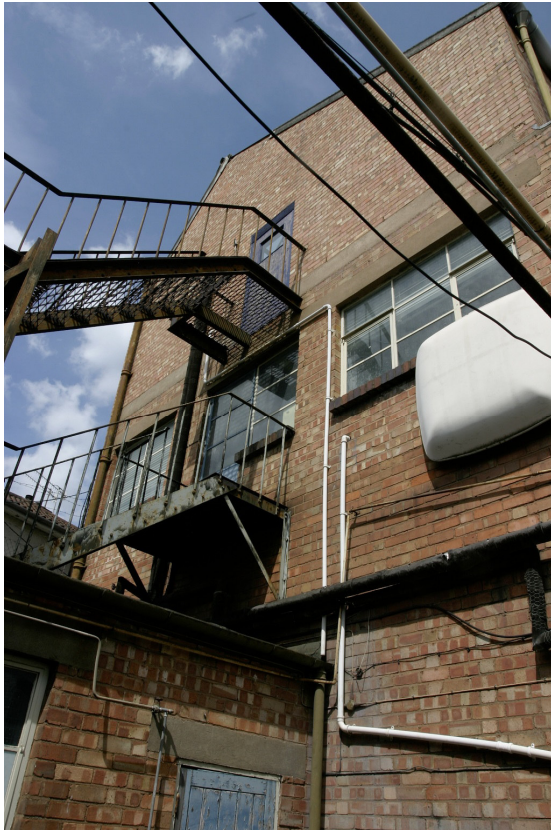
Figure 20: The south elevation of Building U with the asymmetric roof
