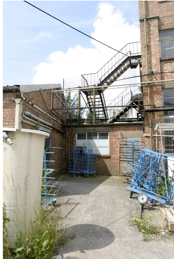
Figure 21: The fire escape as planned in 1970 for Building U with the single storey part of the original building
