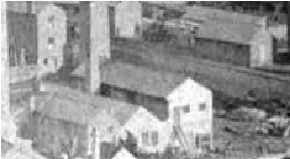
Figure 3: The areas of Buildings W, Y and Z before 1884, looking from the north-west. Mill Street runs diagonally from right to left with the embryonic Albion Mill beyond. To the left (in parallel lines from left to right) lie the 'Store/Plaster House', the 'Frit Kilns and Mixing House' and 'Slip Kilns'. The Bone Houses lie behind (source: Worcester Porcelain Museum).
