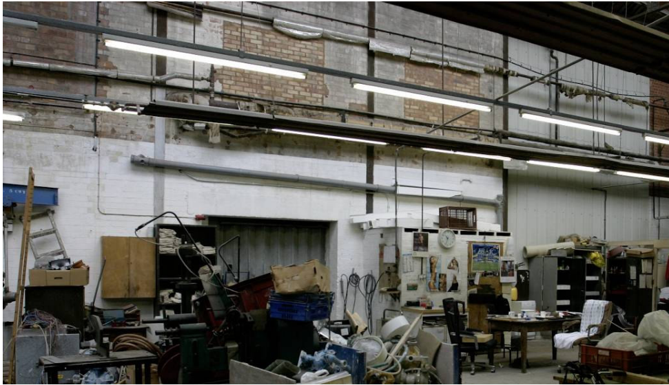
Figure 44: Looking north-east in Building Z towards the division between Buildings W and Z showing the first storey filled windows of the 1937 north elevation which would formerly have looked onto a yard the other side. This became the common wall to Buildings W1 and W2.
