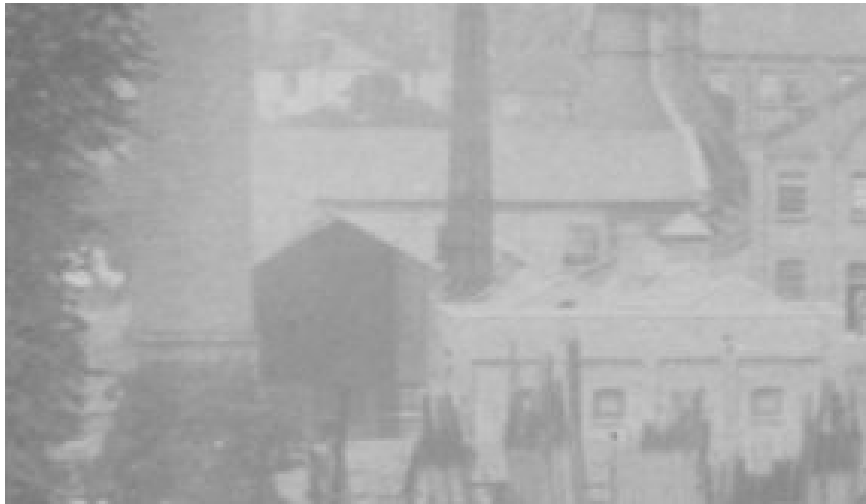
Figure 21: Looking at the area of Buildings W1 and W2 from the east c1900.
