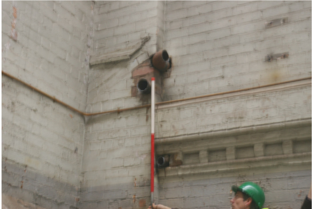
Figure 8: Building Z. Dentil course on the east wall with ghost of gable end
