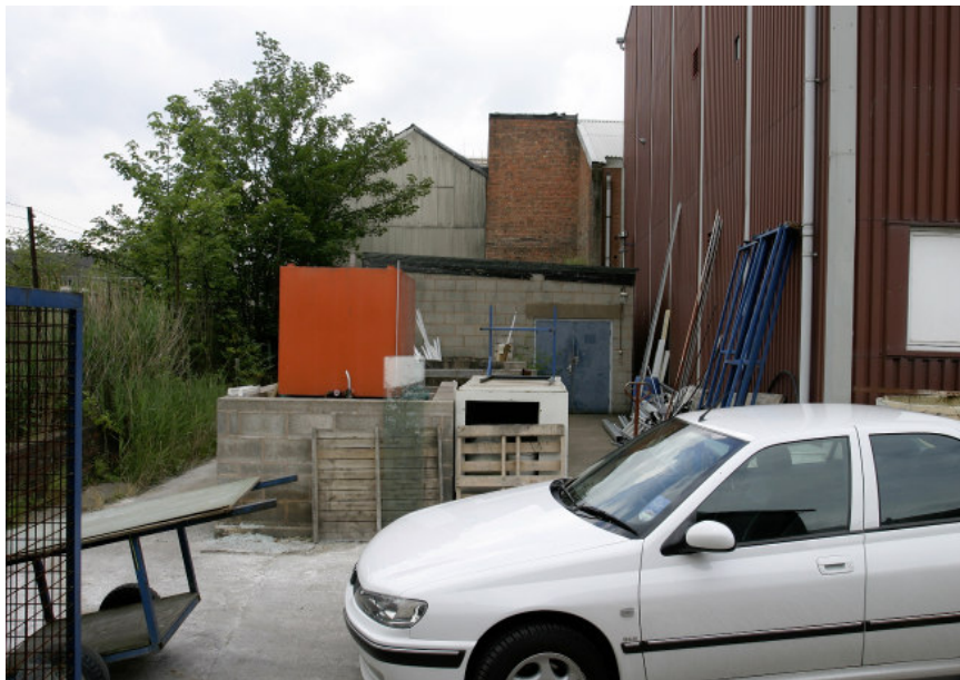
Figure 72: Building W2 (right) looking towards the cross-wing to Building Z. The canal lies to the left. Behind it W2 to the canal were three large oil tanks and a single-storey alternator house, built in 1972 (of breeze blocks with a flat felt roof). The yard was used for storage of kiln furniture.
