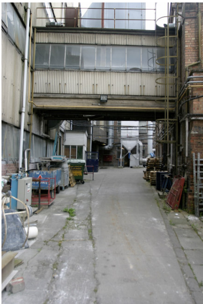
Figure 60: The bridge between Building K3 and W1, looking west
