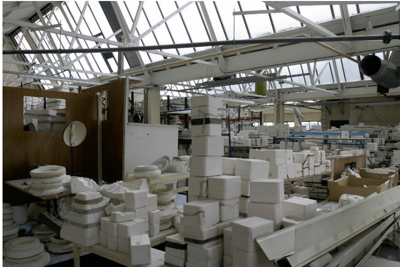
Figure 67: The 'saw-tooth' roof of Building W1, looking south-west. Plate making was on the first floor (together with a tunnel kiln), the cup making shop on the second floor and mould storage on the third floor.
