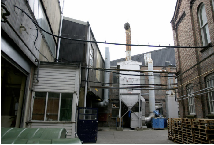
Figure 62: Building K2 (right), Building S (front) with the bridge from Building W1 into Building T (left)
