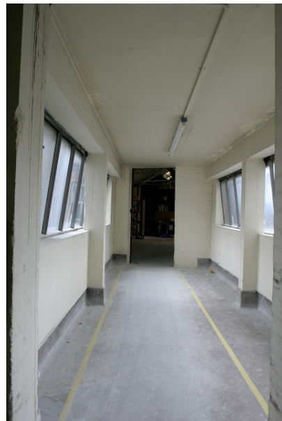
Figure 61: The bridge to Building K3 from Building W1
