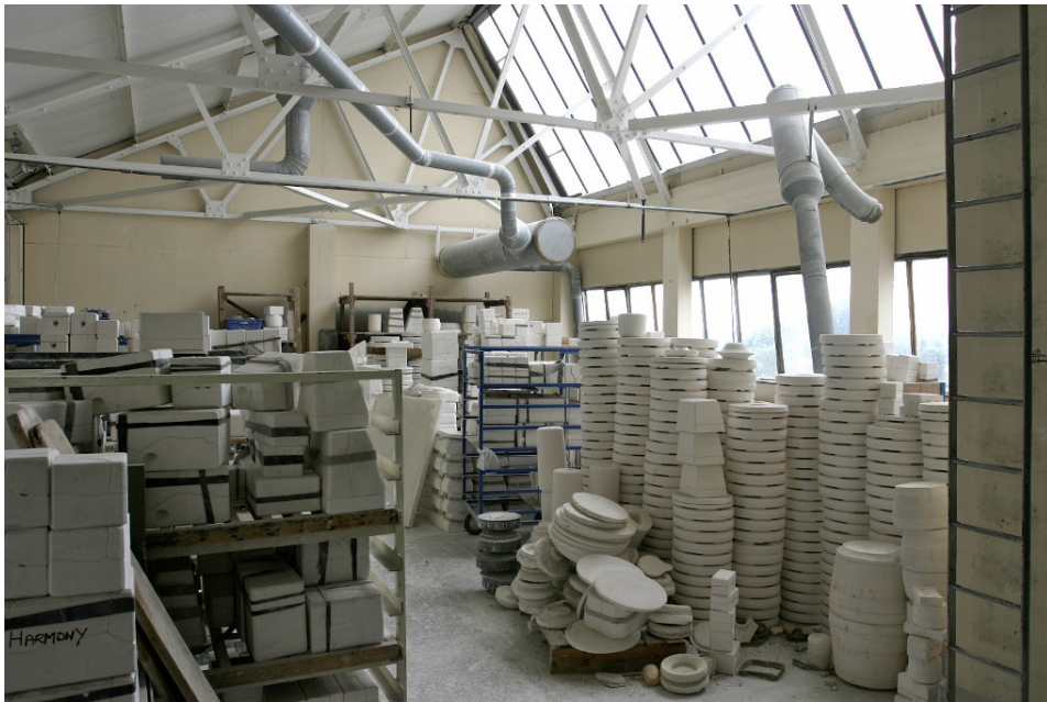
Figure 66: The 'saw-tooth' roof of Building W1, looking south-west
