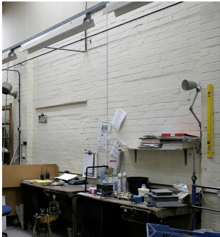
Figure 9: The south wall showing pilasters
