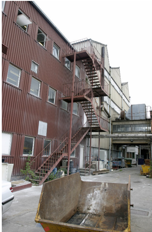
Figure 71: Building W2 with Building W1 beyond with the bridge into Building K3
