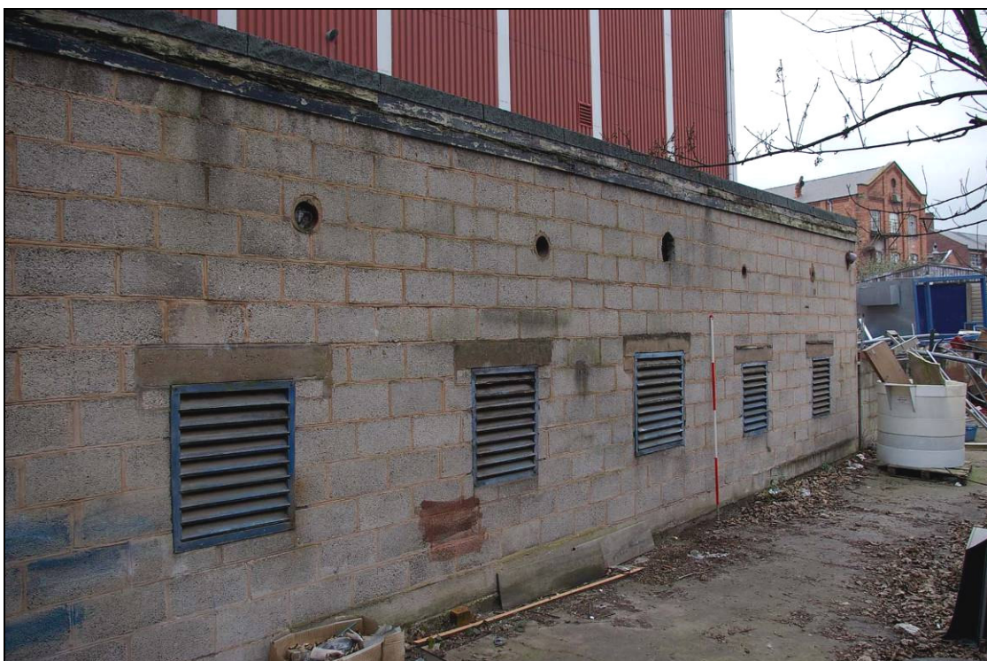
Figure 53: East elevation of eastern block of W2, looking north
