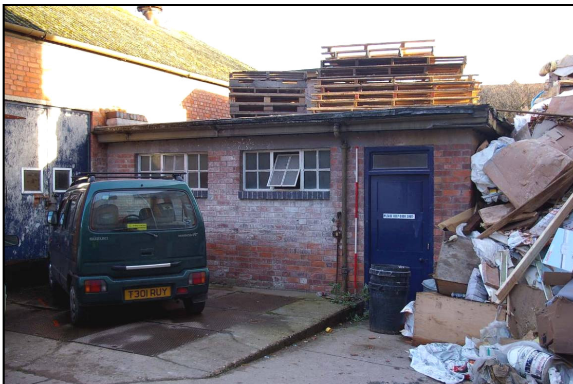
Figure 17: The toilet block of Building I, looking east
