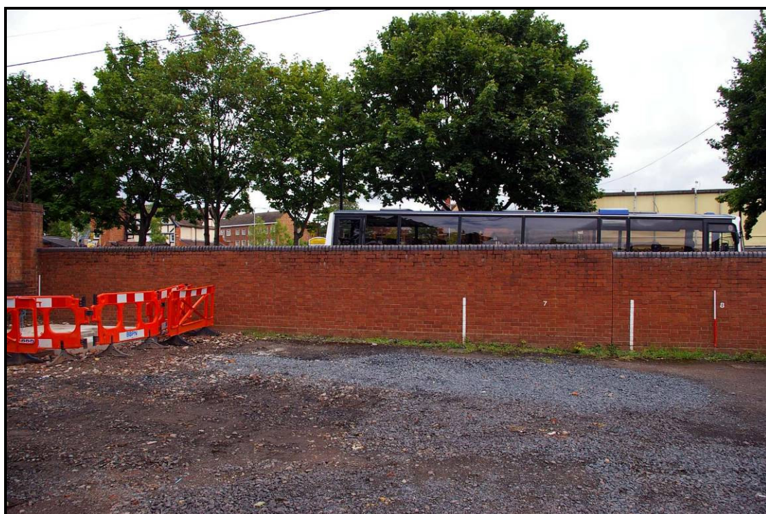
Figure 99: Boundary wall along King Street viewed from the Old School
