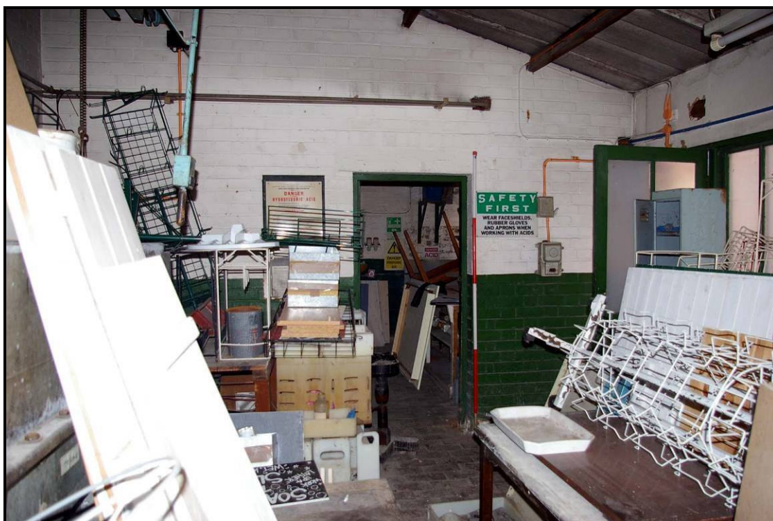
Figure 79: Inside Shed 6, looking west
