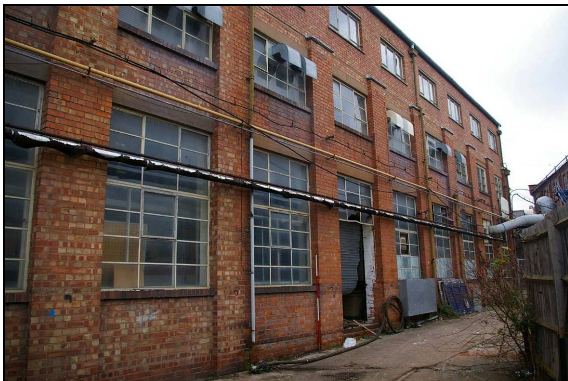
Figure 35: East elevation of Building U
