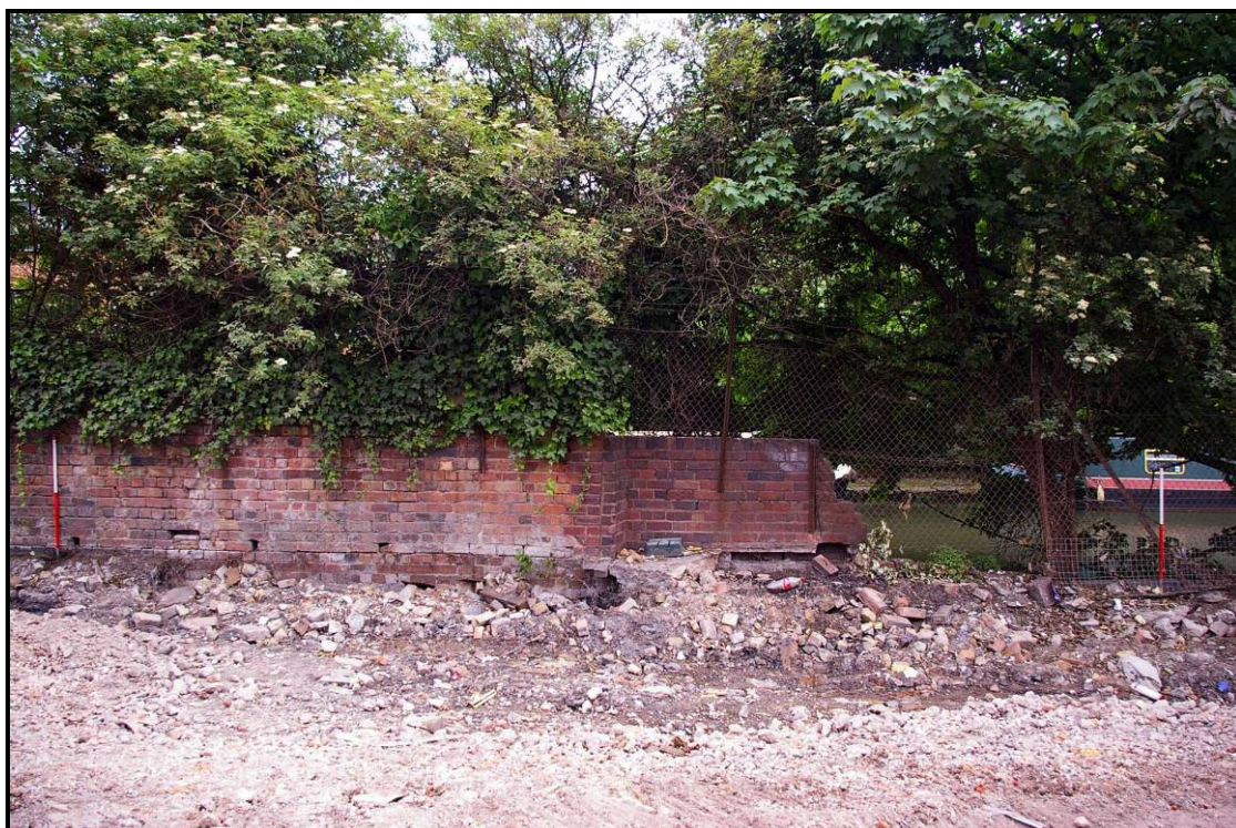
Figure 92: The canal wall on the east of Building K1
