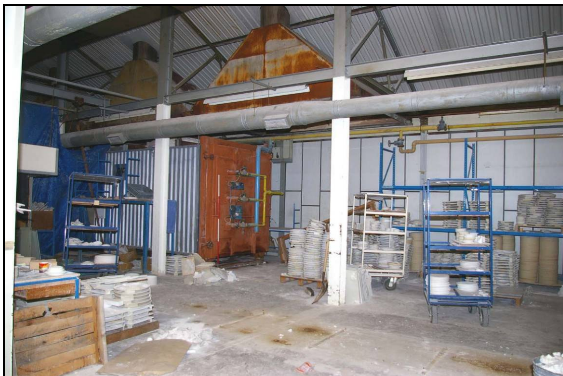
Figure 34: First floor of Building T, looking south
