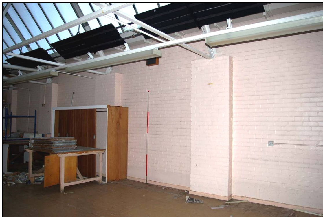
Figure 40: Second floor of Building U, looking south-west
