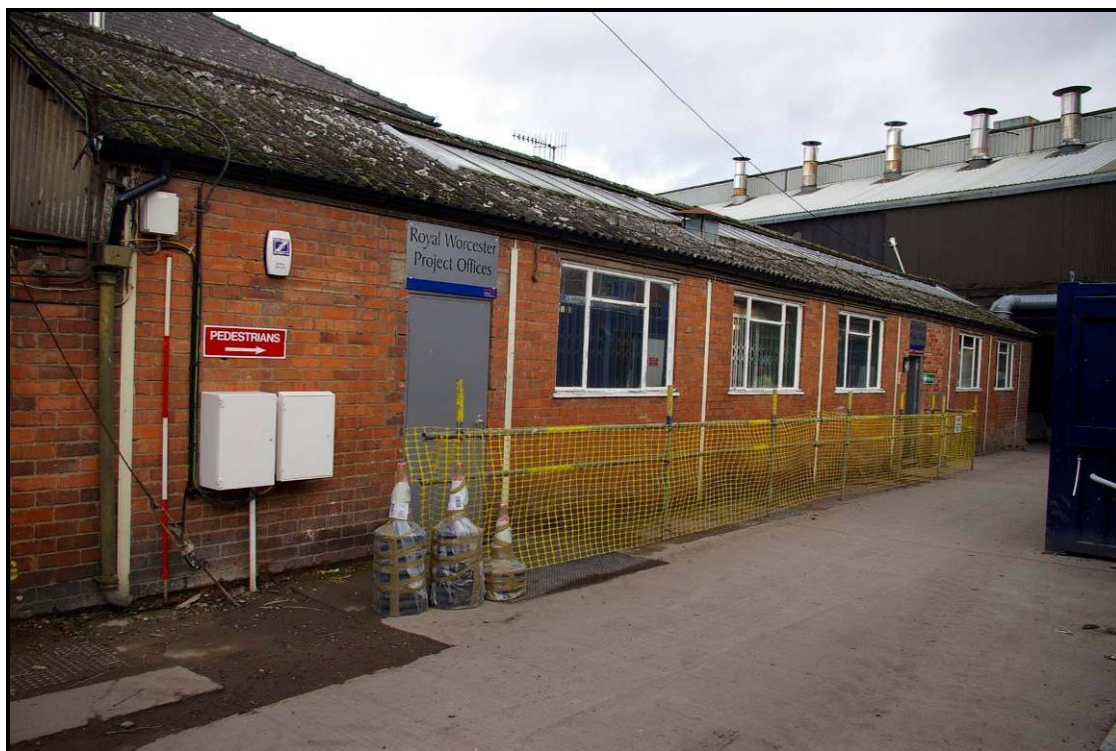
Figure 54: East elevation of Building X
