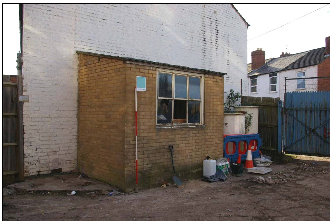
Figure 74: West elevation of Shed 4
