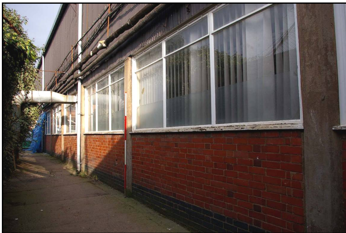
Figure 31: South elevation of Building T
