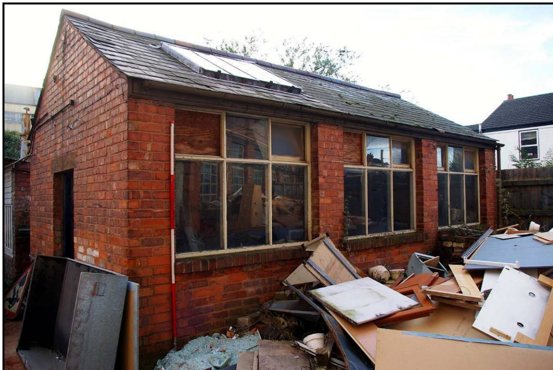
Figure 72: West elevation of Shed 3
