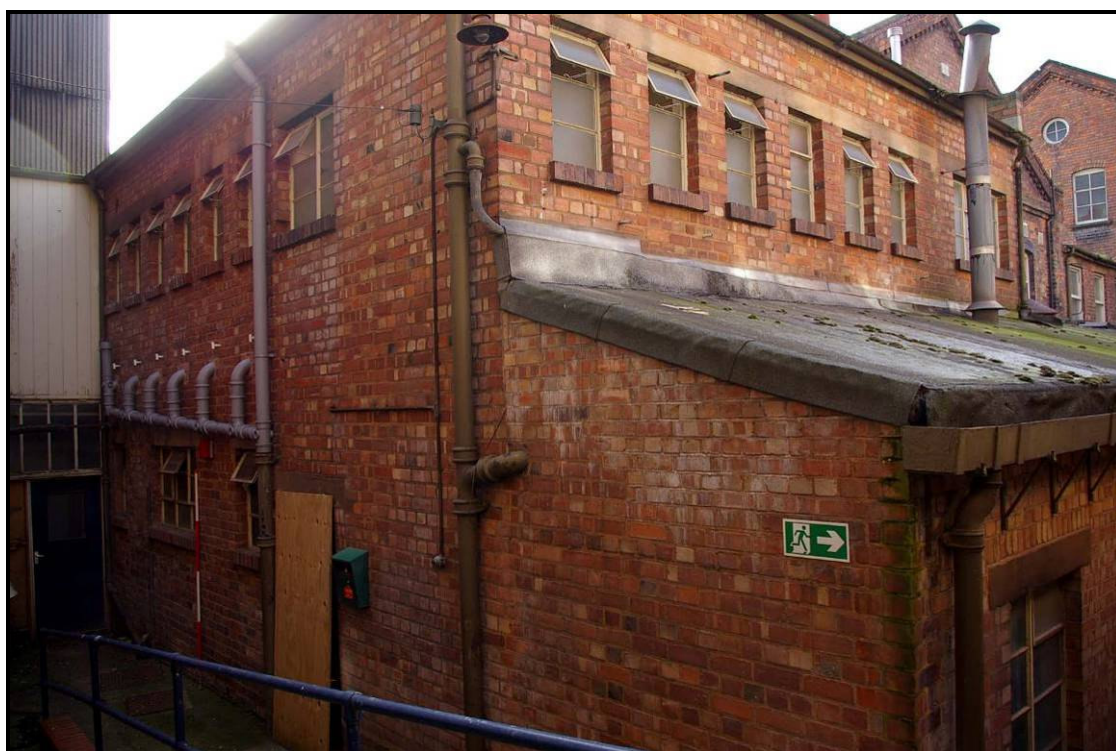
Figure 23: Building L1, looking south-east
