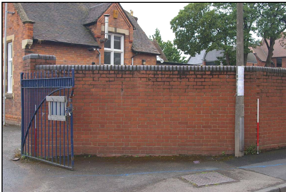
Figure 97: The northern gate to the Work's car park on King Street
