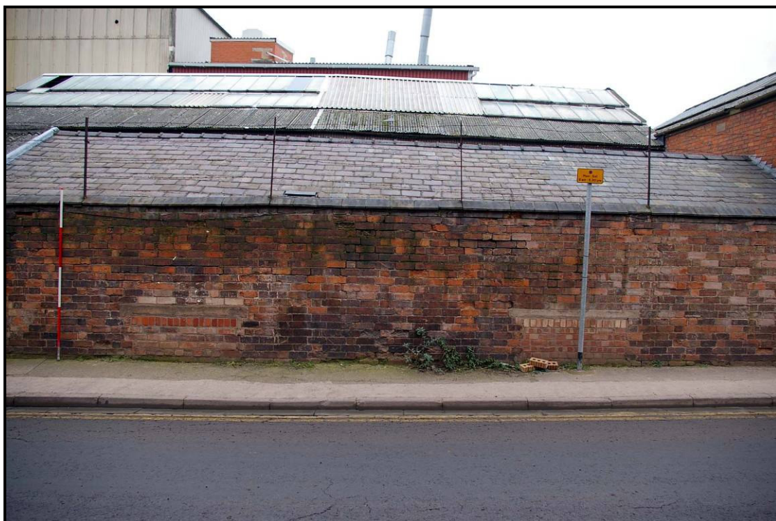
Figure 81: South wall of early phase of Building Z
