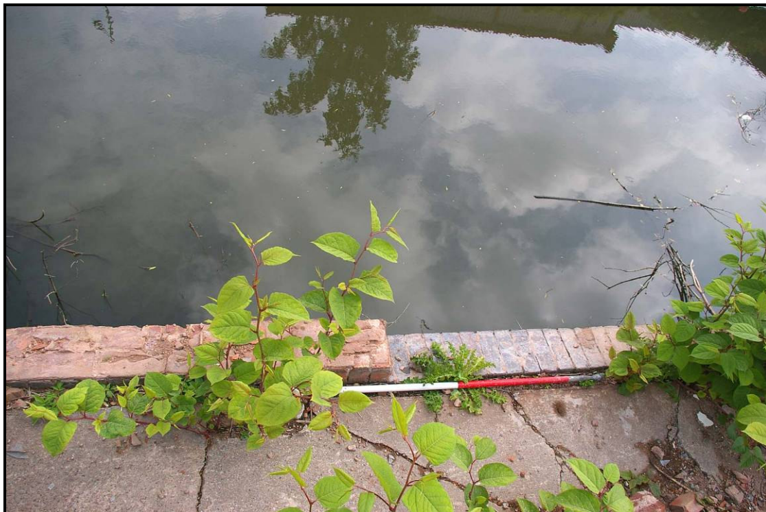
Figure 91: Japanese knotweed on the canal wall east of Building F
