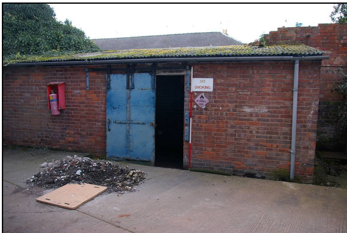
Figure 67: North elevation of Shed 1
