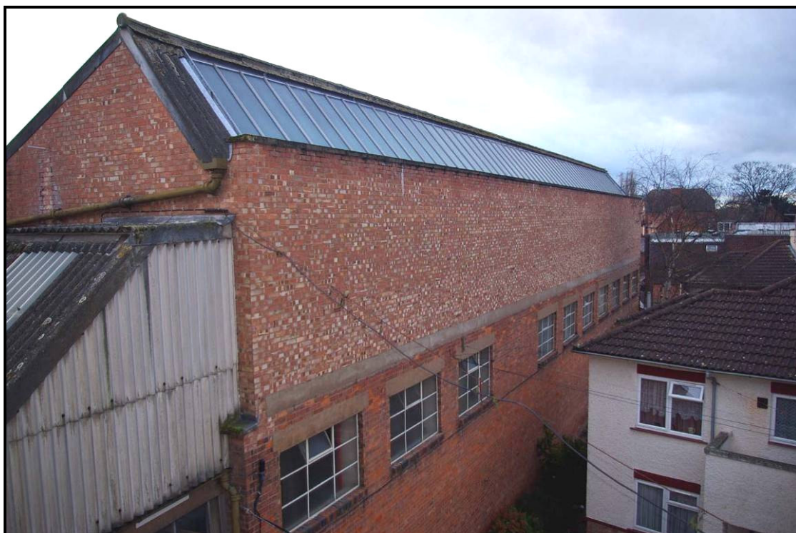
Figure 37: West elevation of Building U
