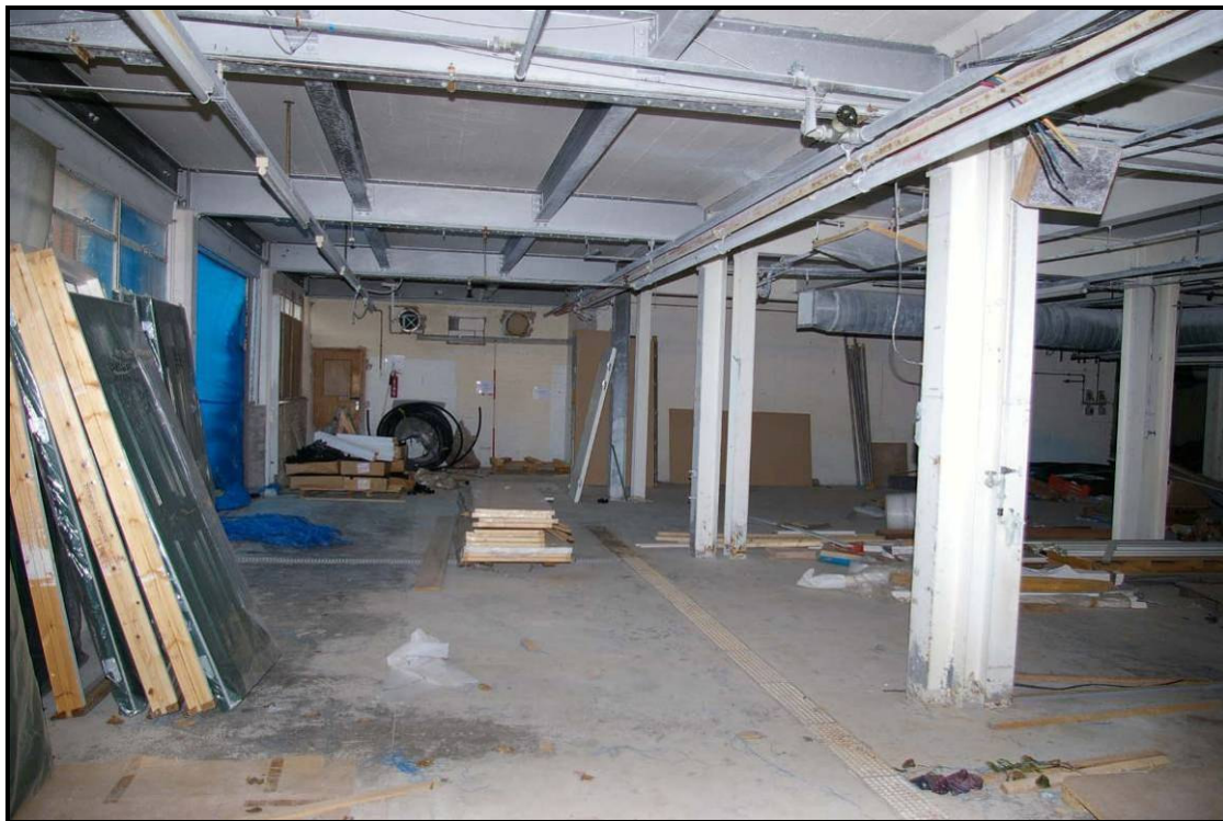
Figure 32: Ground floor of Building T, looking west
