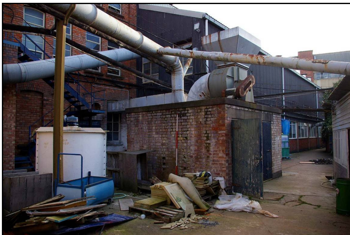
Figure 75: Shed 5, looking north-east
