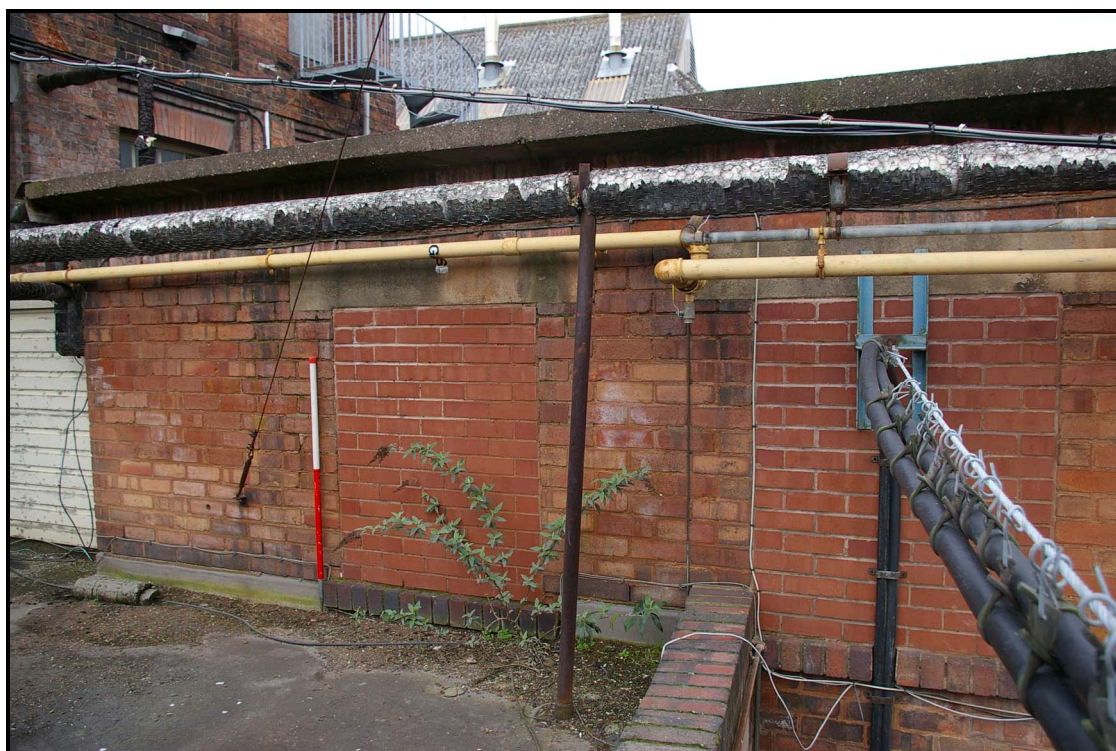
Figure 102: South elevation showing blocked windows
