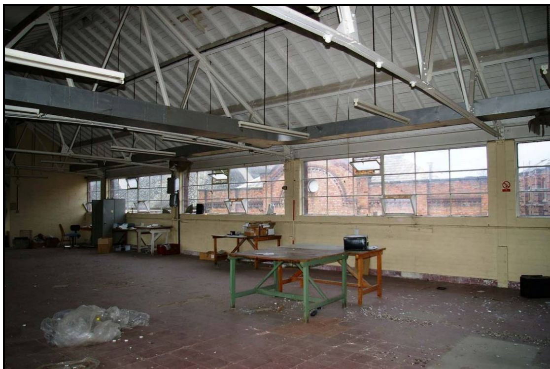
Figure 13: Second floor of Building F, looking south-west
