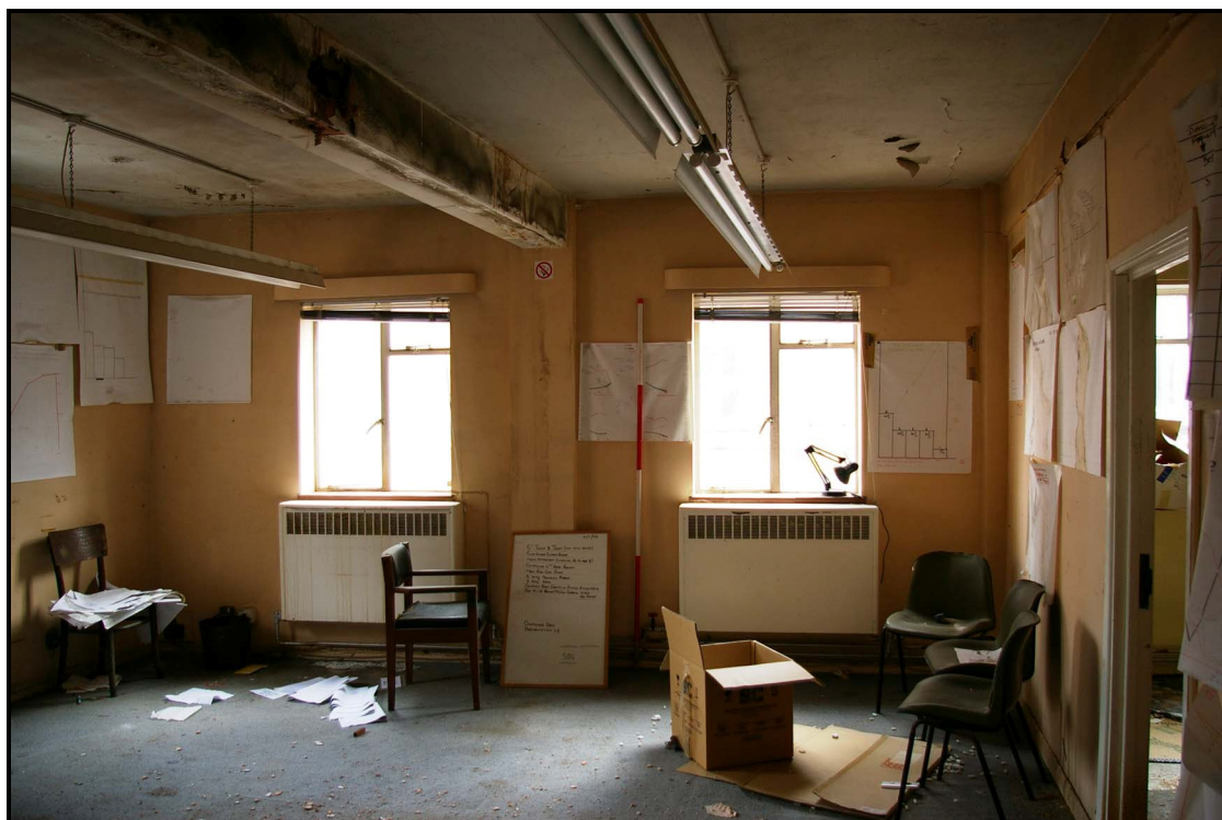
Figure 103: First floor of the maintenance block, looking east
