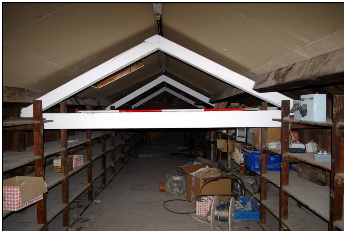
Figure 66: Mezzanine floor of Building Z with collar-beam trusses
