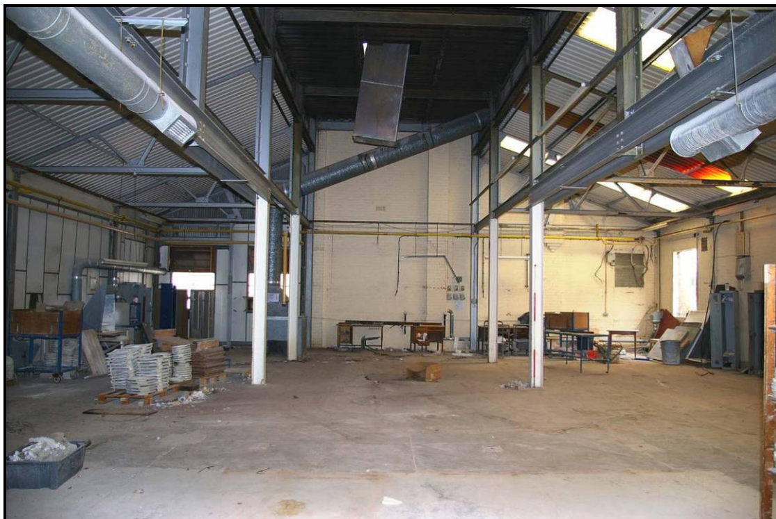
Figure 33: First floor of Building T, looking west
