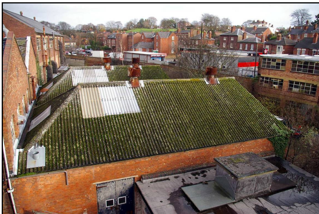
Figure 16: Building I, looking north
