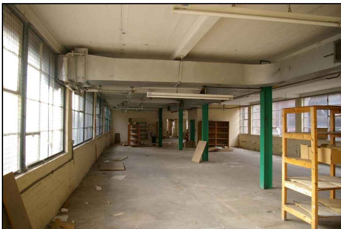
Figure 14: Ground floor of Building F, looking south
