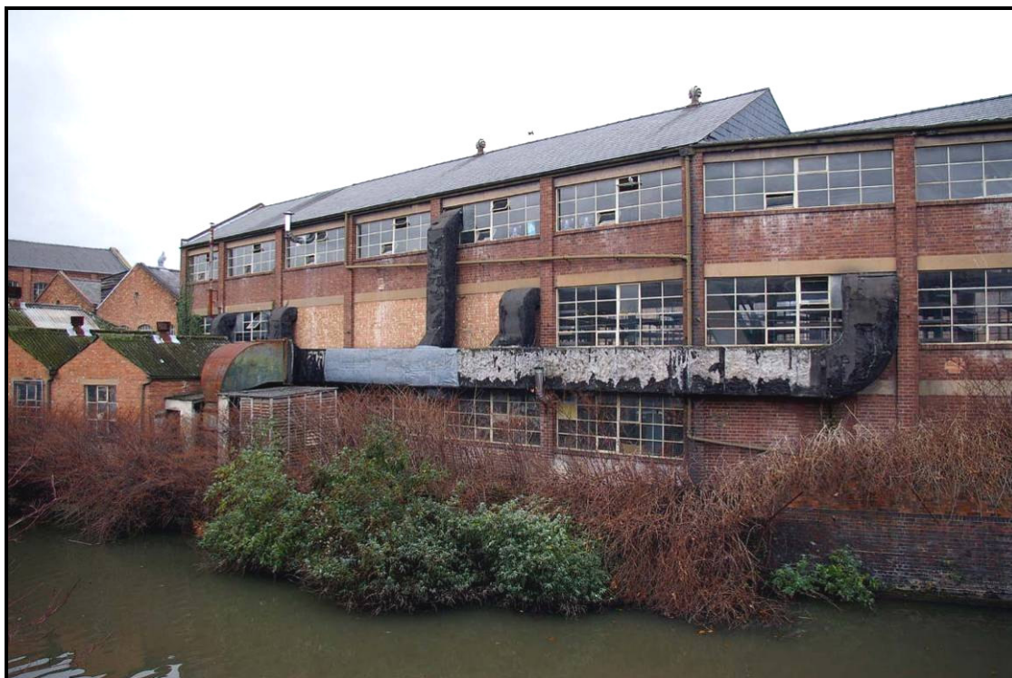
Figure 12: East elevation of Building F
