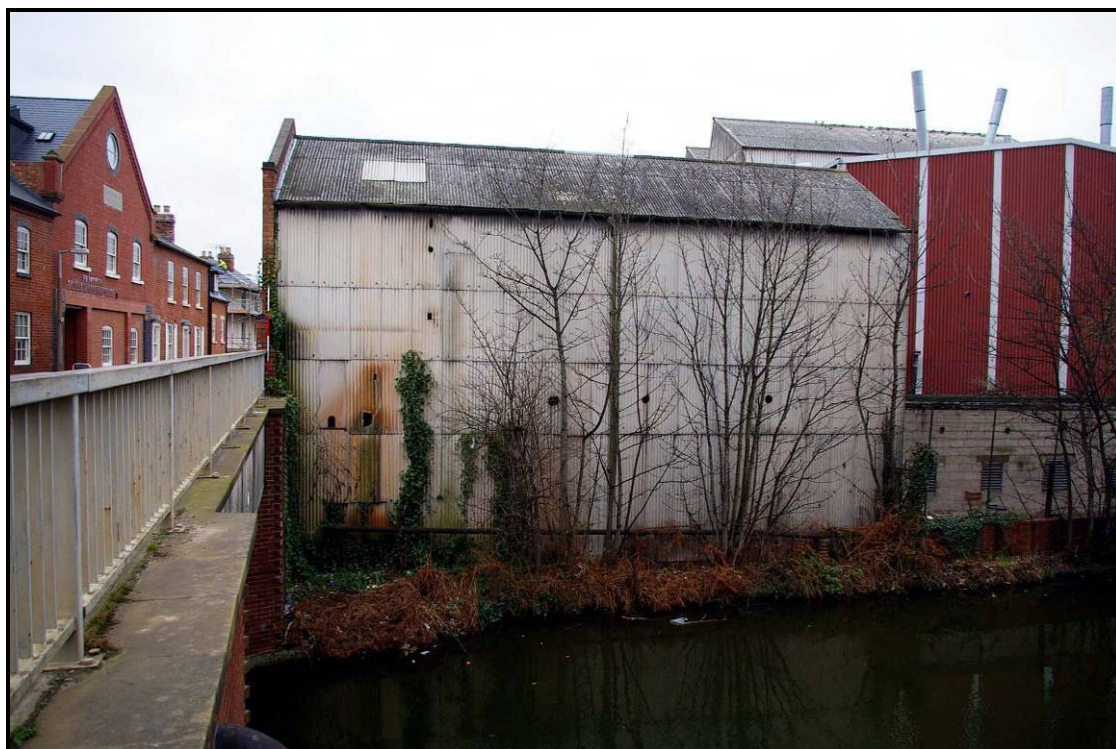
Figure 63: East elevation of the eastern block of Building Z
