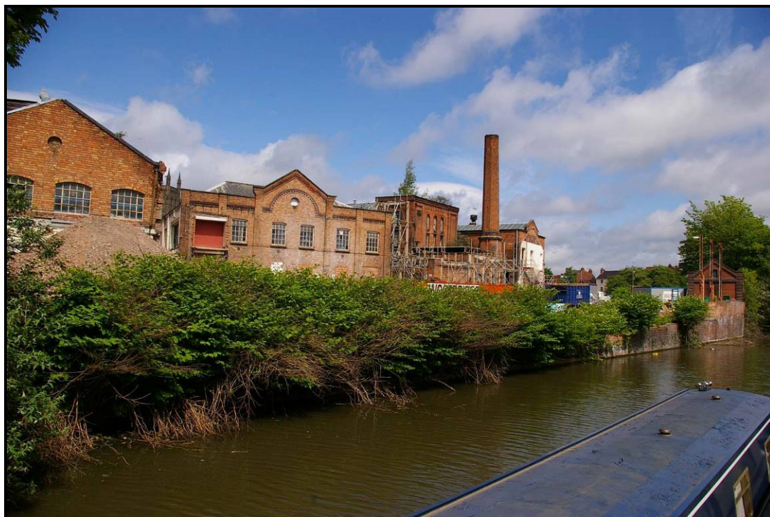
Figure 83: South end of the canal wall
