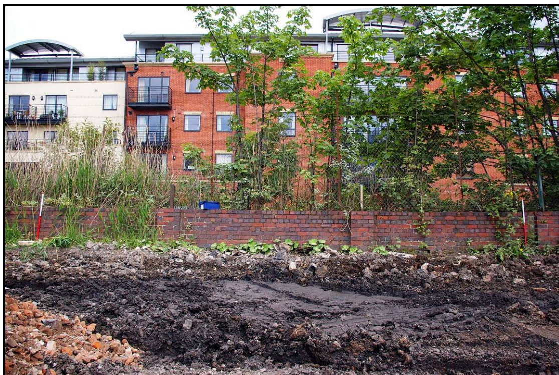
Figure 93: The canal wall on the east of Building W2
