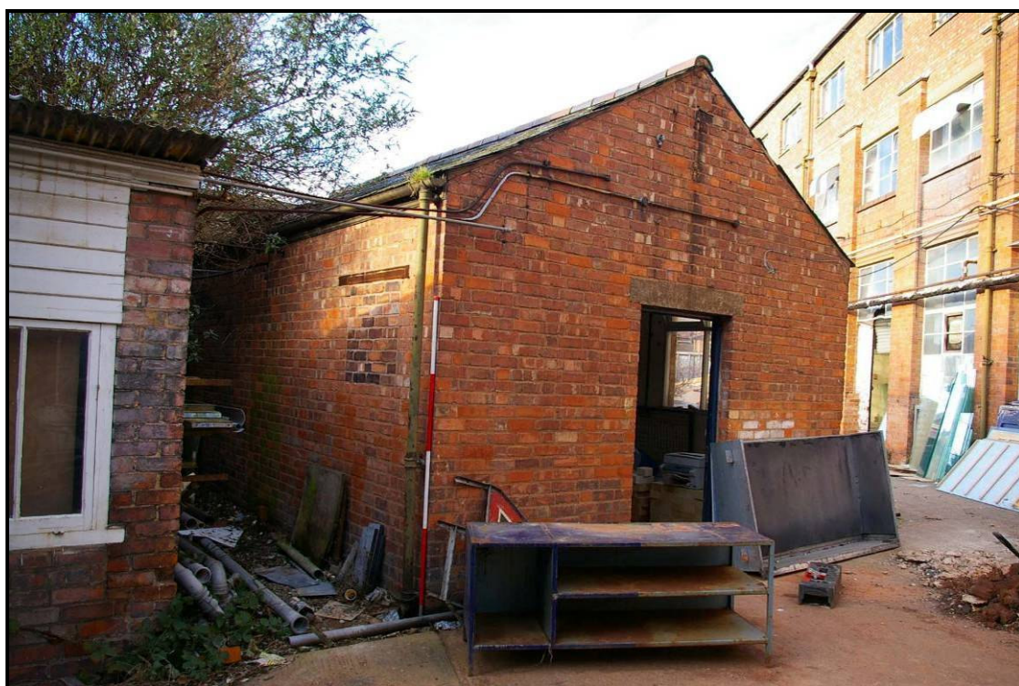
Figure 71: North elevation of Shed 3
