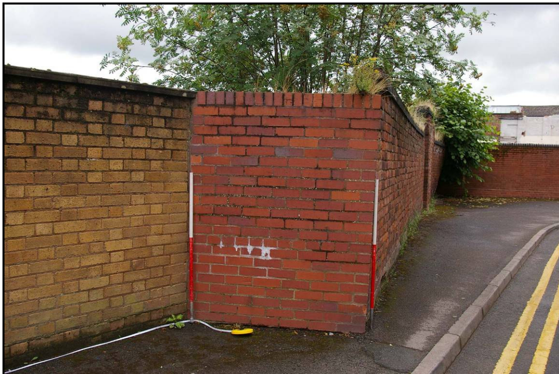
Figure 95: Car park boundary wall on St Peter's Street
