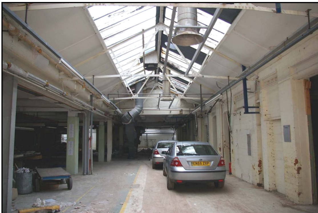
Figure 28: Inside Building O, looking west
