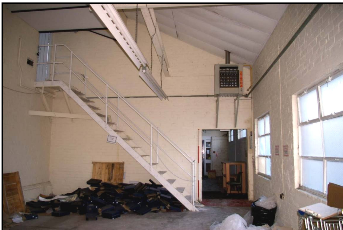
Figure 4: Inside Building A1, looking west
