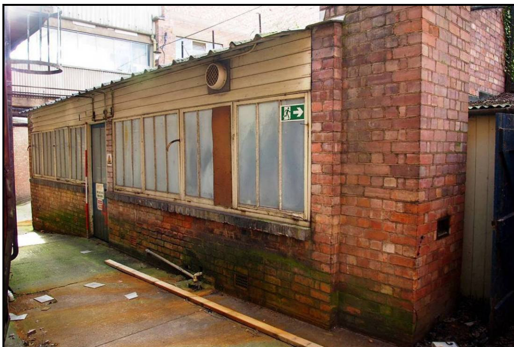
Figure 78: North elevation of Shed 6
