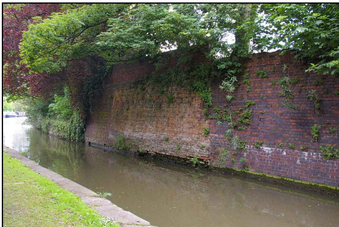
Figure 87: Northern end of the canal wall with repaired section
