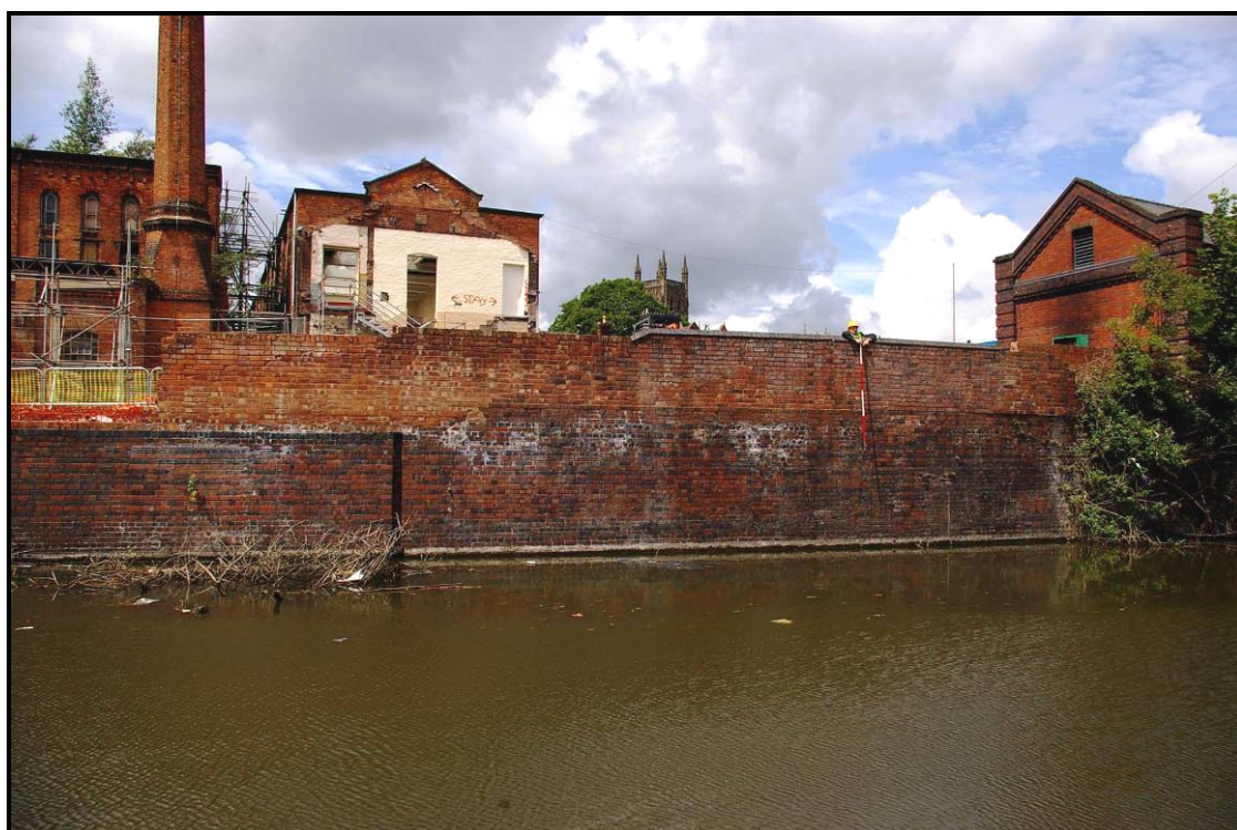
Figure 85: The canal wall between Buildings D (south) and C (north)
