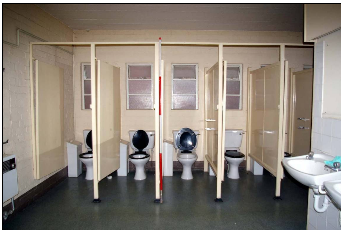
Figure 25: Toilets on the first floor of Building L1
