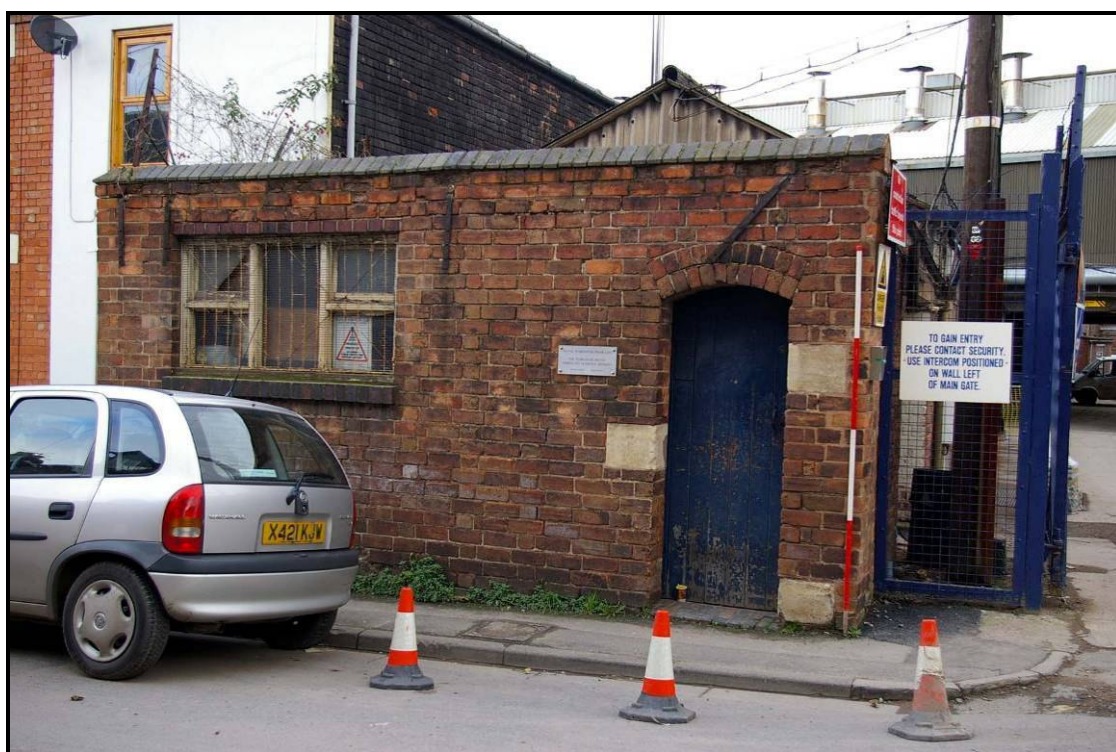
Figure 55: South elevation of Building X1
