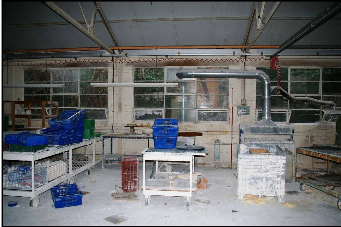
Figure 44: Inside Building V, looking west
