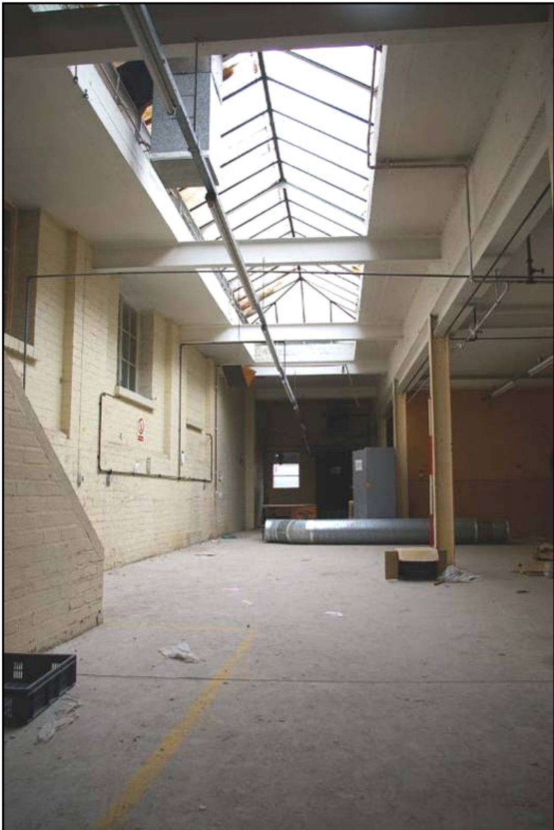
Figure 22: Ground floor of the northern block of Building L, looking east
