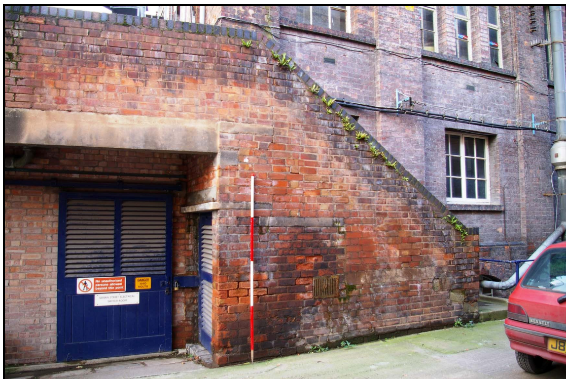
Figure 101: Staircase on the north elevation
