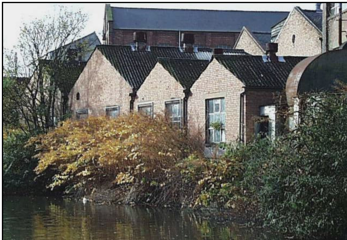
Figure 15: East elevation of Building I
