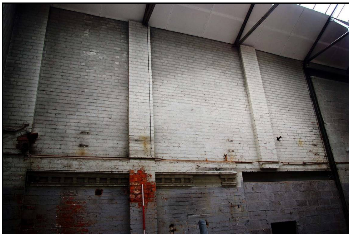
Figure 62: Ghost gable on the east elevation of the early phase of Building Z
