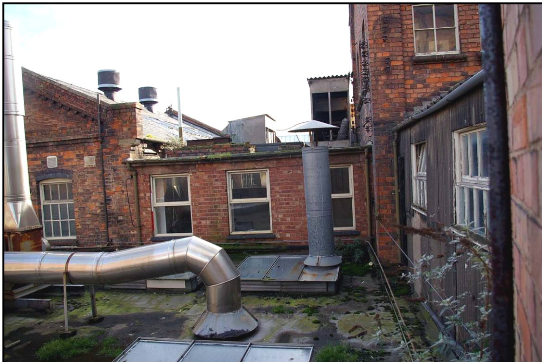
Figure 27: West elevation of Building O
