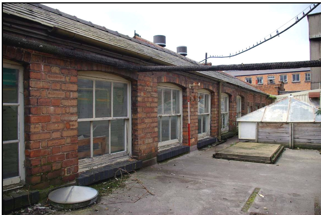
Figure 19: North elevation of the southern block of Building L
