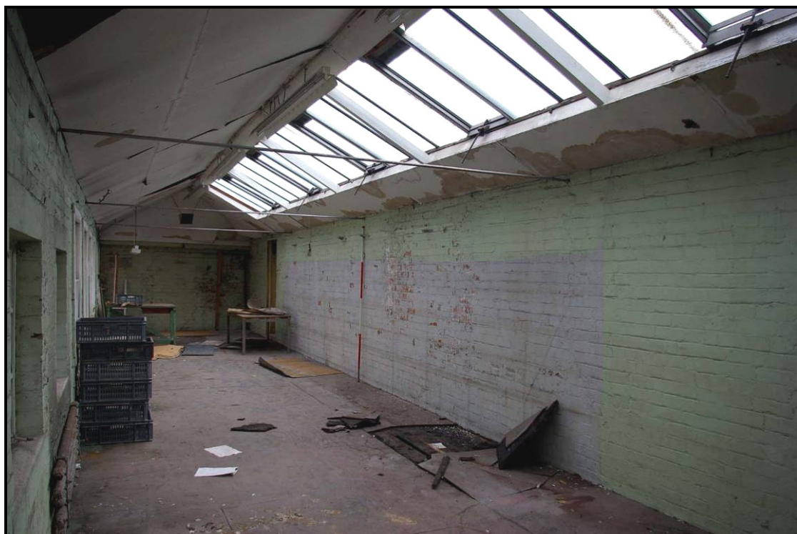
Figure 20: First floor of the southern block of Building L, looking east
