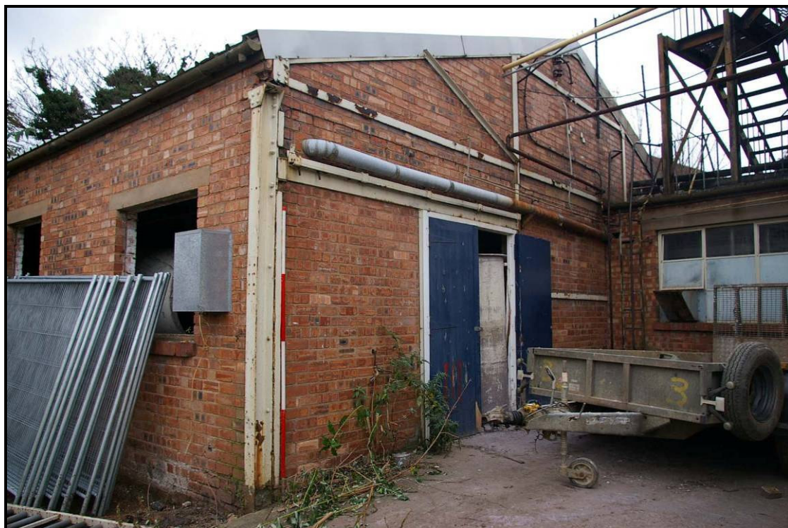
Figure 41: North elevation of Building V
