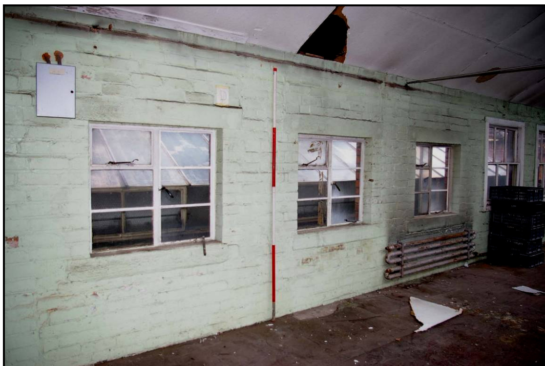
Figure 21: First floor of the southern block of Building L, looking north-east
