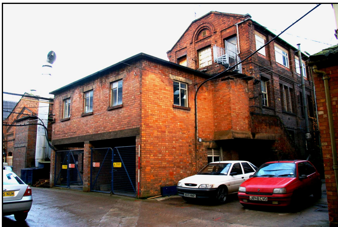
Figure 100: The maintenance block, looking south-west
