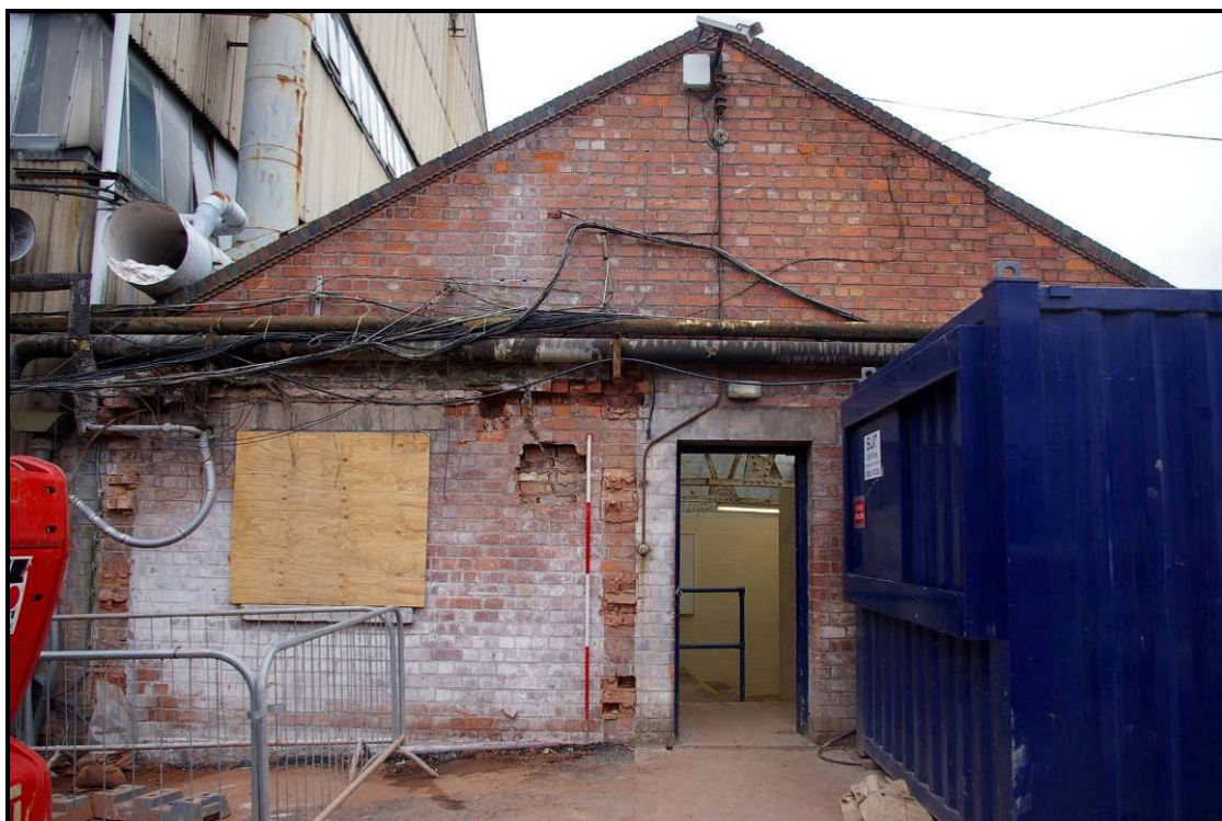
Figure 59: West elevation of the northern block of Building Y
