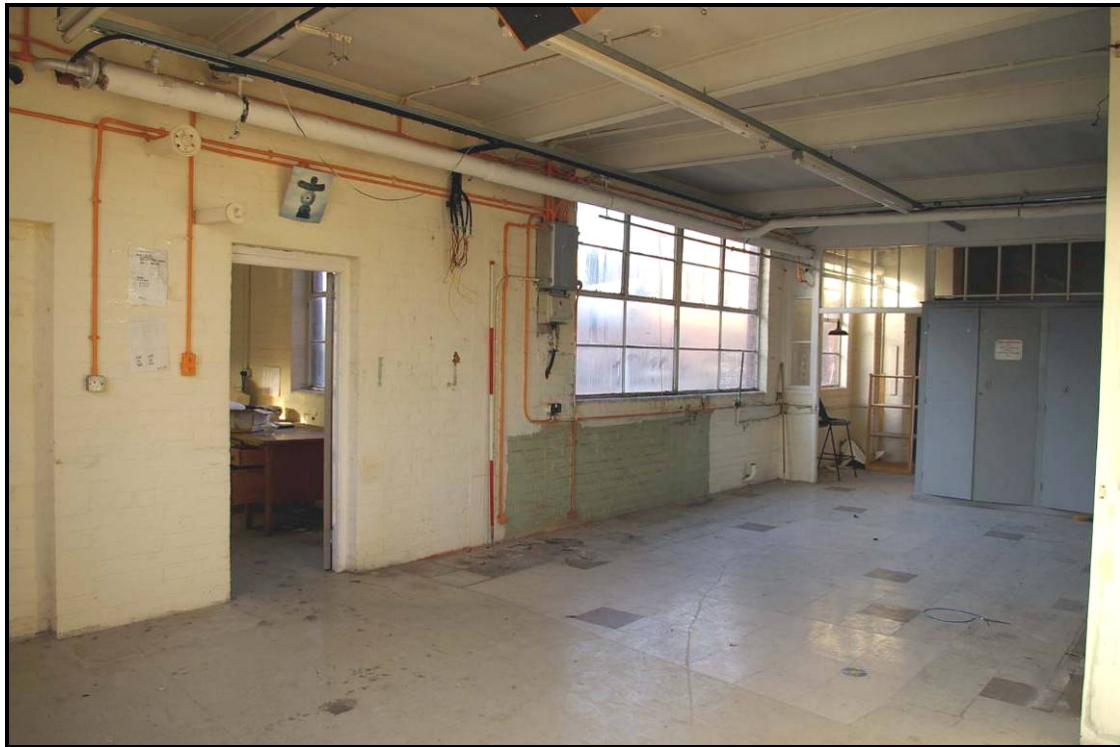
Figure 9: First floor of Building C1, looking west towards Building B
