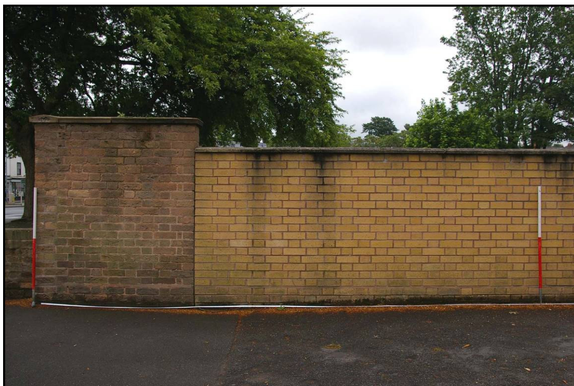
Figure 94: North end of boundary wall on St Peter's Street
