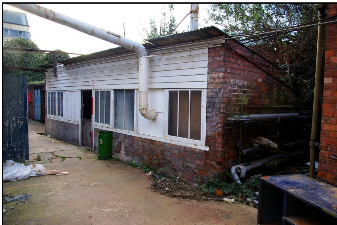
Figure 69: North elevation of Shed 2
