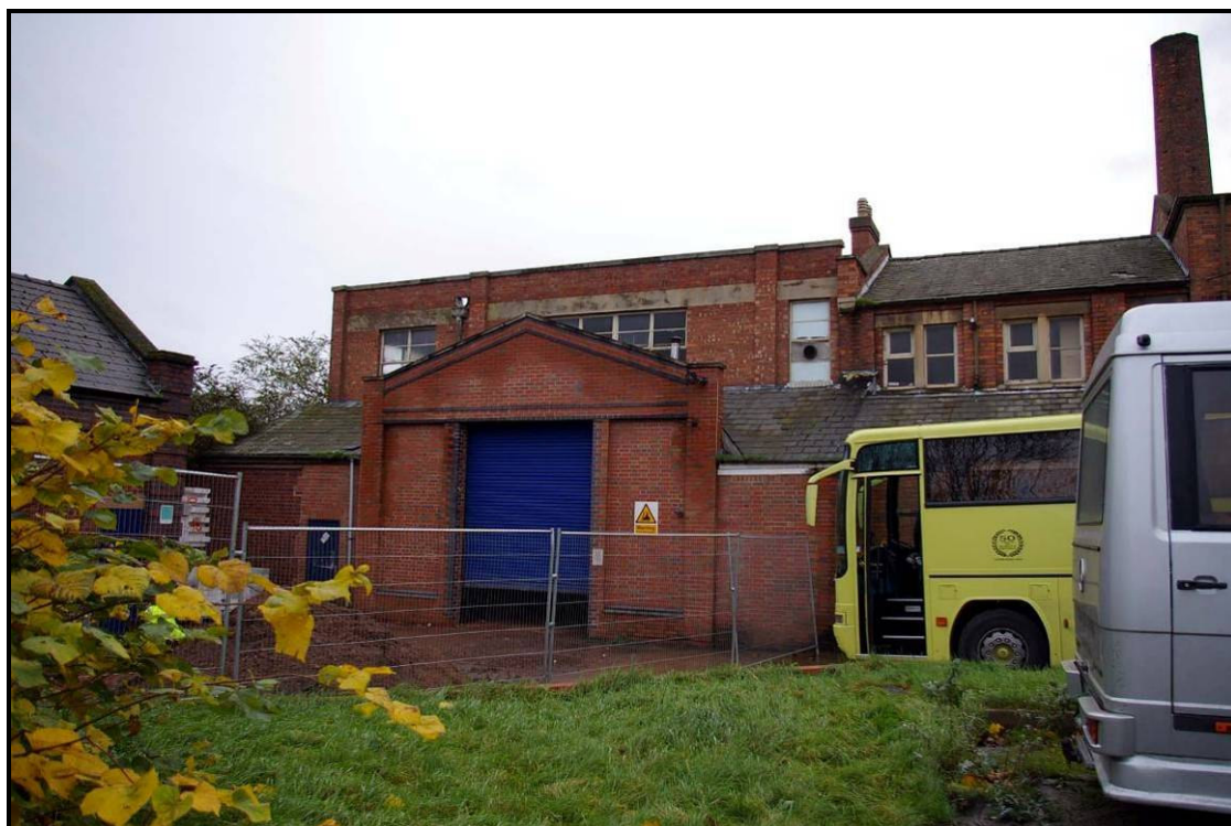
Figure 6: The north-east gate of Building A2
