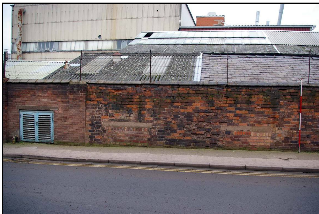
Figure 80: South wall of Building Y (left) and early phase of Building Z (right)
