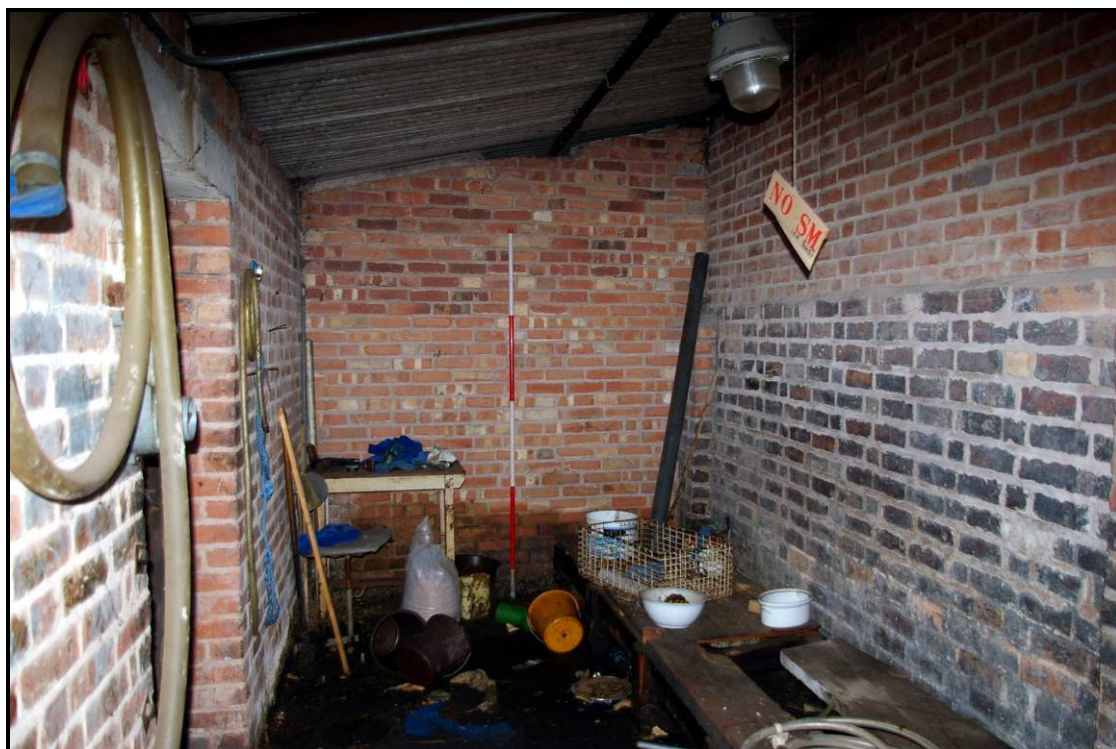
Figure 68: Inside Shed 1, looking east
