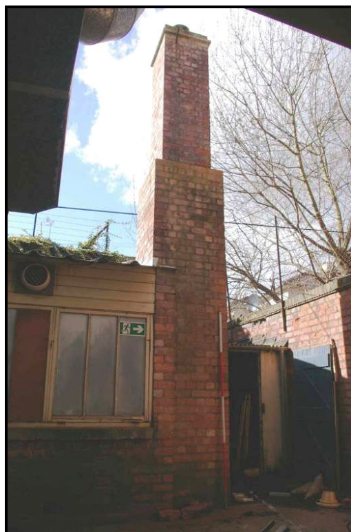
Figure 77: Chimney of Shed 6, looking south
