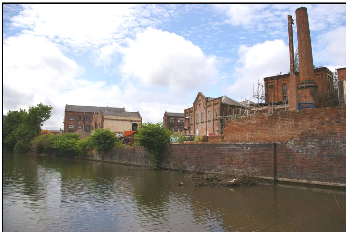
Figure 84: General view of the canal wall, looking south
