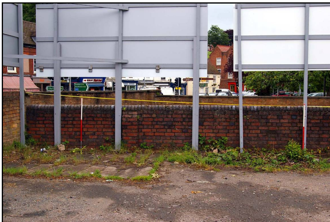
Figure 90: North end of the canal wall viewed from the car park
