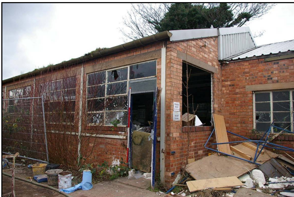
Figure 42: East elevation of Building V
