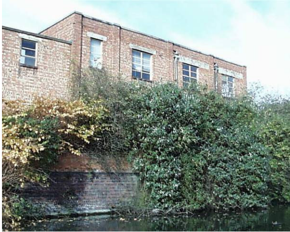
Figure 67: The east elevation of Building C1 from the canal. The link to Building F lies to the left.
