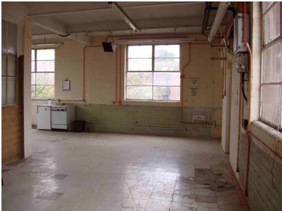
Figure 71: Building C1 looking towards the windows overlooking the canal. Upper floor interior looking towards Building B.
