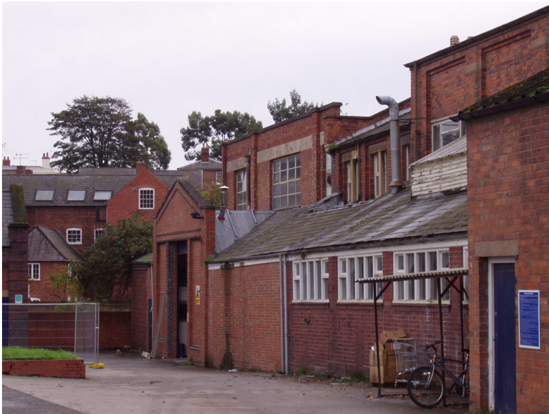
Figure 3: Buildings A1 through to C1 viewed from the north-west
