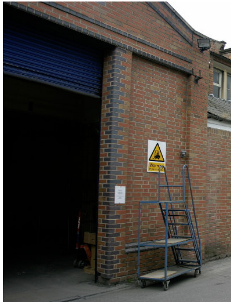
Figure 42: Access to Building C1 through A2 added in 1990
