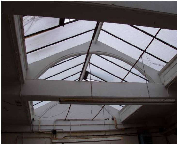
Figure 29: The skylight designed by Thomas Sutton around 1900
