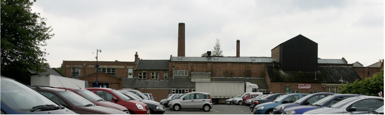
Figure 1: View from the north showing from left to right: buildings C1, B, A2, A1 with A behind
