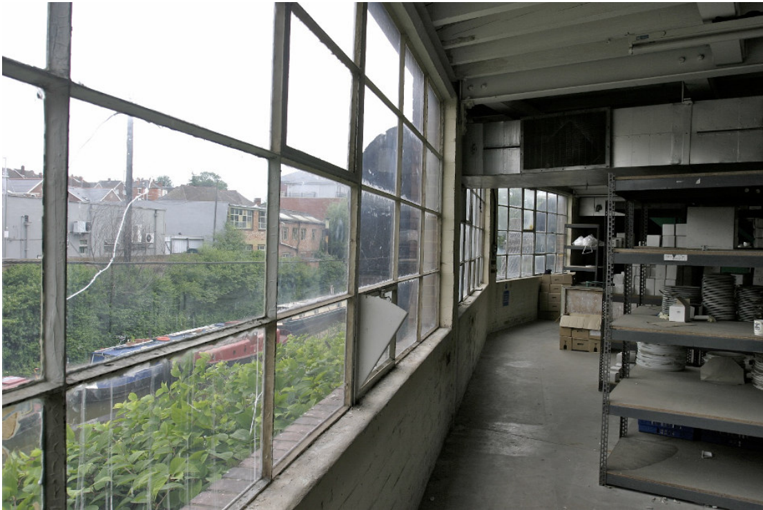
Figure 76: Building F (second floor) looking south-east
