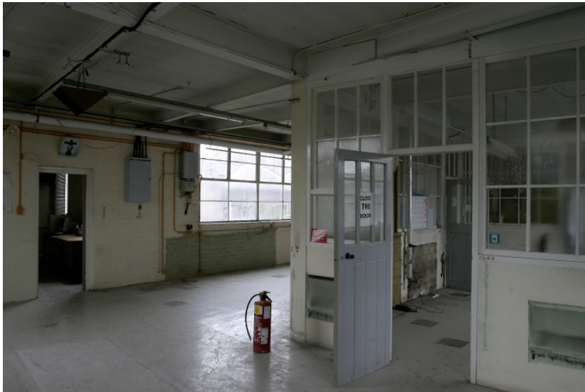
Figure 68: First floor interior looking toward the south window. Building B lies off to the right with the spur towards Building F on the left.
