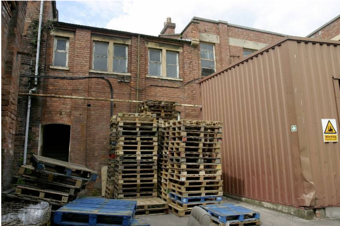
Figure 65: Building B with C1 to the right. Building A is to the left.
