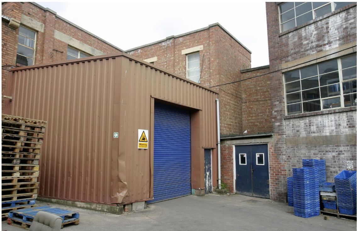
Figure 66: The steel sheeting lies on Prince's Drive and hides the bunkers shown in Figure 61
