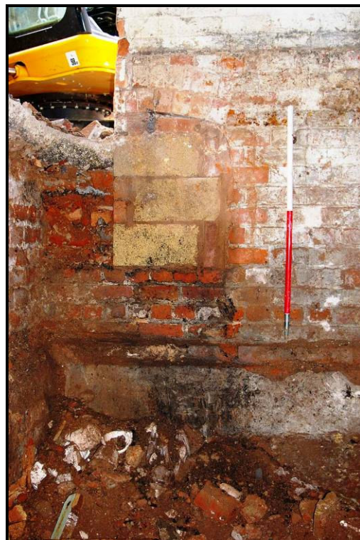
Figure 21: Former blocked-up window
