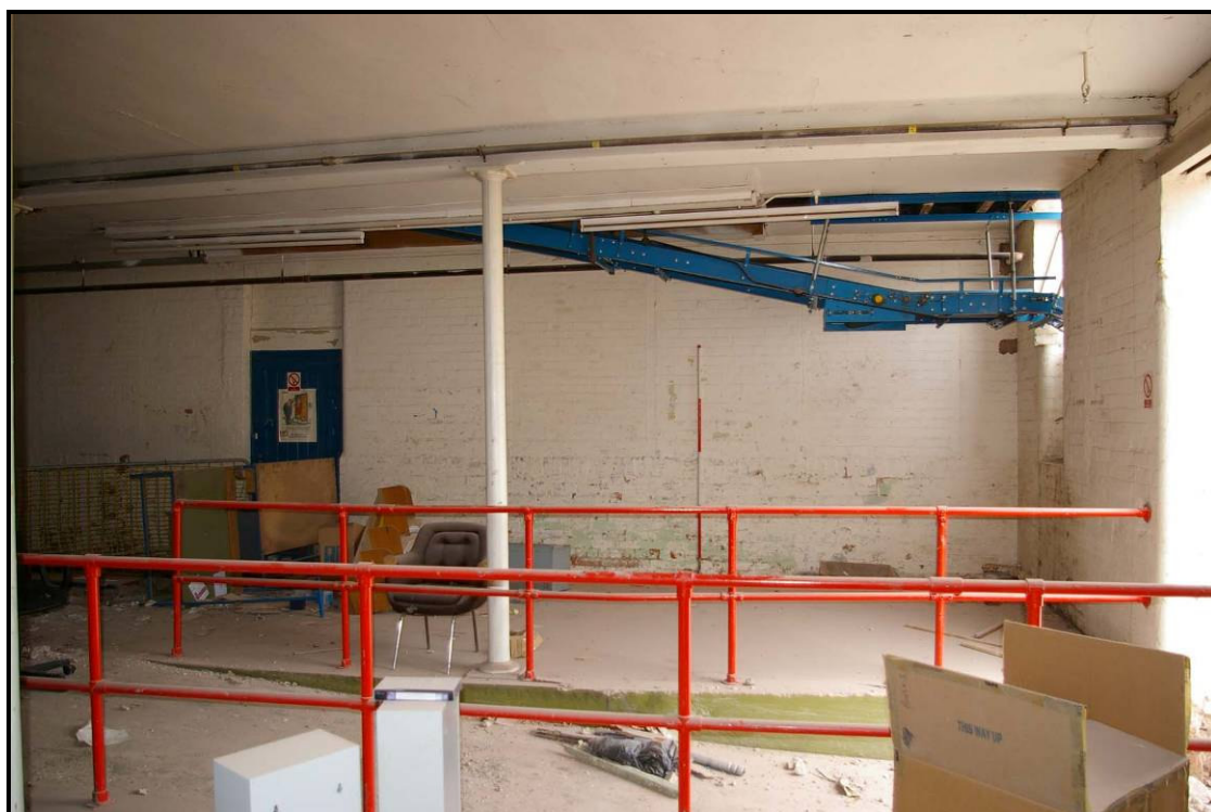
Figure 24: Ground floor, looking east
