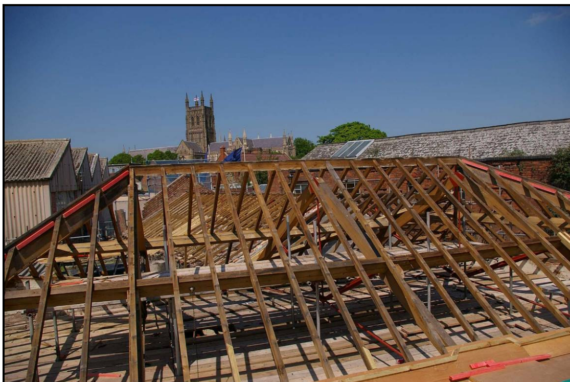
Figure 34: Hipped roof structure, looking west
