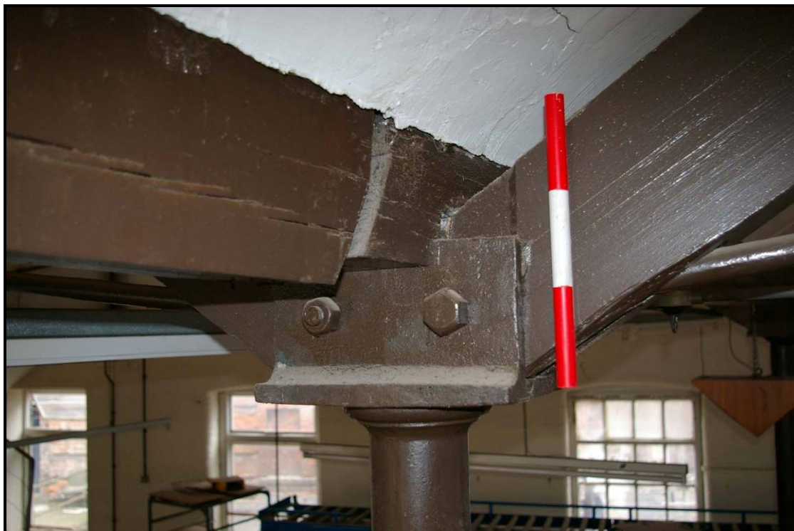
Figure 33: Detail of cast-iron column supporting a principal rafter
