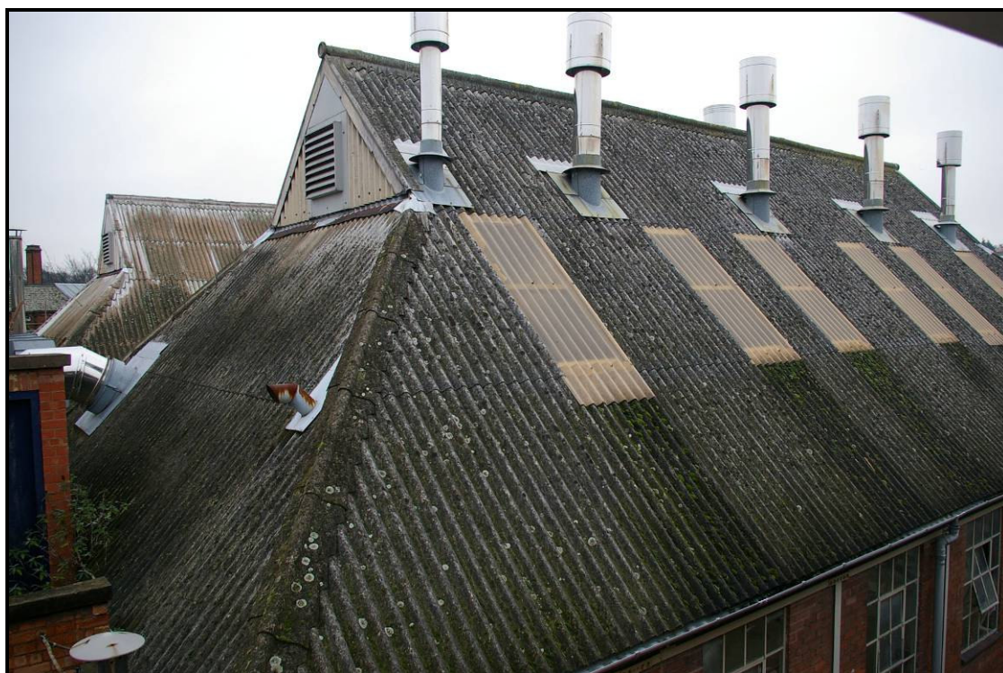
Figure 45: Detail of double-gabled roof on the west elevation
