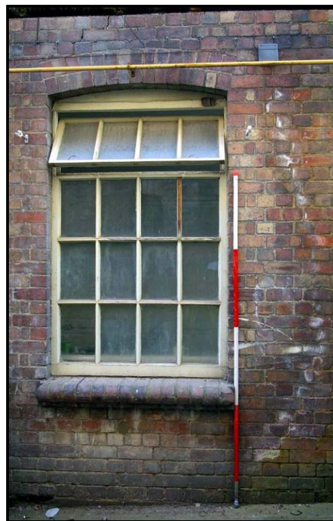
Figure 8: Detail of window
