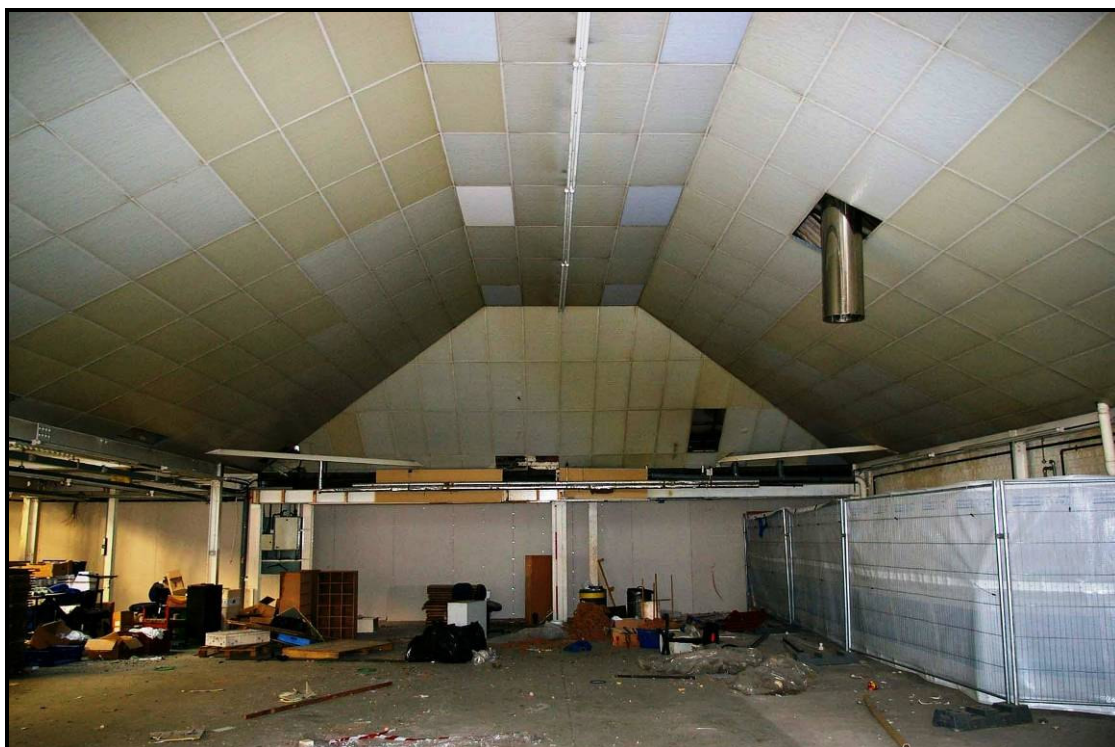
Figure 50: Suspended ceiling on the northern block, looking west
