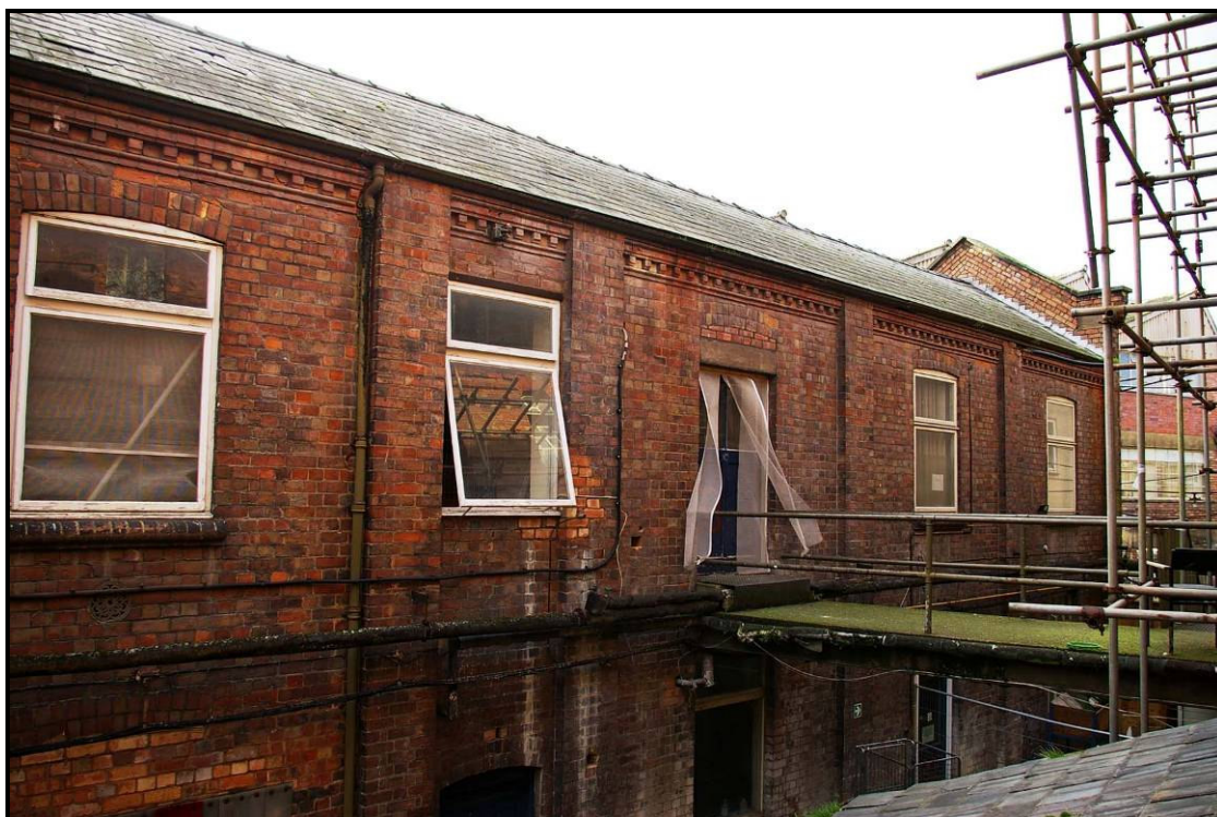
Figure 11: Western side of the north elevation
