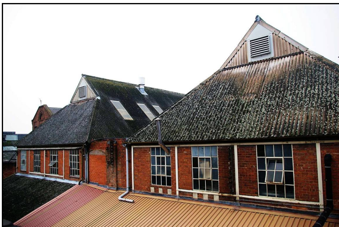
Figure 41: First floor windows on the east elevation
