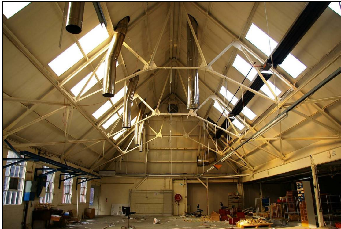
Figure 49: Roof structure on the southern block, looking west
