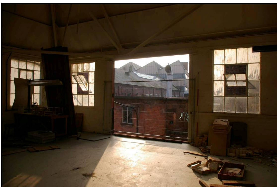
Figure 48: First floor of the southern block, looking towards Building W1
