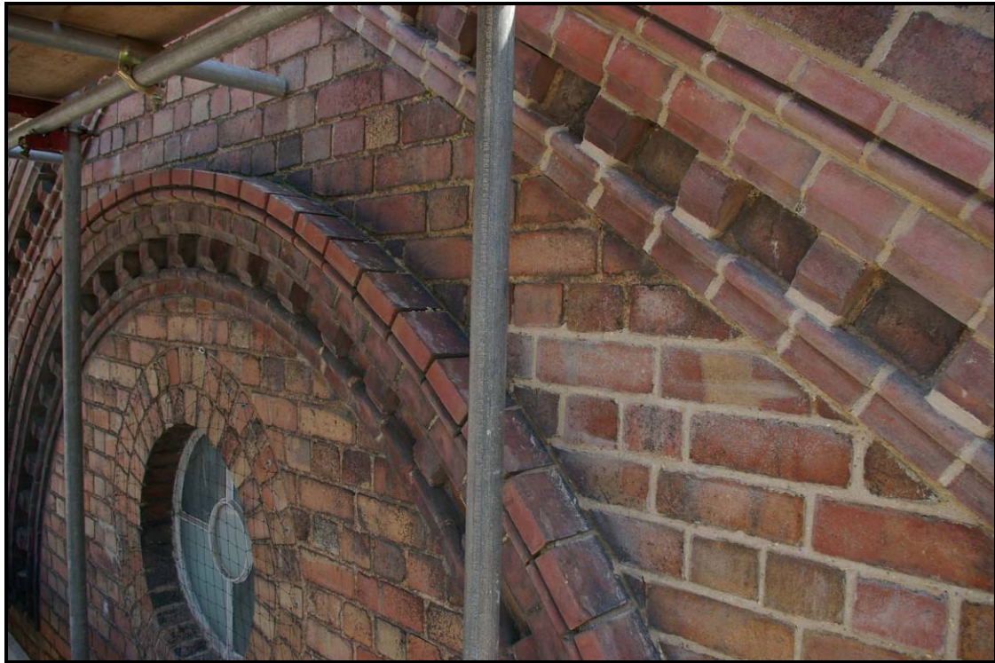
Figure 17: Detail of lunette brickwork of the west elevation
