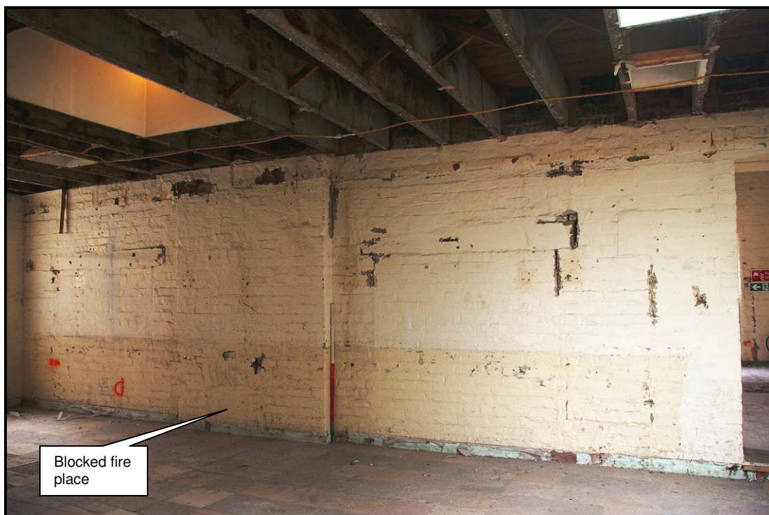
Figure 37: South elevation of partition wall
