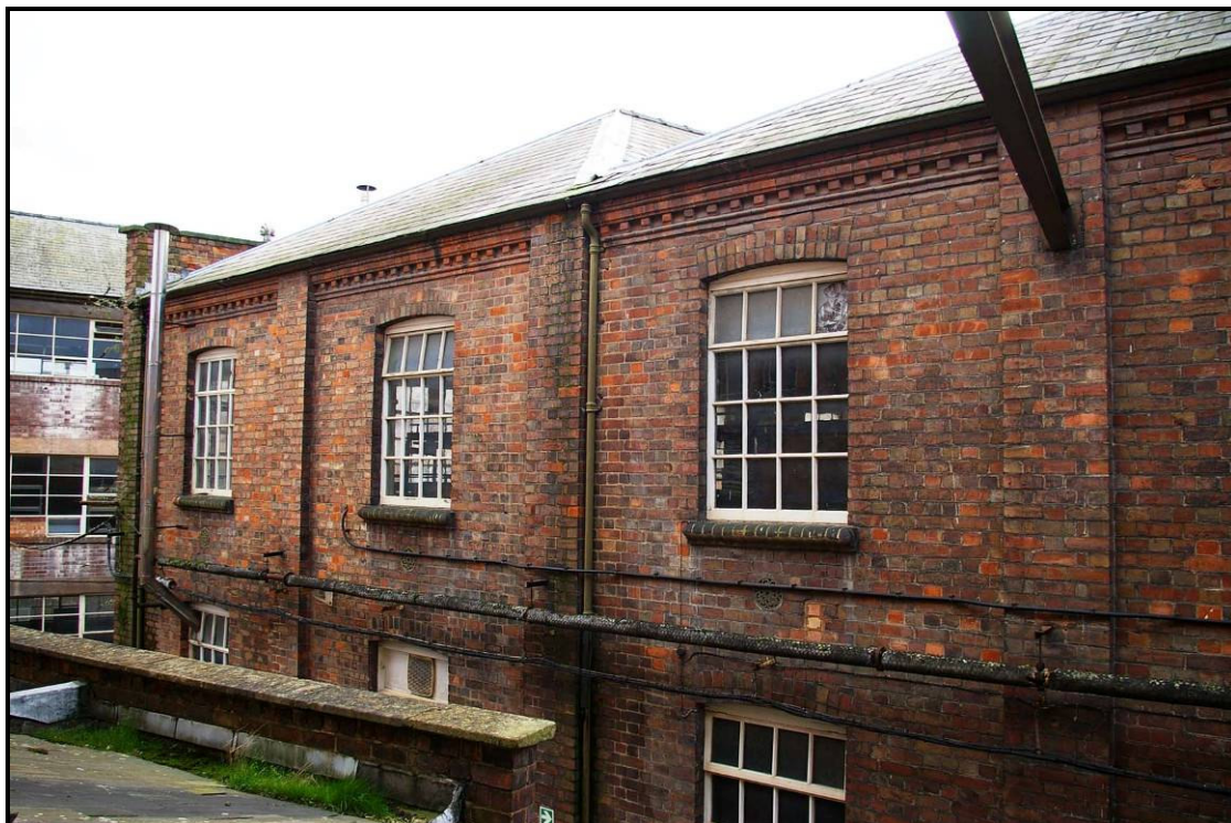
Figure 10: Eastern side of the north elevation
