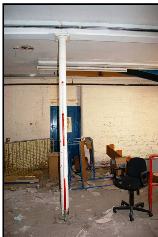
Figure 26: Cast-iron column
