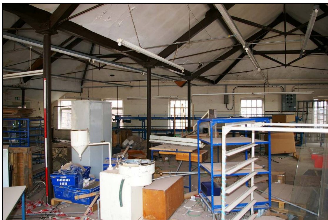
Figure 31: First floor, looking north
