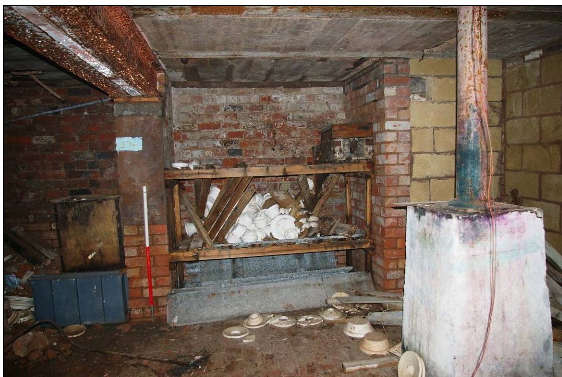
Figure 19: Inside the cellar, looking north
