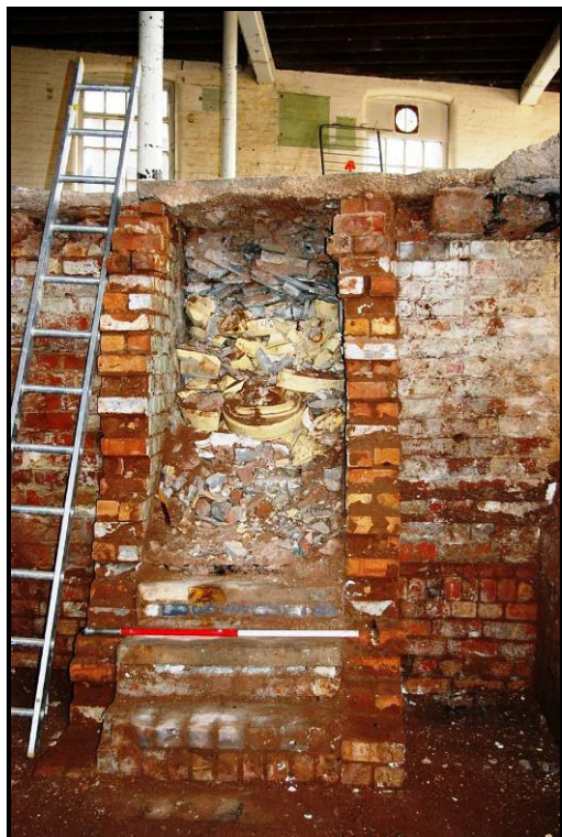
Figure 20: Staircase backfill
