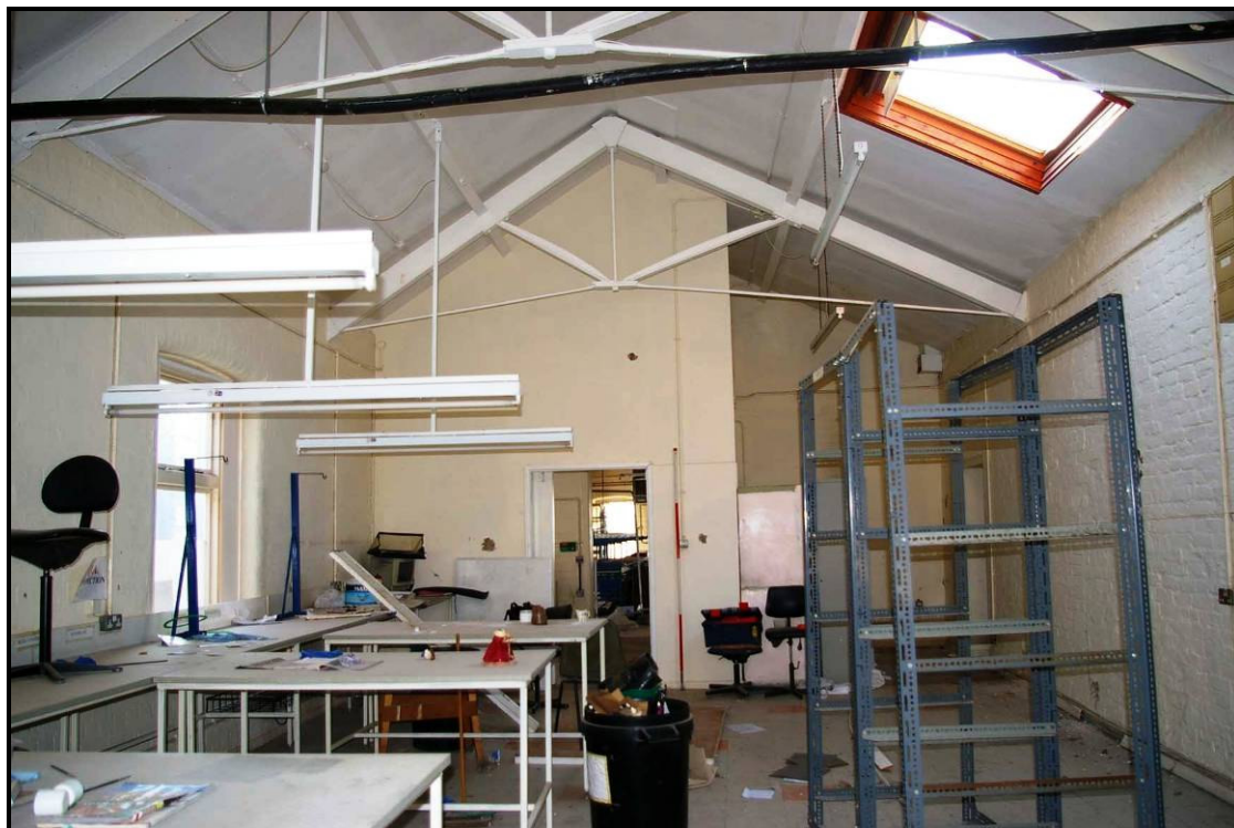
Figure 36: North-west room of the first floor
