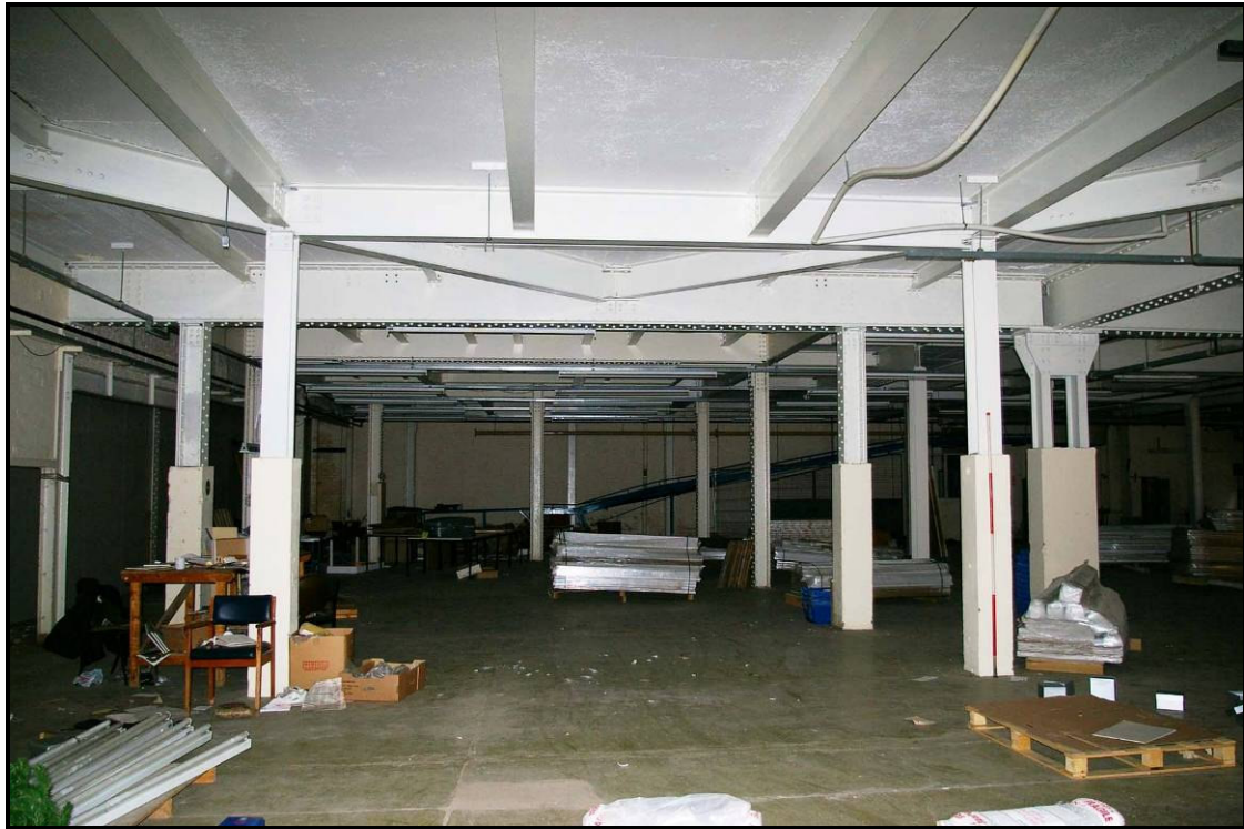
Figure 46: Ground floor, looking north
