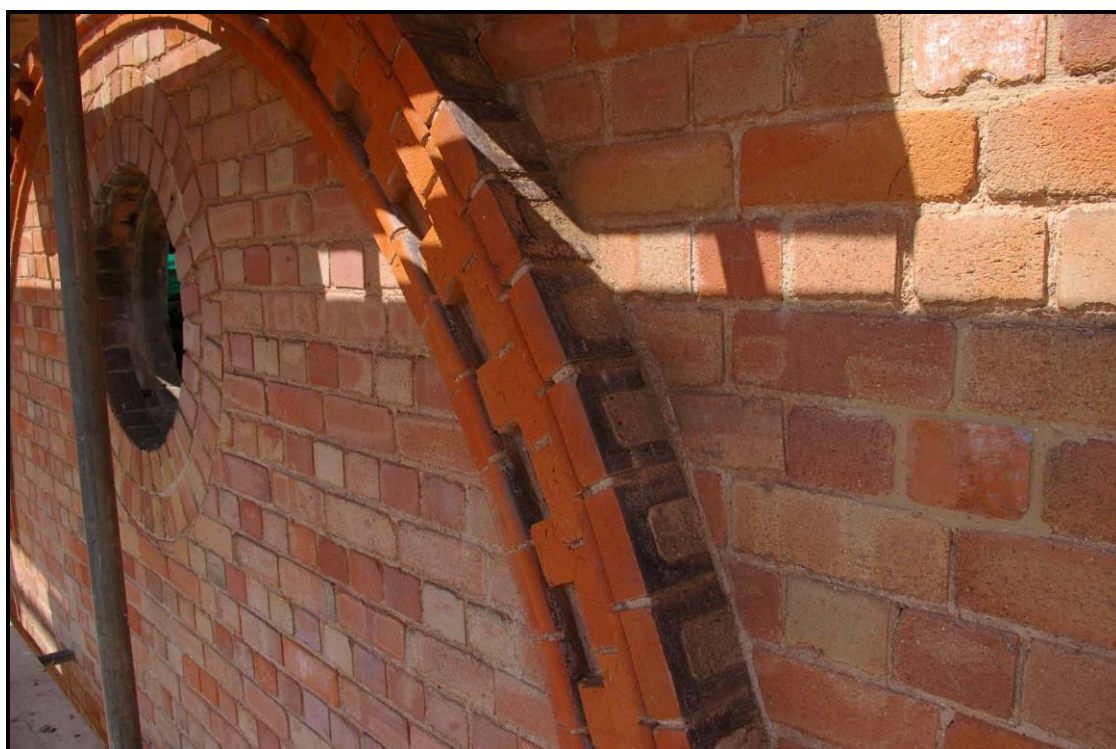
Figure 5: Detail of lunette showing frog bricks on the uppermost string course
