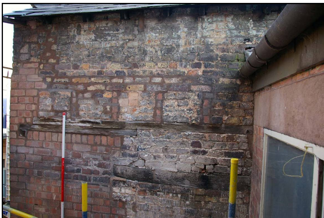
Figure 14: The westernmost end wall of the south elevation
