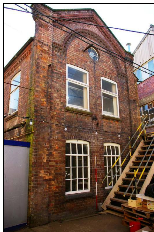
Figure 16: West elevation, from the ground
