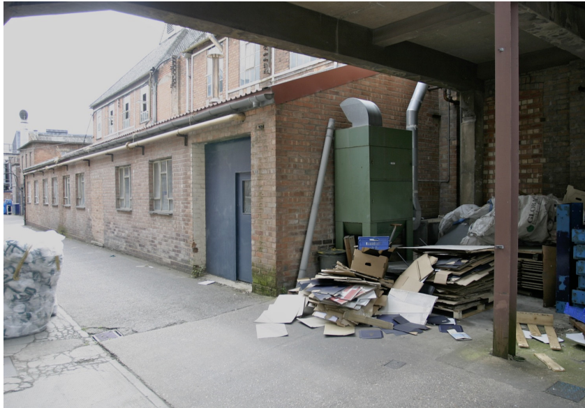
Figure 21: The post-1964 single-storey run in front of Building G from the north-east
