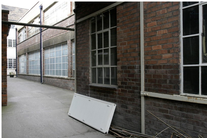
Figure 20: Detail of steel framing on Building G
