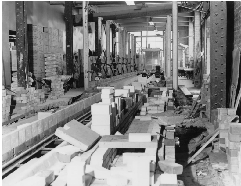
Figure 40: Construction of the Reidhammer tunnel kiln in G c1947 – 1950
