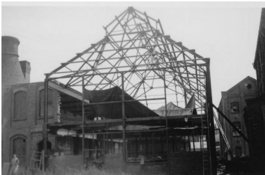
Figure 34: Building G. Building the south-westerly kiln c1935
