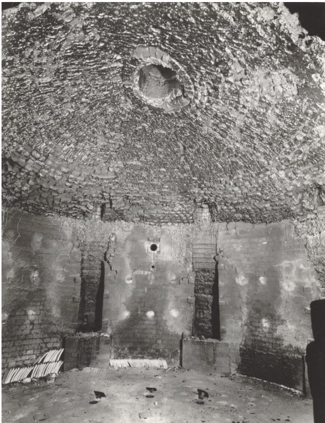
Figure 27: Inside a kiln at Royal Worcester showing the firing holes (source: Worcester Porcelain Museum)
