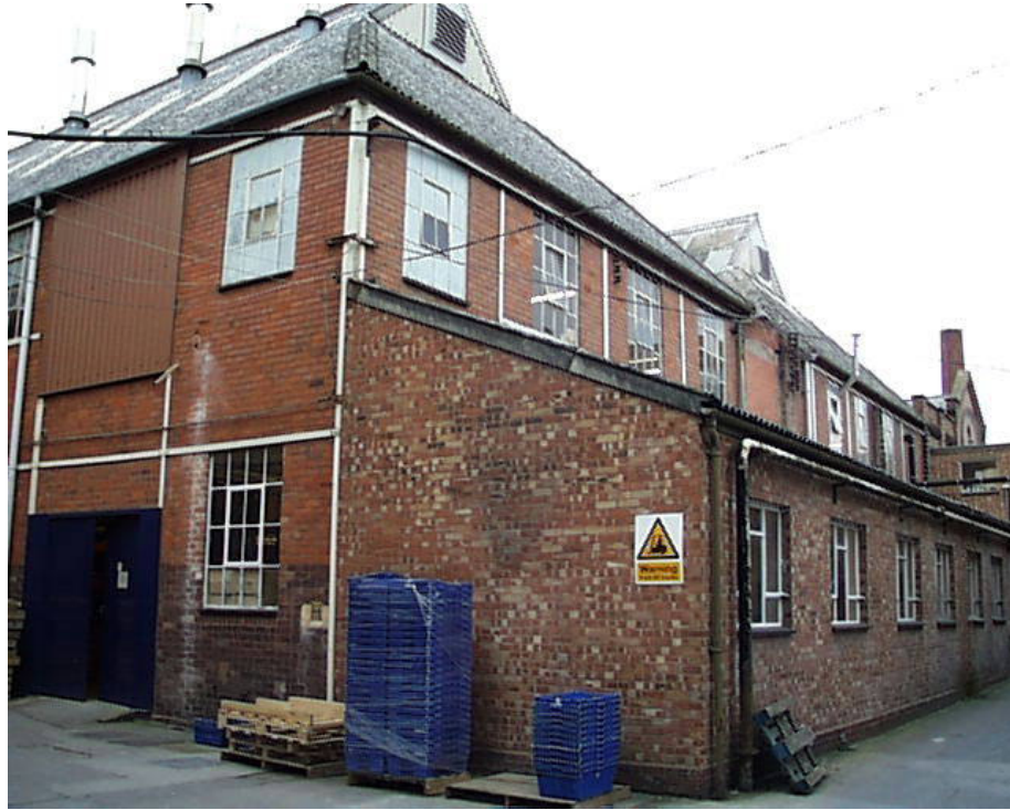
Figure 19: Building G from the south-east. The lean-to was built after 1964
