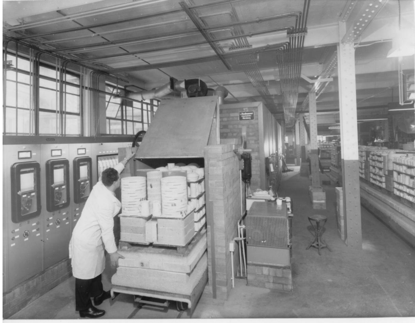
Figure 41: Pushing a loaded kiln truck into the new kiln. This would cause another truck to emerge from the far end of the kiln (source: Worcester Porcelain Museum).
