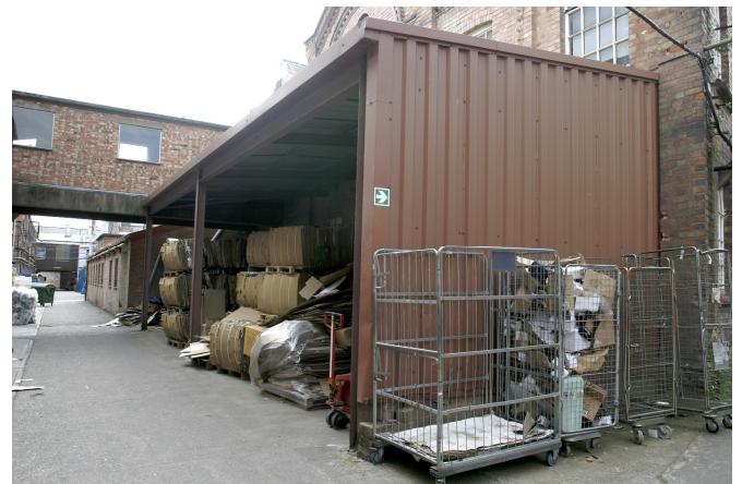
Figure 49: Shed in front of Building E from the north-east. The new bridge is between Buildings F and E
