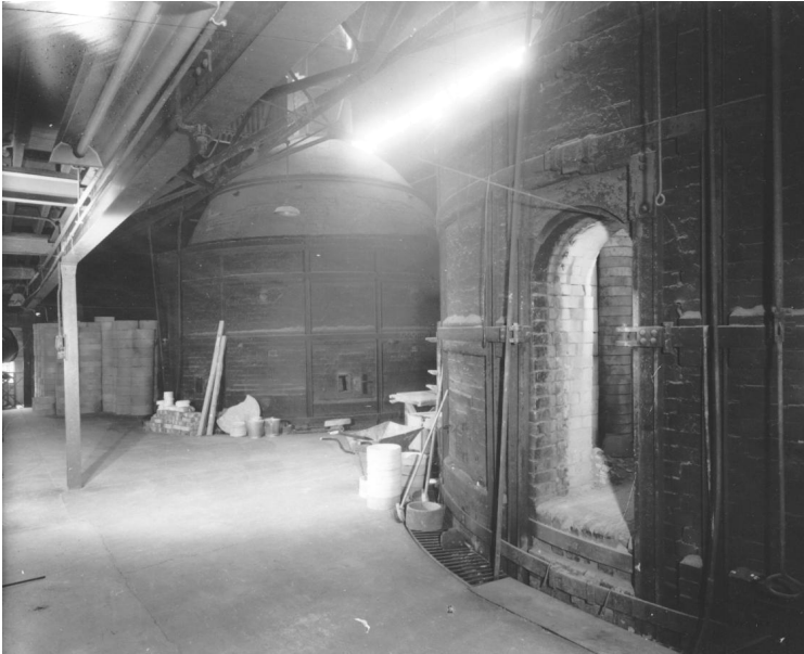
Figure 26: The gap between the kiln and hovel at Building G (source: Worcester Porcelain Museum)
