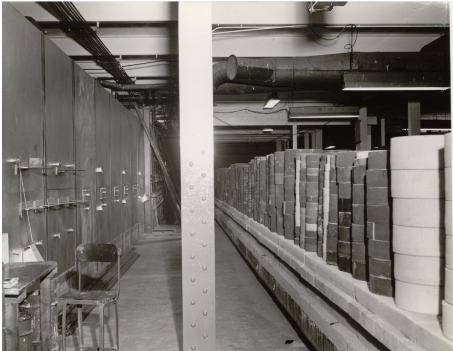
Figure 43: For a couple of years the old and new kilns sat side by side in the same building (Figure 39) This photograph taken around 1950 – 51 shows saggars for the bottle kilns sitting next to the side of the tunnel kiln on the left (source: Worcester Porcelain Museum).
