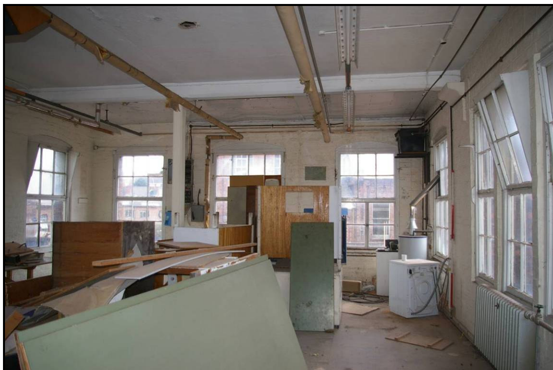
Figure 24: First floor, looking east
