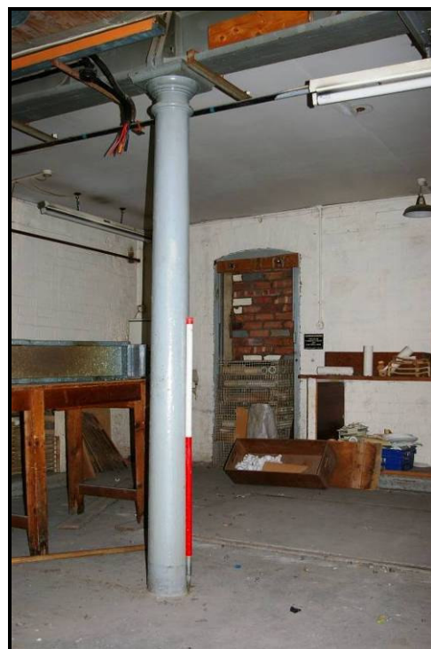
Figure 18: Cast iron column
