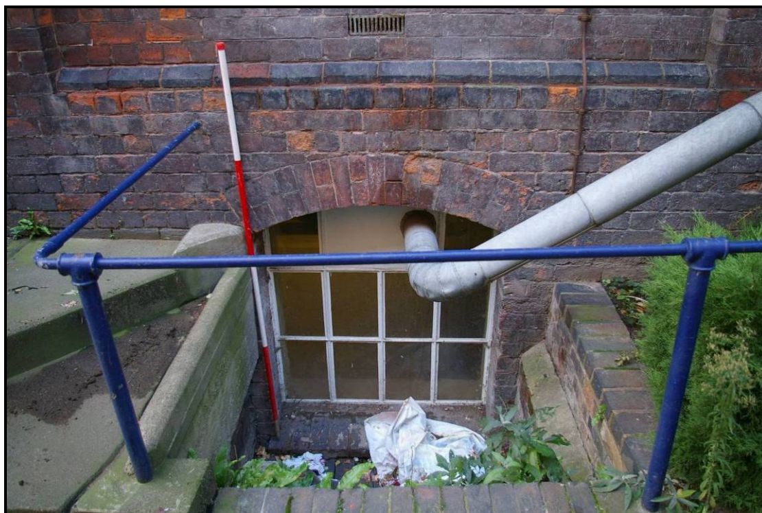
Figure 5: Basement window and light well
