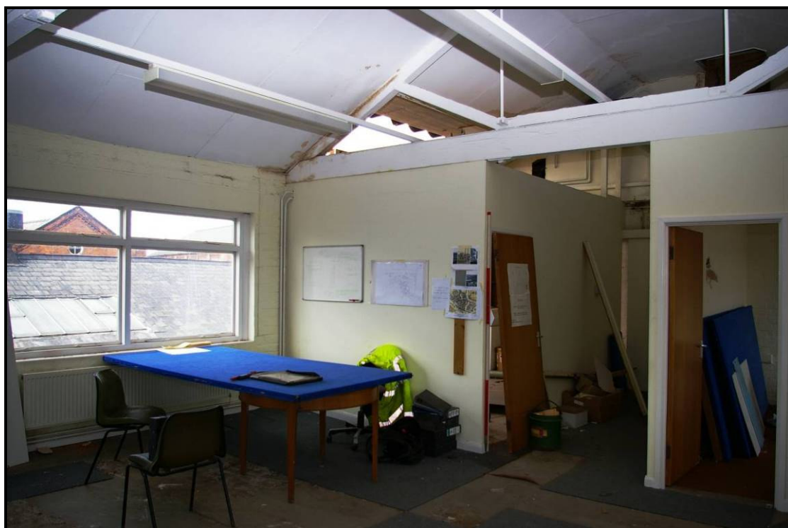
Figure 32: Second floor, looking south-west
