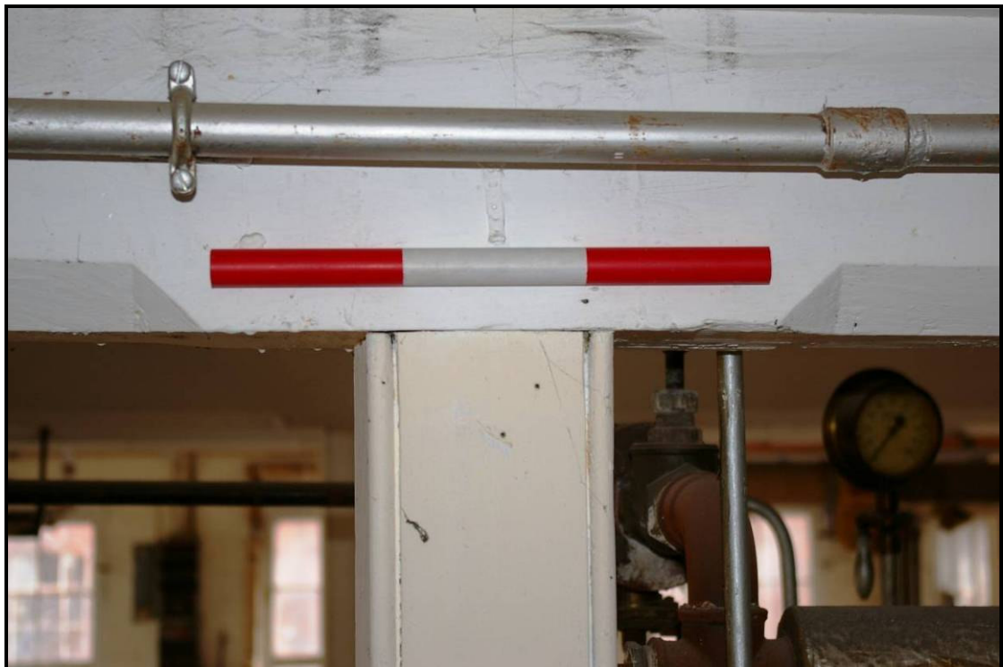
Figure 26: Detail of flat chamfer stop and vertical post with bead moulding
