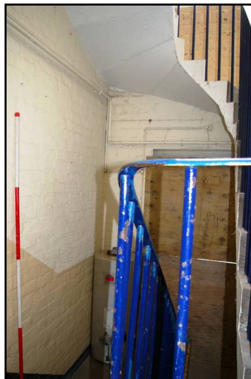
Figure 14: Cantilever staircase
