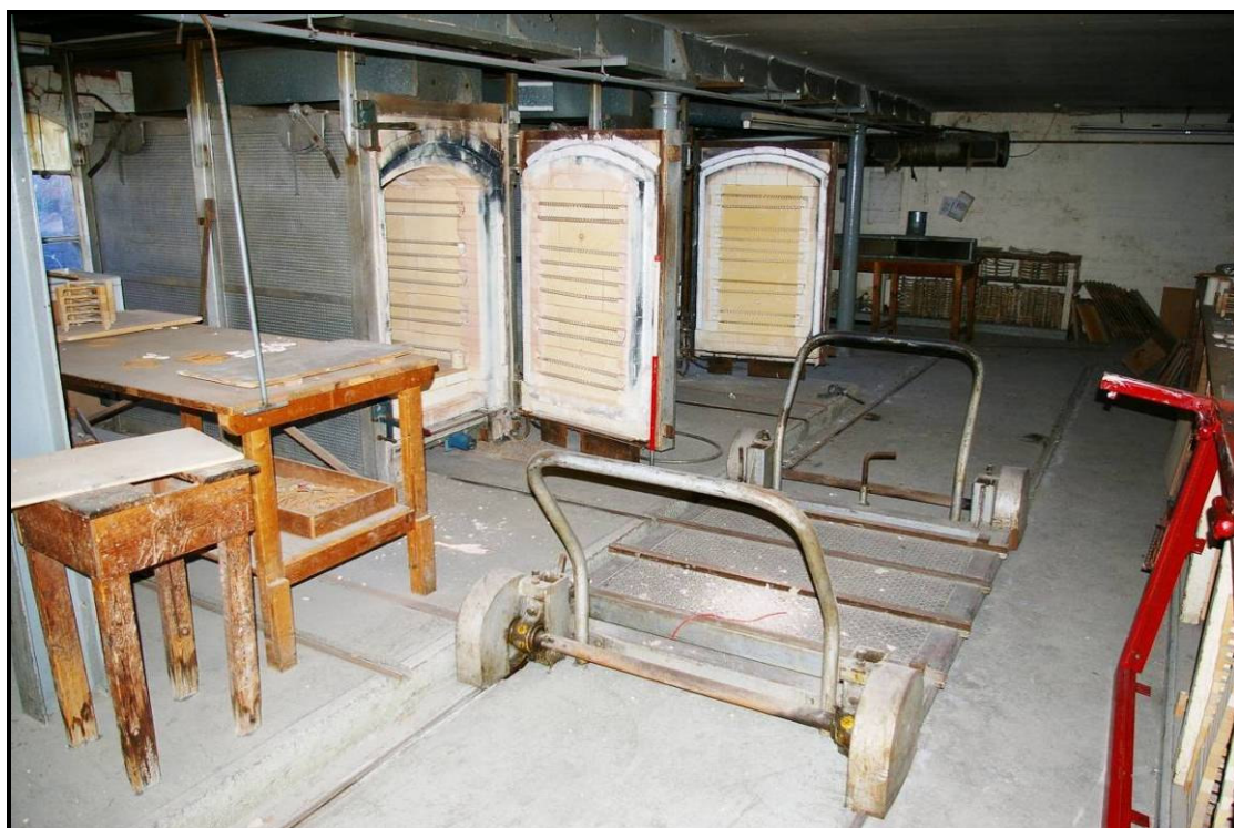
Figure 16: Kilns on the basement floor
