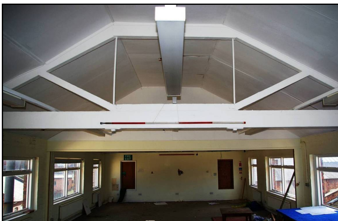
Figure 33: Example of roof truss
