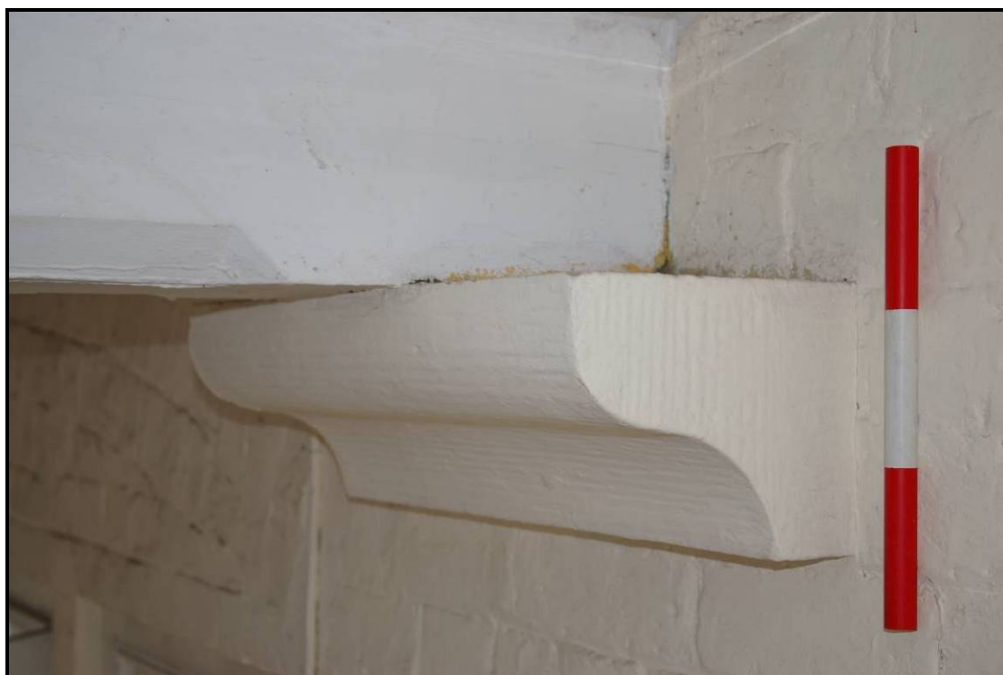
Figure 27: Limestone cyma reversa corbel
