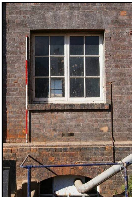
Figure 6: Ground floor window
