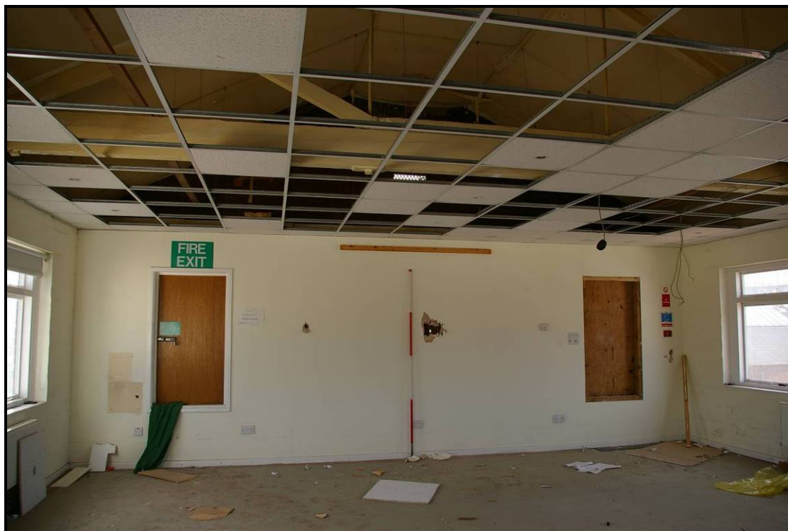
Figure 30: Second floor, looking east
