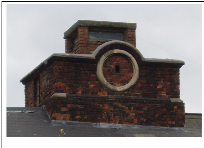
Figure 9: The chimney as modified into a lookout during WWII. The clock lay in the circular surround and probably served as the official factory timepiece
