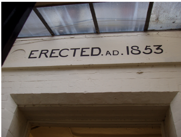
Figure 3: Painted and incised date applied above the entrance to Building J
