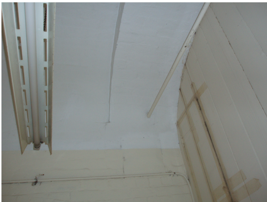
Figure 10: The vaulted ceiling beneath the chimney
