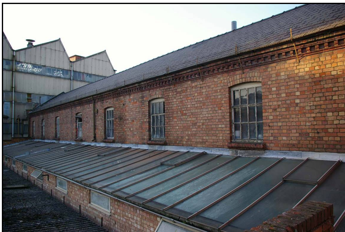
Figure 53: East elevation of K3, looking south
