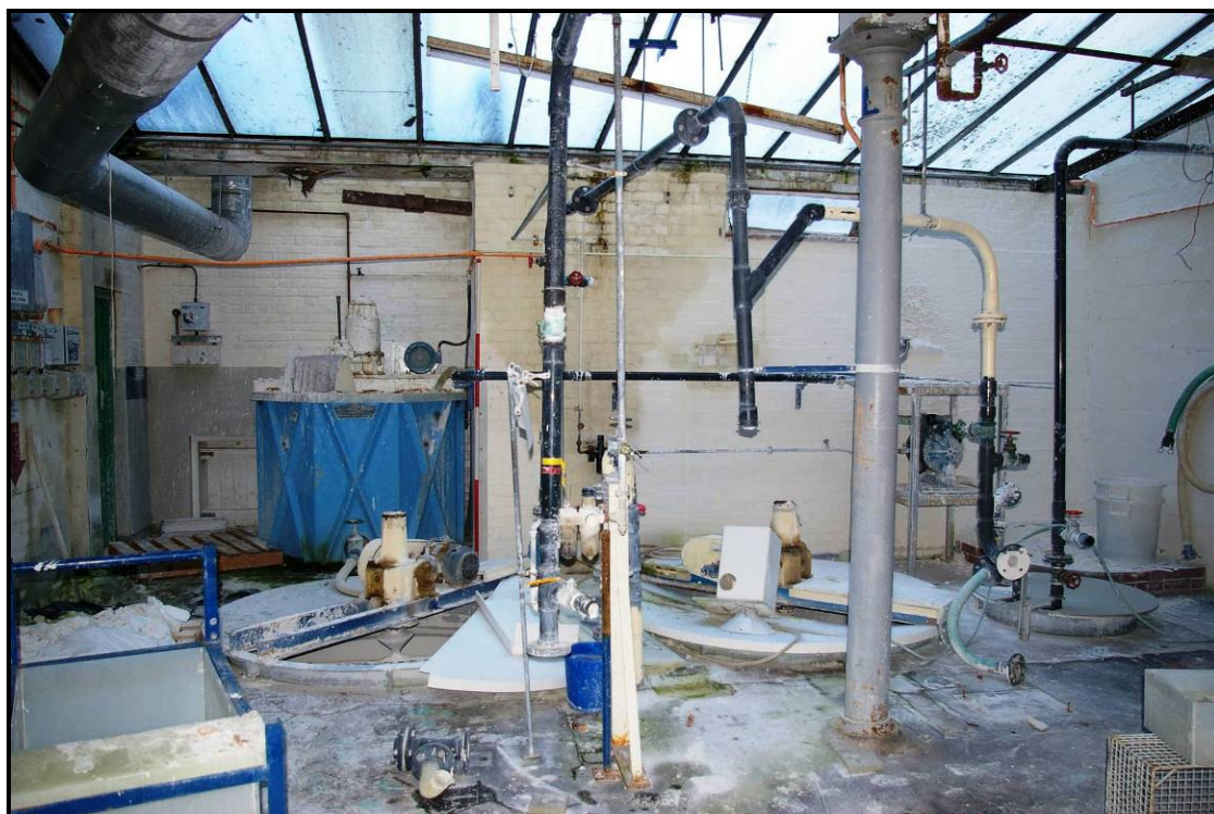
Figure 61: Underground arks in K3, looking east
