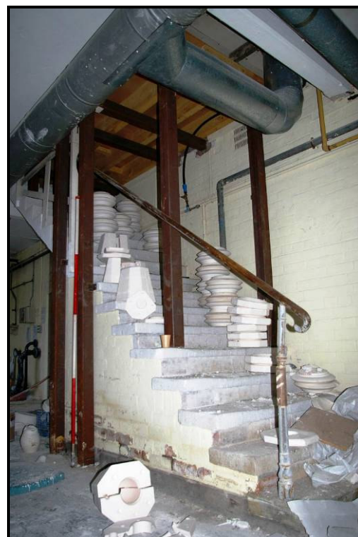
Figure 64: Staircase of K3
