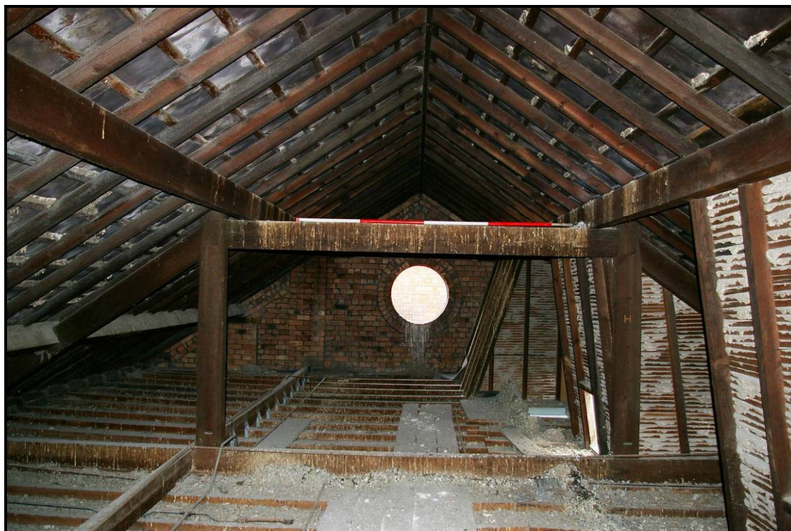
Figure 47: Queen-post timber truss on the northern end of K2
