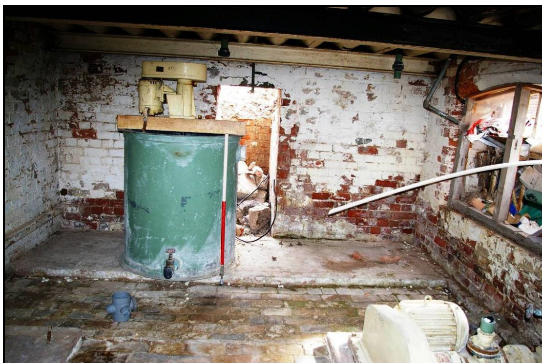
Figure 9: Basement floor, looking north
