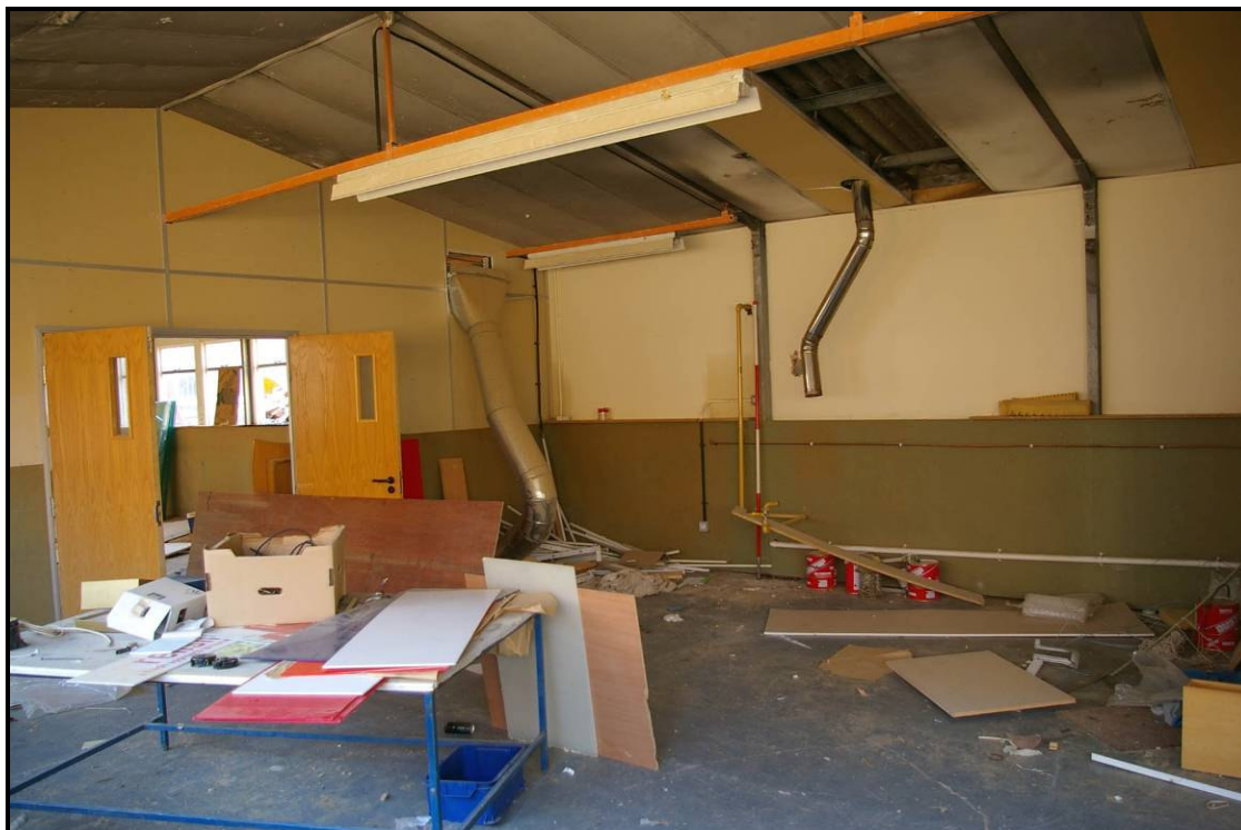
Figure 72: Eastern block, looking south
