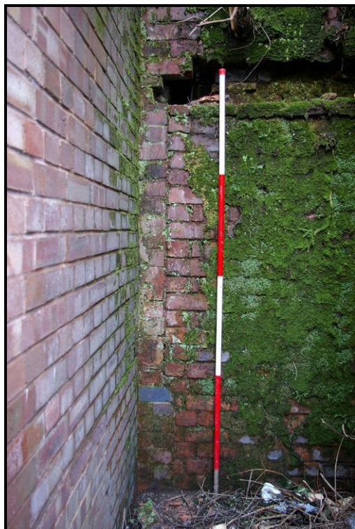
Figure 57: Pilaster of former wing
