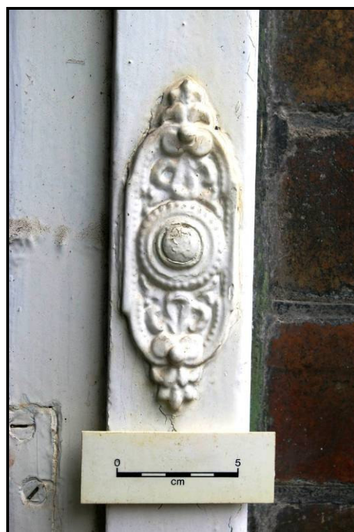
Figure 28: Detail of doorbell
