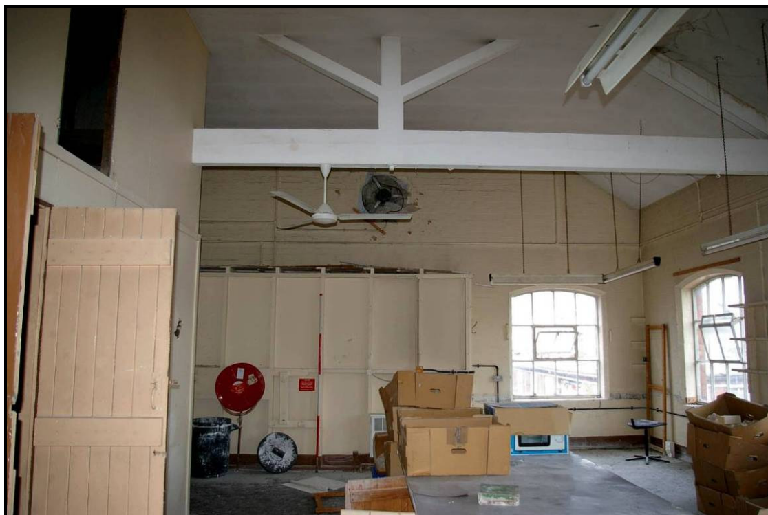
Figure 17: Second floor of K1, looking west
