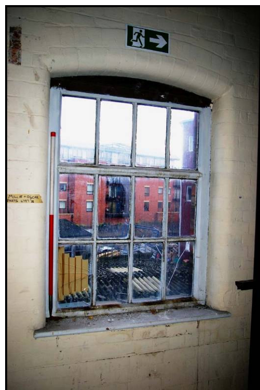
Figure 67: Detail of window
