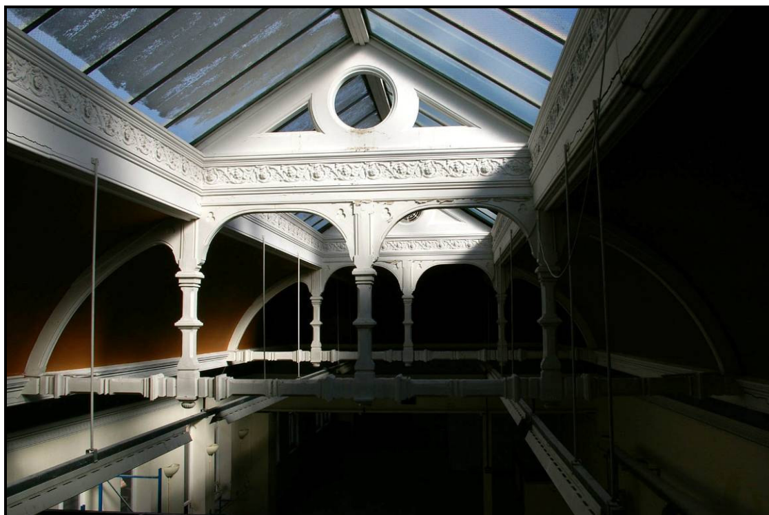
Figure 39: Decorated trusses of K2
