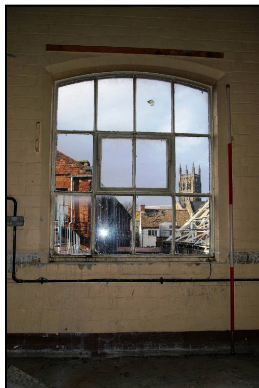
Figure 16: Window on the second floor of K1
