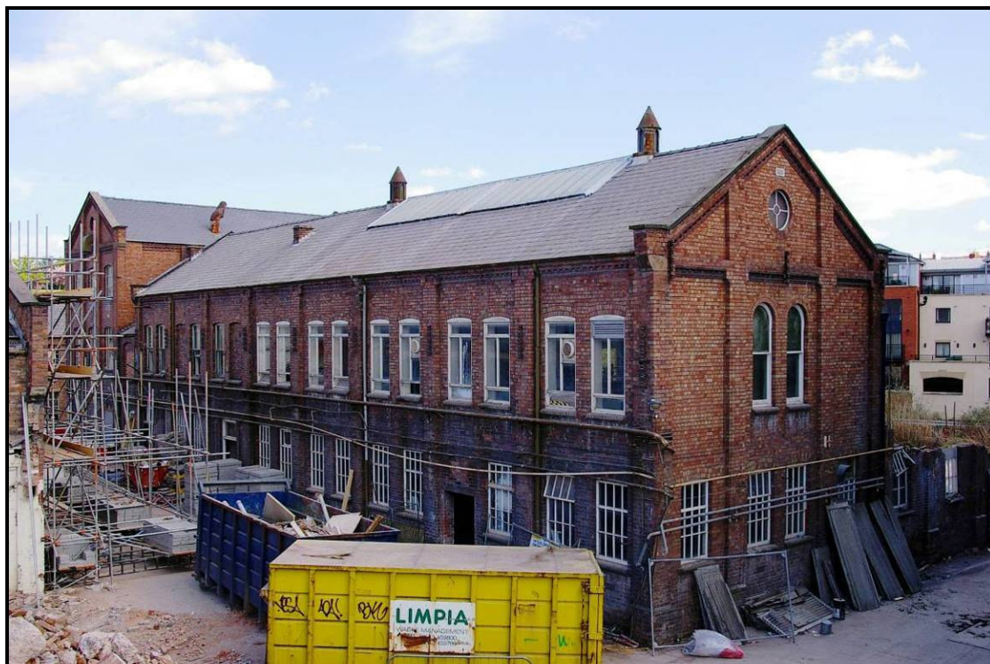
Figure 24: Building K2, looking north-east
