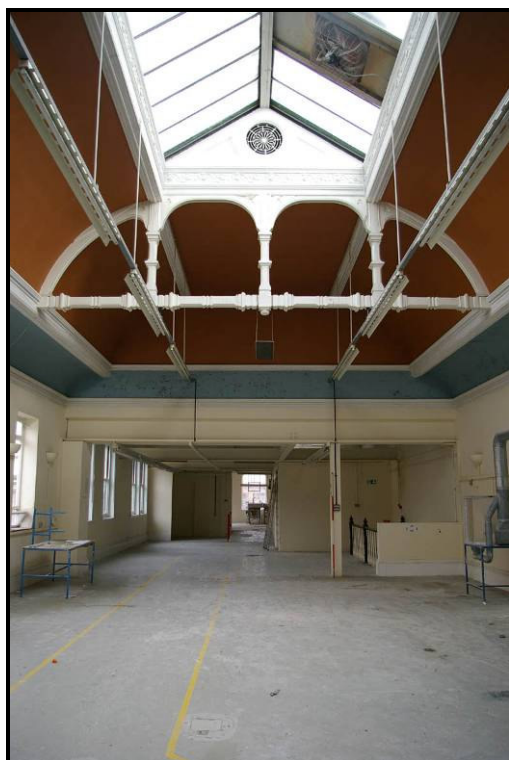
Figure 36: First floor of K2, looking north
