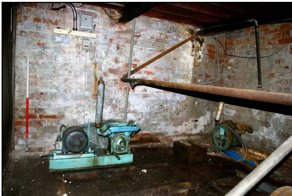
Figure 8: Basement floor with electric pump, looking east
