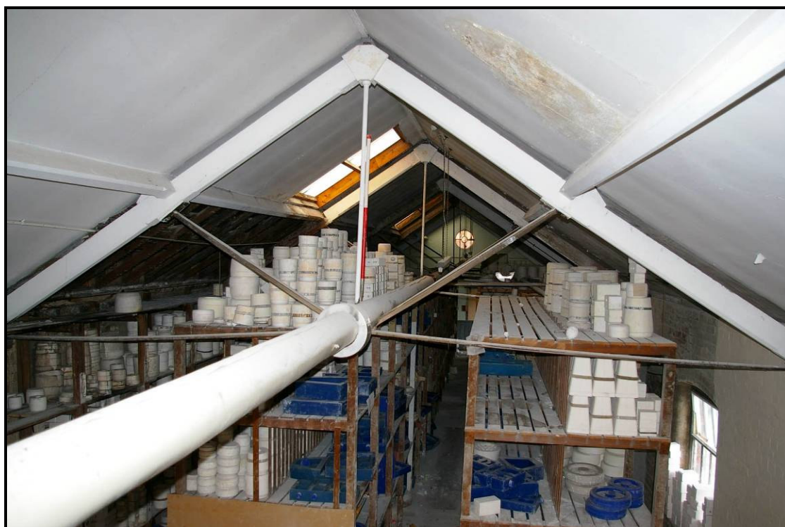
Figure 68: Composite truss on the first floor of K3, looking north
