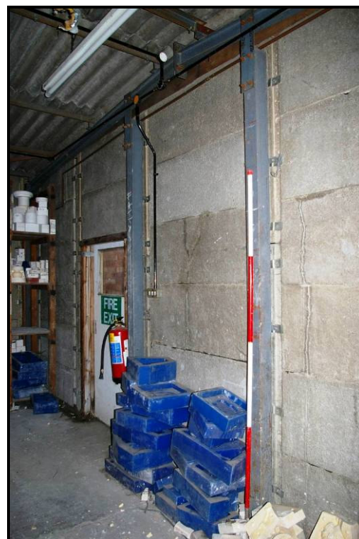
Figure 71: Fire escape of western block
