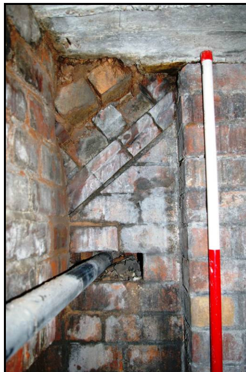
Figure 58: Surviving dentilled brickwork
