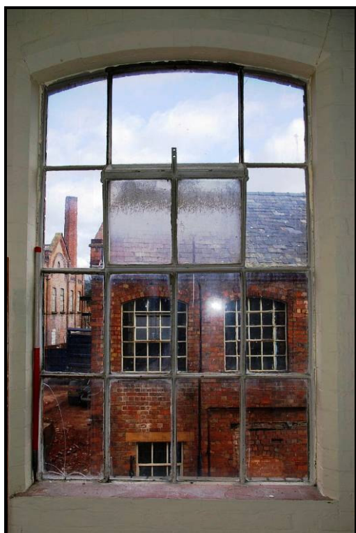
Figure 15: Window on the first floor of K1
