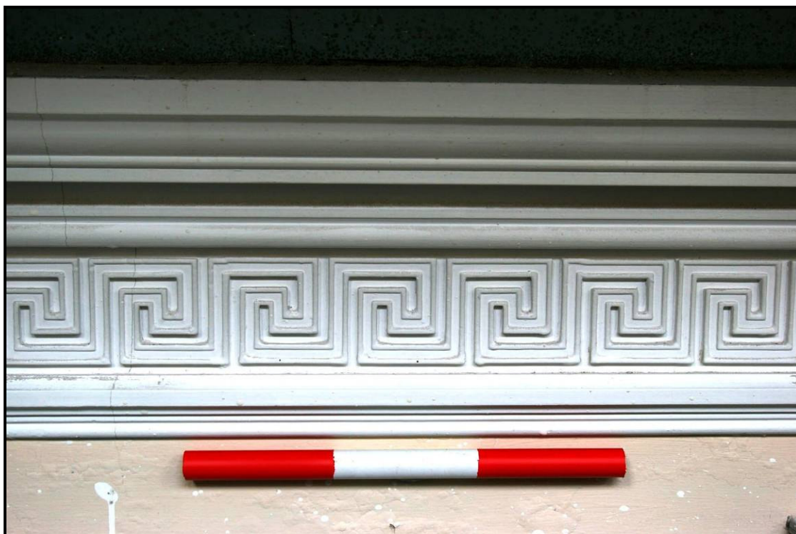
Figure 43: Detail of plastered cornice with a continuous key pattern decoration
