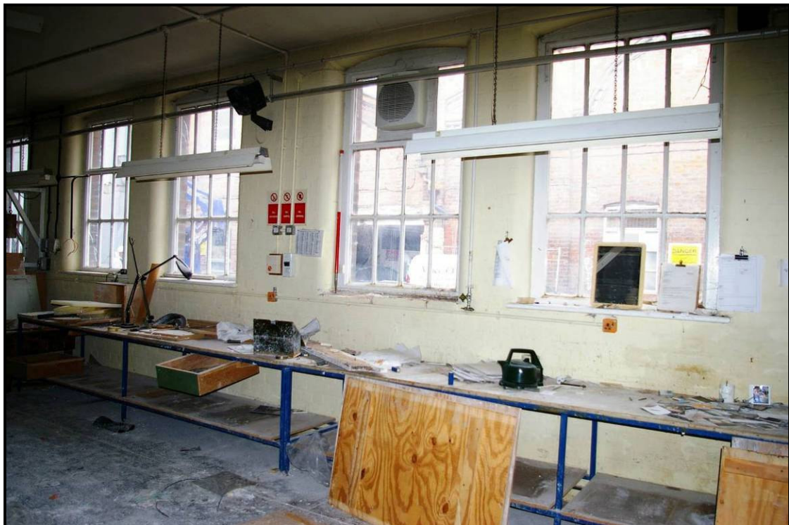
Figure 33: The Scouring Room of K2, looking south-west
