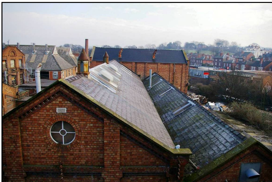
Figure 26: The roofs of K2 and K3, looking north
