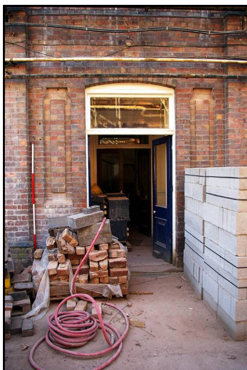
Figure 27: Main entrance of K2
