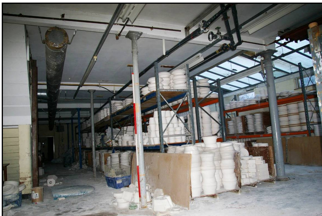
Figure 62: Ground floor of K3, looking north
