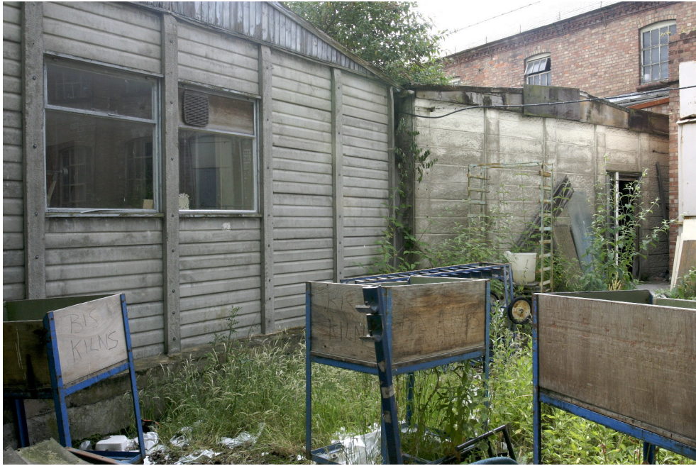
Figure 40: The north elevations of the Banbury Buildings
