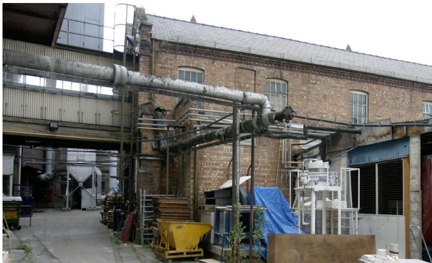
Figure 28: The bridge from Building K3 (right) to Building W1
