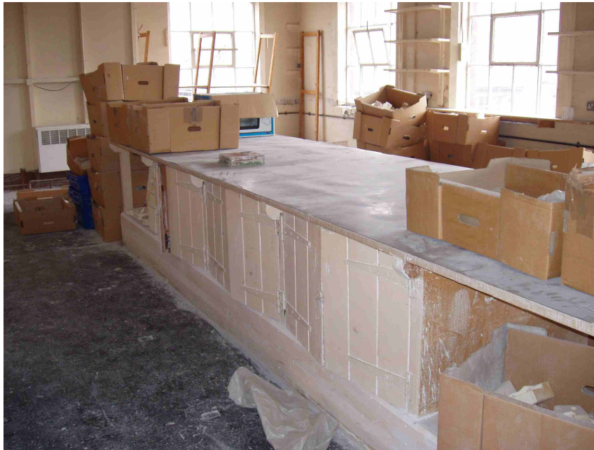
Figure 15: The second floor of Building K1
