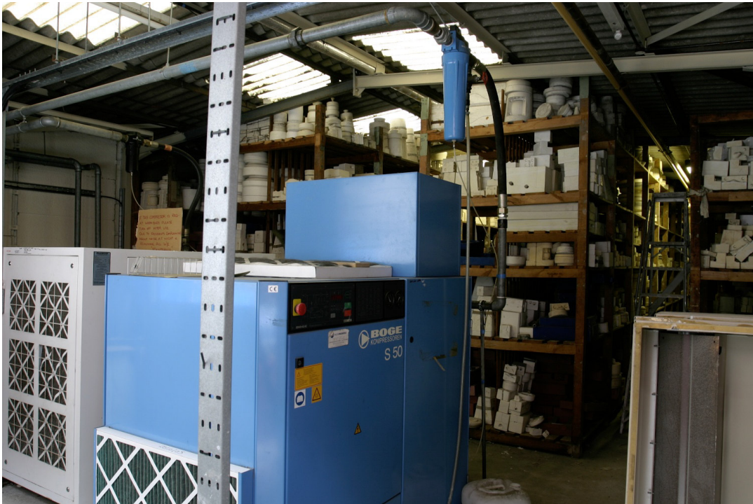
Figure 42: Looking south inside the 1966 Banbury Building of 1973
