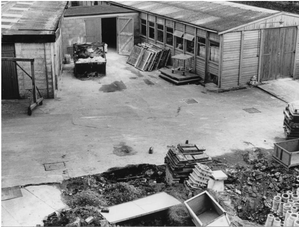
Figure 38: The Banbury Buildings. The 1966 'Superspan' lies to the left with the 1973 one right
