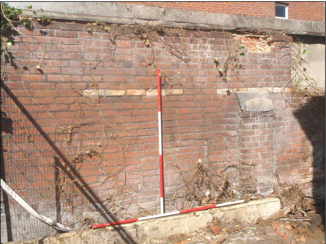
Plate 2: Western boundary wall of site, looking south-west
