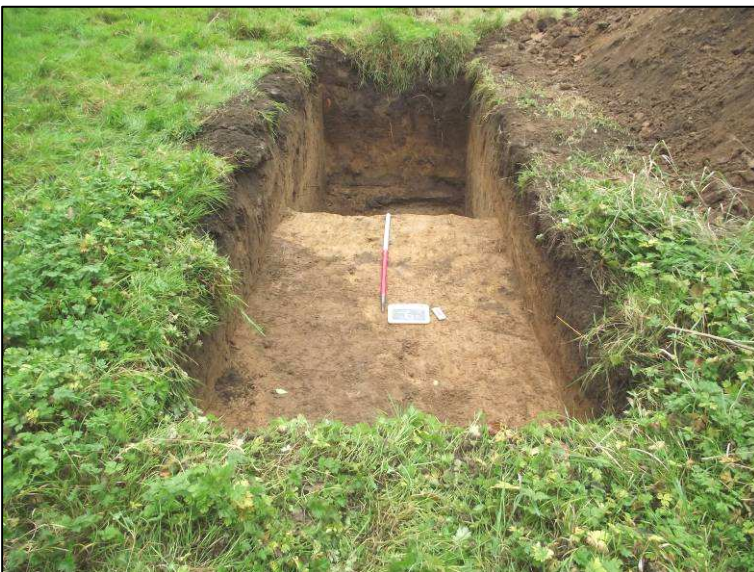
Plate 3: Trench 3 following machine excavation, looking north-north-east
