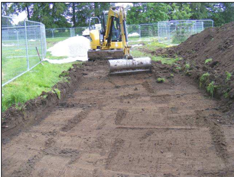
Plate 3: Soil stripping at site entrance, looking north
