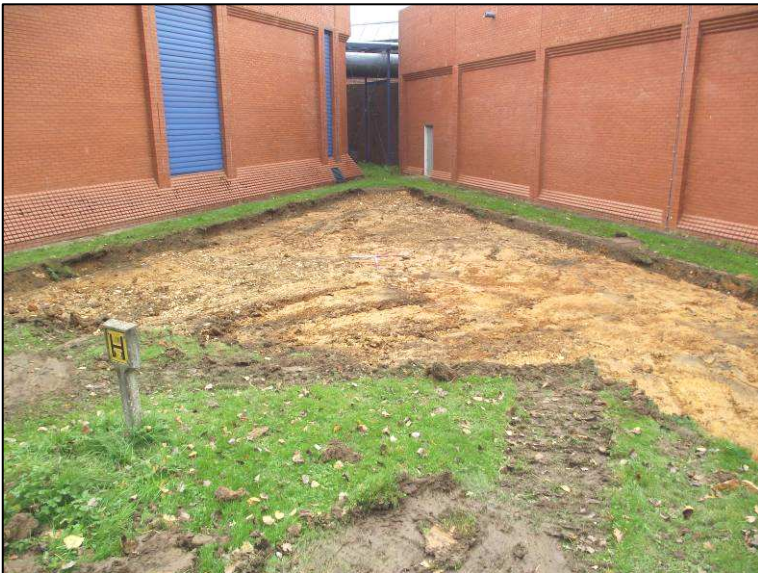
Plate 2: View of the stripped area, looking north
