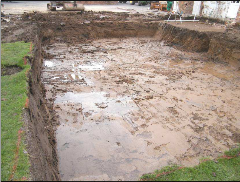
Plate 1: General site shot of excavated area, looking north-west
