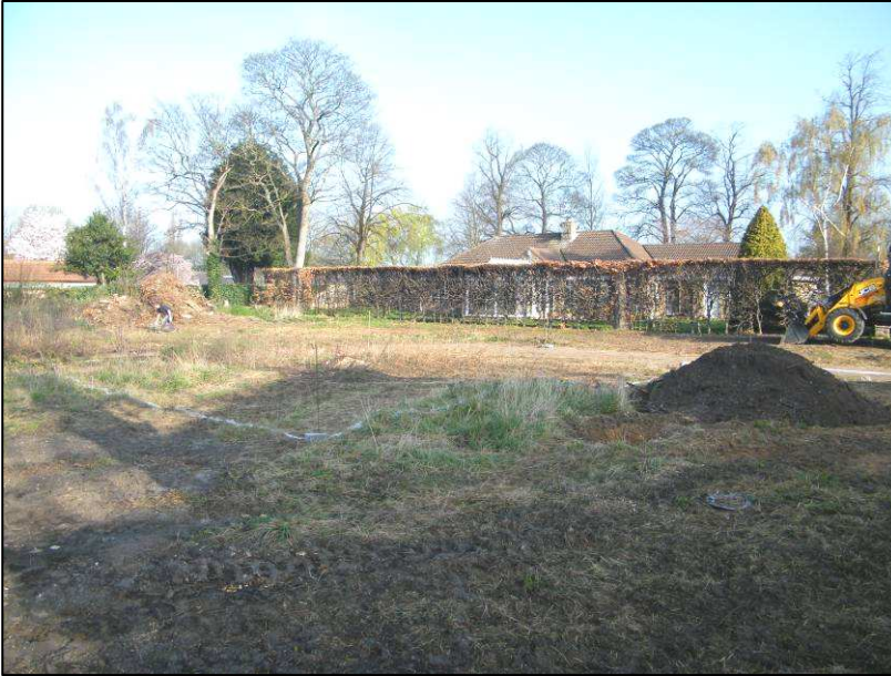
Plate 1: General view of the development area, looking north-west from the south-east corner of the site
