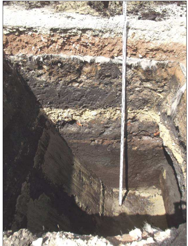
Plate 3: Test Pit 2 following excavation, showing east facing section and looking west. Measuring staff to top of trench is 4m high
