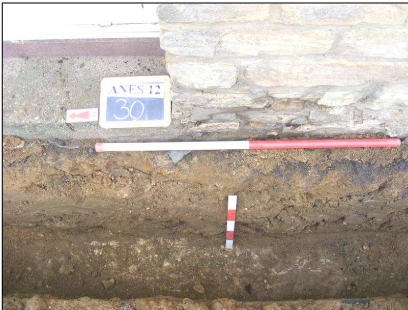
Plate 11: Section 5.5 showing structure 38 and surface 39, looking east-southeast. Scales are 1m and 0.5m
