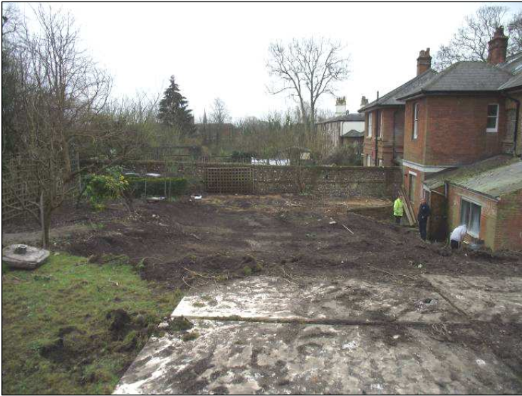
Plate 1: Overall view of the site following removal of the garden topsoil. Looking south-east
