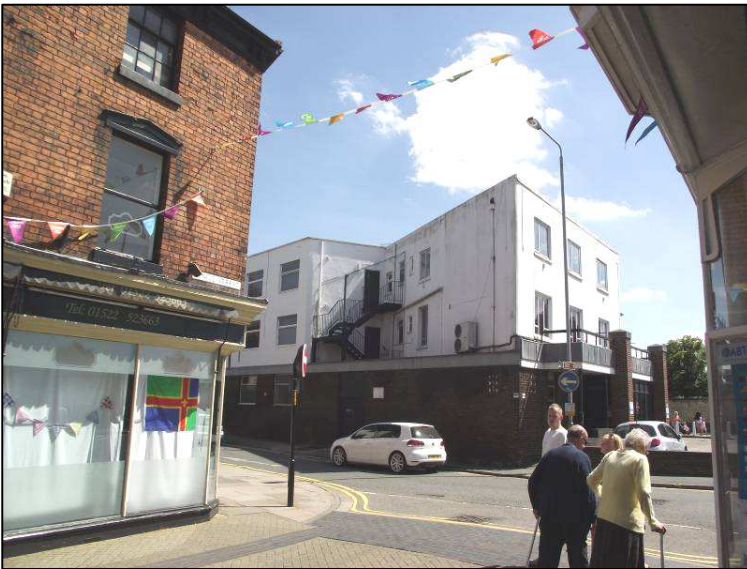
Plate 2 (Shot 80): East and north elevations, looking southeast
