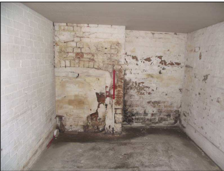
Plate 11 (Shot 56): Bricked up fireplace partially obscured by later partition, looking north-northeast. Scale is 1m
