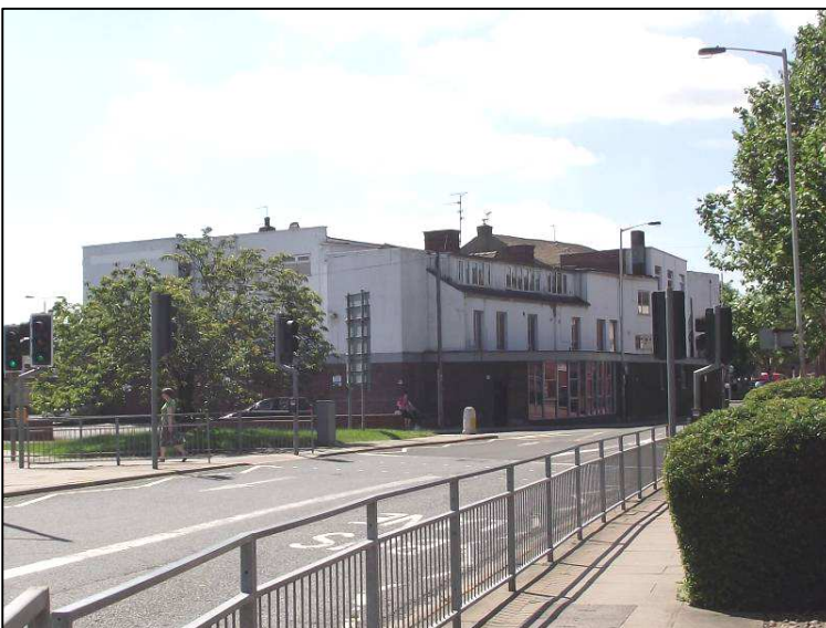
Plate 3 (Shot 81): North and west elevations, looking west-southwest
