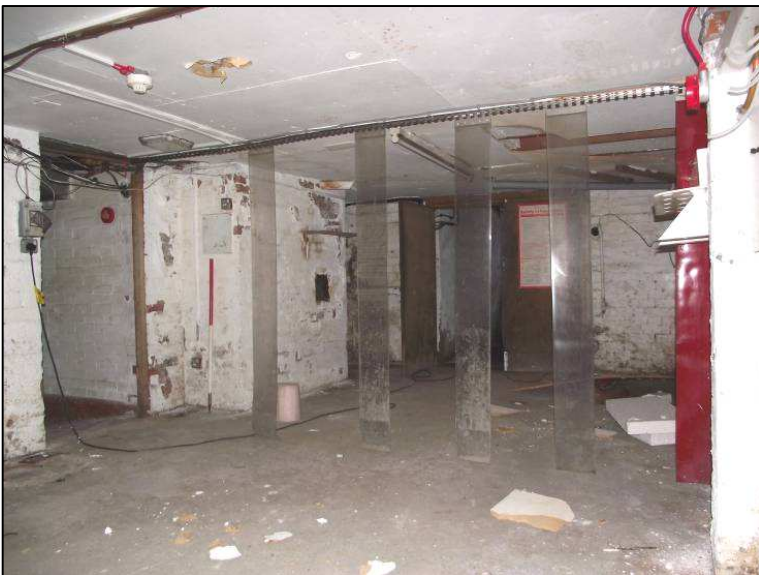
Plate 9 (Shot 45): Basement under the Buttery Bar, looking south-southeast. Scale is 1m
