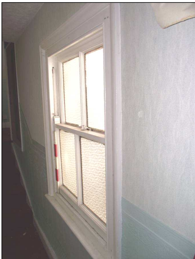
Plate 22 (Shot 30): Sash window on first floor, looking west-southwest. Scale is 0.5m
