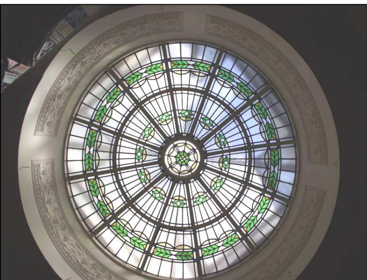
Plate 18 (Shot 37): Domed roof light in dining room
