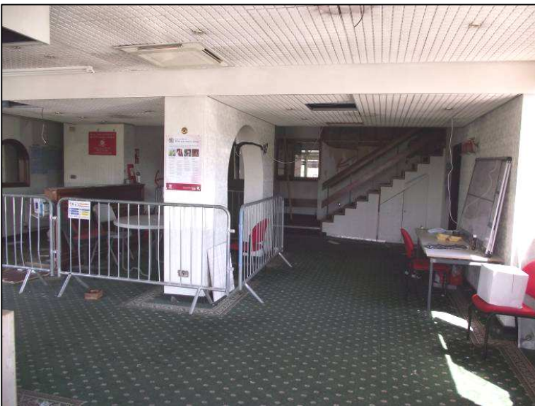
Plate 15 (Shot 32): Modern foyer with reception to the left and main access to first floor in the background, looking north-northwest
