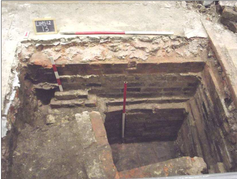
Plate 2: Trench 1 looking north, showing cellar walls 108 and 109. Scales are 1m and 0.5m
