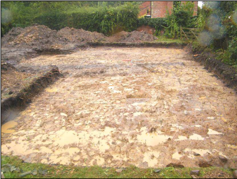
Plate 1: General site shot, looking southeast. Scales are 1m
