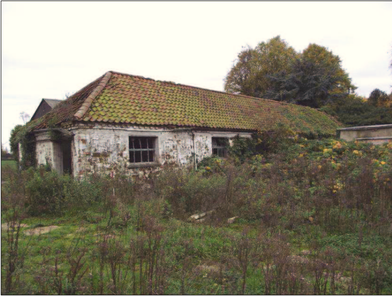
Plate 10 (Shot 11): Barn 2 looking southwest. Scale is 1m
