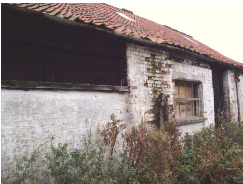
Plate 6 (Shot 42): North end of west elevation of Barn 1, looking southwest
