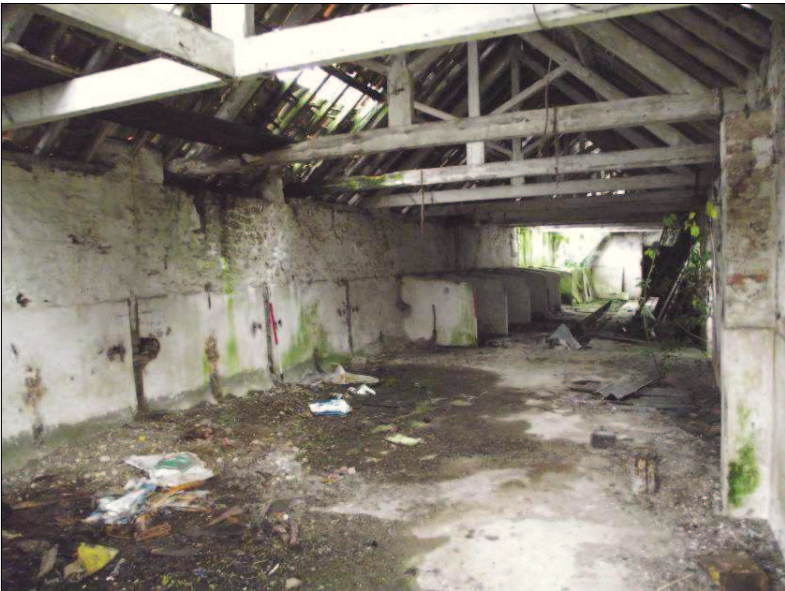
Plate 14 (Shot 17): Interior of Barn 2, looking west. Scales are 1m
