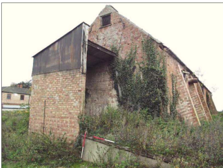
Plate 3 (Shot 6): South elevation of Barn 1 showing later outbuilding. Scales are 1m
