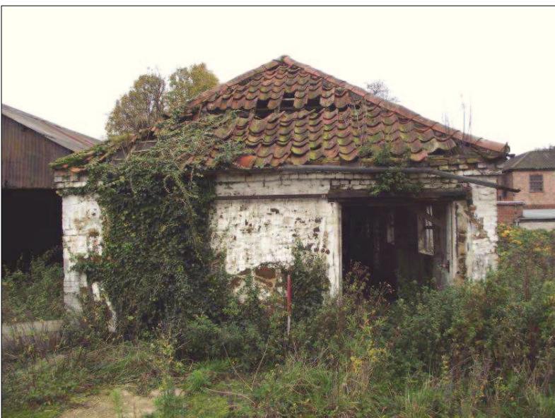
Plate 12 (Shot 61): East elevation of Barn 2, looking west-southwest. Scale is 1m
