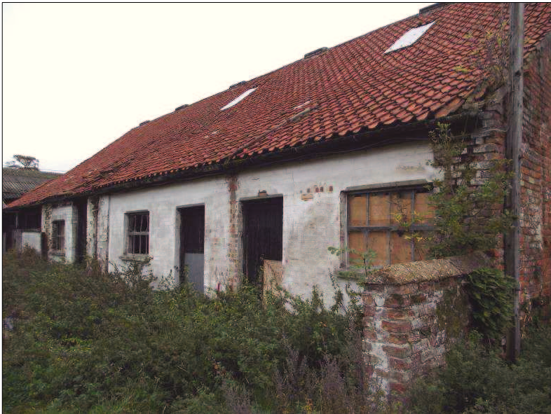
Plate 5 (Shot 9): West elevation of Barn 1, looking northeast
