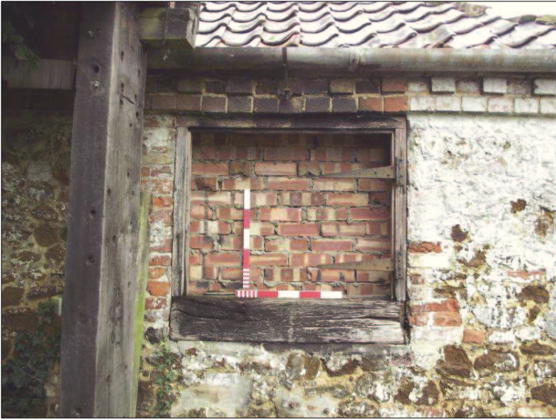
Plate 13 (Shot 44): Blocked window in south elevation of Barn 2, looking north-northwest. Scales are 0.5m
