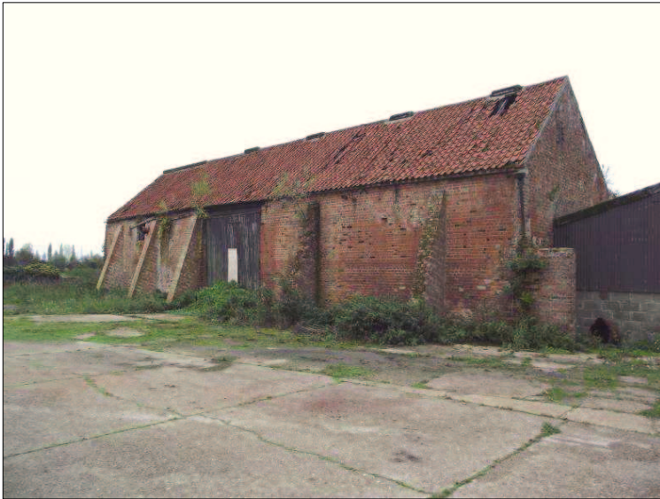
Plate 1 (Shot 1): East elevation of Barn 1, looking southwest
