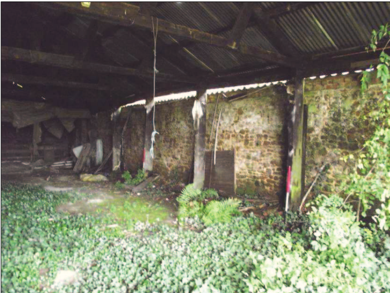
Plate 17 (Shot 32): Interior of 20 th century barn on the south elevation, showing ironstone wall of Barn 2. Looking west. Scale is 1m
