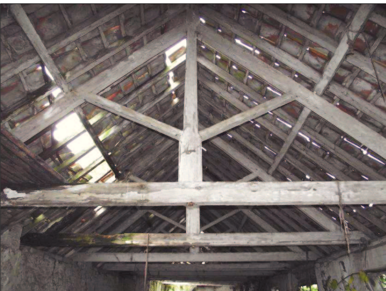
Plate 15 (Shot 22): Roof structure of Barn 2, looking west-southwest
