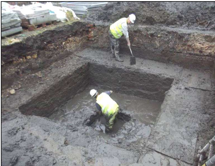
Plate 2: Trench 1 under excavation, looking southwest
