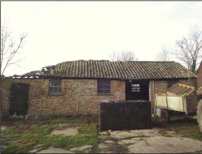
Plate 22 (Shot 32): East elevation of Outbuildings 3 and 4, looking west. Scale is 1m
