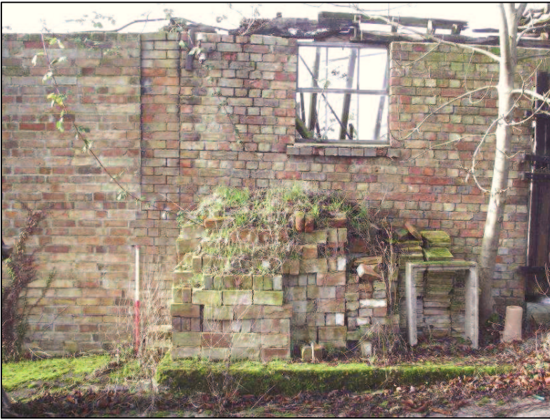
Plate 19 (Shot 30): East elevation of Outbuildings 2 and 3, looking west. Scale is 1m
