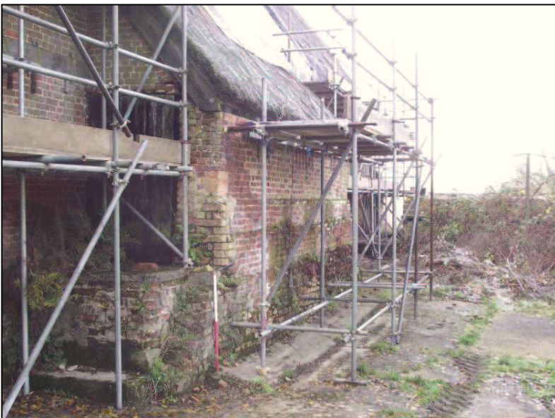
Plate 6 (Shot 24): Close up of outshut, looking southwest. Scale is 1m
