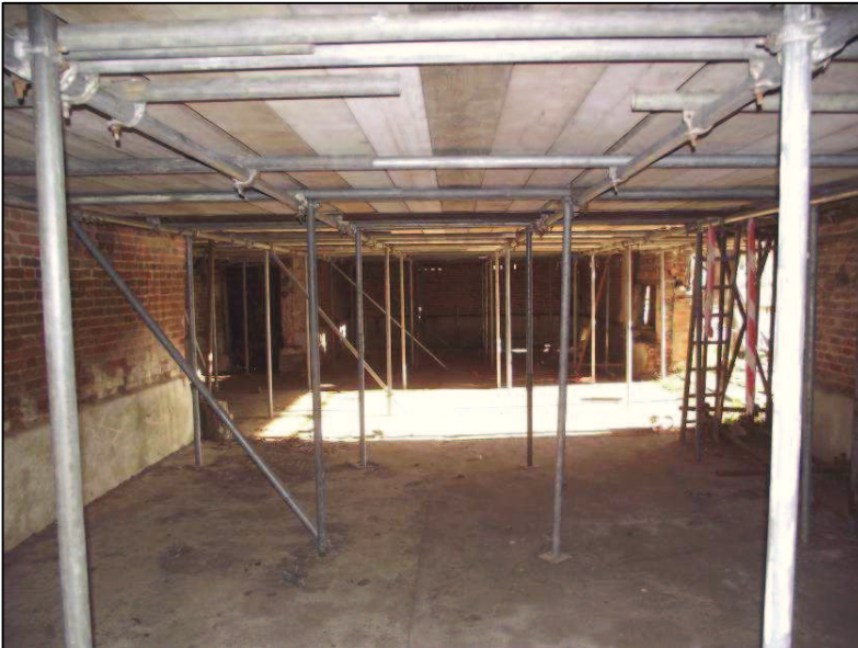
Plate 8 (Shot 7): Interior view of the barn, looking east
