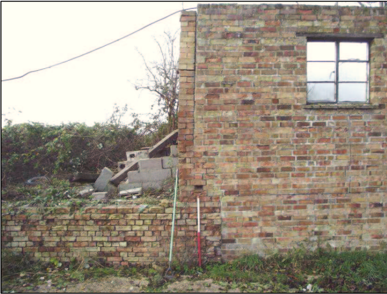
Plate 16 (Shot 26): East elevation and join between Outbuilding 1 and 2, looking west
