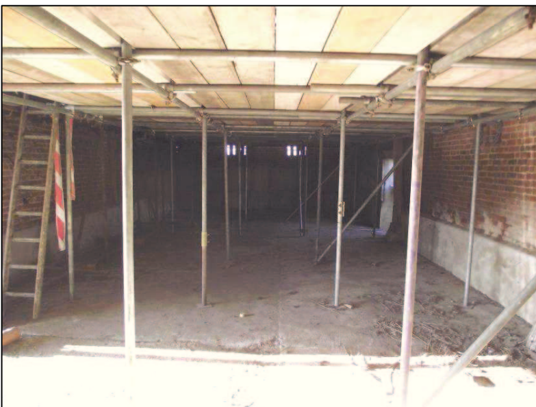
Plate 9 (Shot 9): Interior view of the barn, looking west
