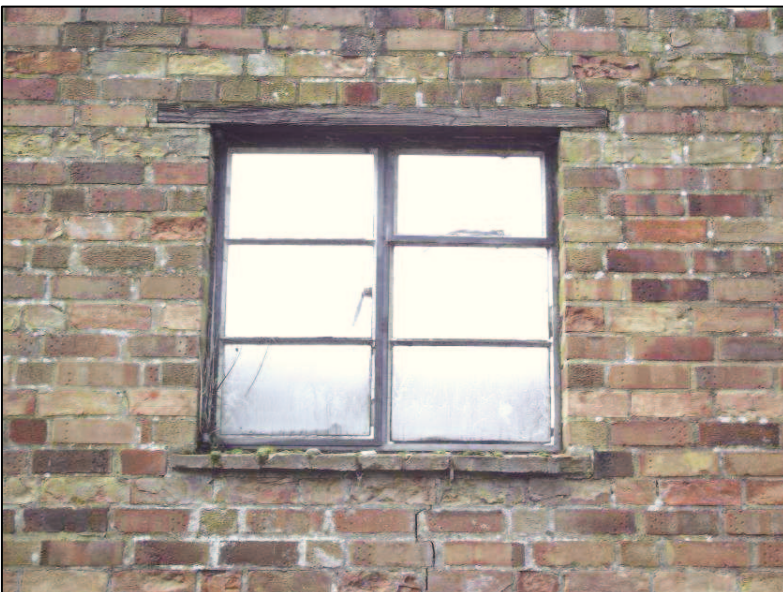
Plate 18 (Shot 28): Representative window on east elevation of Outbuilding 2, looking west
