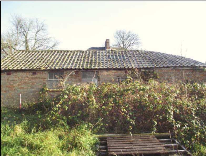
Plate 23 (Shot 41): West elevation of Outbuildings 3 and 4, looking east. Scale is 1m
