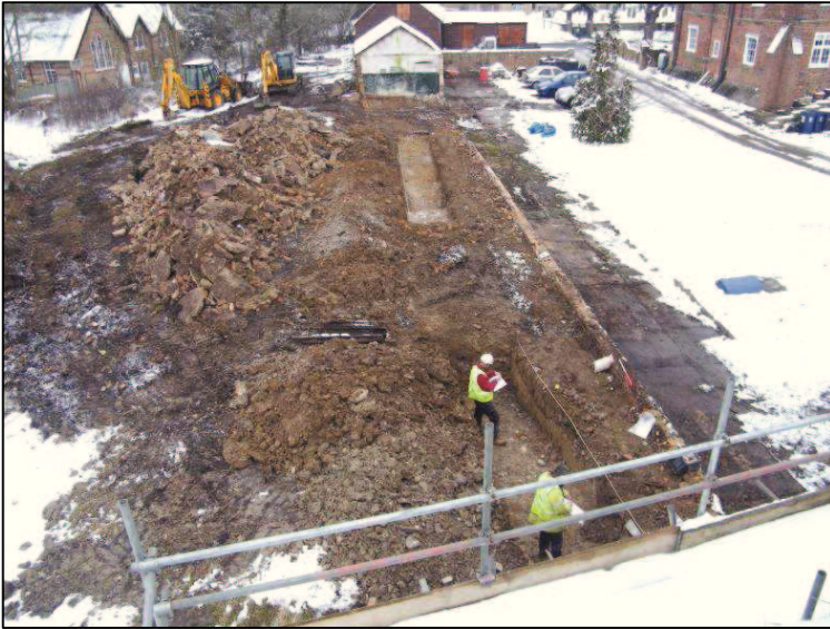
Plate 1: General view of the site with Trench 1 in the foreground and Trench 2 in the background, looking north
