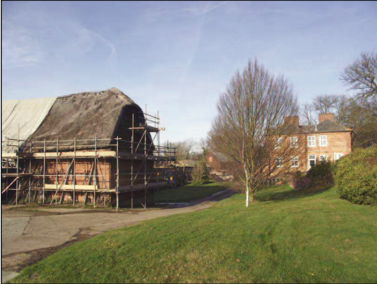
Plate 1 (Shot 46): General view of site, looking northwest
