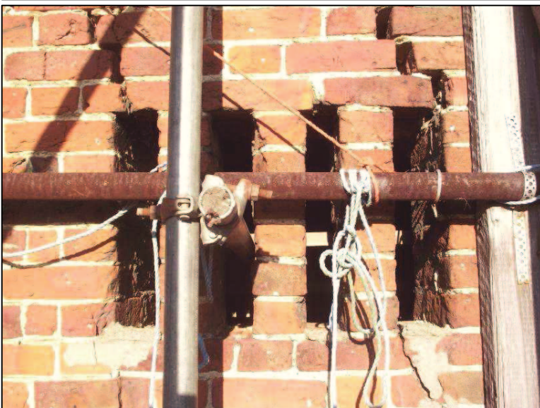
Plate 3 (Shot 2): Representative shot of the barn's ventilation slits (here on the south elevation), looking north
