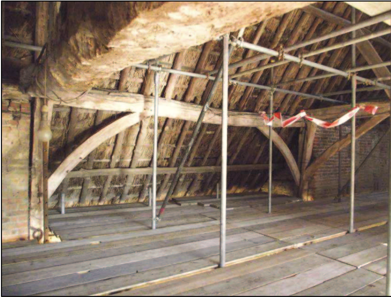
Plate 13 (Shot 17): Arched braces and tie beams and posts, looking northeast
