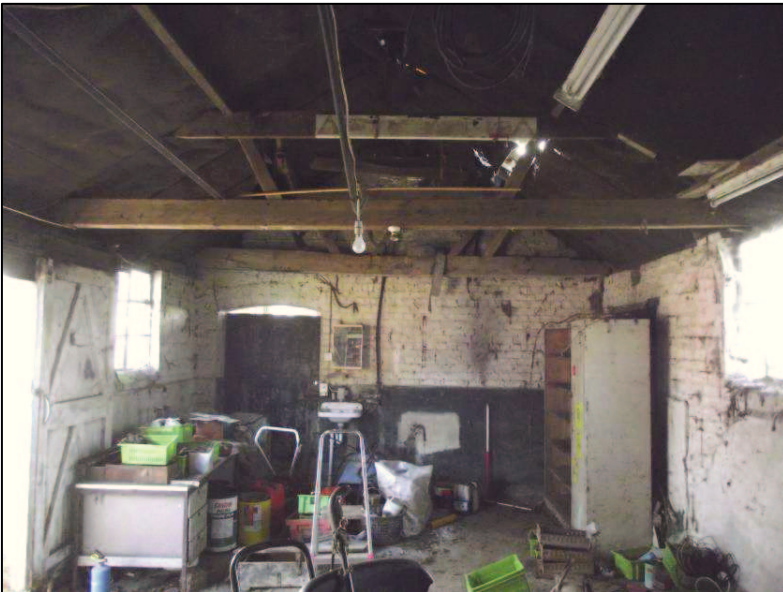
Plate 24 (Shot 33): Interior view of Outbuilding 4, looking south. Scale is 1m
