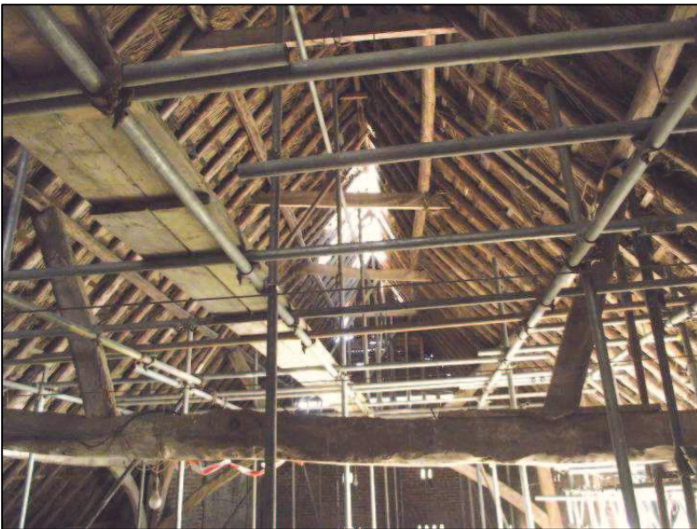
Plate 11 (Shot 15): Roof truss structure with ridge and trenched purlins, looking east
