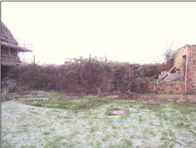
Plate 15 (Shot 25): Overgrown remnants of Outbuilding 1 east elevation, looking west. Scale is 1m
